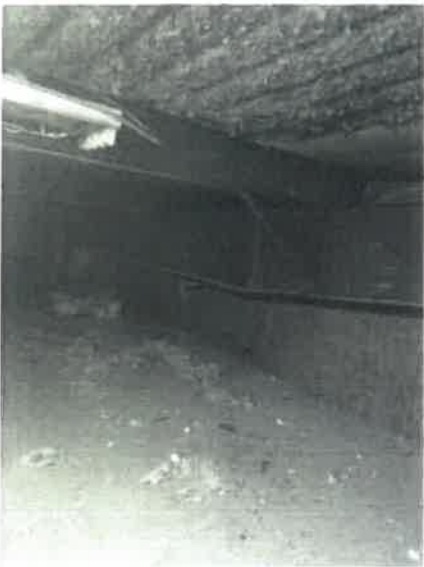
IMAGES 2 & 3 - SPRAY ON CELLULOSE INSULATION
