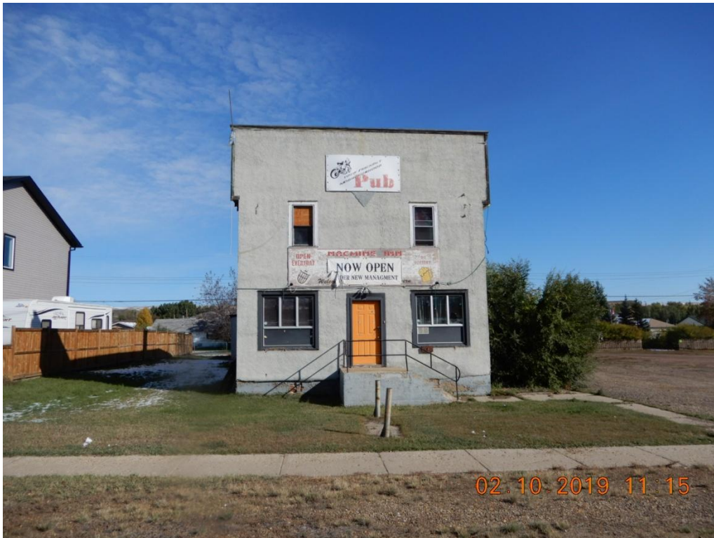
Figure 1 South wall (building front)
