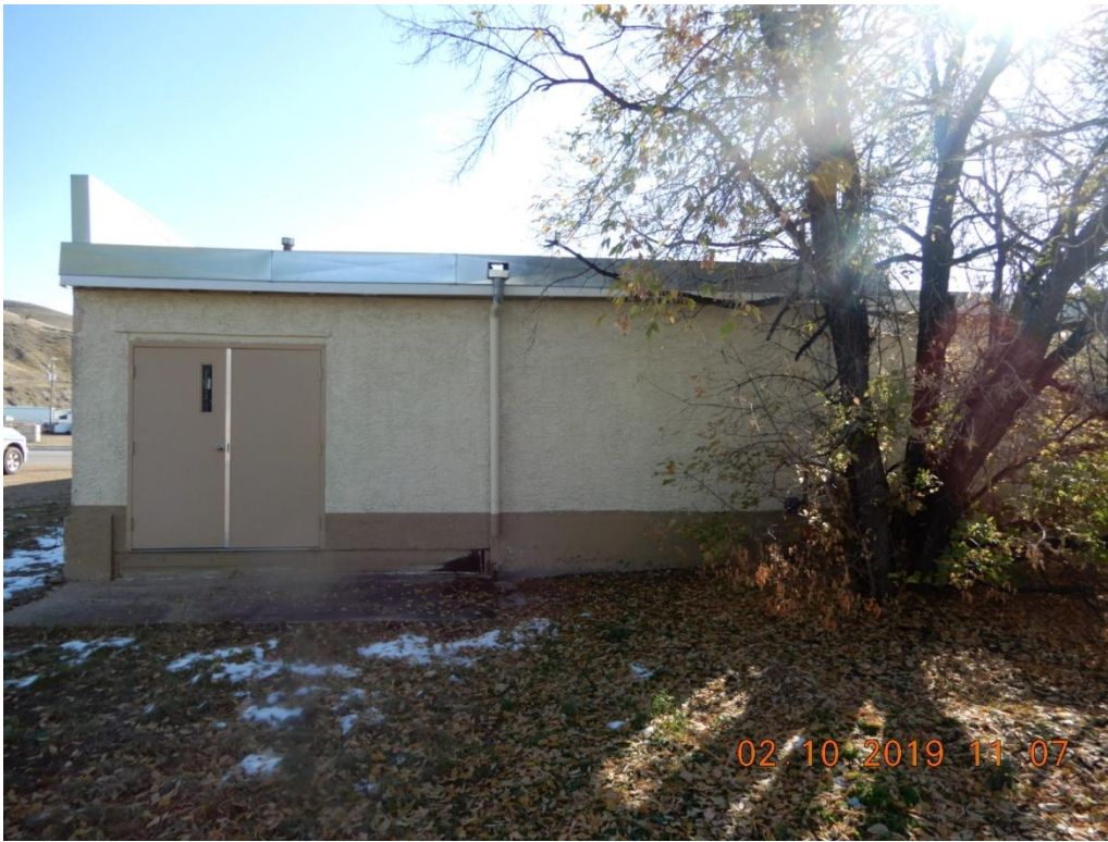
Figure 7 West wall (at alley)
