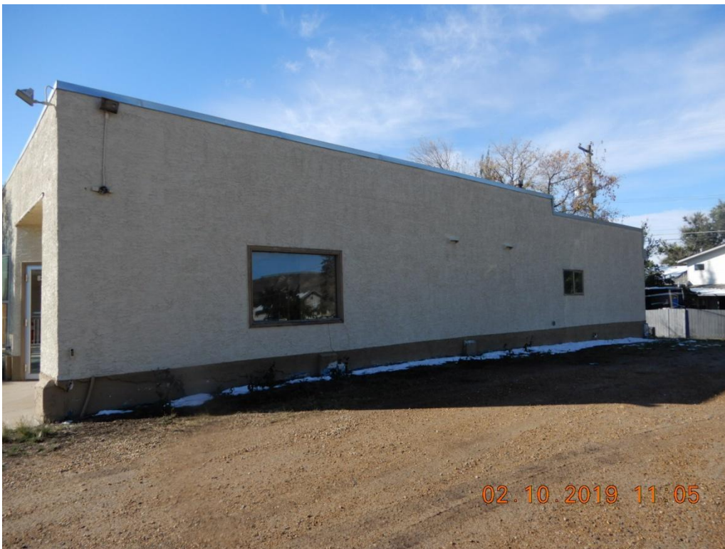
Figure 6 North wall (parking lot adjacent)
