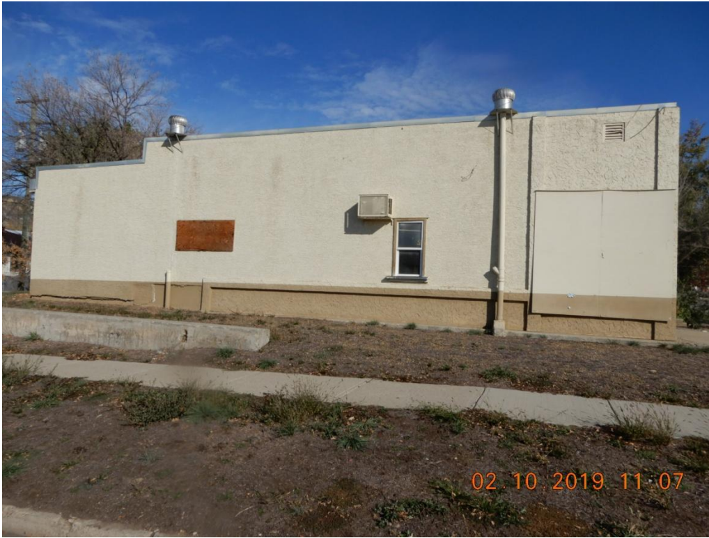
Figure 8 South wall (adjacent street)
