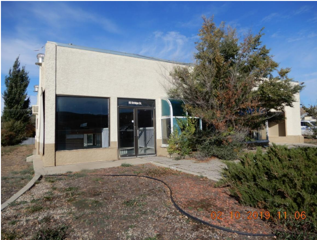
Figure 5 East Wall (building front)
