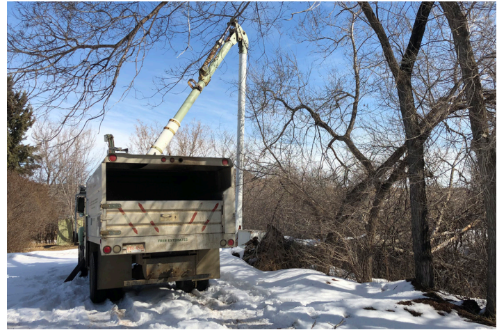
Drainage ditch clearing of fallen tree debris to facilitate inspection
