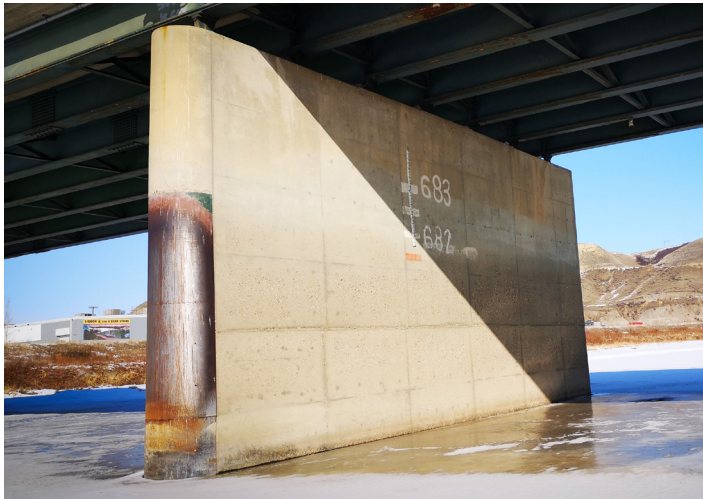
Gordon Taylor Bridge February 2020
