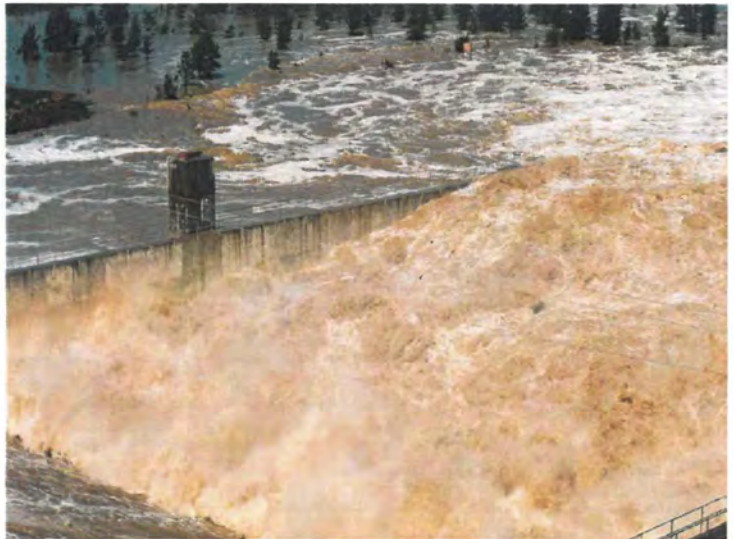
Dickson Dam Service Spillway Chute & Stilling Basin
