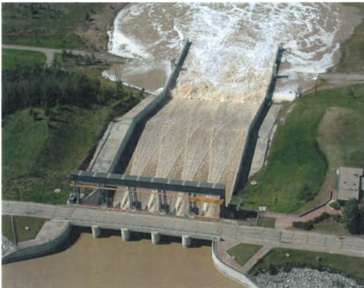
Dickson Dam Service Spillway Aerial View
