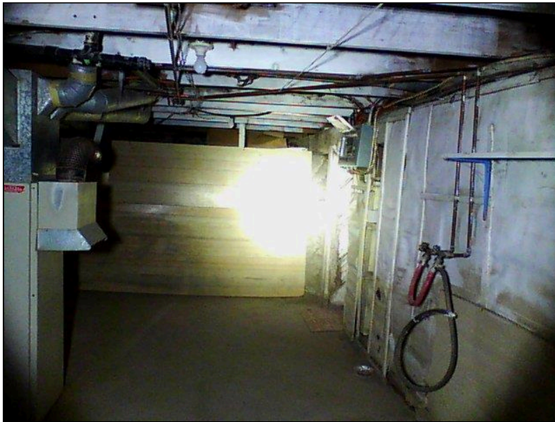
7.0 Item 4(Picture) Basement Foundation
