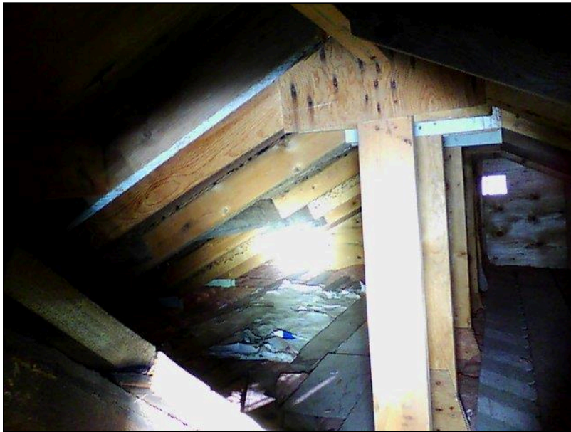
2.0 Item 4(Picture) Attic
