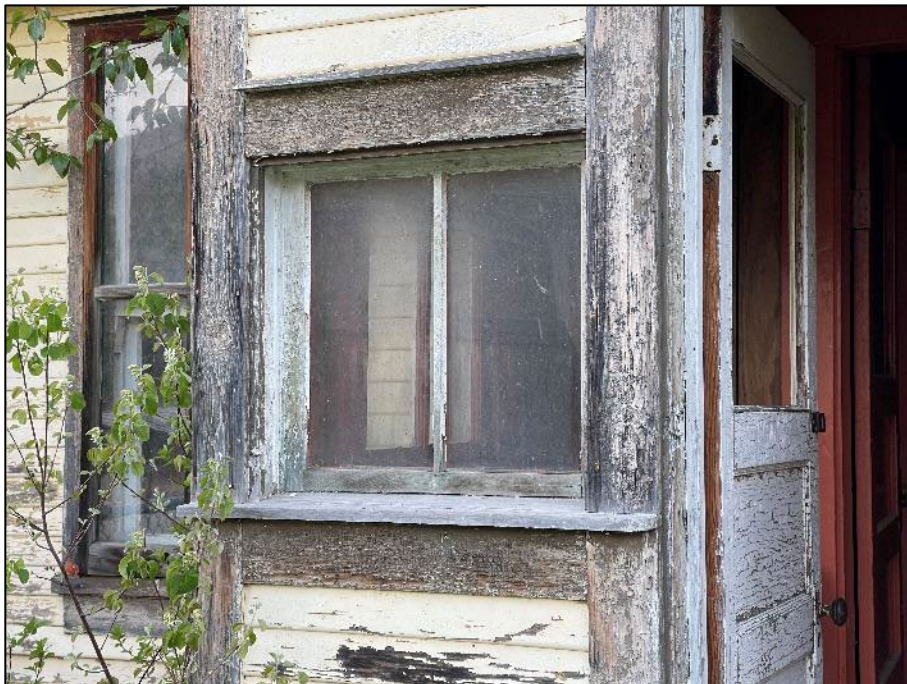
PHOTOGRAPH #26: Window Caulking - Small House (Non-Asbestos)
