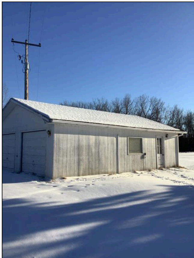
4.0 Item 1(Picture) Garage Roof
