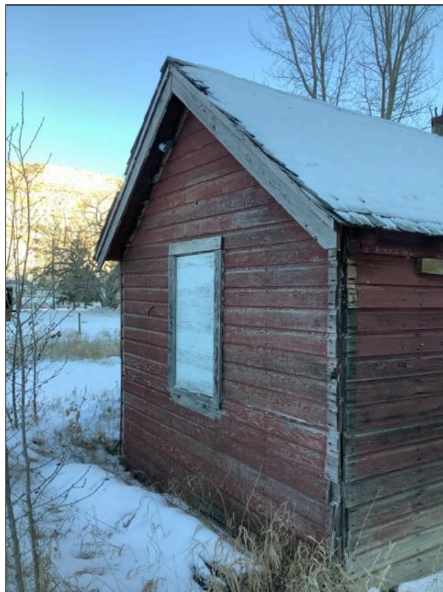
3.1 Item 14(Picture) Outbuilding - aged, structure demo recommended
