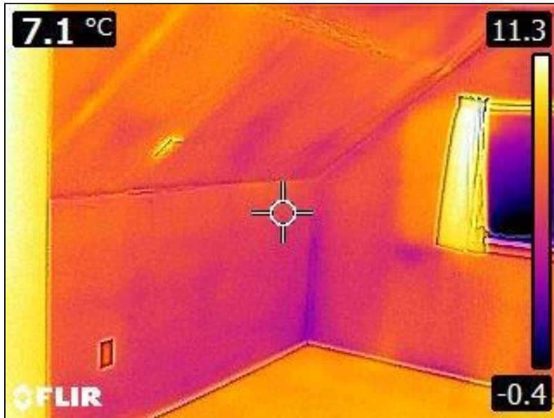
5.1 Item 11(Picture) Interior Walls
