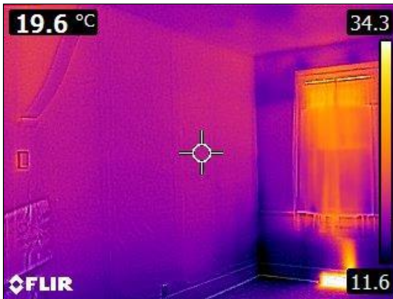
5.1 Item 29(Picture) Interior Walls
