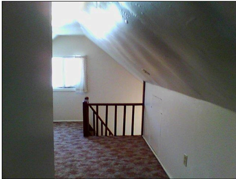
5.1 Item 16(Picture) Interior Walls
