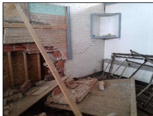
Lead-based white paint (sample L0005) and presumed lead-based light green paint on the brick wall in the Daycare (location 2).
