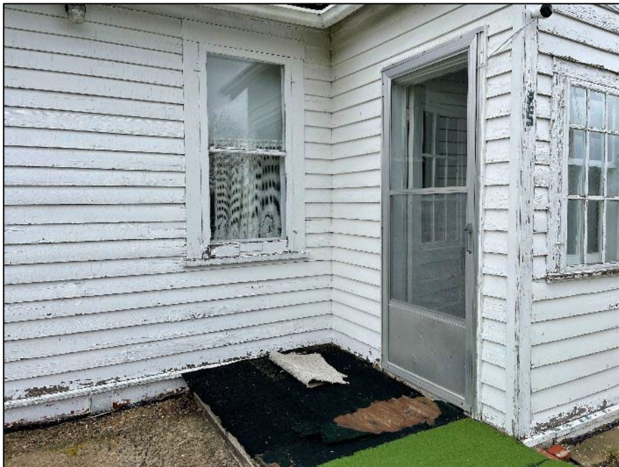
PHOTOGRAPH #12: Window Caulking - Exterior (Non-Asbestos)
