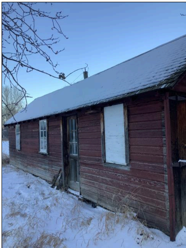
3.1 Item 13(Picture) Outbuilding - aged, structure demo recommended
