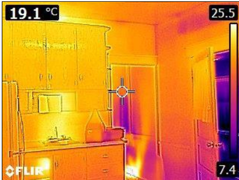
5.1 Item 25(Picture) Interior Walls
