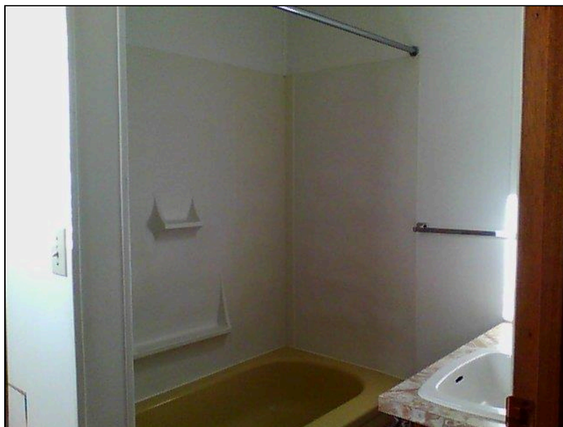
9.0 Item 4(Picture) Bathroom Walls
