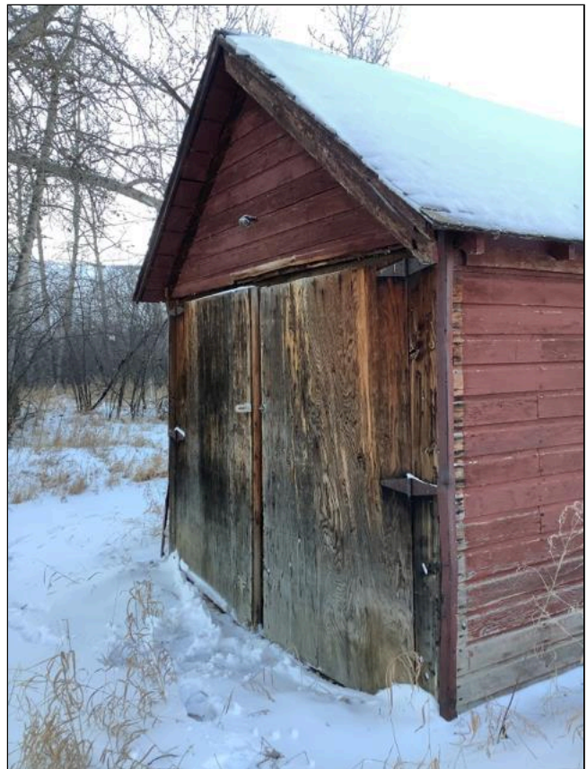
3.1 Item 12(Picture) Outbuilding - aged, structure demo recommended
