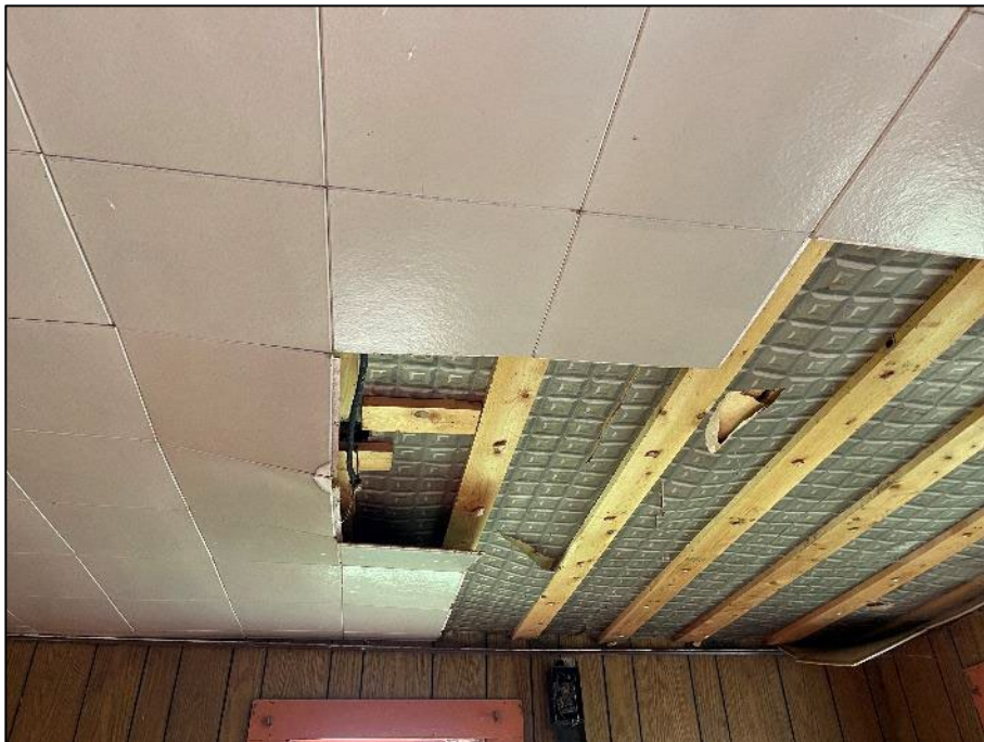
PHOTOGRAPH #24: Ceiling Tile - Small House (Non-Asbestos)
