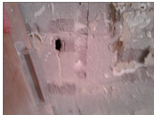
Intrusive inspection location in Room 43 (location 45).
