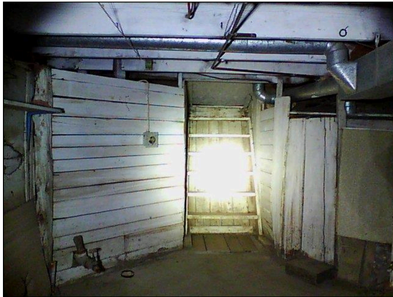
7.0 Item 2(Picture) Basement Foundation
