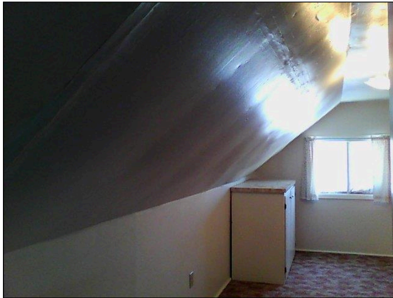
5.1 Item 14(Picture) Interior Walls
