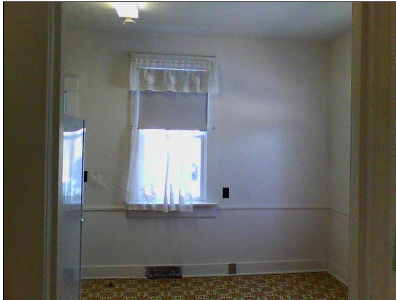
5.1 Item 24(Picture) Interior Walls
