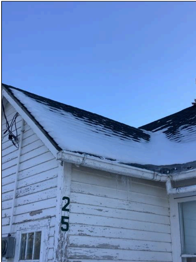
1.0 Item 3(Picture) Roof
