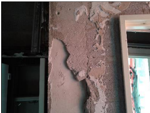
Non-asbestos plaster on the wall (sample S0014B) in Room 42 (location 47).
