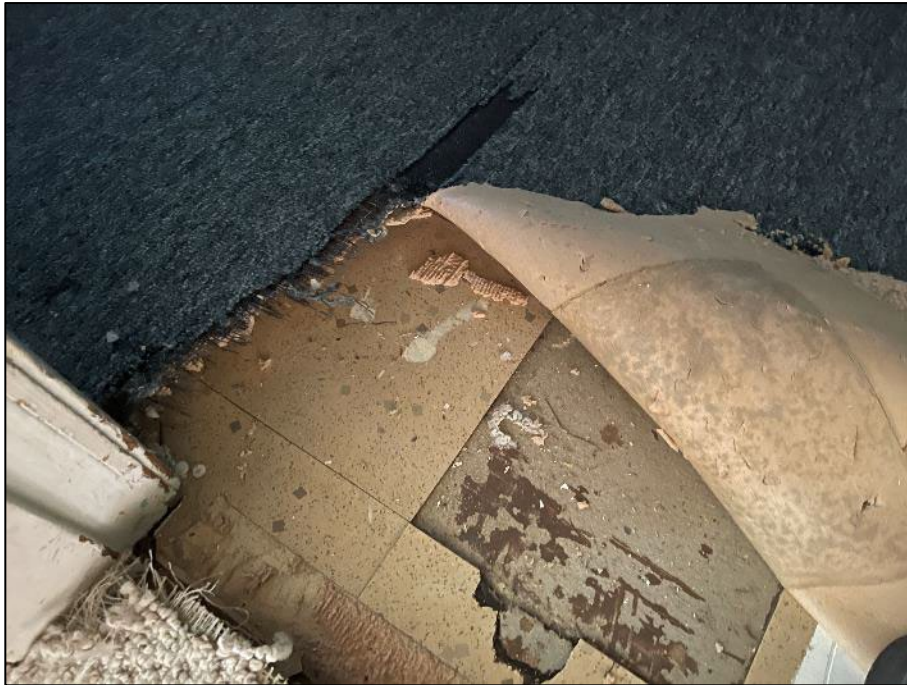
PHOTOGRAPH #15: Floor Tile - Level 1 North Bedroom (Non-Asbestos)
