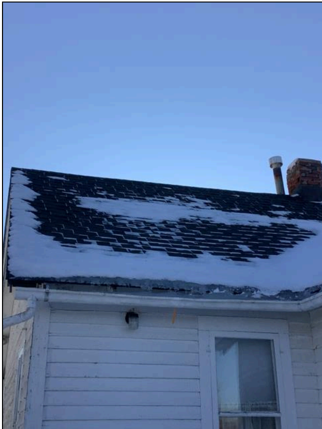
1.0 Item 1(Picture) Roof
