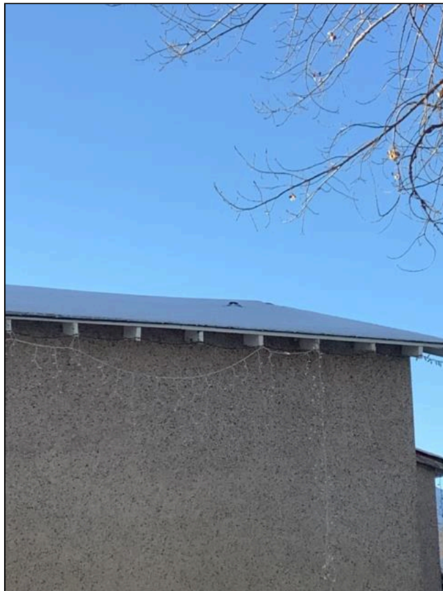
1.0 Item 1(Picture) Roof
