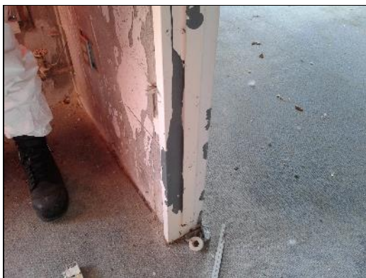
Lead-based white paint (sample L0003) on the metal door frame in the Office (location 3).
