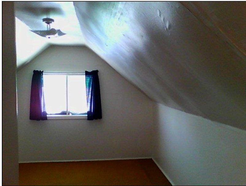
5.1 Item 10(Picture) Interior Walls
