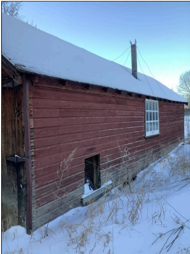
3.1 Item 11(Picture) Outbuilding - aged, structure demo recommended
