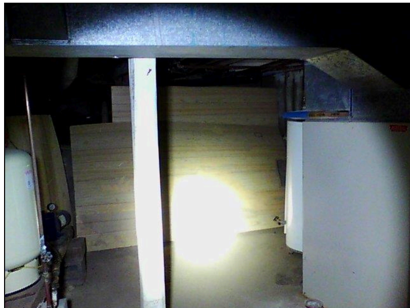
7.0 Item 6(Picture) Basement Foundation
