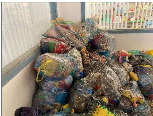
View of accumulated bird droppings in the Classroom (location 3).
