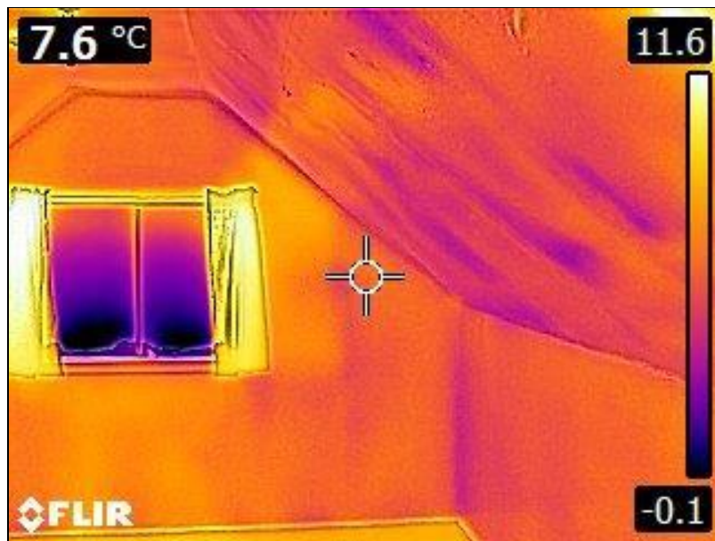
5.1 Item 9(Picture) Interior Walls
