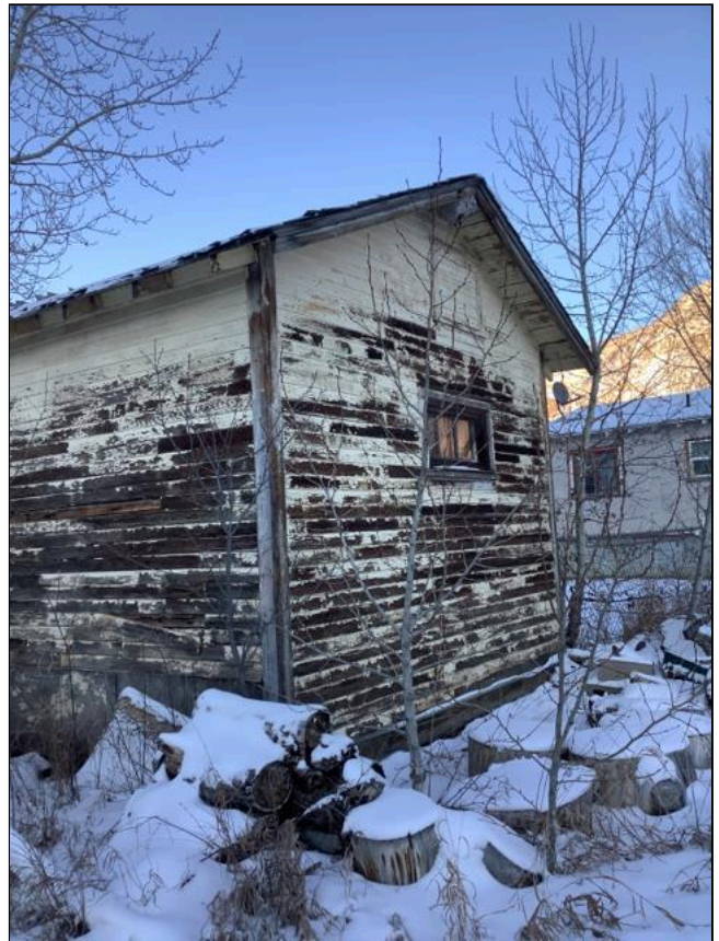
3.1 Item 10(Picture) Outbuilding - aged, structure demo recommended
