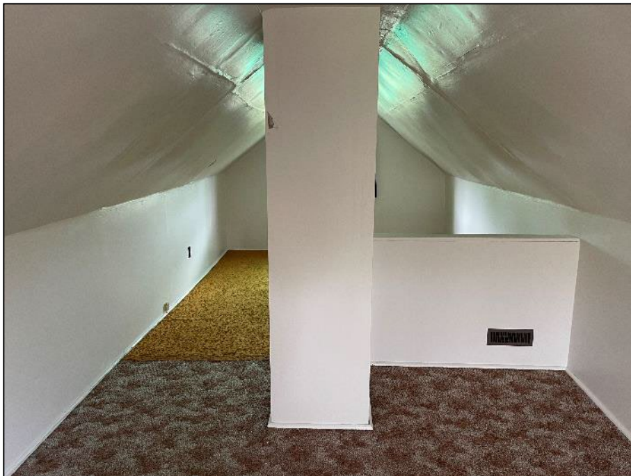
PHOTOGRAPH #2: Drywall Joint Compound – Floor 2 Int Chimney (Non-Asbestos)
