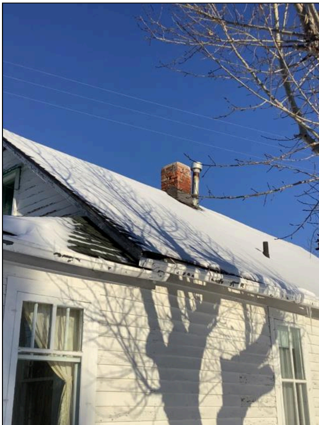
1.0 Item 5(Picture) Roof
