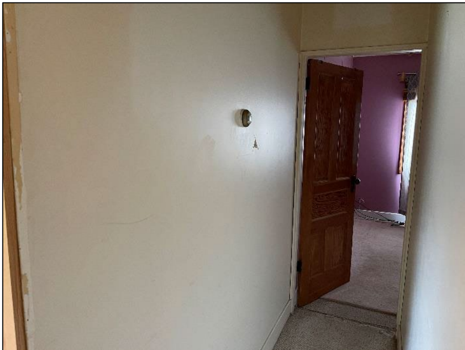
PHOTOGRAPH #4: Drywall Joint Compound - Level 1 Hallway Interior (2% Chrysotile)
