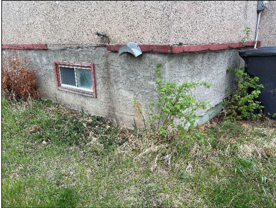
PHOTOGRAPH #19: Parging - Exterior NW Corner (Non-Asbestos)
