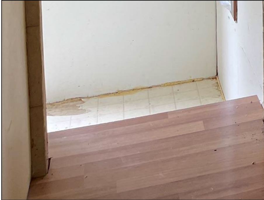
PHOTOGRAPH #13: Sheet Flooring - Level 1 Foyer (Non-Asbestos)
