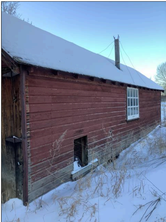
3.1 Item 11(Picture) Outbuilding - aged, structure demo recommended
