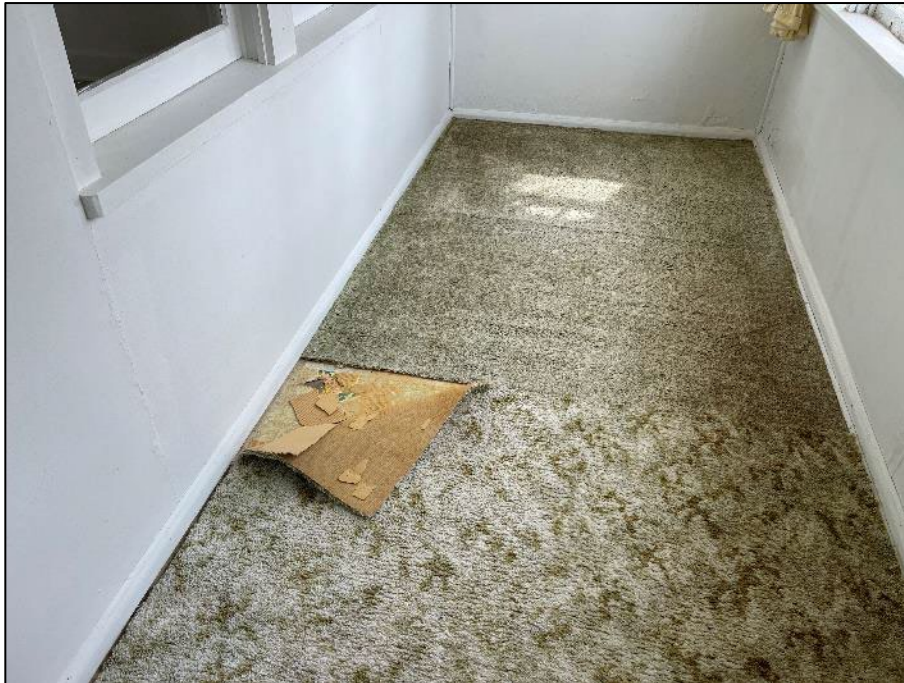
PHOTOGRAPH #7: Flooring – Floor 1 Sun Room (Non-Asbestos)
