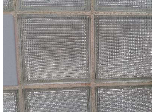
Non-asbestos mortar around glass blocks (sample S0003A) on the Exterior (location 1).
