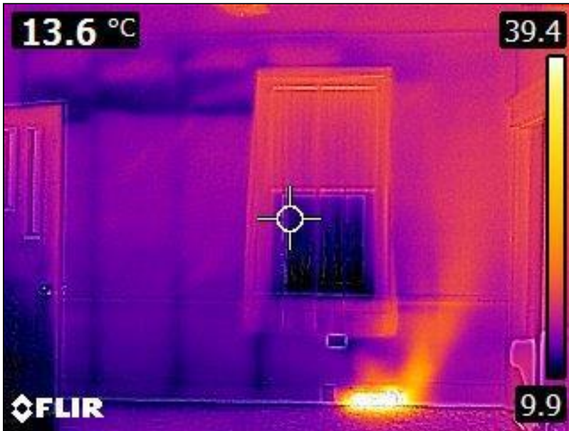
5.1 Item 31(Picture) Interior Walls
