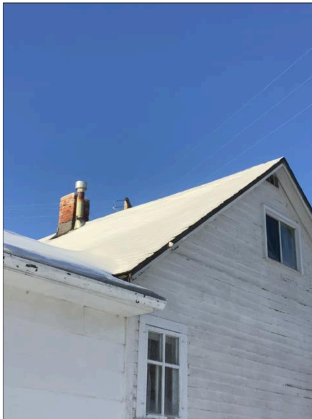
1.0 Item 8(Picture) Roof
