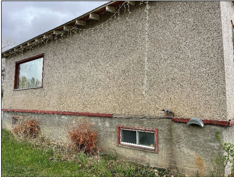
PHOTOGRAPH #17: Stucco - Exterior East Face (Non-Asbestos)
