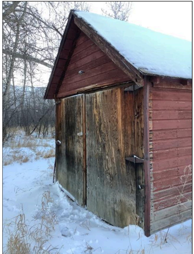
3.1 Item 12(Picture) Outbuilding - aged, structure demo recommended
