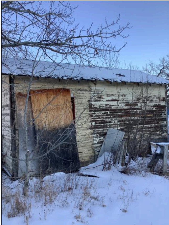
3.1 Item 9(Picture) Outbuilding - aged, structure demo recommended
