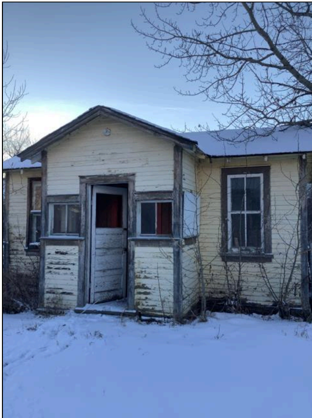
3.1 Item 7(Picture) Outbuilding - aged, structure demo recommended
