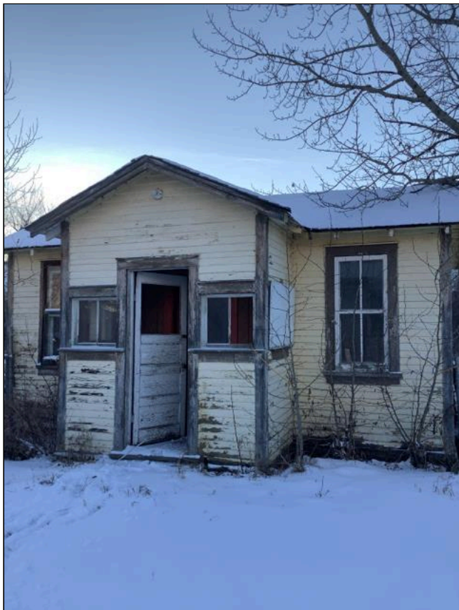
3.1 Item 7(Picture) Outbuilding - aged, structure demo recommended
