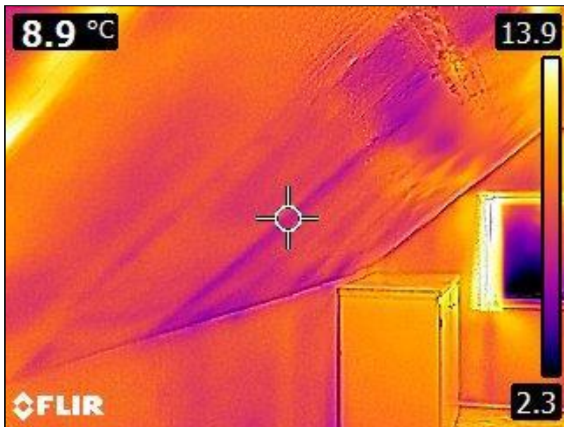
5.1 Item 13(Picture) Interior Walls
