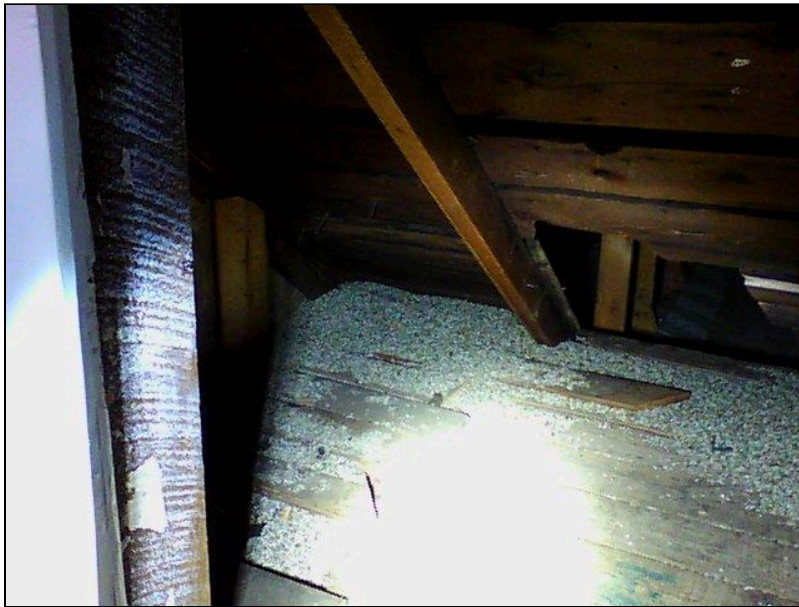
2.0 Item 8(Picture) Attic
