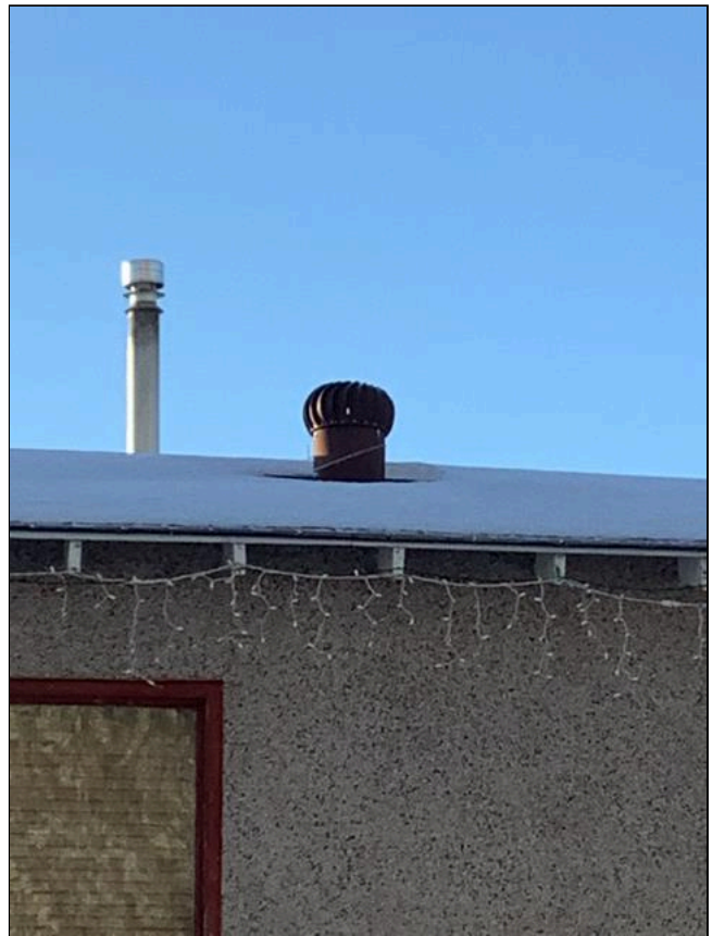
1.0 Item 2(Picture) Roof
