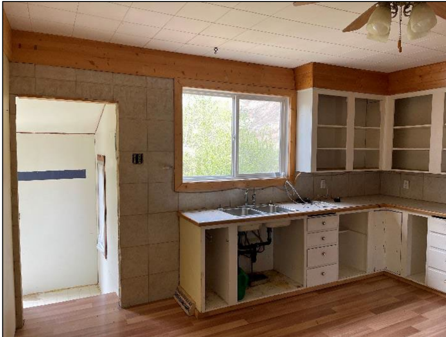
PHOTOGRAPH #1: Drywall Joint Compound - Floor 1 Exterior Kitchen (2% Chrysotile)
