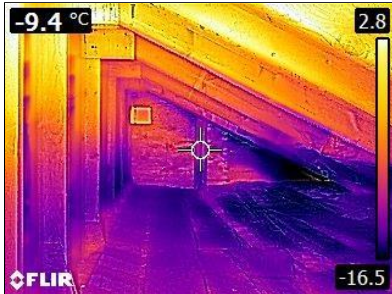
2.0 Item 1(Picture) Attic
