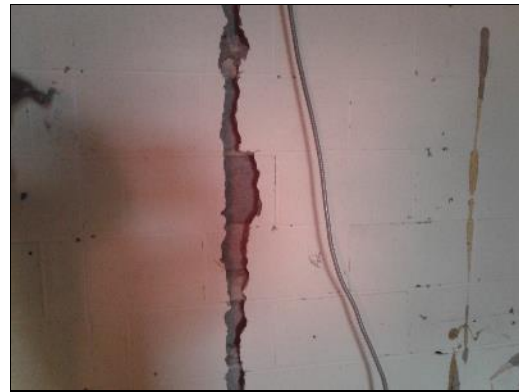
Non-lead based white paint (sample L0002) on the masonry block wall in the Administration Area (location 2).
