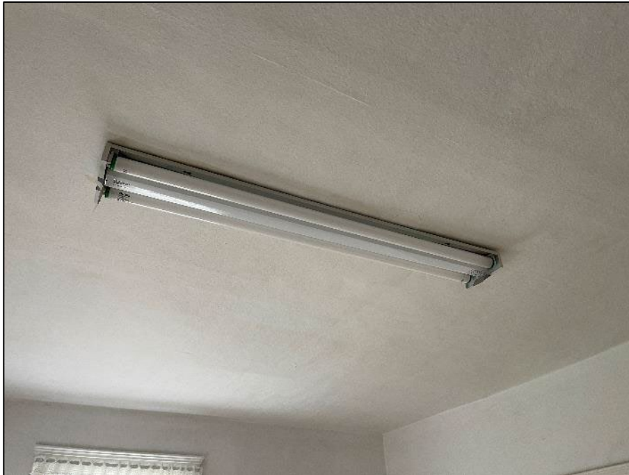
PHOTOGRAPH #19: Fluorescent Light Tubes (Mercury)
