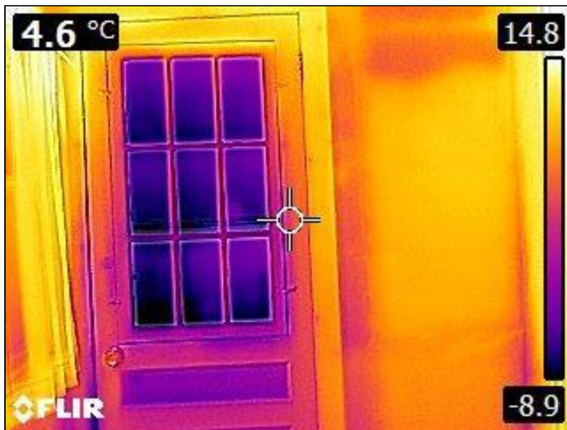
5.1 Item 43(Picture) Interior Walls
