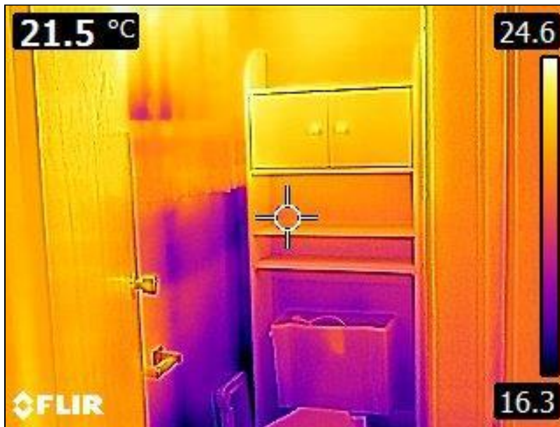
9.0 Item 1(Picture) Bathroom Walls
