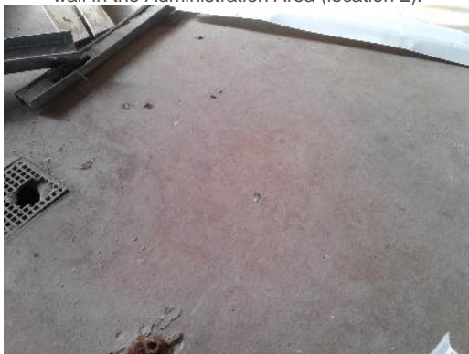
Non-asbestos non-slip flooring (sample S0015) in the Cafeteria (location 28).
