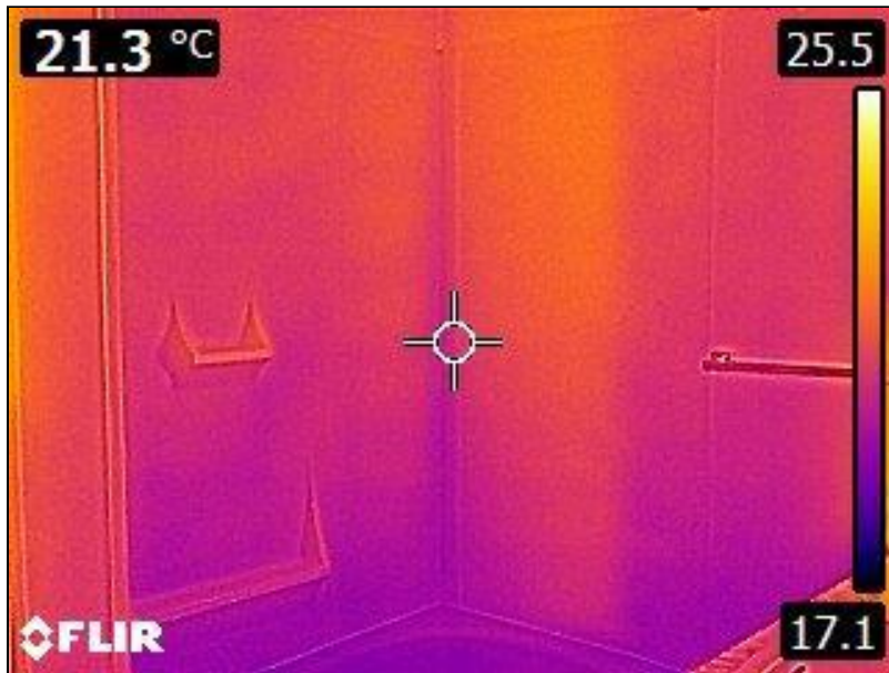
9.0 Item 3(Picture) Bathroom Walls
