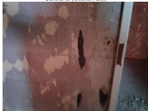
Non-asbestos black mastic (sample S0024) on the wall in Room 23 (location 81).
