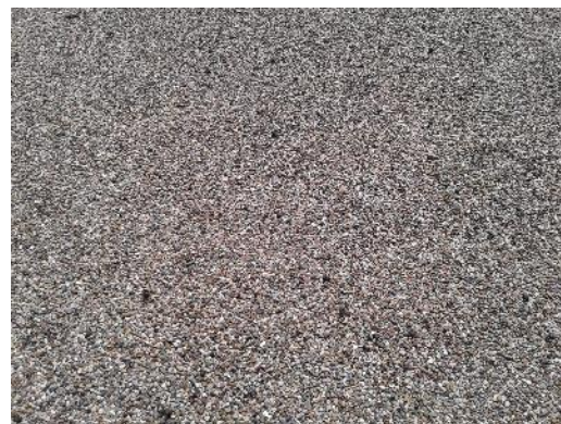
Non-asbestos built-up roofing (sample S0006A) on the Roof (location 133).
