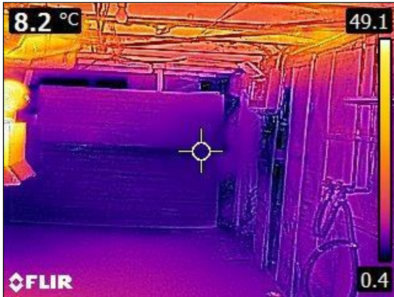
7.0 Item 3(Picture) Basement Foundation
