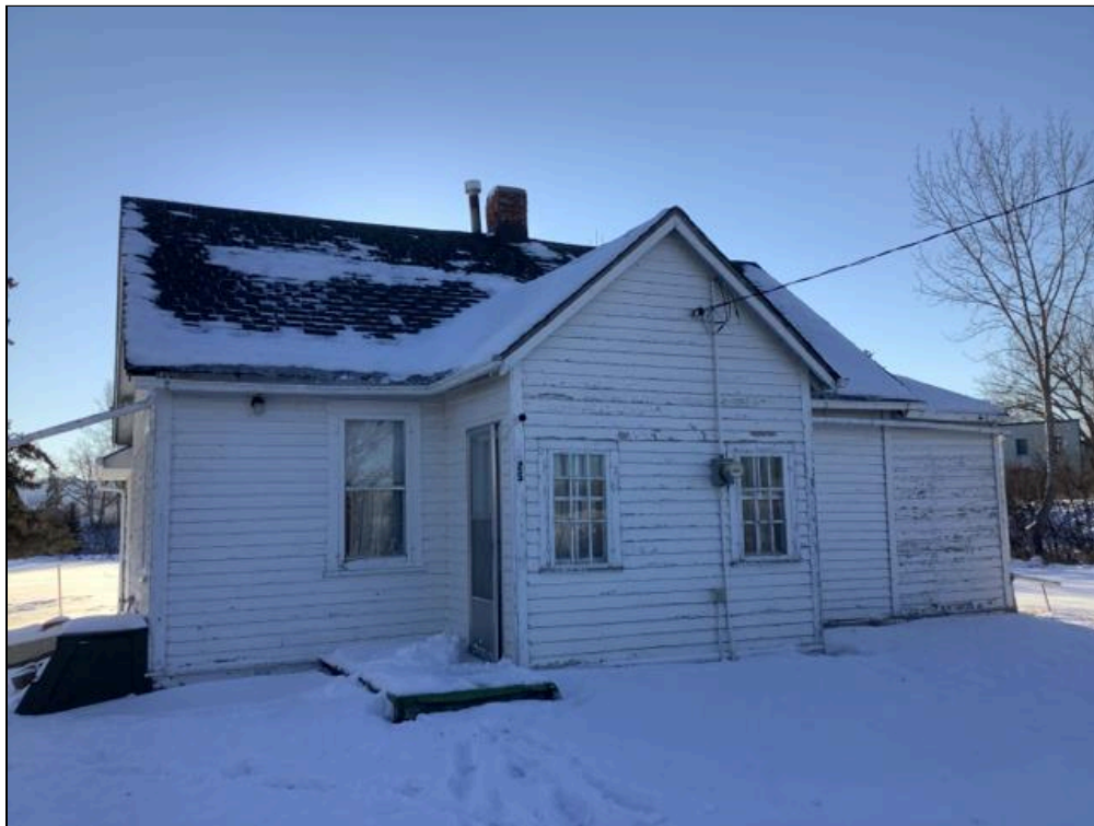
25 Roper Road - Rosedale
