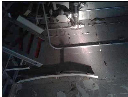
Non-asbestos cementitious firestopping (sample S0013) in the Hallway (location 22).
