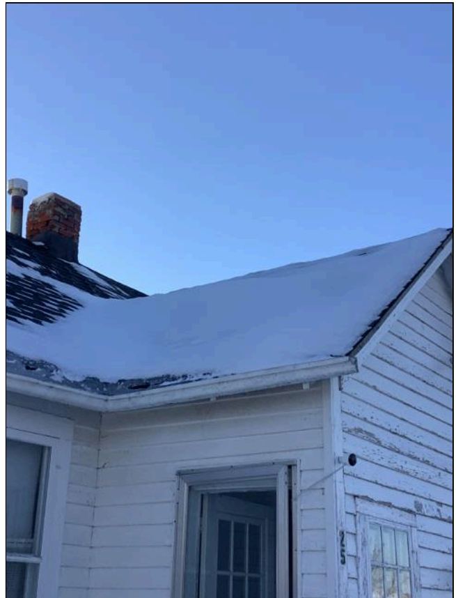
1.0 Item 2(Picture) Roof
