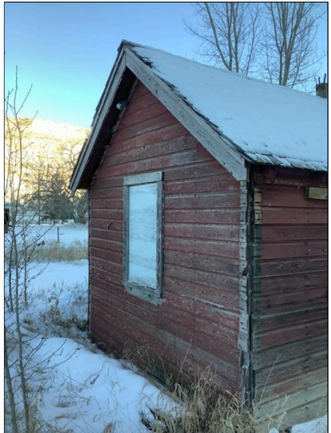
3.1 Item 14(Picture) Outbuilding - aged, structure demo recommended
