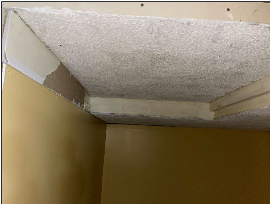
PHOTOGRAPH #10: Ceiling Texture - Basement Closet (Non-Asbestos)
