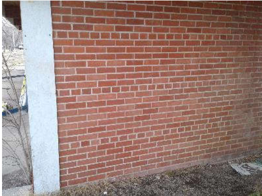
Non-asbestos brick mortar (sample S0002C) on the Exterior (location 1).
