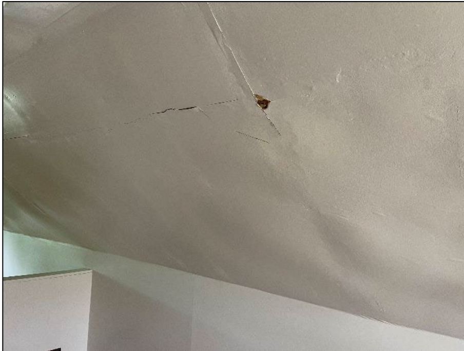
PHOTOGRAPH #9: Skim Coat (White) - Floor 2 West Wall (Non-Asbestos)
