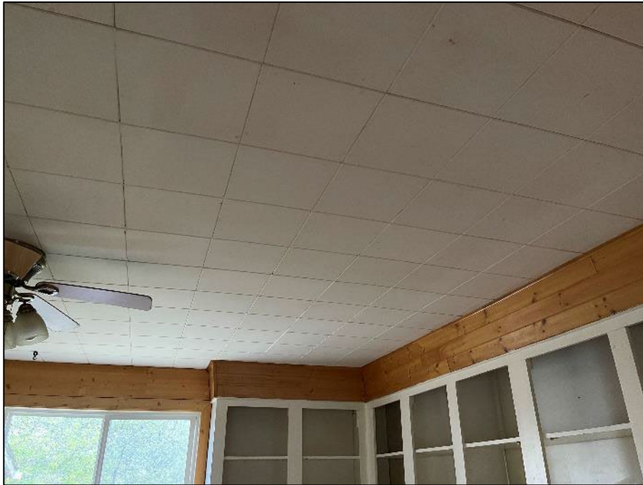
PHOTOGRAPH #11: Ceiling Tile - Level 1 Kitchen (1x1) (Non-Asbestos)
