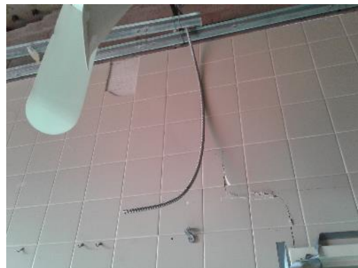
Non-asbestos thin-set (sample S0011D) on the wall in the Cafeteria (location 28).
