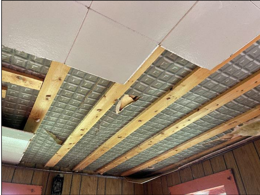
PHOTOGRAPH #25: Ceiling Board - Small House (Non-Asbestos)
