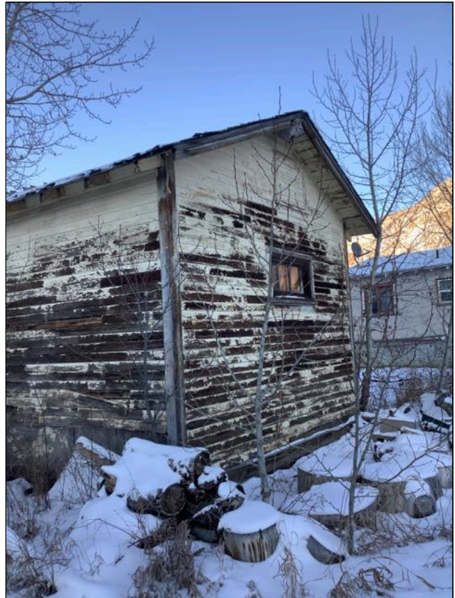
3.1 Item 10(Picture) Outbuilding - aged, structure demo recommended
