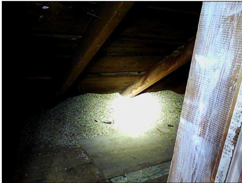
2.0 Item 10(Picture) Attic
