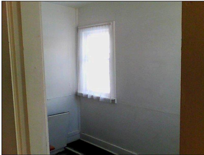
5.1 Item 42(Picture) Interior Walls
