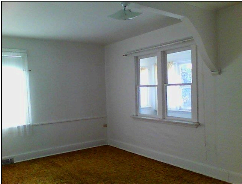
5.1 Item 28(Picture) Interior Walls
