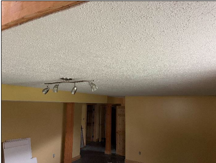
PHOTOGRAPH #9: Ceiling Texture - Basement Living Room (Non-Asbestos)
