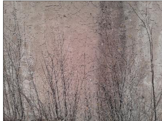
Non-asbestos stucco (sample S0005C) on the exterior (location 1).
