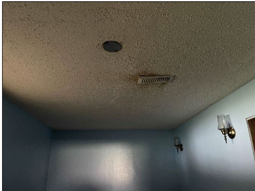
PHOTOGRAPH #8: Ceiling Texture - Basement Bedroom (Non-Asbestos)
