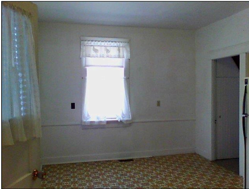
5.1 Item 22(Picture) Interior Walls
