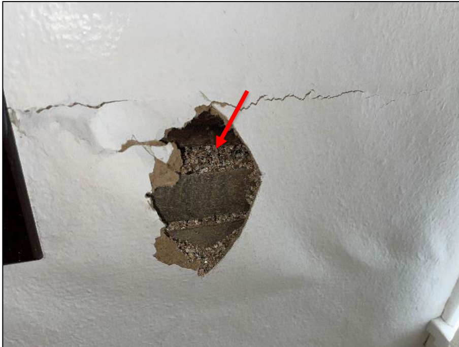
PHOTOGRAPH #13: Vermiculite – West Wall (<1% Actinolite)
