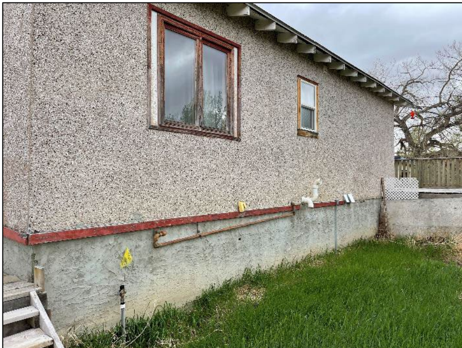
PHOTOGRAPH #18: Stucco - Exterior West Face (Non-Asbestos)
