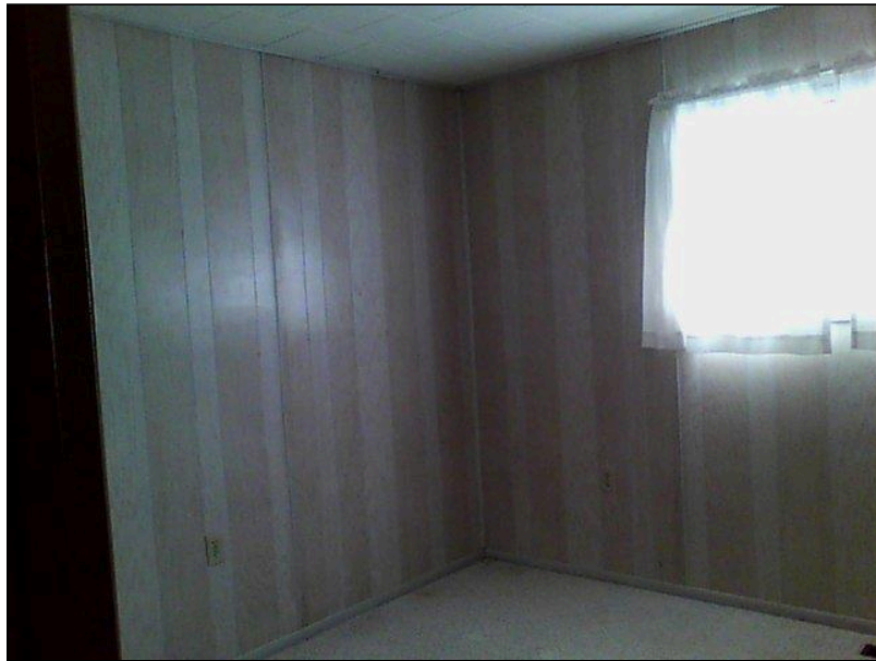
5.1 Item 40(Picture) Interior Walls
