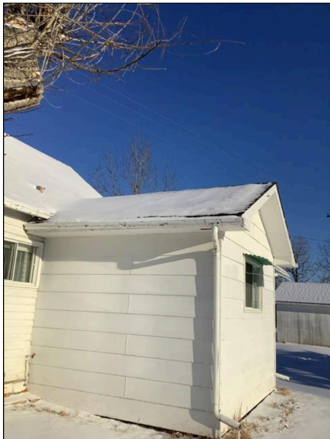
1.0 Item 7(Picture) Roof
