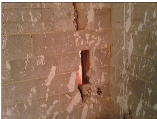
Intrusive inspection location in the Office (location 3).
