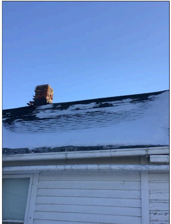
1.0 Item 4(Picture) Roof
