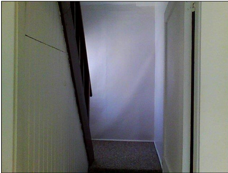
5.1 Item 20(Picture) Interior Walls
