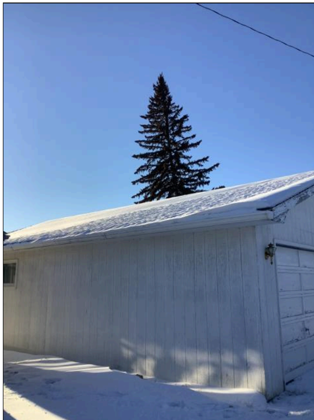
4.0 Item 2(Picture) Garage Roof
