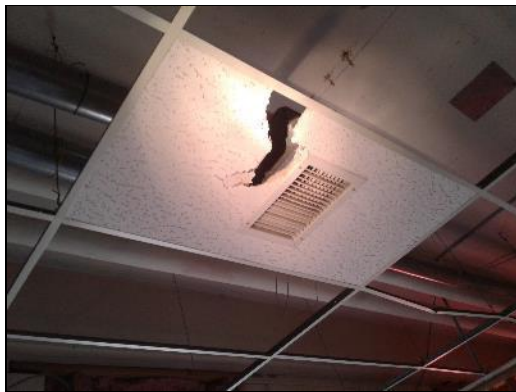
Non-asbestos 24"x48" large fissures and pinholes patterned acoustic ceiling tile (sample S0009A) in the Administration Area (location 2).
