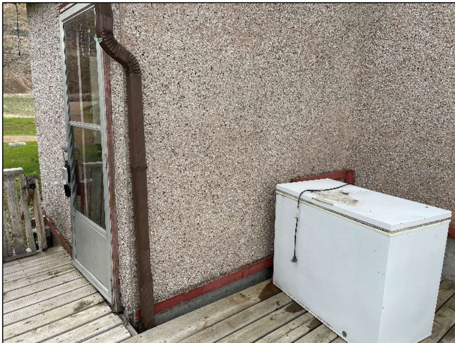
PHOTOGRAPH #16: Stucco - Exterior North Face (Non-Asbestos)
