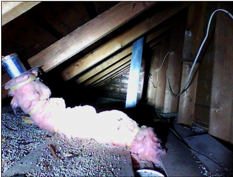
2.0 Item 6(Picture) Attic
