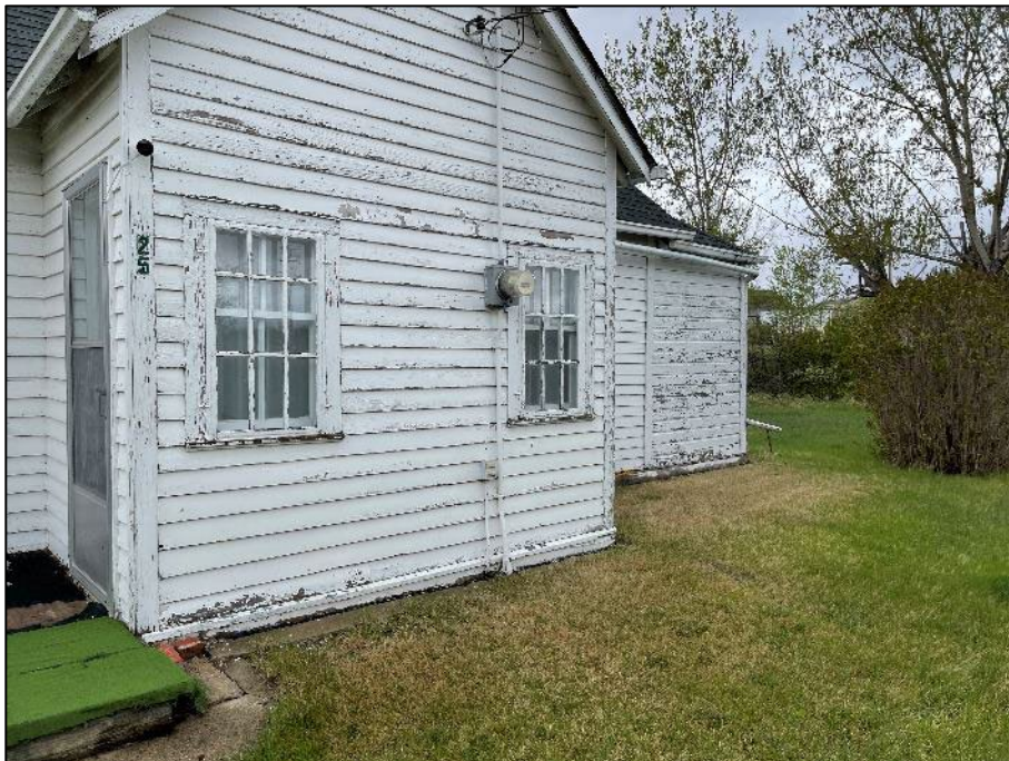
PHOTOGRAPH #16: Paint – White Exterior of Home (Lead Based)
