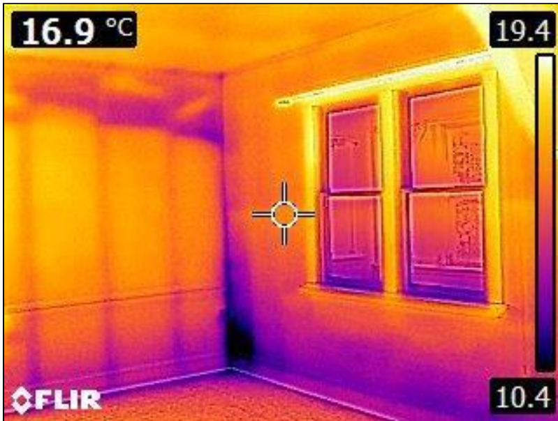
5.1 Item 27(Picture) Interior Walls
