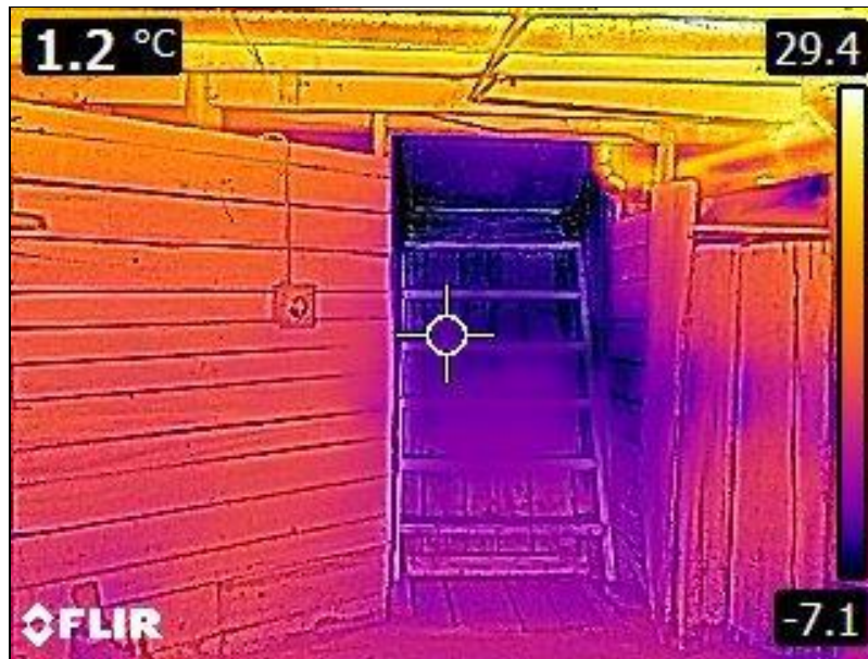
7.0 Item 1(Picture) Basement Foundation
