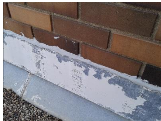
Non-asbestos grey caulking (sample S0030) on seams on the Roof (location 133).
