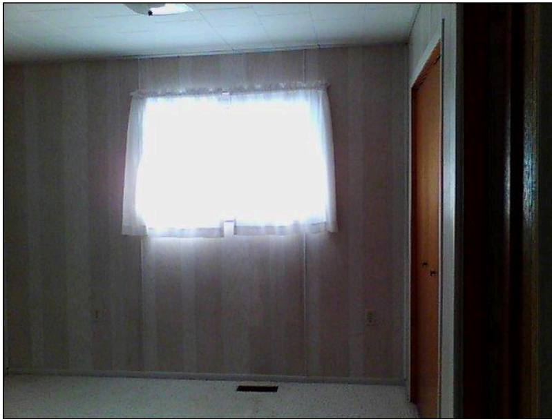
5.1 Item 38(Picture) Interior Walls
