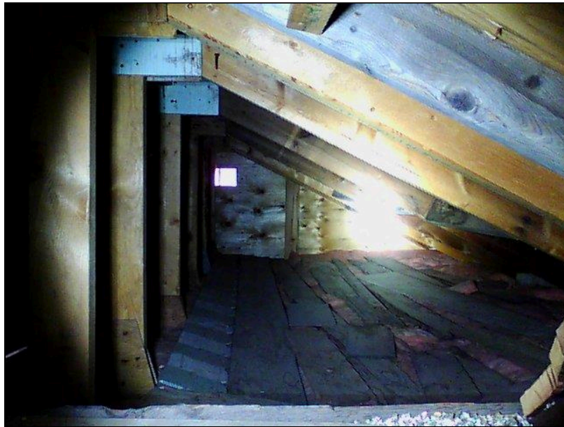
2.0 Item 2(Picture) Attic
