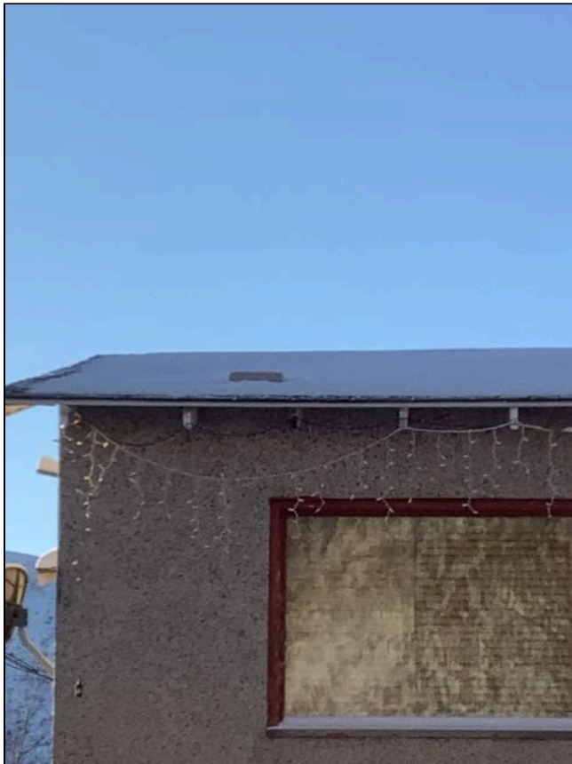
1.0 Item 3(Picture) Roof
