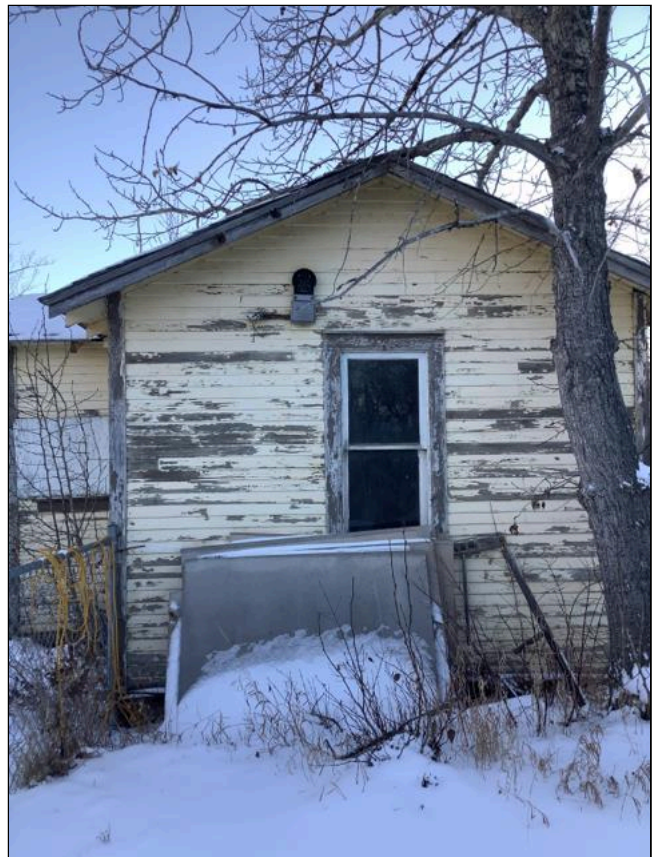
3.1 Item 8(Picture) Outbuilding - aged, structure demo recommended
