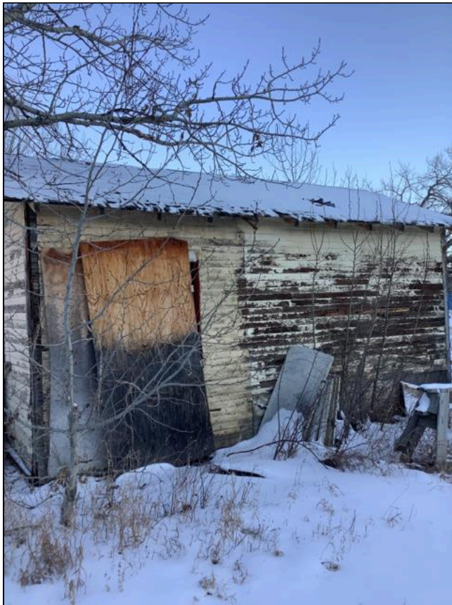
3.1 Item 9(Picture) Outbuilding - aged, structure demo recommended
