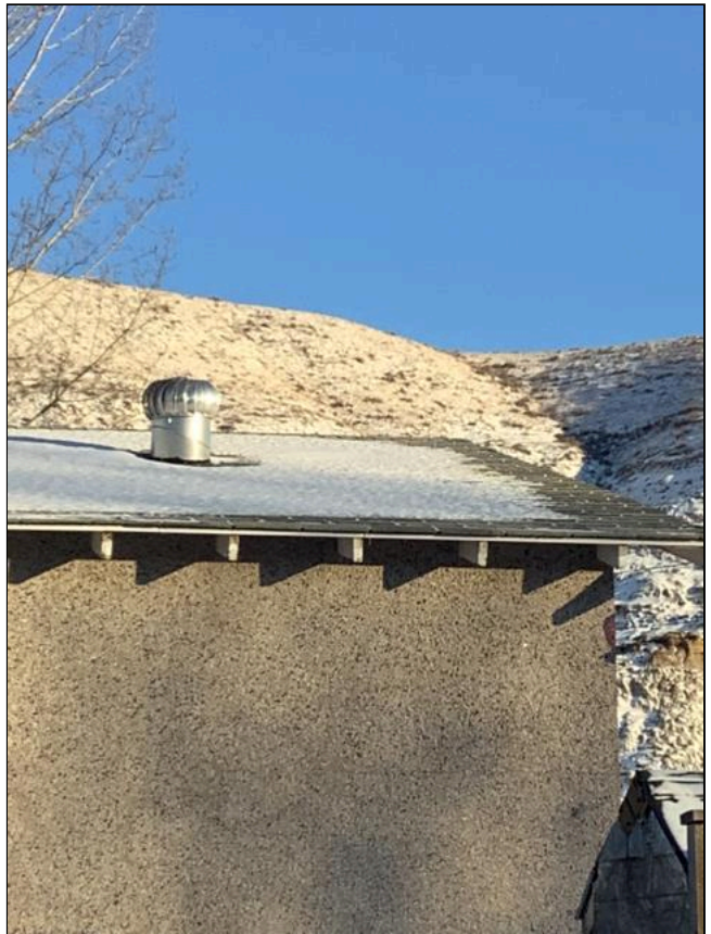
1.0 Item 4(Picture) Roof
