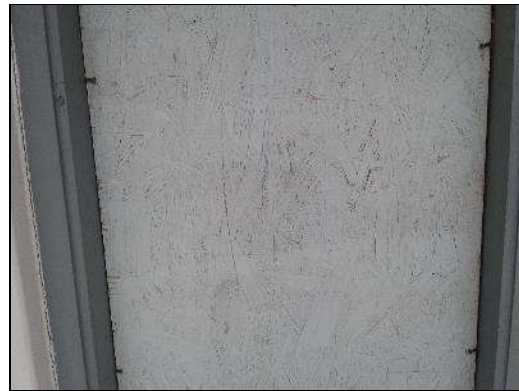
Non-lead based light blue paint (sample L0003) on the wood wall on the Exterior (location 1).
