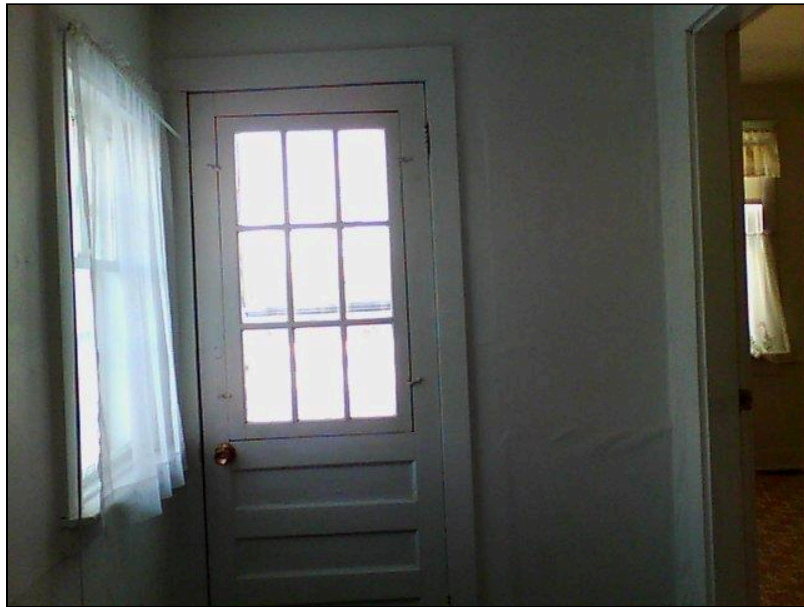
5.1 Item 44(Picture) Interior Walls
