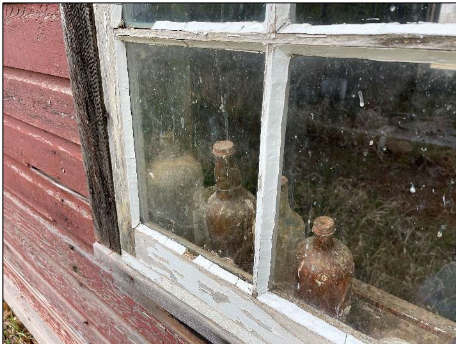
PHOTOGRAPH #22: Window Caulking - Large Shed Interior (Non-Asbestos)
