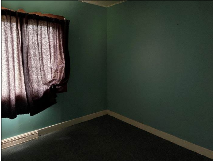
PHOTOGRAPH #3: Drywall Joint Compound - Level 1 North Bedroom Exterior (Assume Positive)
