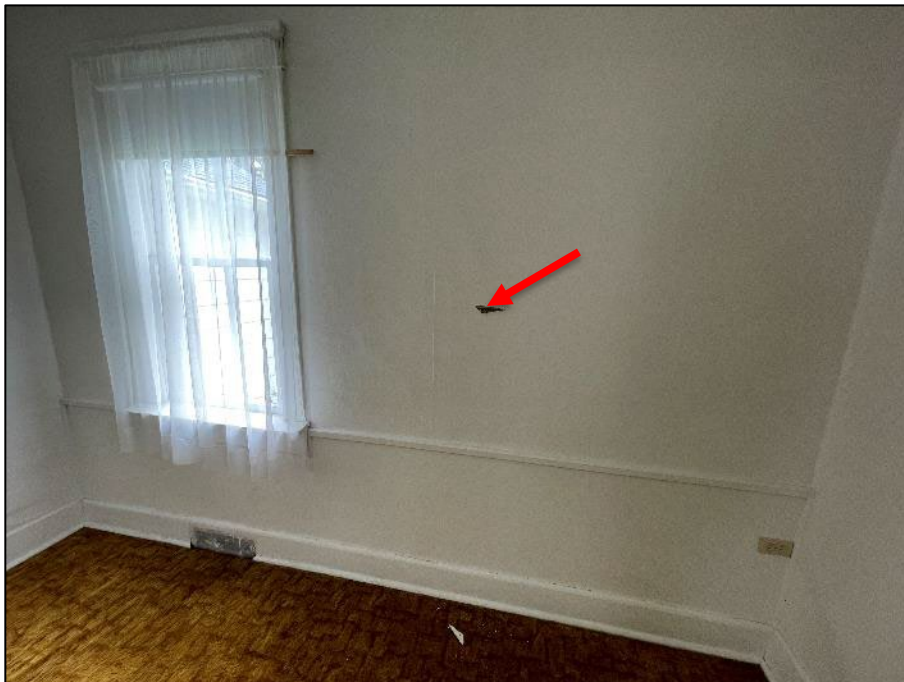
PHOTOGRAPH #14: Vermiculite – East Wall (<1% Actinolite)
