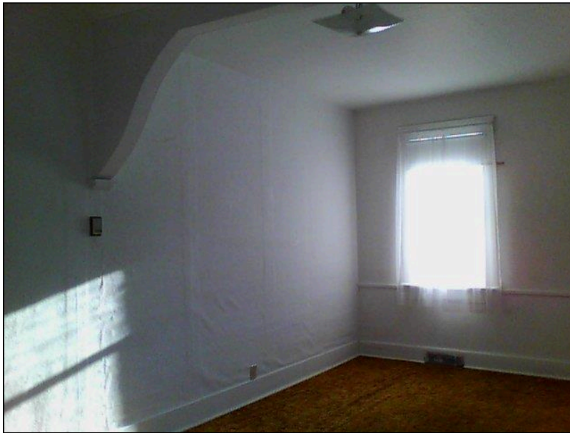
5.1 Item 30(Picture) Interior Walls
