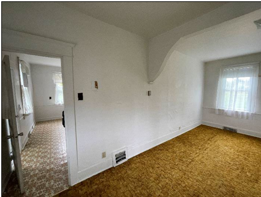
PHOTOGRAPH #10: Wall Board - Floor 1 Living Room (Non-Asbestos)
