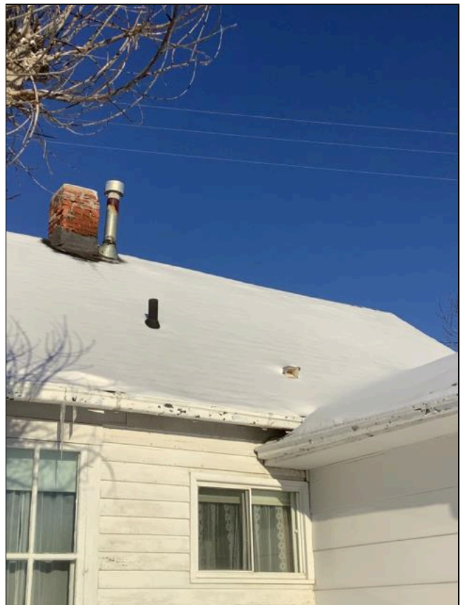
1.0 Item 6(Picture) Roof
