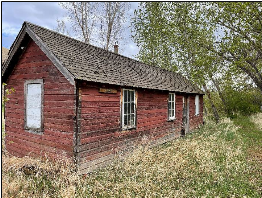
PHOTOGRAPH #38: Large Shed – No Access Provided (Door Locked)
