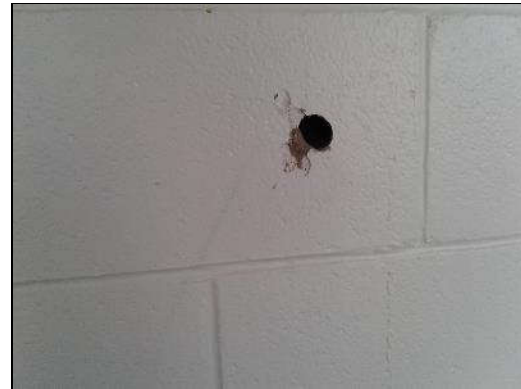
Intrusive inspection location in the Hallway (location 6).
