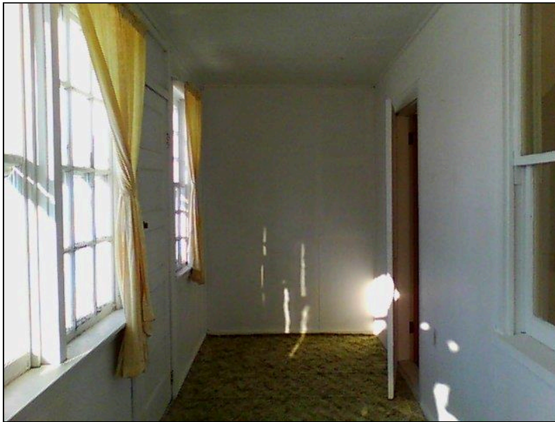
5.1 Item 36(Picture) Interior Walls
