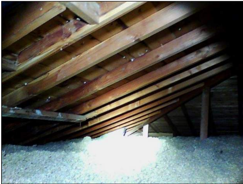
2.0 Item 6(Picture) Attic
