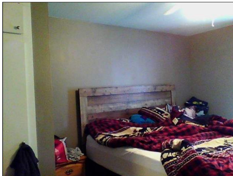
5.1 Item 2(Picture) Interior Walls
