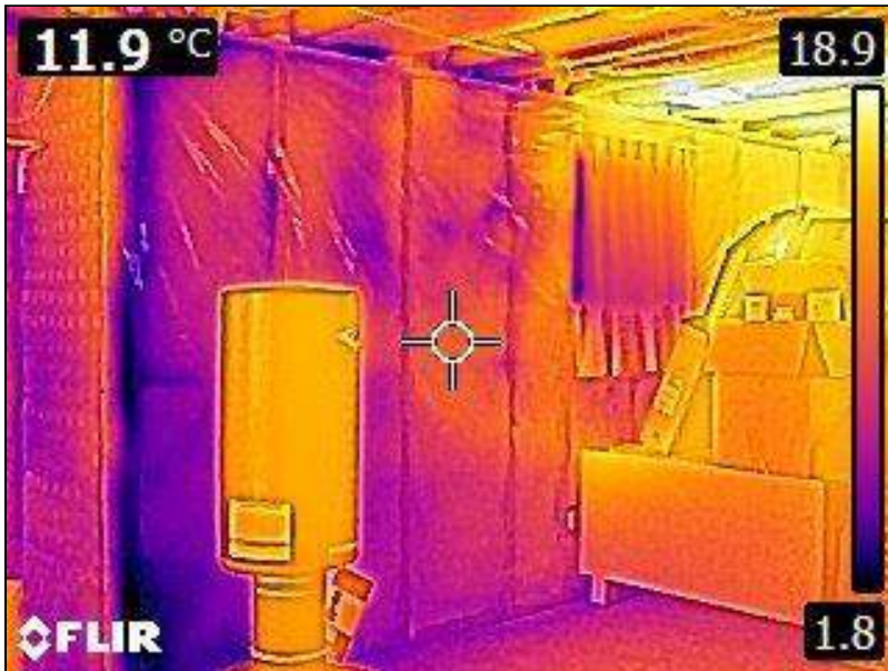
7.0 Item 9(Picture) Basement Foundation
