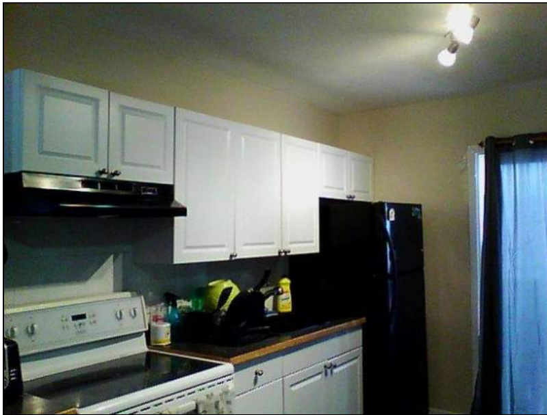
5.1 Item 33(Picture) Interior Walls
