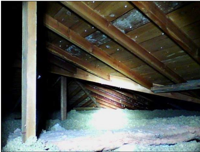
2.0 Item 2(Picture) Attic
