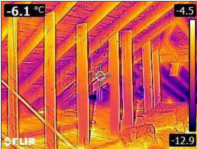
2.0 Item 5(Picture) Attic
