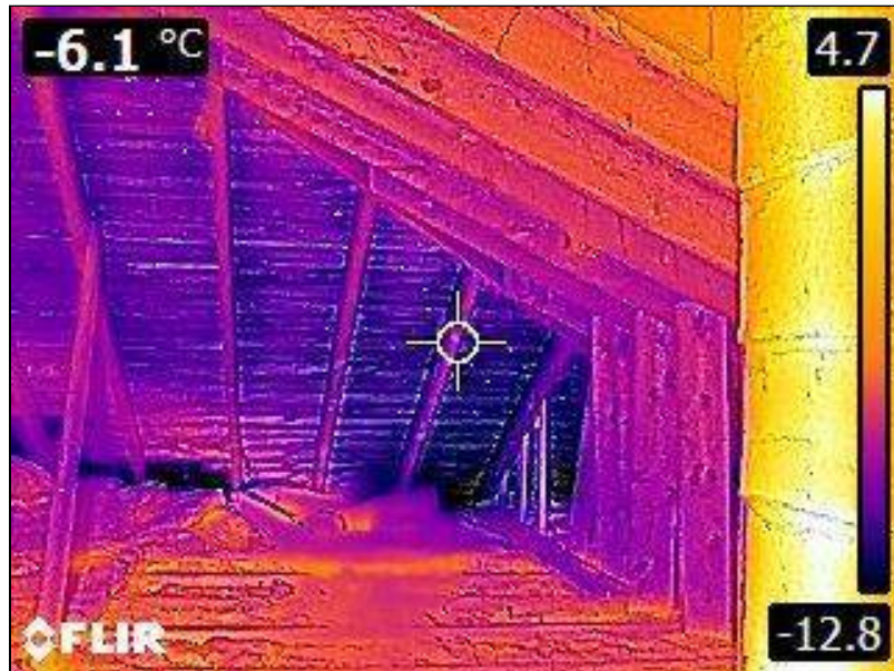
2.0 Item 1(Picture) Attic
