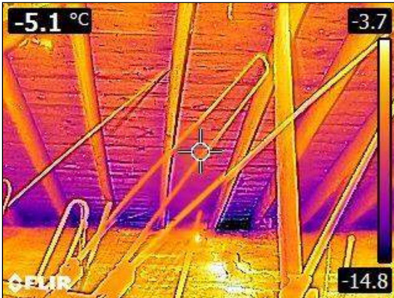
2.0 Item 15(Picture) Attic
