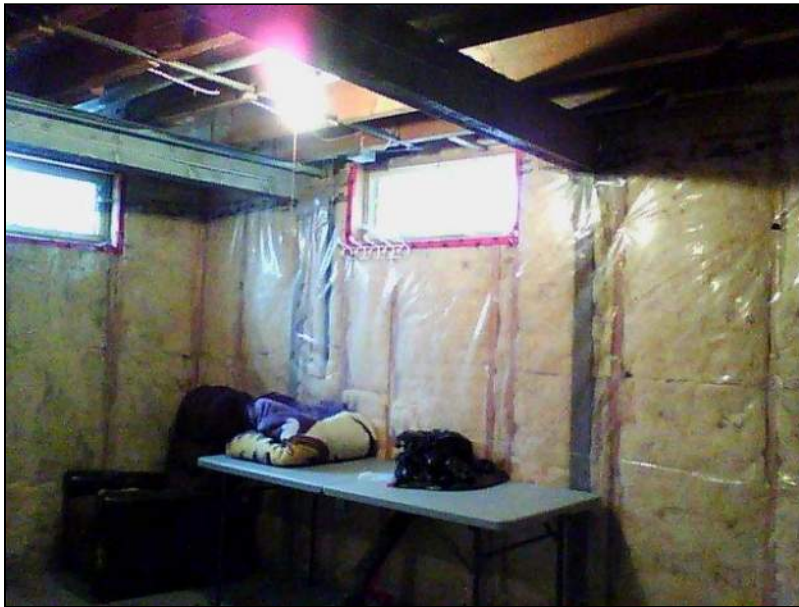
7.0 Item 20(Picture) Basement Foundation
