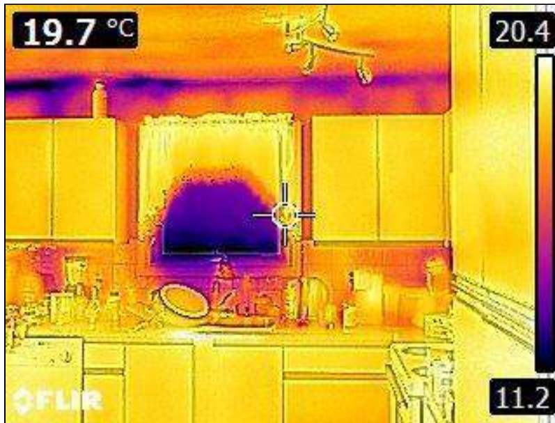
5.1 Item 33(Picture) Interior Walls
