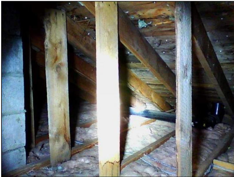
2.0 Item 12(Picture) Attic
