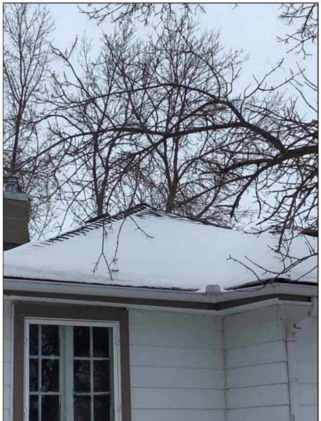
1.0 Item 10(Picture) Roof
