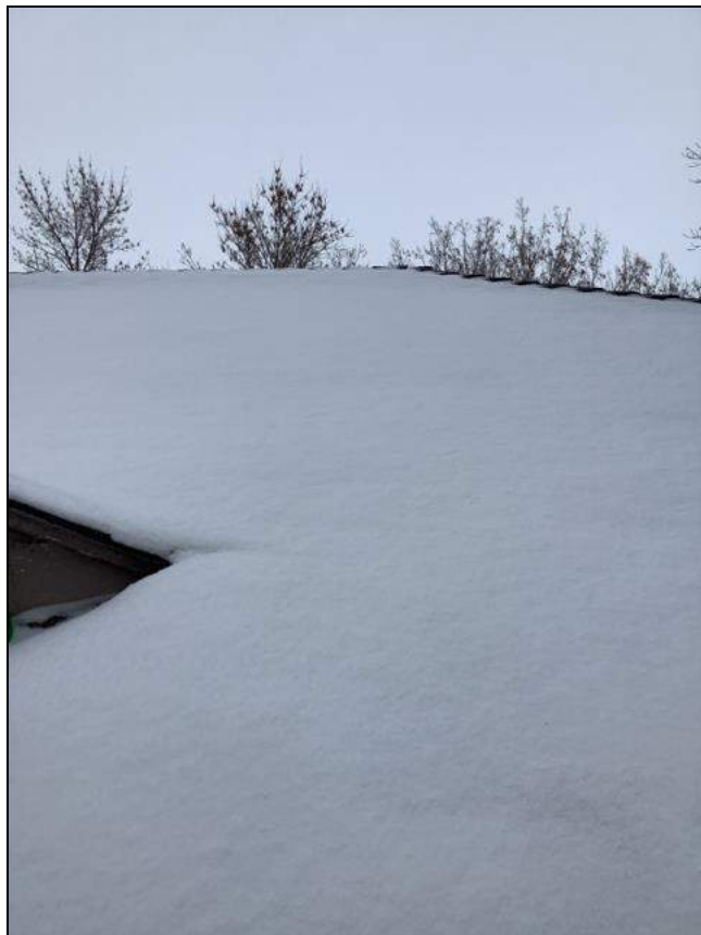
1.0 Item 1(Picture) Roof
