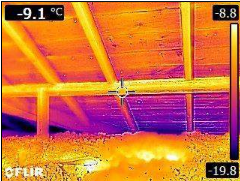
2.0 Item 13(Picture) Attic
