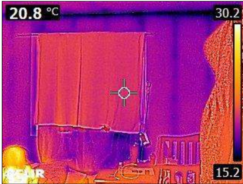
5.1 Item 15(Picture) Interior Walls
