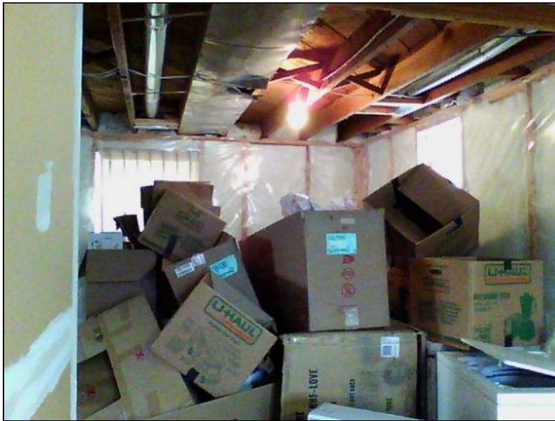
7.0 Item 6(Picture) Basement Foundation
