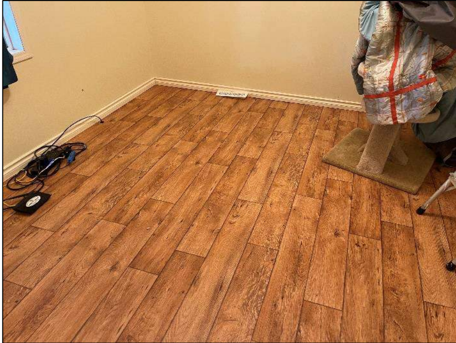
PHOTOGRAPH #11: Flooring - Level 1 SW Bedroom (Non-Asbestos)
