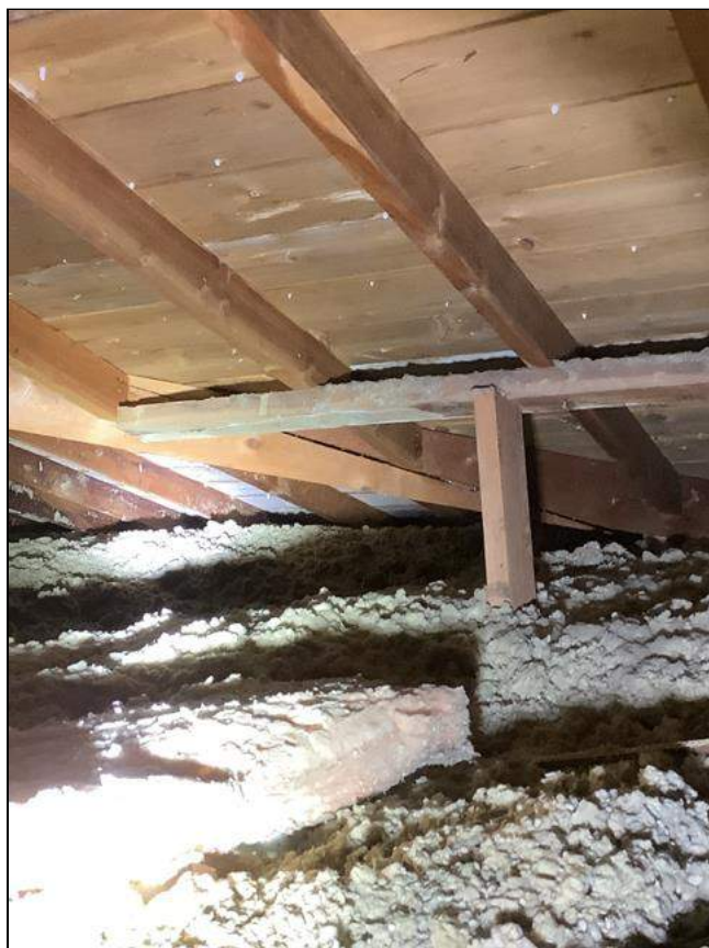
2.3 Item 1(Picture) Rafter - split, cross support bowed
