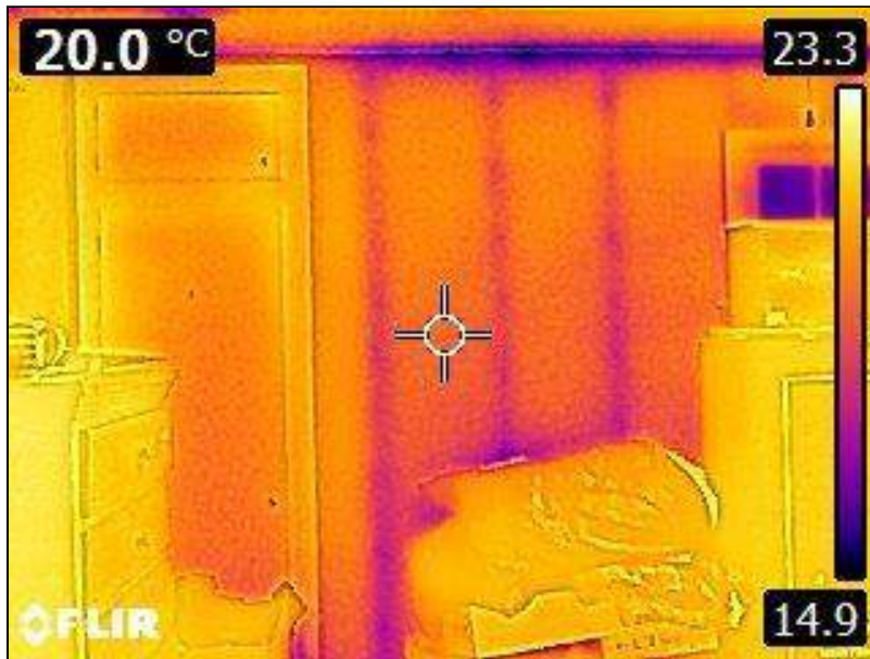
5.1 Item 11(Picture) Interior Walls
