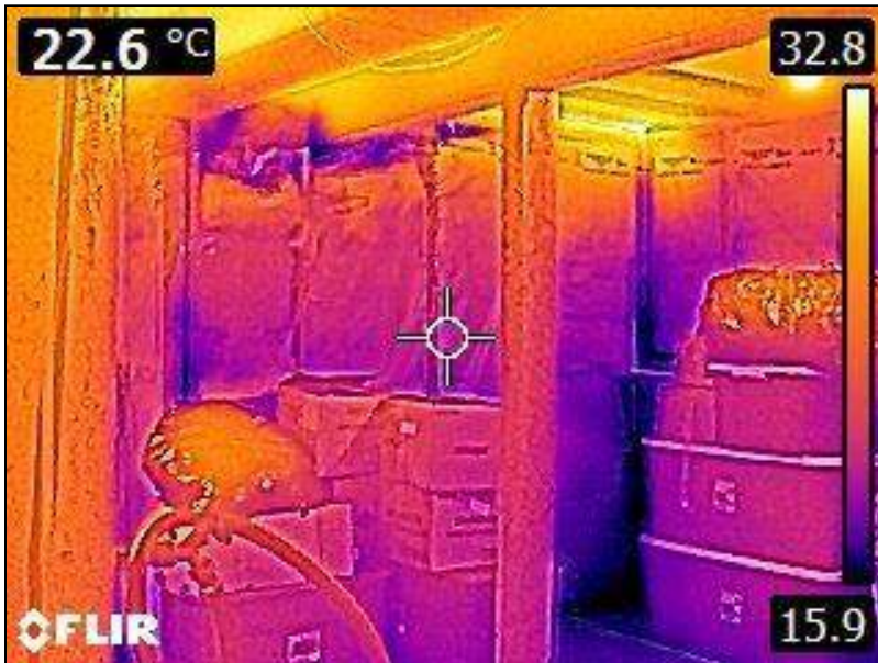
7.0 Item 17(Picture) Basement Foundation
