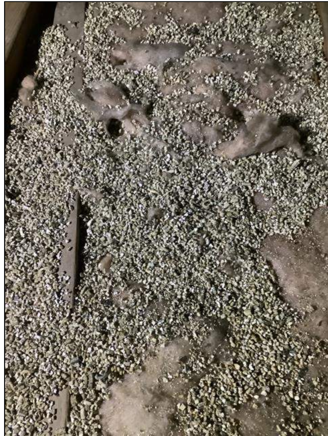
2.4 Item 1(Picture) Attic Insulation - vermiculite
