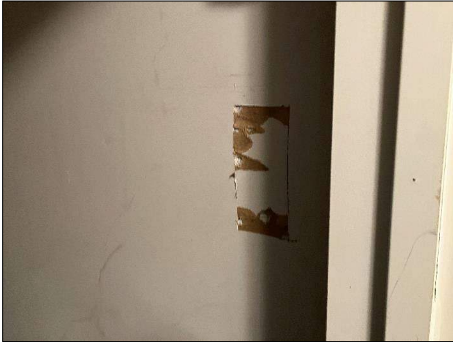
PHOTOGRAPH #23: Paint – White Stairs (Non-Lead Based)
