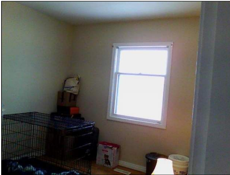
5.1 Item 13(Picture) Interior Walls
