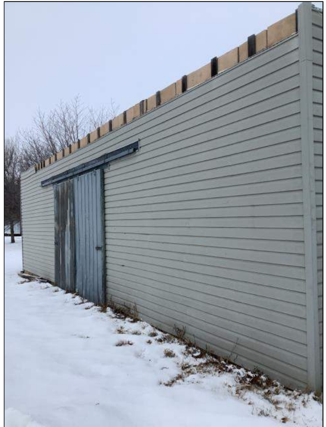
4.4 Item 2(Picture) Garage Exterior
