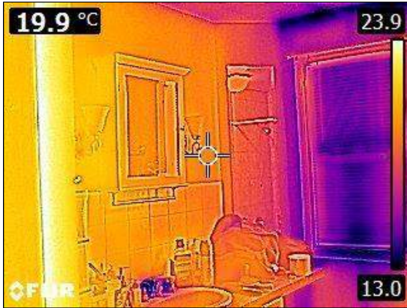
9.0 Item 2(Picture) Bathroom Walls
