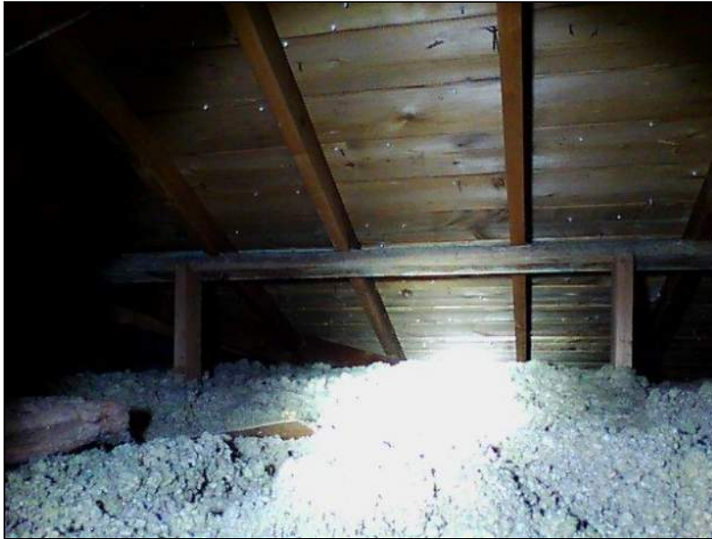
2.0 Item 14(Picture) Attic
