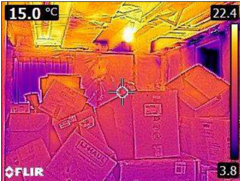
7.0 Item 5(Picture) Basement Foundation
