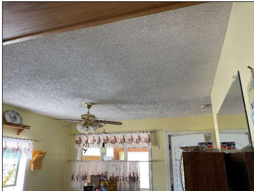
PHOTOGRAPH #8: Ceiling Texture - Level 1 Kitchen (Non-Asbestos)
