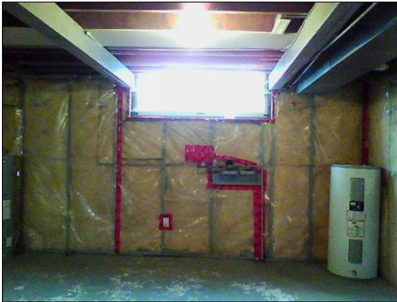
7.0 Item 16(Picture) Basement Foundation
