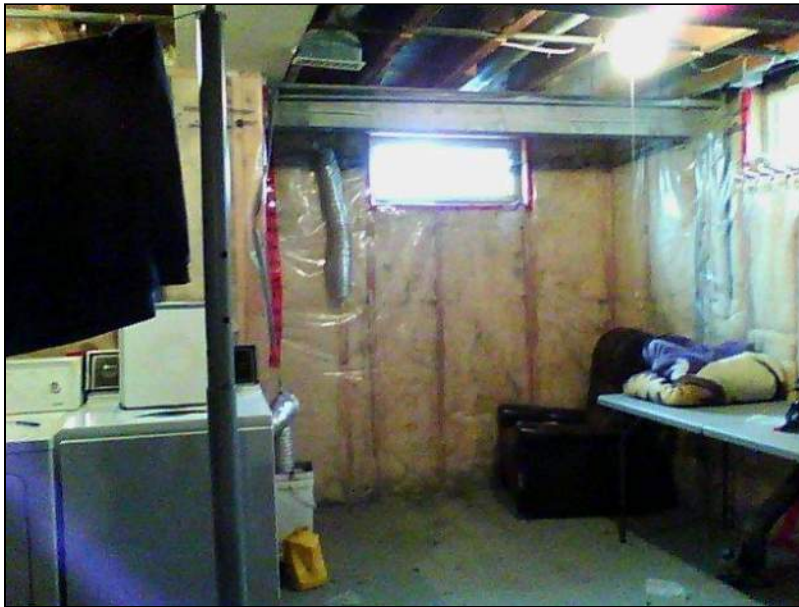
7.0 Item 22(Picture) Basement Foundation
