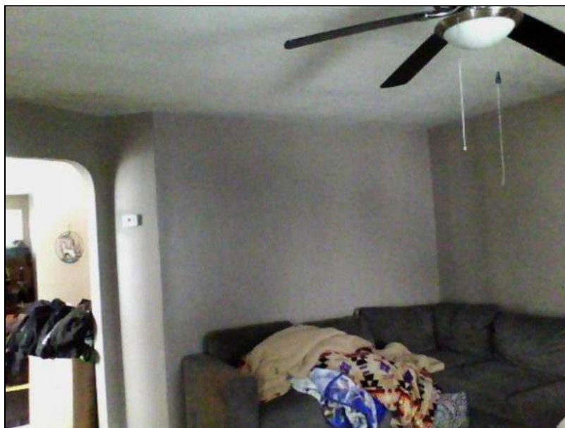
5.1 Item 28(Picture) Interior Walls
