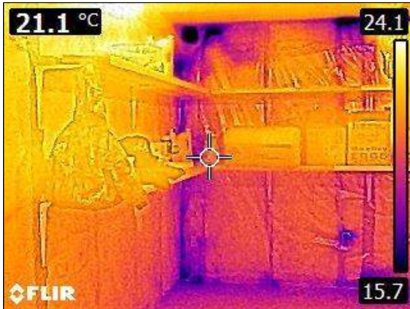
7.0 Item 25(Picture) Basement Foundation
