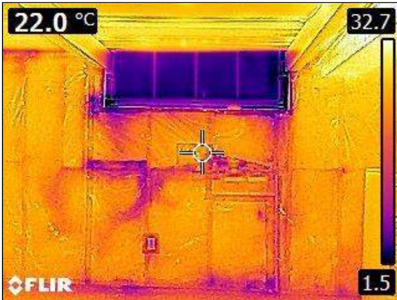
7.0 Item 15(Picture) Basement Foundation
