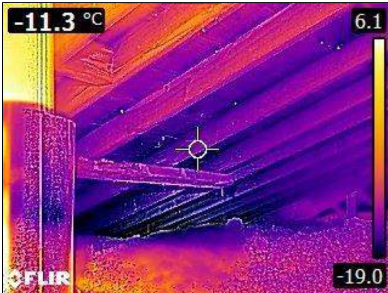
2.0 Item 7(Picture) Attic
