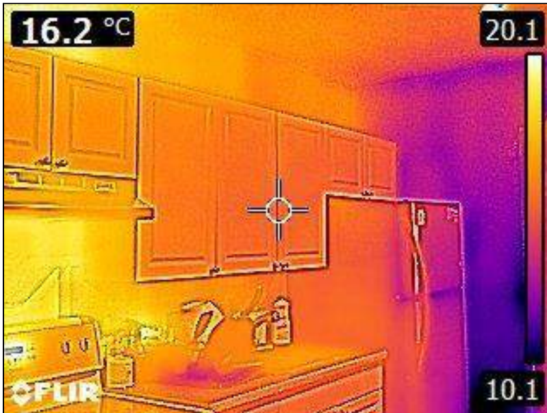
5.1 Item 32(Picture) Interior Walls
