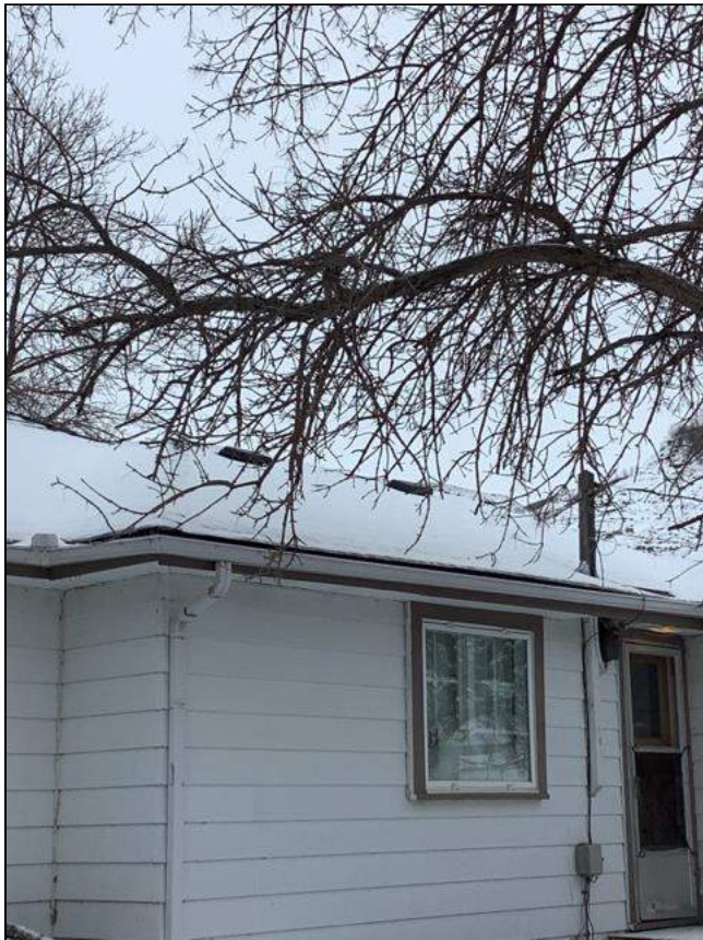
1.0 Item 11(Picture) Roof
