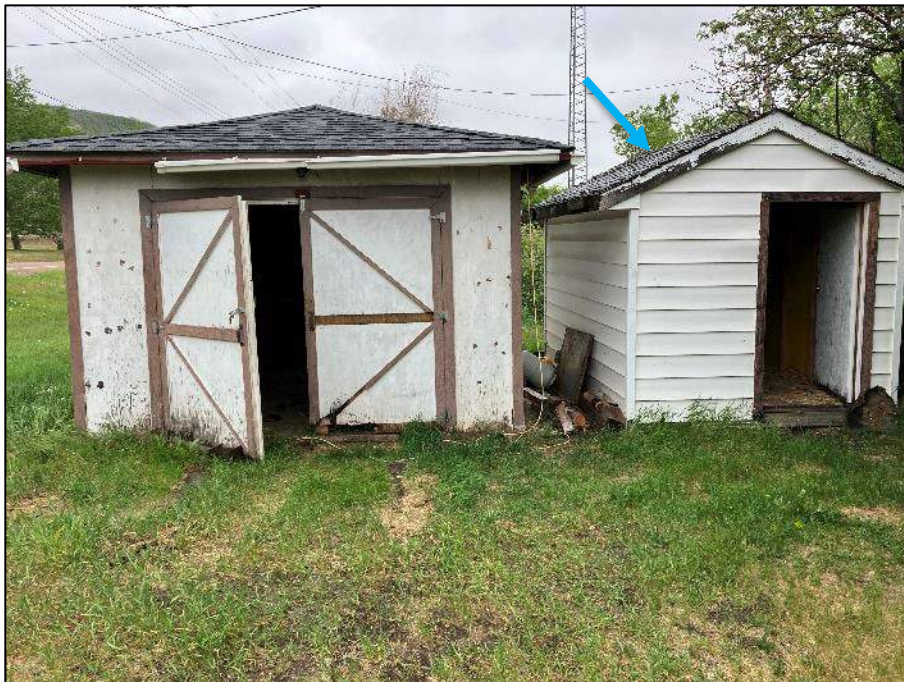
PHOTOGRAPH #20: Roof Shingle – Shed (Non-Asbestos)
