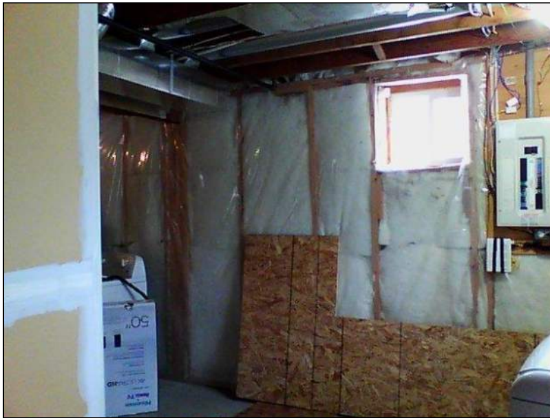
7.0 Item 4(Picture) Basement Foundation
