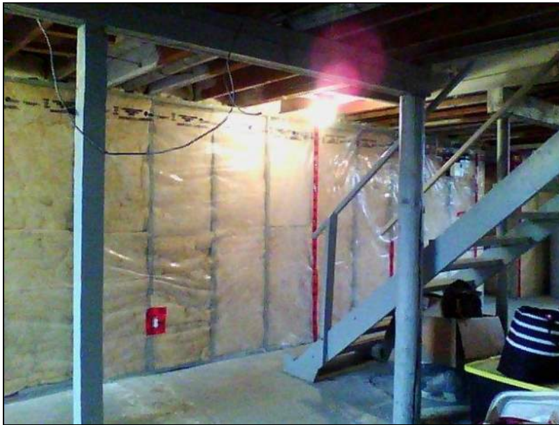
7.0 Item 10(Picture) Basement Foundation
