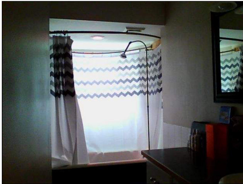
9.0 Item 5(Picture) Bathroom Walls
