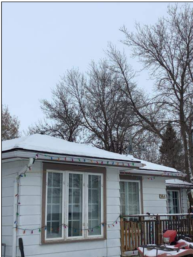
1.0 Item 13(Picture) Roof
