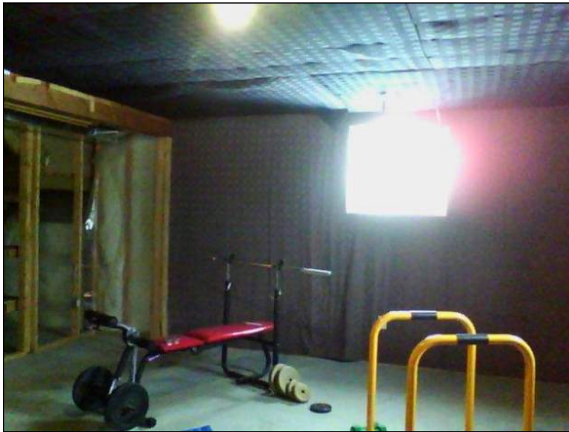
7.0 Item 16(Picture) Basement Foundation
