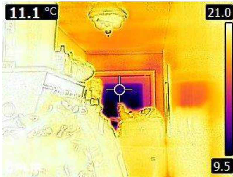
5.1 Item 19(Picture) Interior Walls
