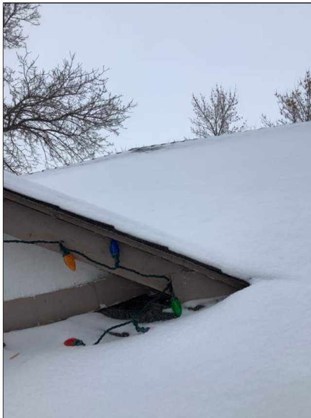
1.0 Item 2(Picture) Roof
