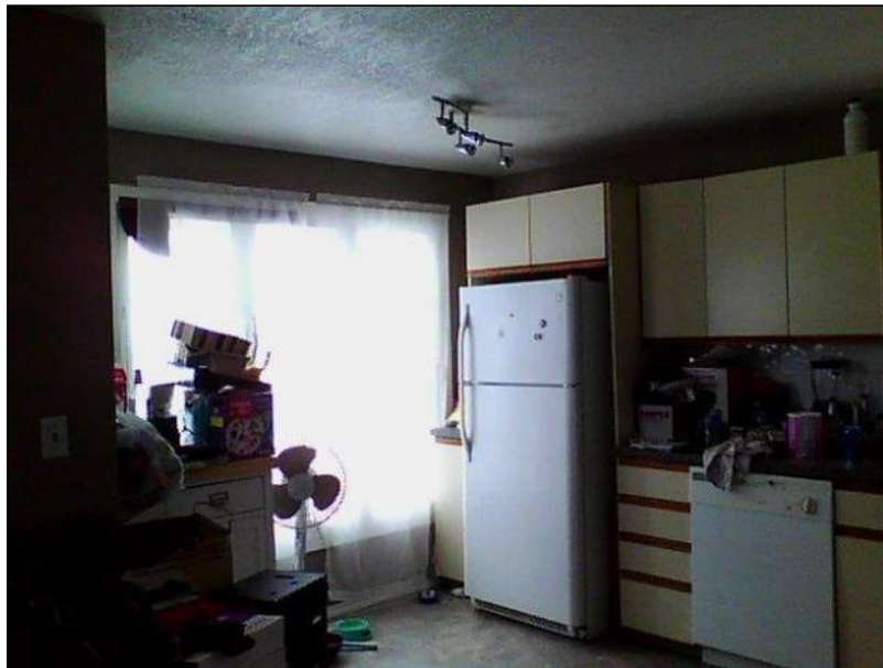
5.1 Item 36(Picture) Interior Walls
