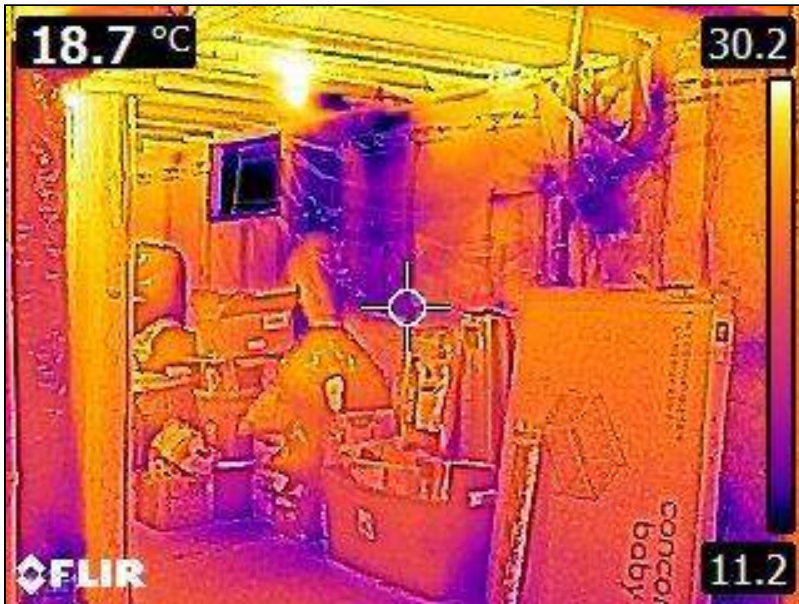
7.0 Item 11(Picture) Basement Foundation
