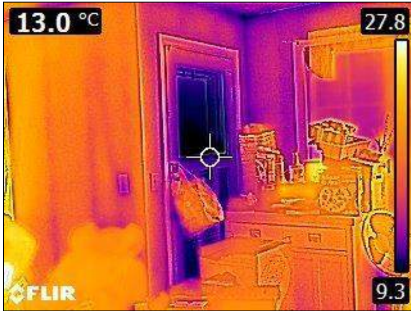
5.1 Item 37(Picture) Interior Walls
