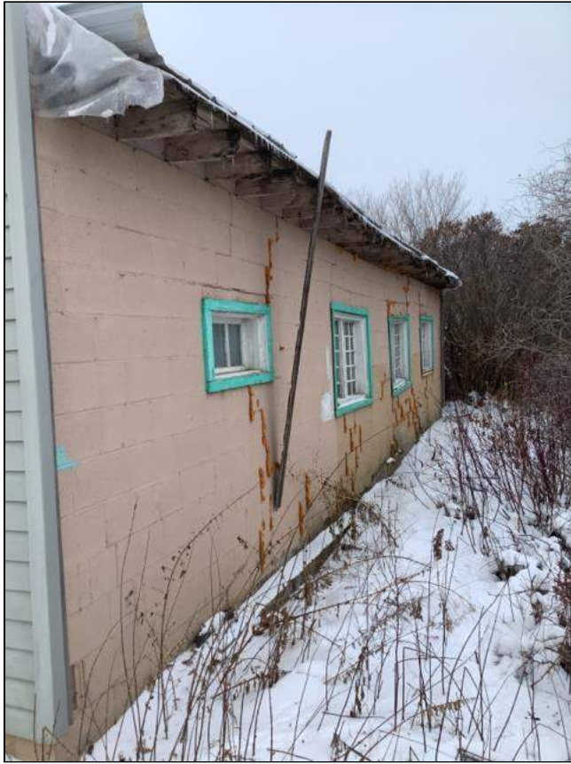
4.4 Item 3(Picture) Garage Exterior
