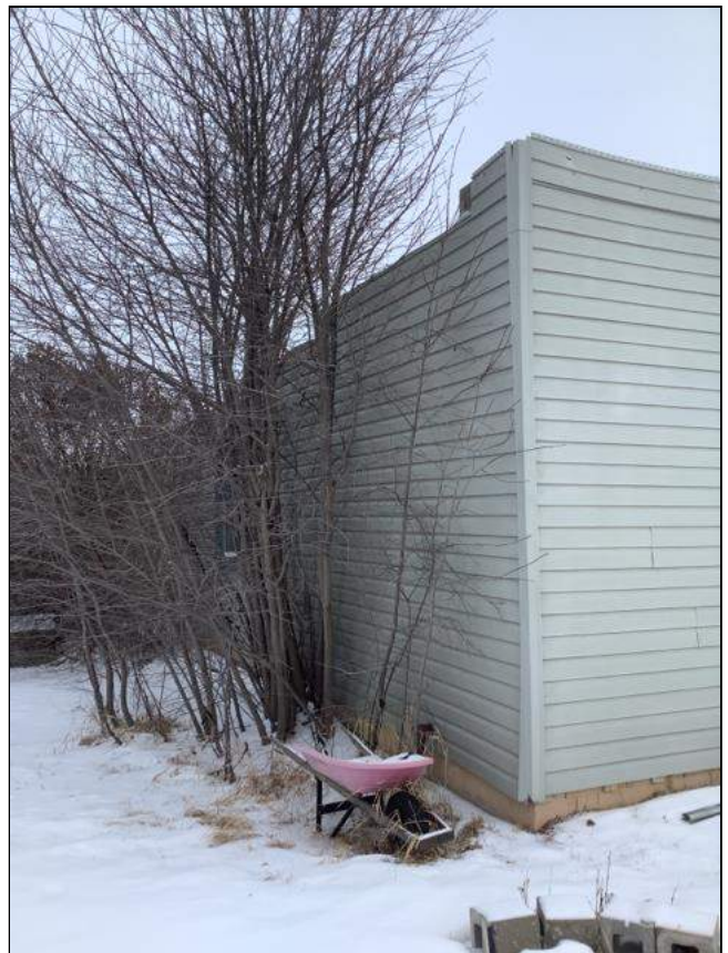
4.4 Item 4(Picture) Garage Exterior
