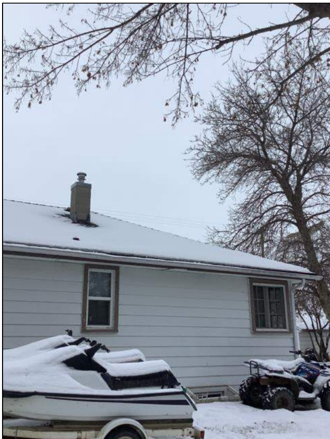
1.0 Item 9(Picture) Roof
