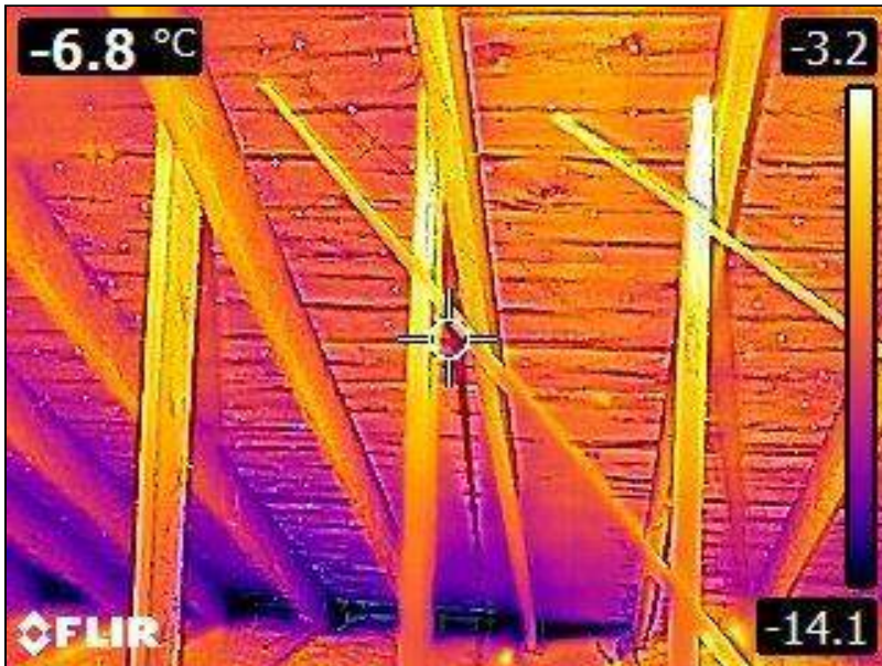
2.0 Item 7(Picture) Attic
