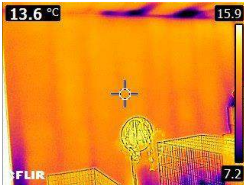
5.1 Item 10(Picture) Interior Walls
