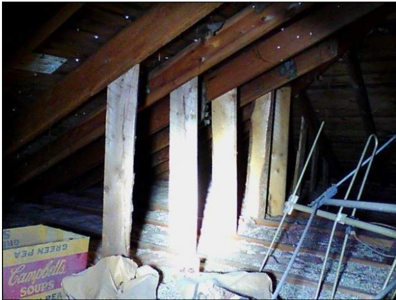
2.0 Item 14(Picture) Attic
