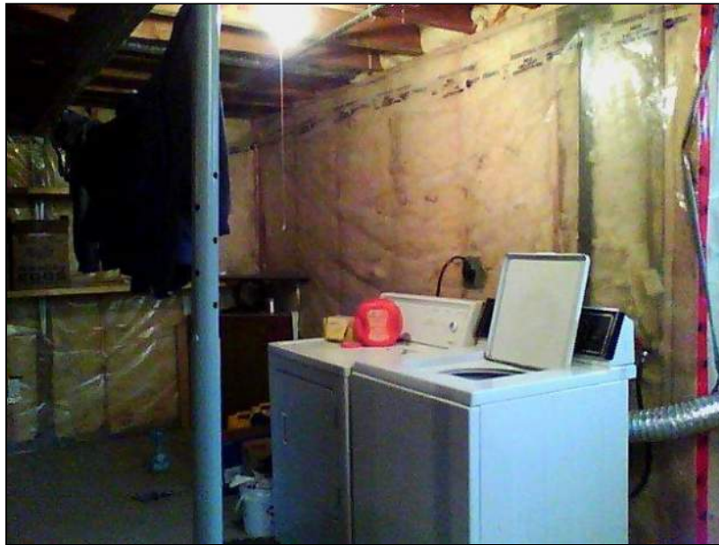
7.0 Item 24(Picture) Basement Foundation
