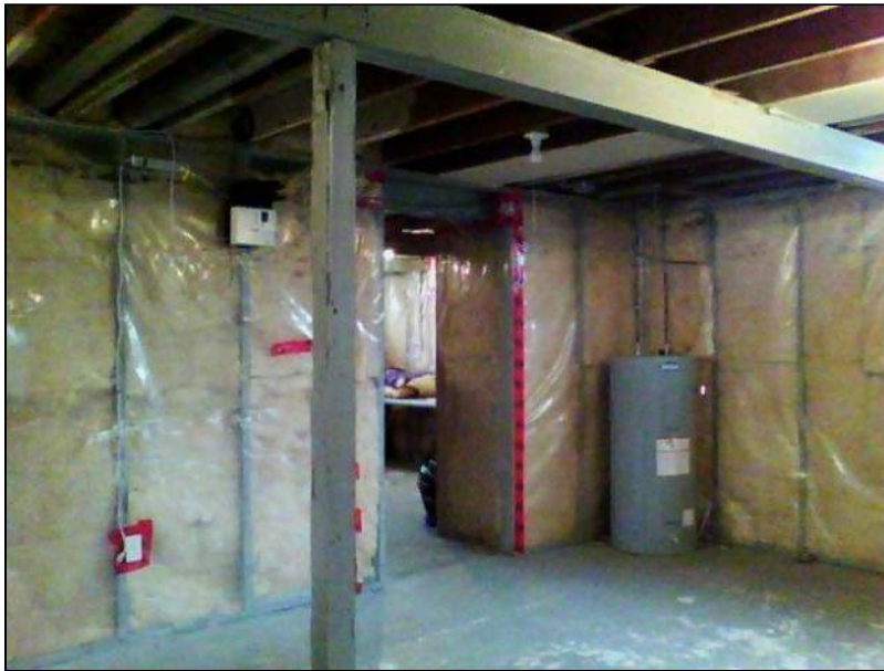
7.0 Item 14(Picture) Basement Foundation
