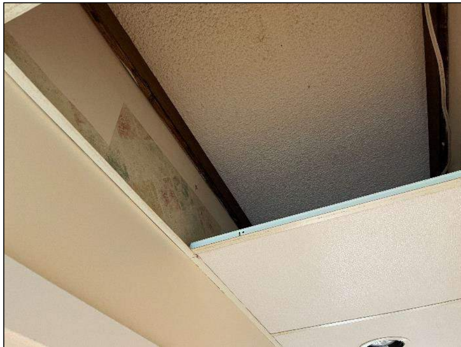
PHOTOGRAPH #4: Drywall Joint Compound - Level 1 SW Hallway (Non-Asbestos)
