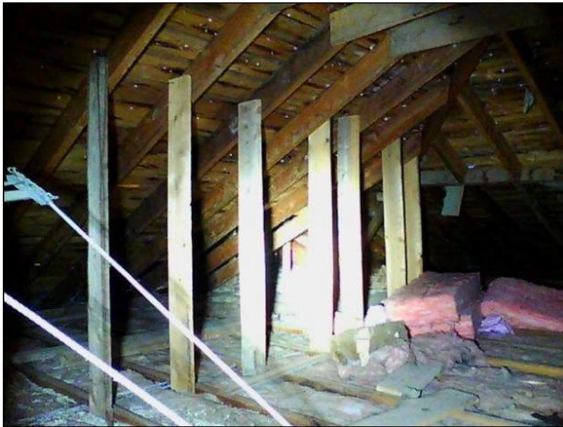
2.0 Item 6(Picture) Attic
