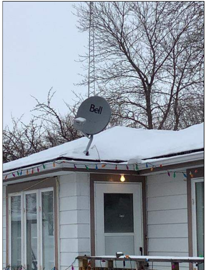
1.0 Item 4(Picture) Roof
