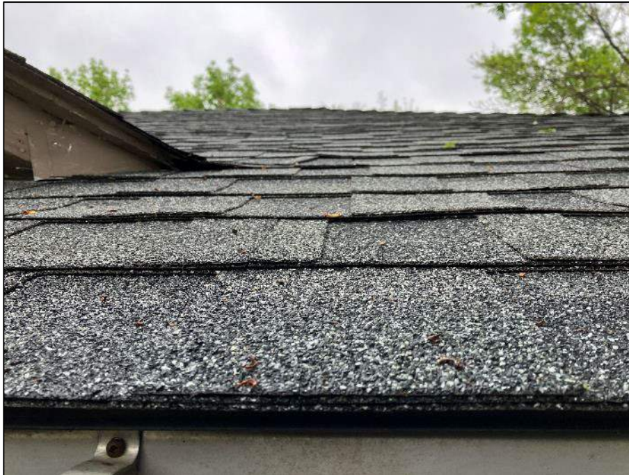
PHOTOGRAPH #19: Roof Shingle – Exterior (Non-Asbestos)
