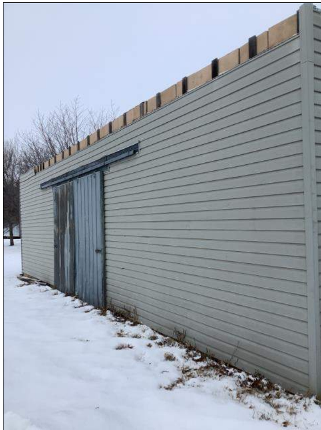
4.4 Item 2(Picture) Garage Exterior
