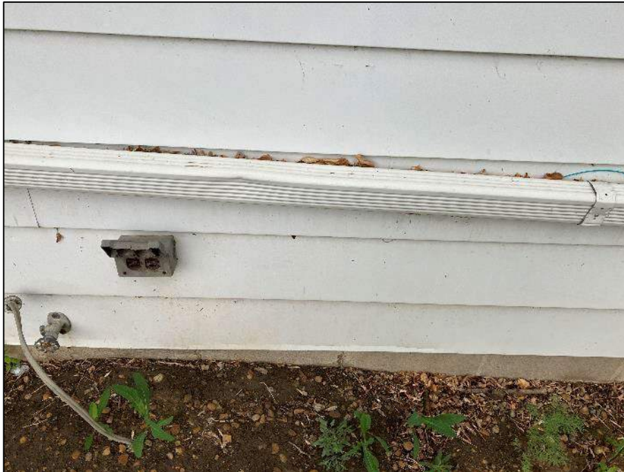
PHOTOGRAPH #17: Parging 1 – Exterior (Non-Asbestos)
