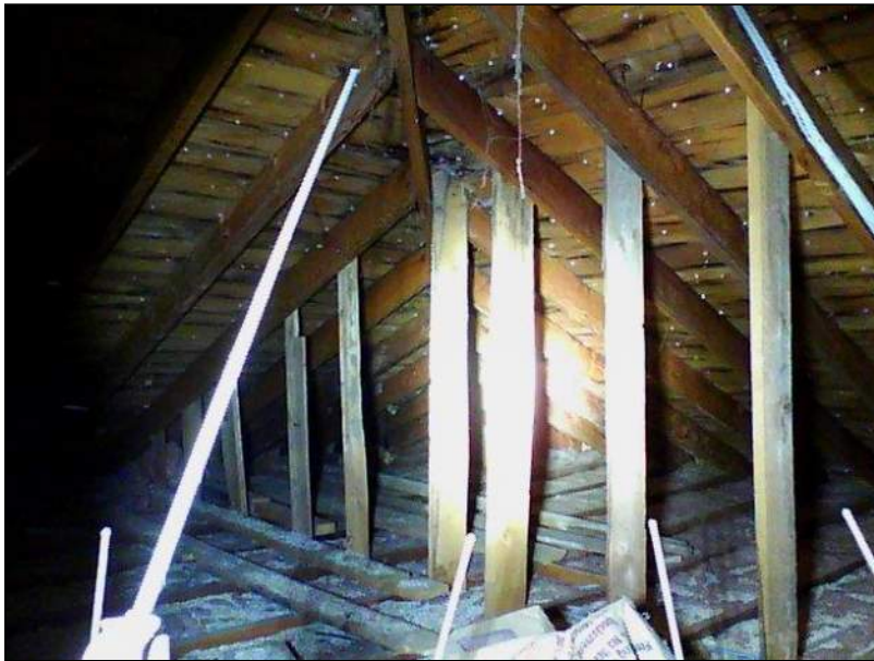
2.0 Item 10(Picture) Attic
