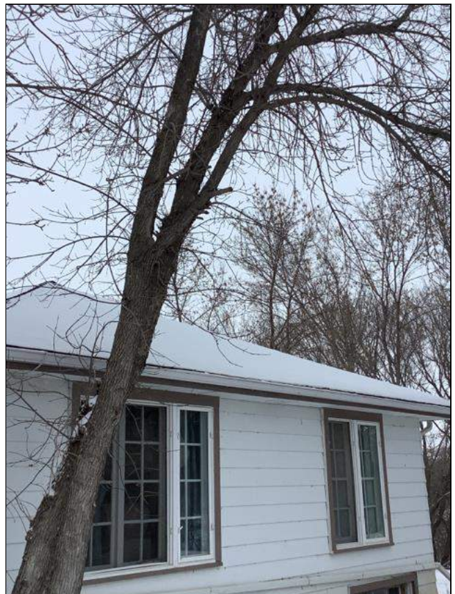
1.0 Item 6(Picture) Roof
