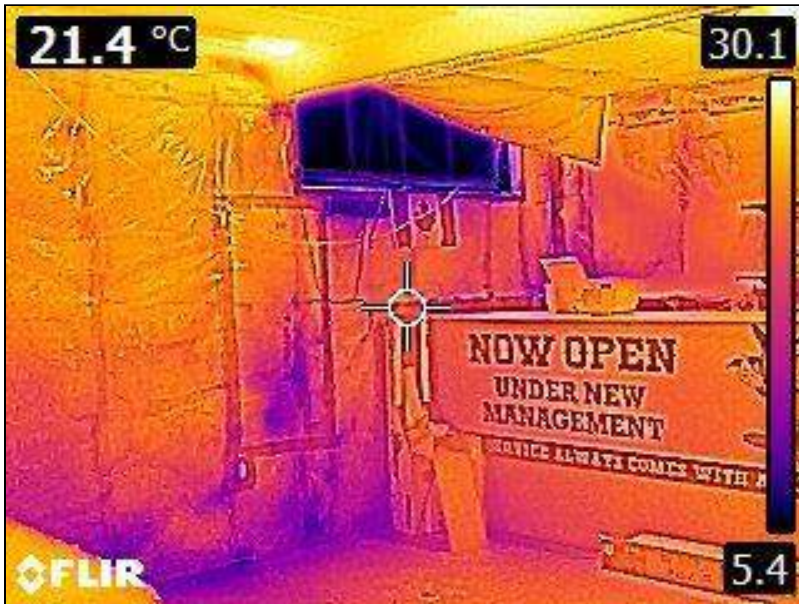
7.0 Item 5(Picture) Basement Foundation
