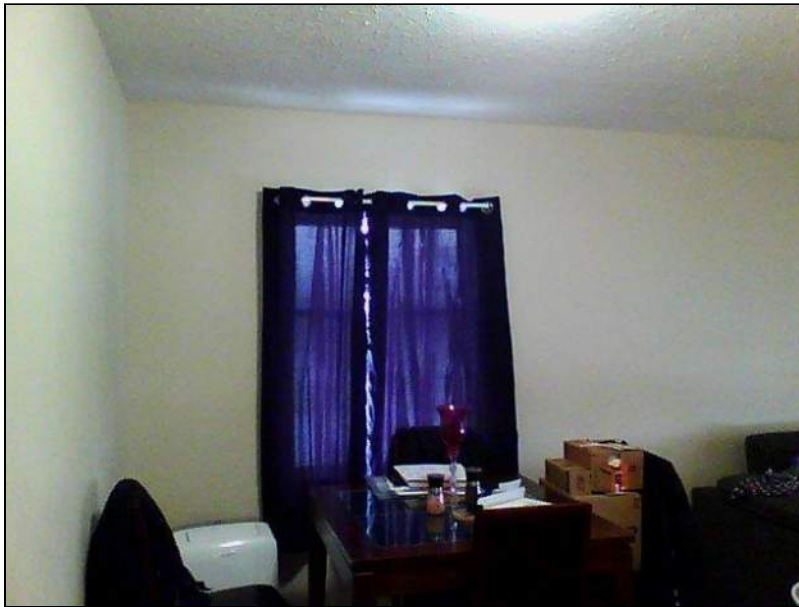
5.1 Item 31(Picture) Interior Walls
