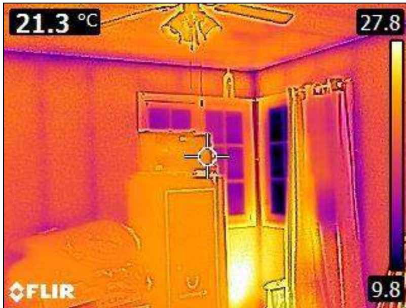
5.1 Item 9(Picture) Interior Walls
