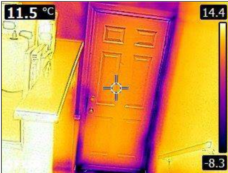
5.1 Item 40(Picture) Interior Walls
