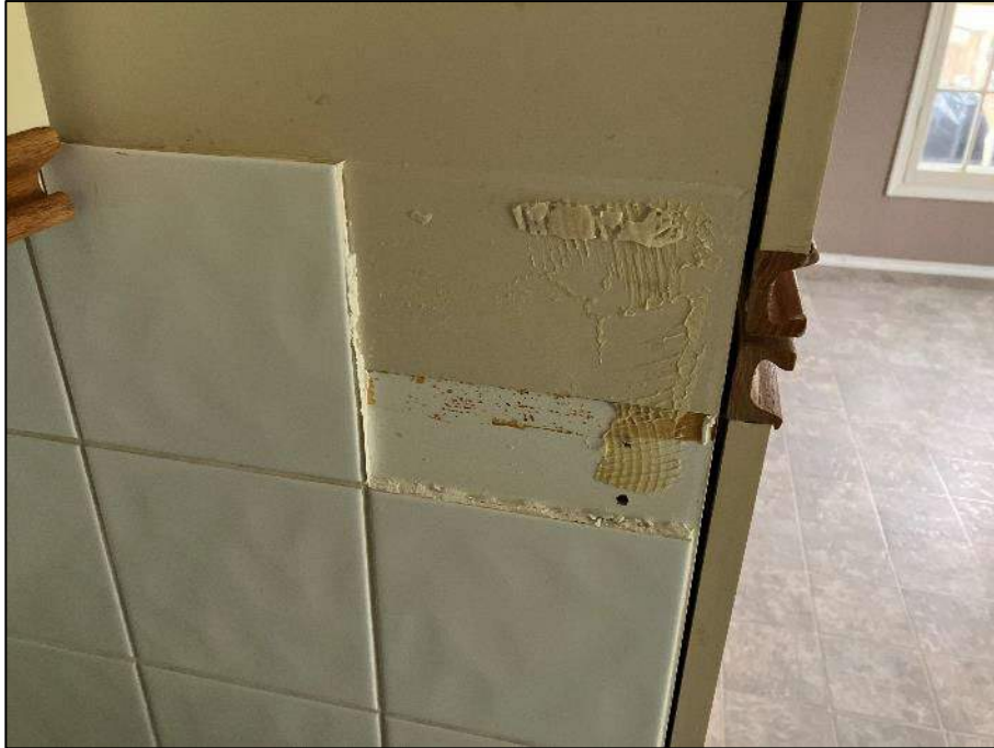
PHOTOGRAPH #13: Thinset – Kitchen (Non-Asbestos)
