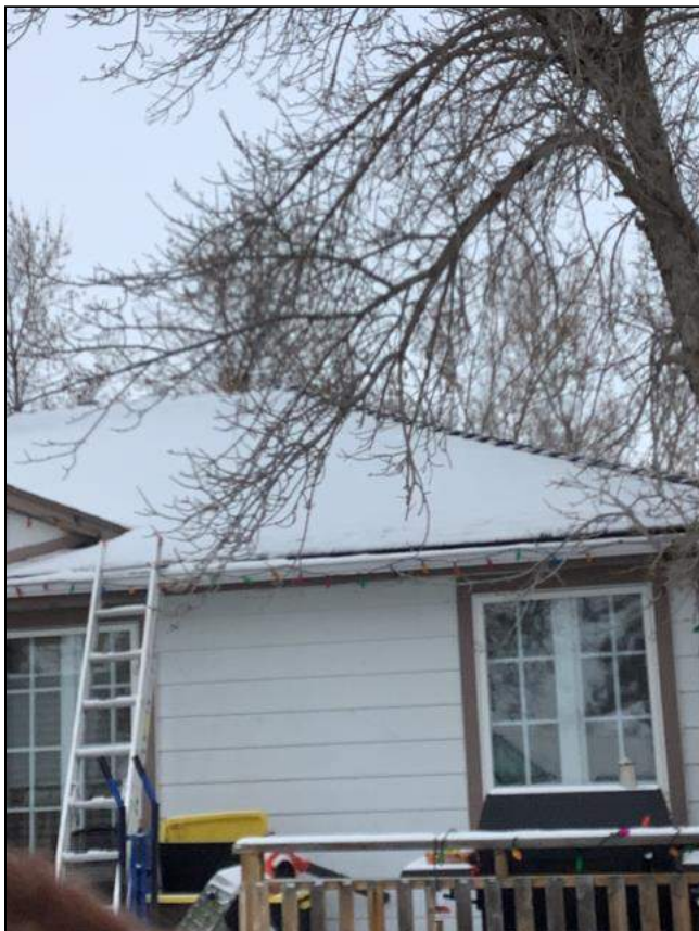
1.0 Item 5(Picture) Roof
