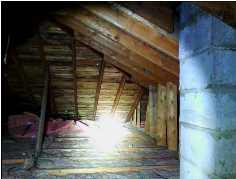
2.0 Item 2(Picture) Attic
