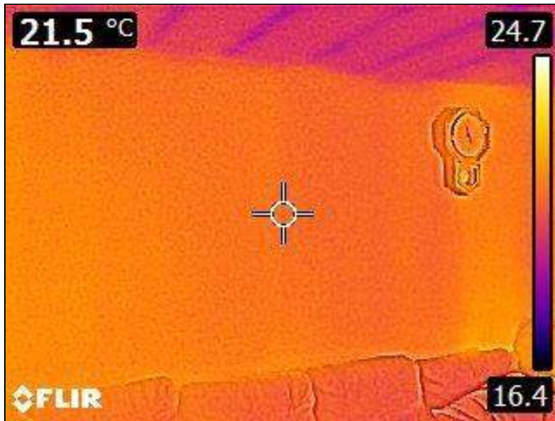
5.1 Item 21(Picture) Interior Walls
