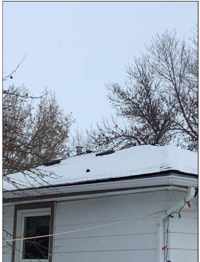
1.0 Item 12(Picture) Roof
