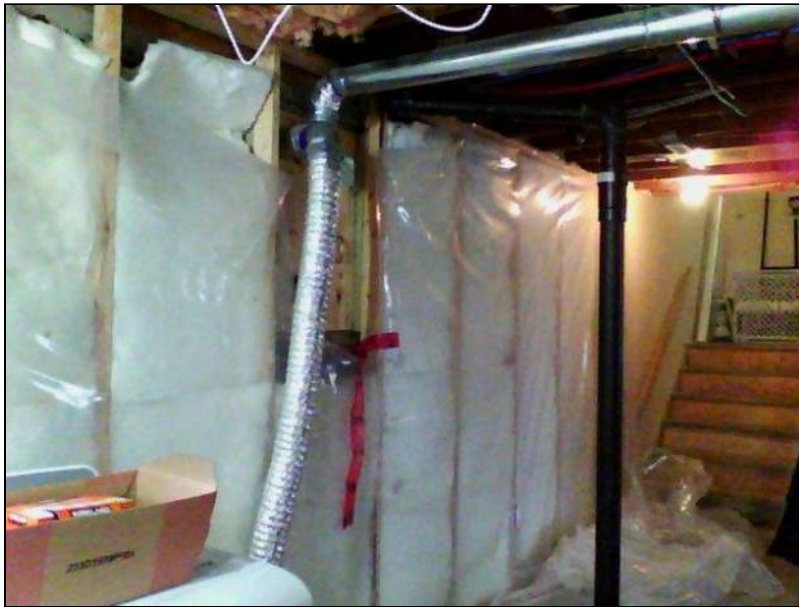
7.0 Item 8(Picture) Basement Foundation
