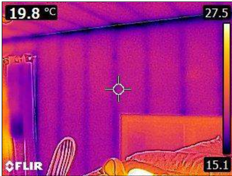
5.1 Item 7(Picture) Interior Walls
