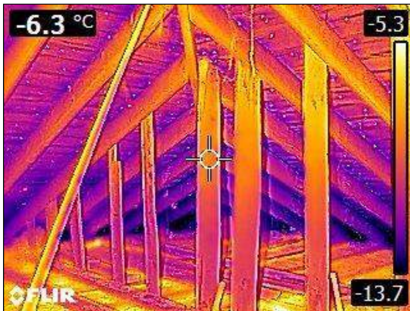
2.0 Item 9(Picture) Attic
