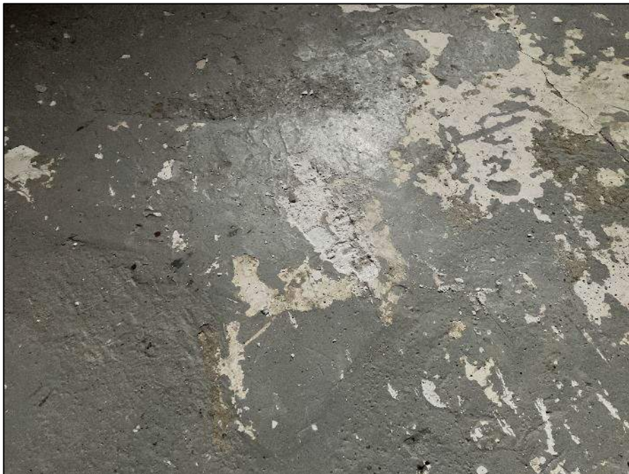
PHOTOGRAPH #14: Leveling Compound – Basement (Non-Asbestos)
