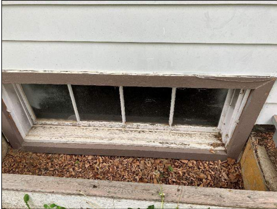
PHOTOGRAPH #15: Window Caulking – Exterior (Non-Asbestos)
