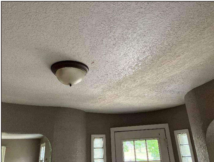
PHOTOGRAPH #10: Ceiling Texture - Floor 1 Foyer (Non-Asbestos)
