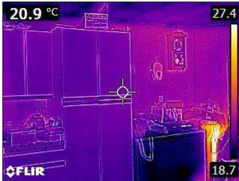
5.1 Item 43(Picture) Interior Walls
