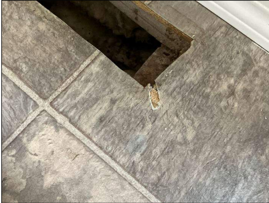
PHOTOGRAPH #11: Sheet Flooring – Floor 1 Kitchen (Non-Asbestos)
