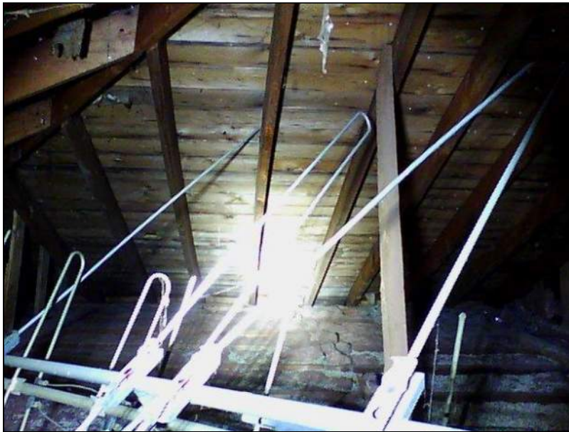
2.0 Item 16(Picture) Attic
