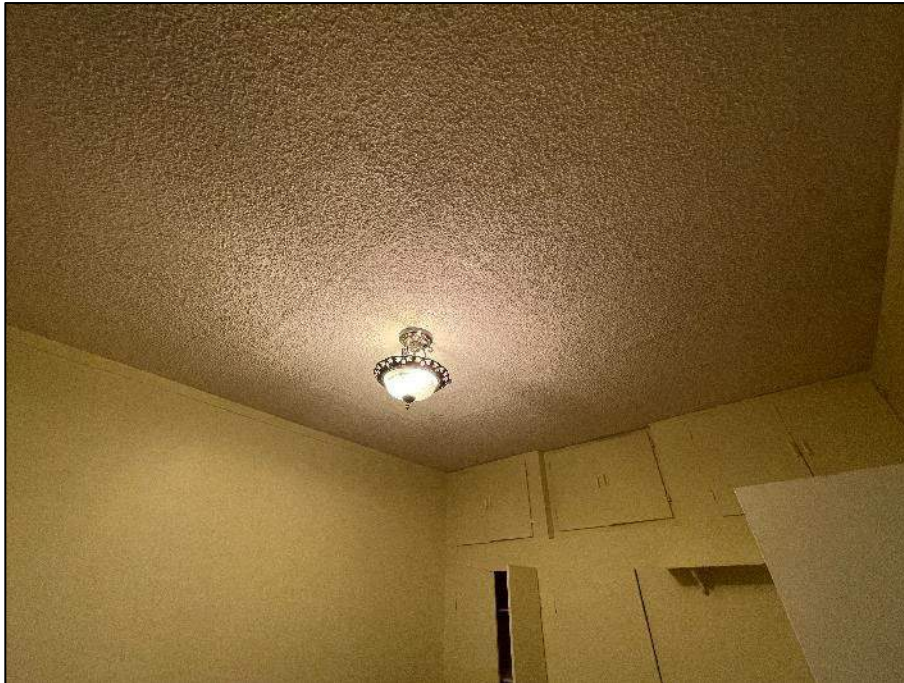
PHOTOGRAPH #9: Ceiling Texture - Level 1 SW Bedroom (Non-Asbestos)
