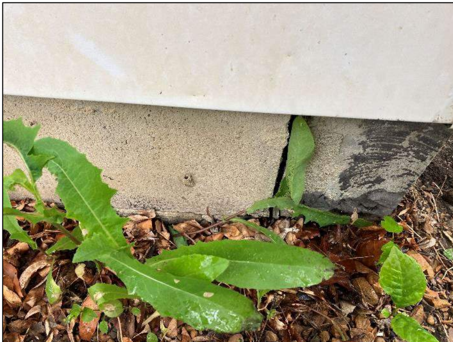
PHOTOGRAPH #18: Parging 2 – Exterior (Non-Asbestos)
