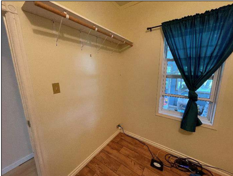
PHOTOGRAPH #1: Drywall Joint Compound - Level 1 SW Bedroom (Non-Asbestos)
