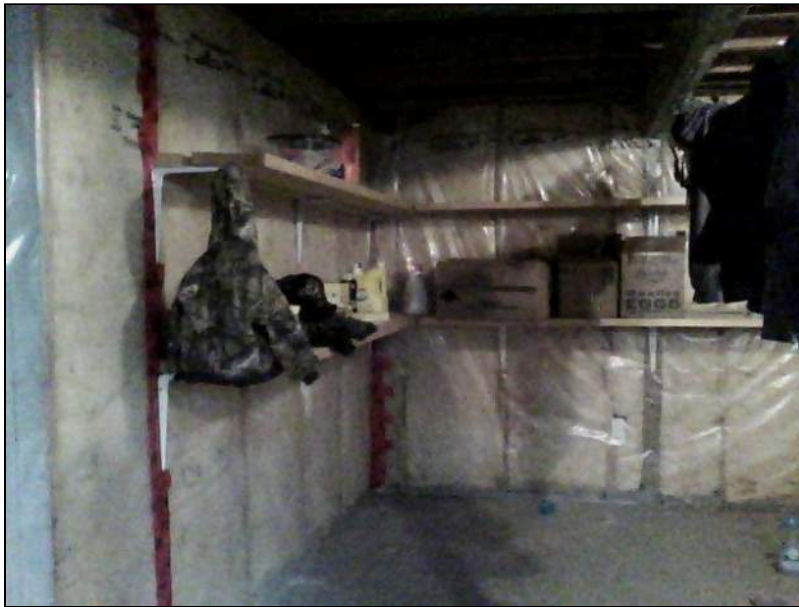
7.0 Item 26(Picture) Basement Foundation
