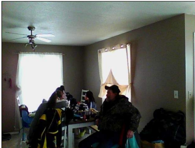
5.1 Item 40(Picture) Interior Walls
