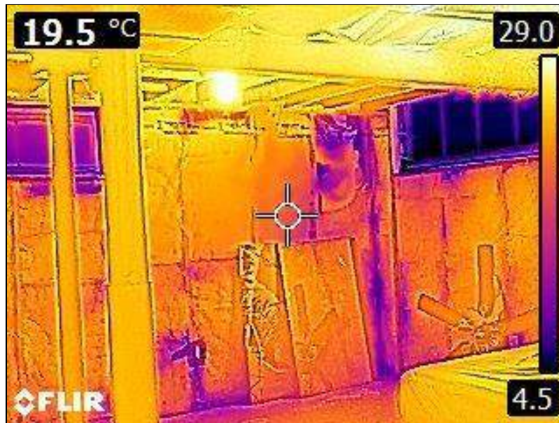
7.0 Item 1(Picture) Basement Foundation
