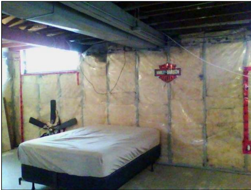
7.0 Item 4(Picture) Basement Foundation
