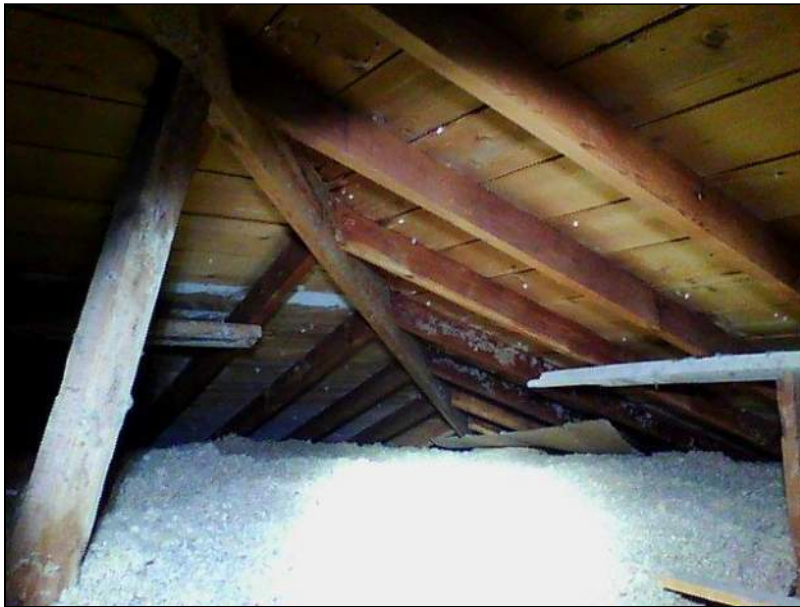
2.0 Item 12(Picture) Attic
