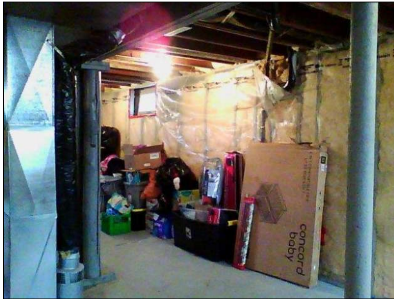
7.0 Item 12(Picture) Basement Foundation
