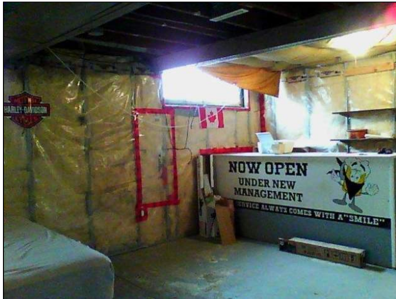
7.0 Item 6(Picture) Basement Foundation
