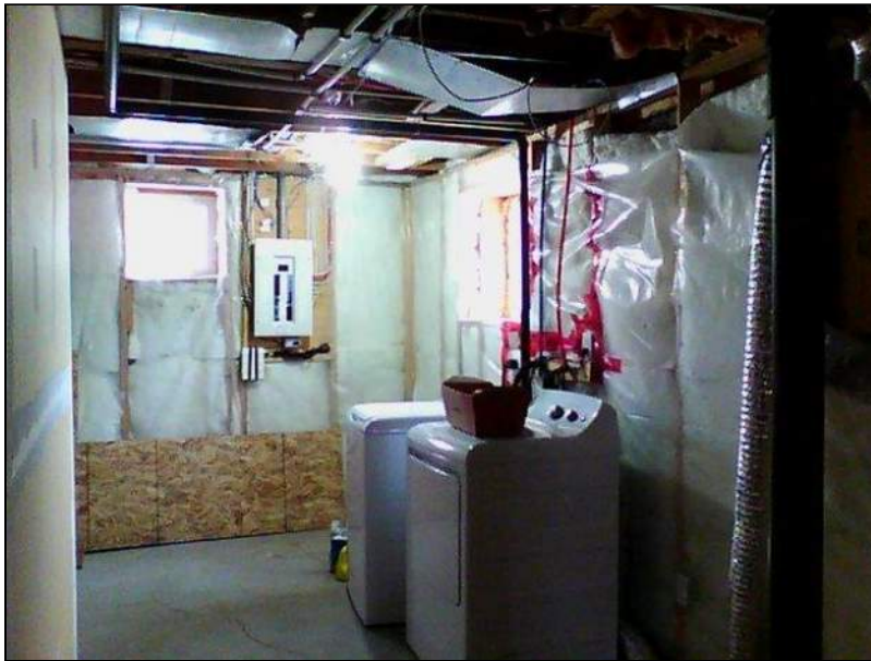
7.0 Item 2(Picture) Basement Foundation
