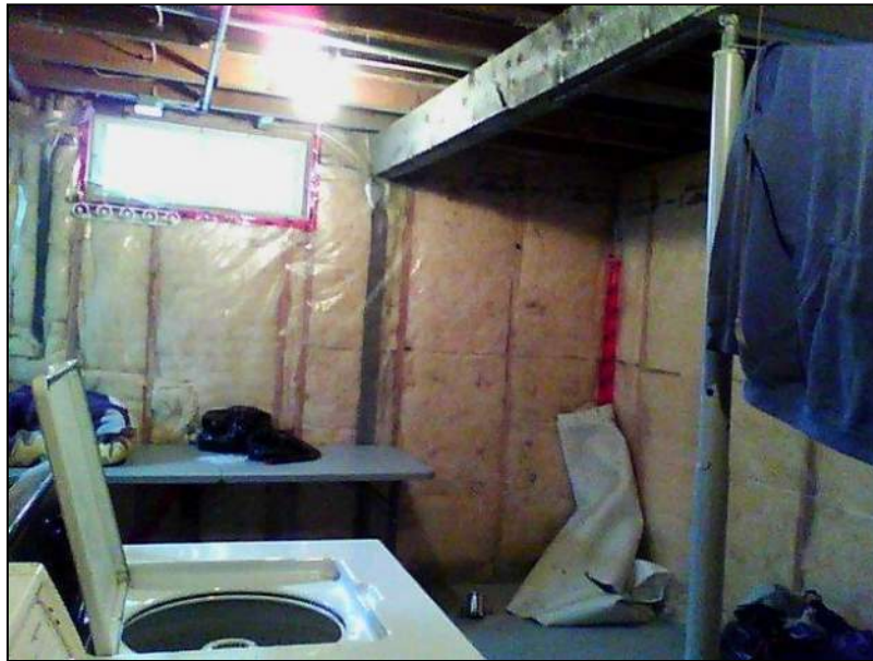
7.0 Item 28(Picture) Basement Foundation
