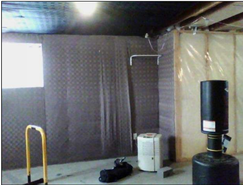
7.0 Item 12(Picture) Basement Foundation
