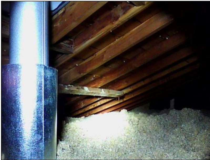
2.0 Item 8(Picture) Attic
