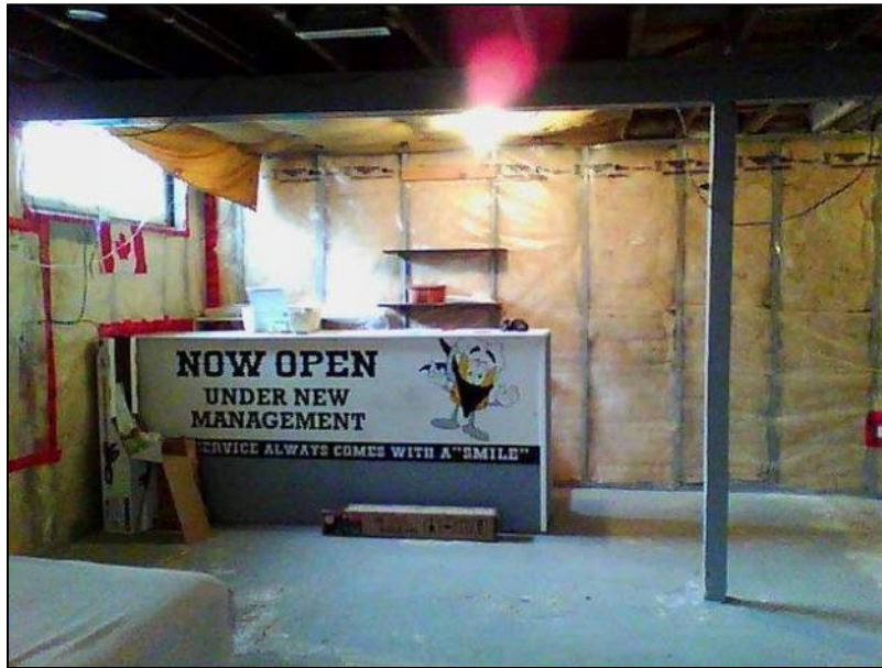
7.0 Item 8(Picture) Basement Foundation
