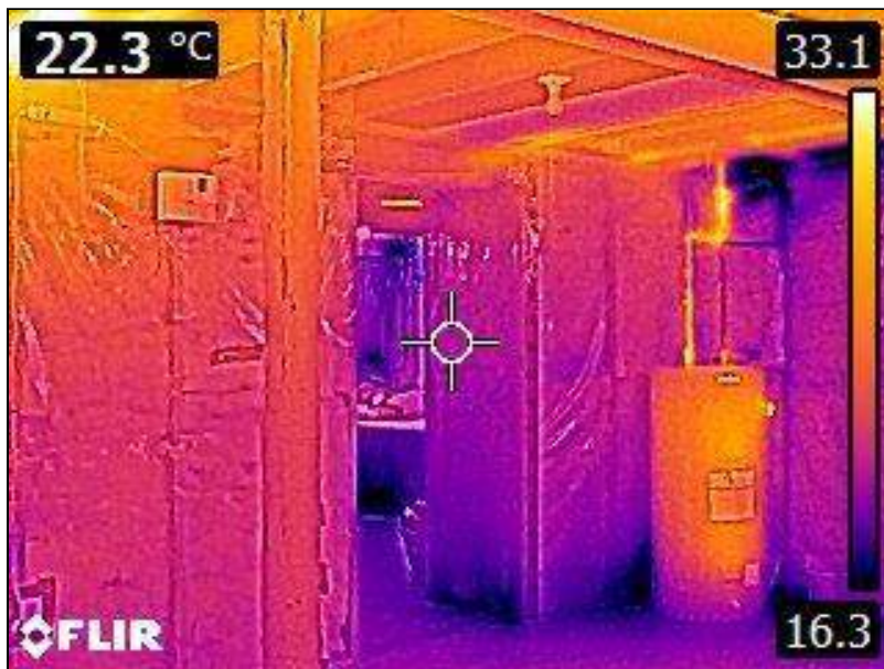
7.0 Item 13(Picture) Basement Foundation
