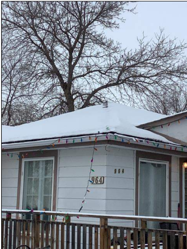
1.0 Item 3(Picture) Roof
