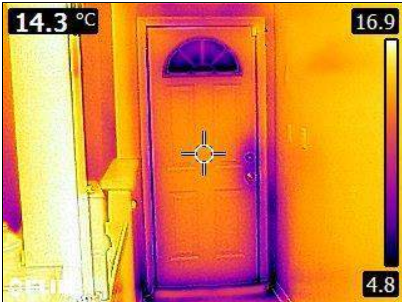
5.1 Item 22(Picture) Interior Walls
