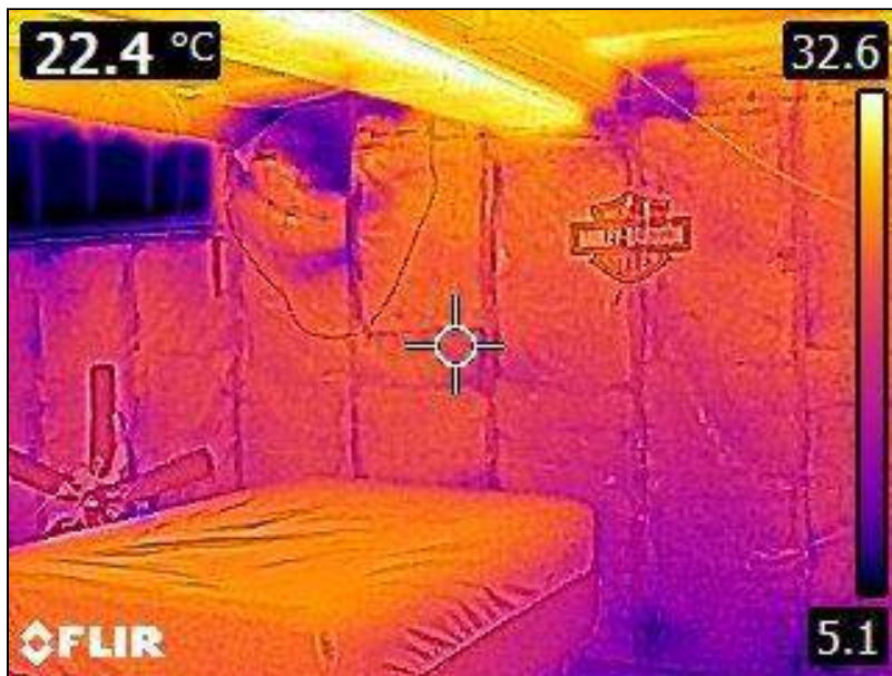
7.0 Item 3(Picture) Basement Foundation
