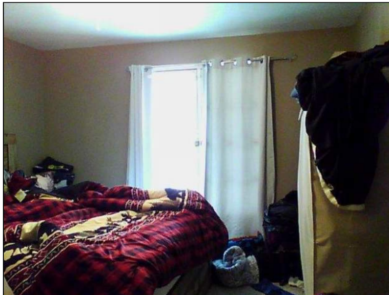
5.1 Item 4(Picture) Interior Walls
