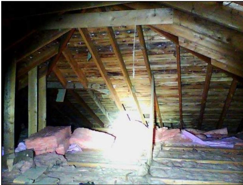
2.0 Item 4(Picture) Attic
