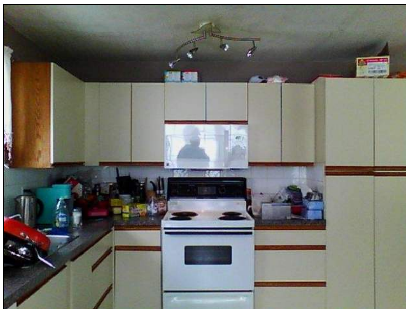
5.1 Item 46(Picture) Interior Walls
