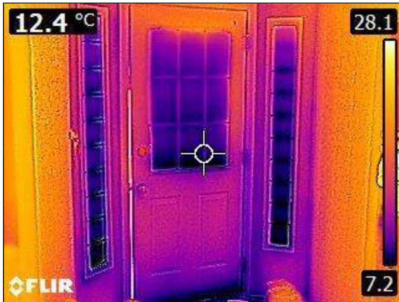
5.1 Item 31(Picture) Interior Walls
