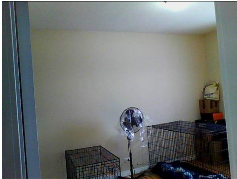
5.1 Item 11(Picture) Interior Walls
