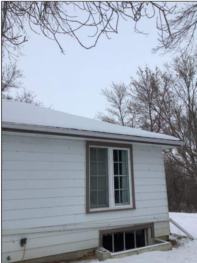
1.0 Item 7(Picture) Roof
