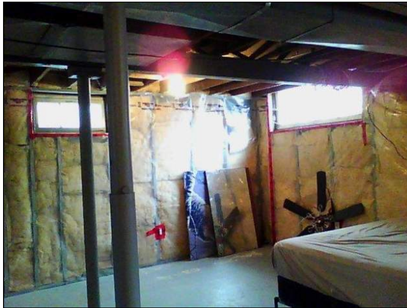
7.0 Item 2(Picture) Basement Foundation
