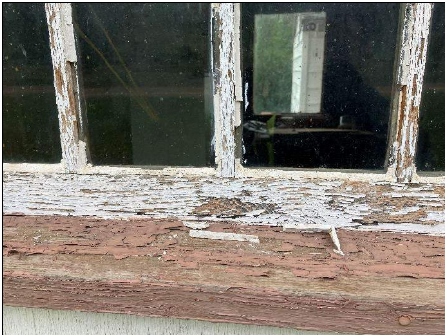
PHOTOGRAPH #16: Window Caulking – Shed (Non-Asbestos)
