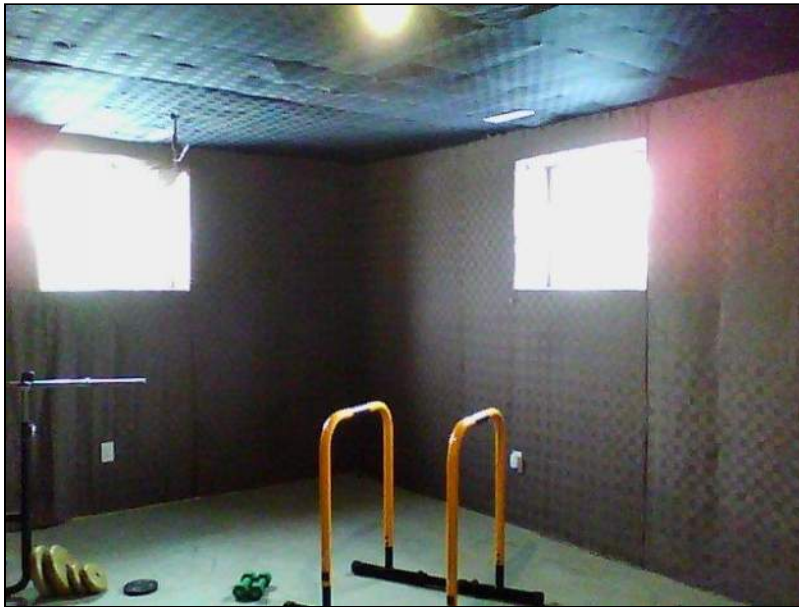
7.0 Item 14(Picture) Basement Foundation
