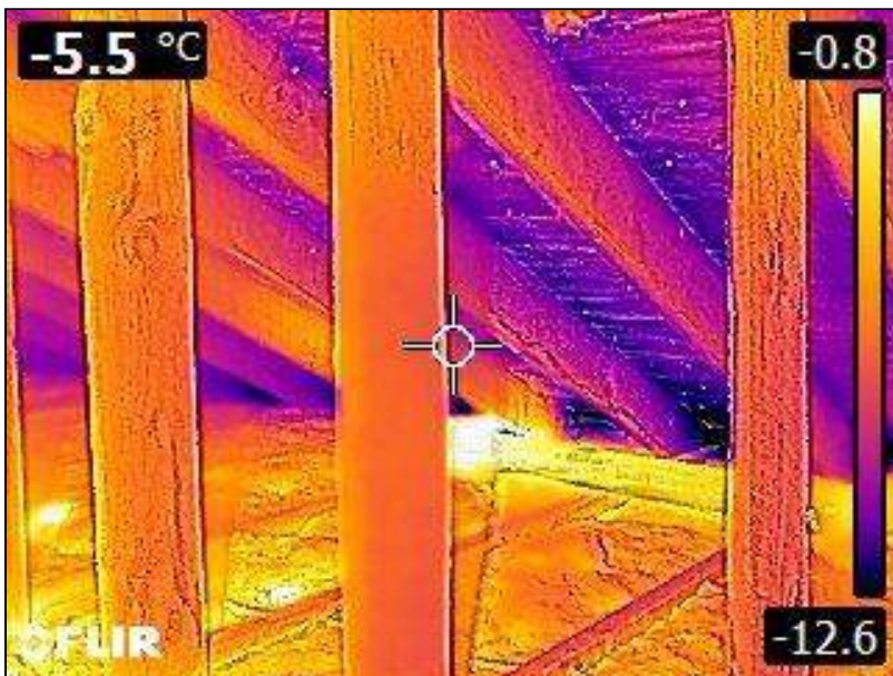
2.0 Item 11(Picture) Attic
