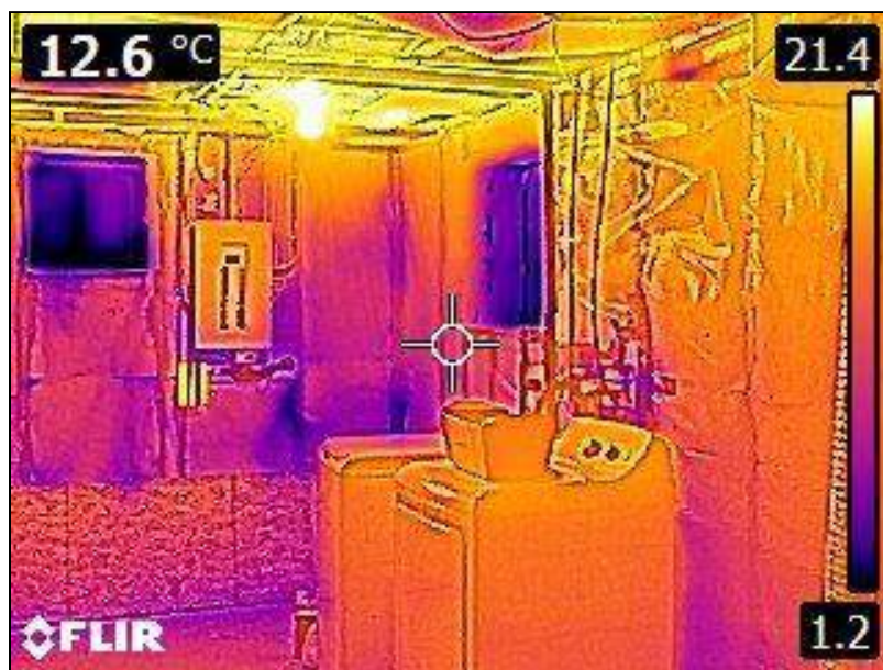
7.0 Item 1(Picture) Basement Foundation
