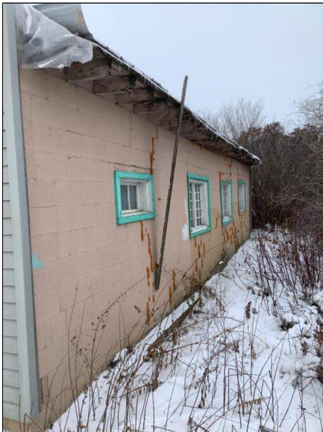
4.4 Item 3(Picture) Garage Exterior
