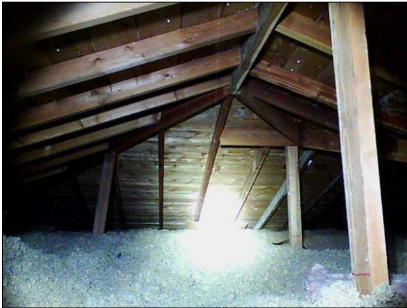
2.0 Item 4(Picture) Attic
