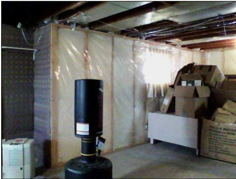
7.0 Item 10(Picture) Basement Foundation
