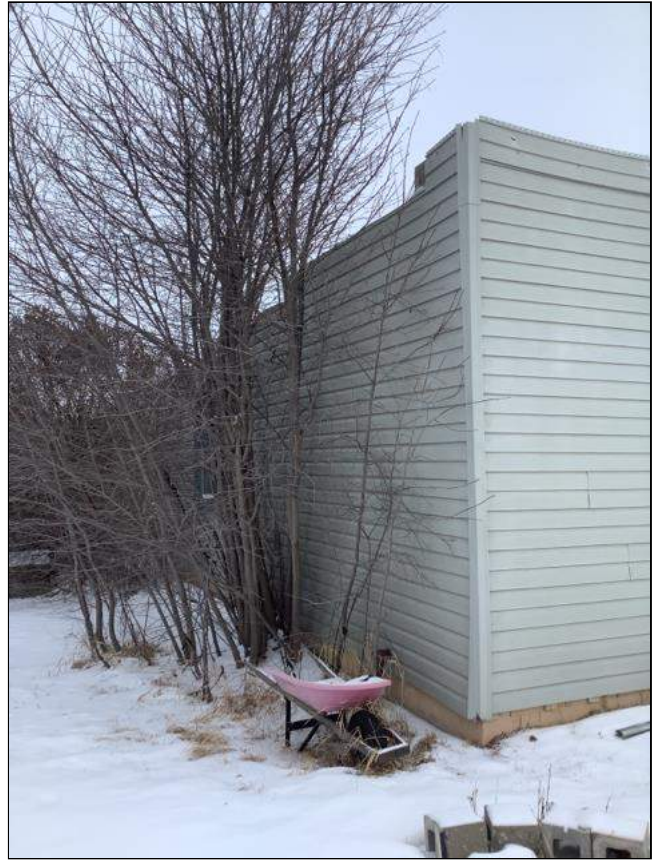
4.4 Item 4(Picture) Garage Exterior
