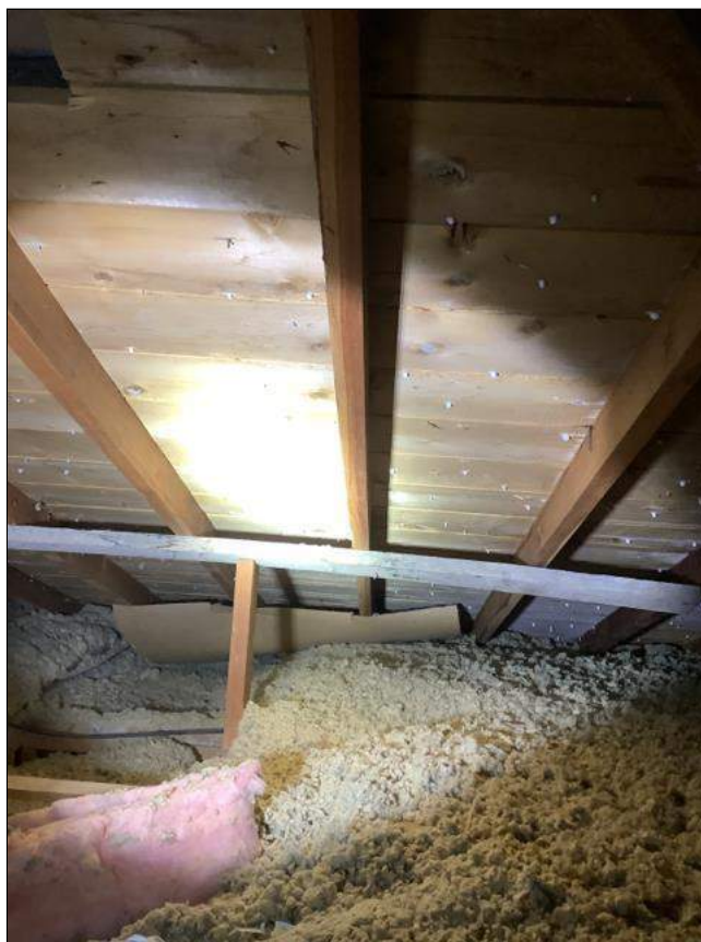
2.3 Item 2(Picture) Rafter - split, cross support bowed
