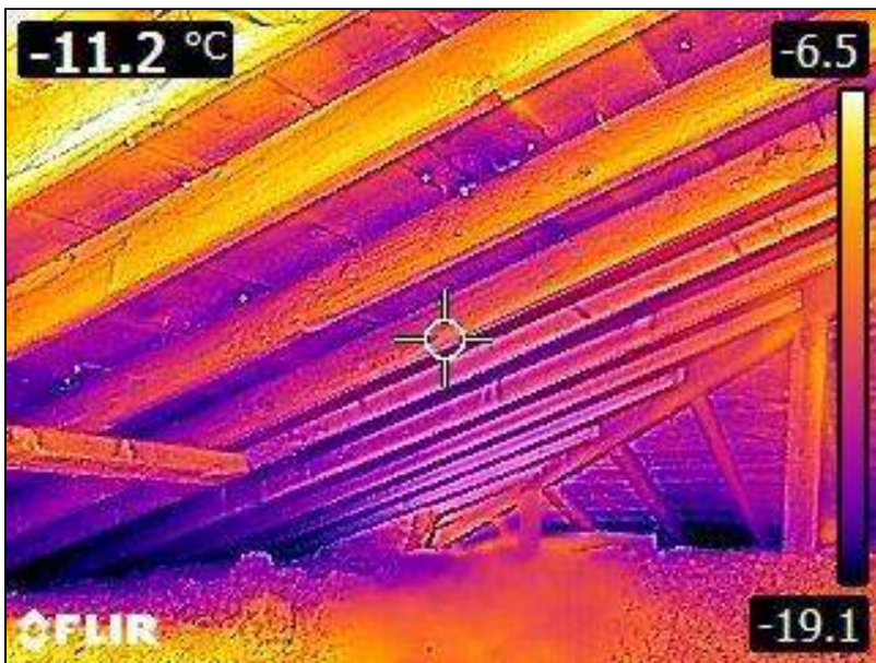
2.0 Item 5(Picture) Attic
