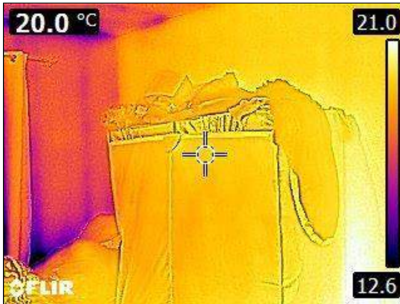
5.1 Item 5(Picture) Interior Walls
