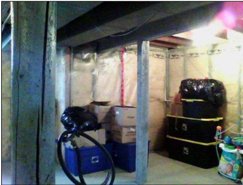
7.0 Item 18(Picture) Basement Foundation
