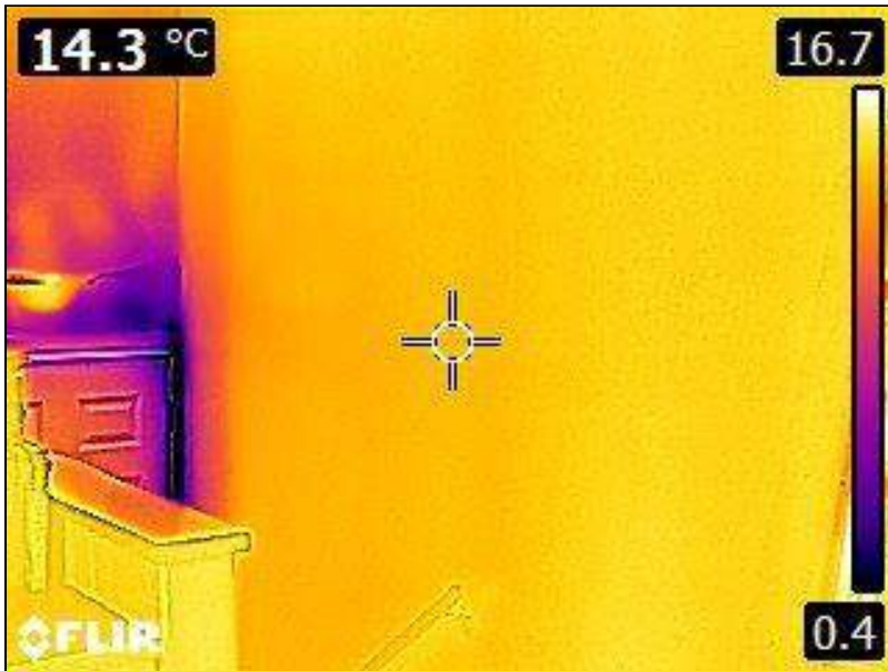
5.1 Item 38(Picture) Interior Walls
