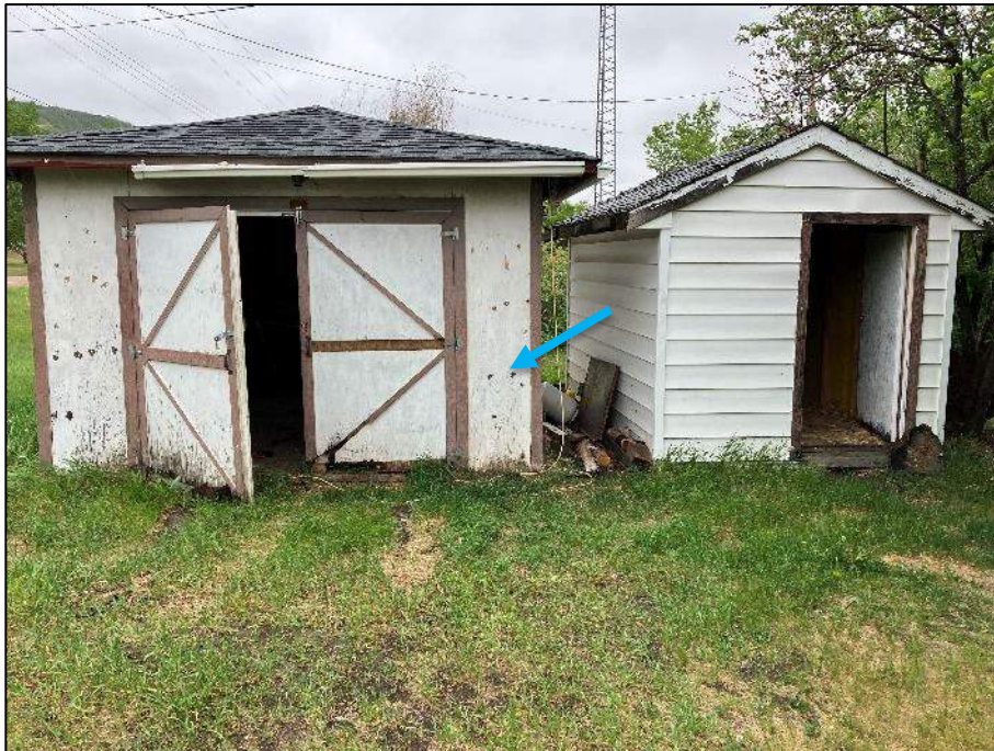
PHOTOGRAPH #27: Paint – White Shed (Non-Lead Based)
