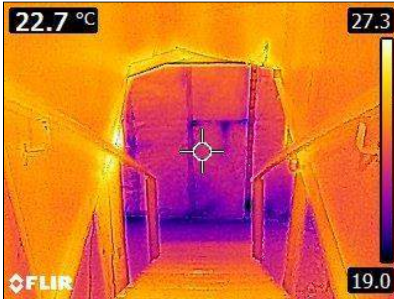
5.1 Item 47(Picture) Interior Walls
