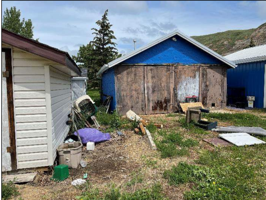
PHOTOGRAPH #17: Stucco - Shed SW Corner (2% Chrysotile)
