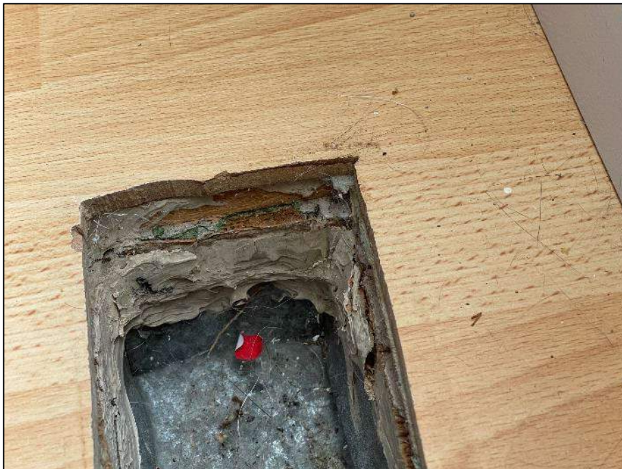
PHOTOGRAPH #12: Flooring - Level 1 Living Room (Non-Asbestos)
