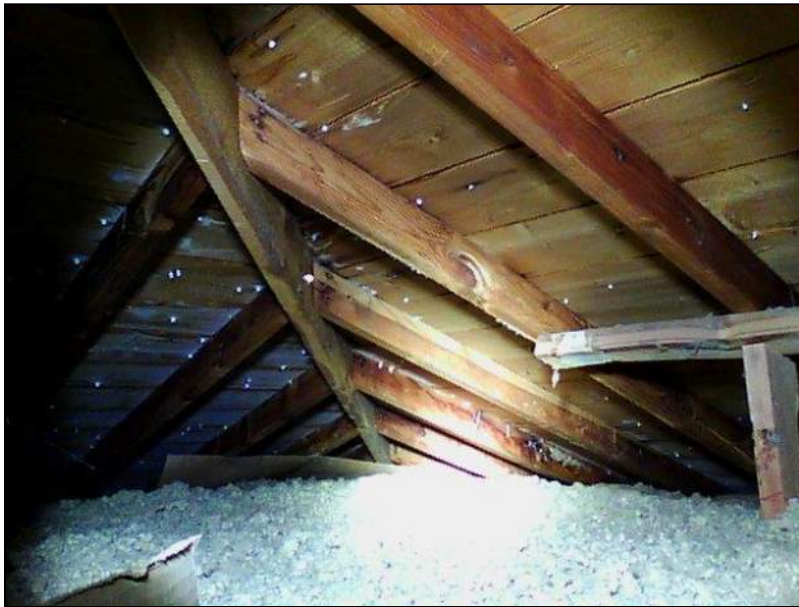
2.0 Item 10(Picture) Attic
