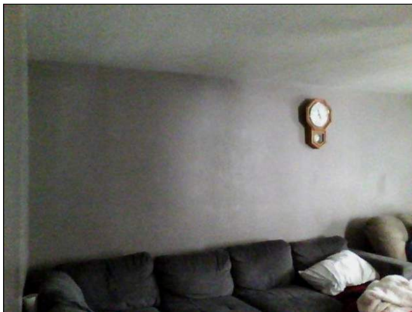
5.1 Item 22(Picture) Interior Walls
