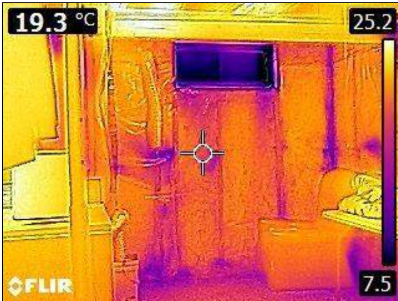
7.0 Item 21(Picture) Basement Foundation
