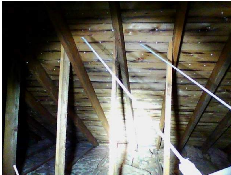
2.0 Item 8(Picture) Attic
