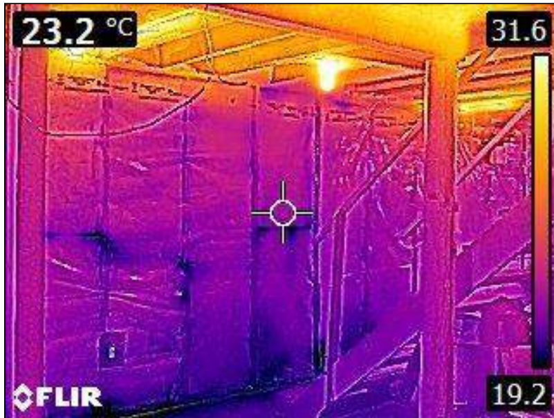
7.0 Item 9(Picture) Basement Foundation
