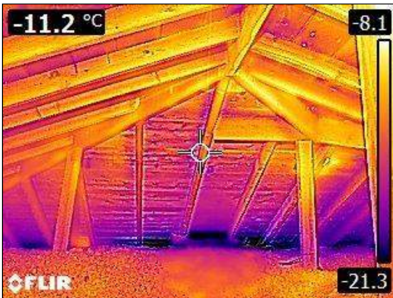
2.0 Item 3(Picture) Attic
