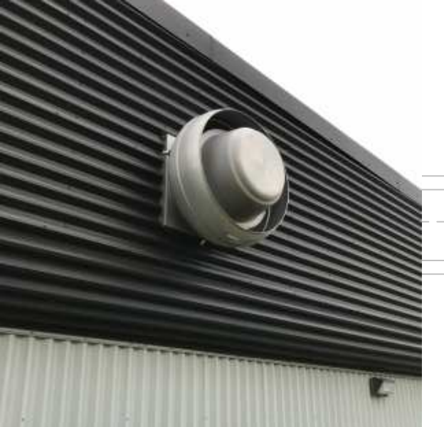
PICTURE #3 - TYPICAL WALL MOUNTED EXHAUST FAN TO BE REMOVED
