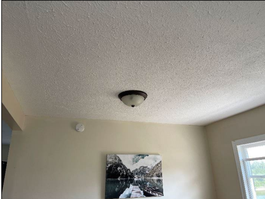
PHOTOGRAPH #19: Ceiling Texture - Level 1 Living Room (Non-Asbestos)
