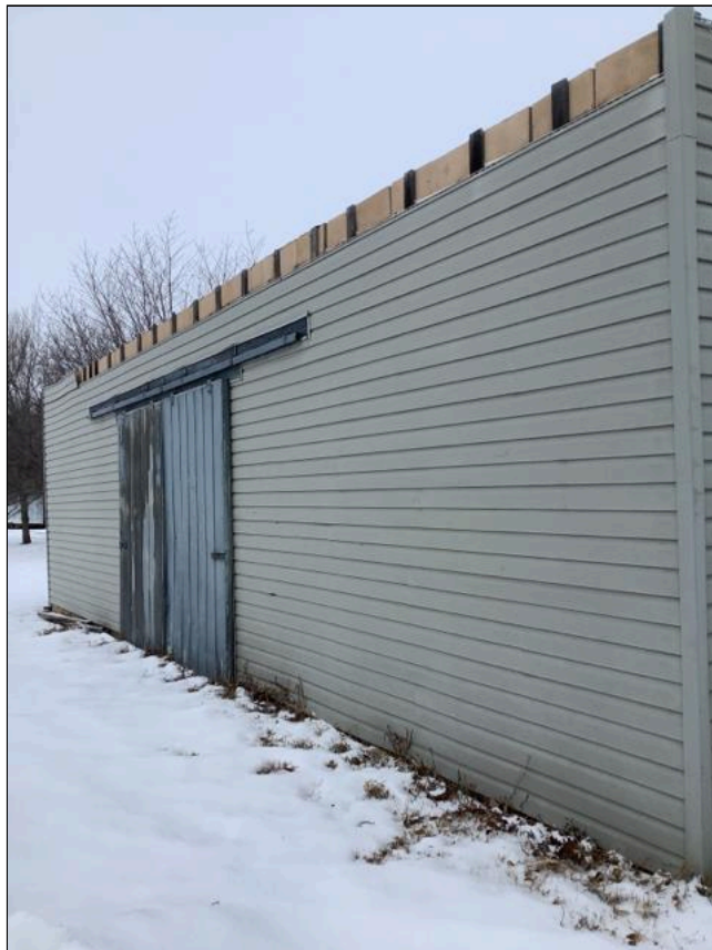
4.4 Item 2(Picture) Garage Exterior
