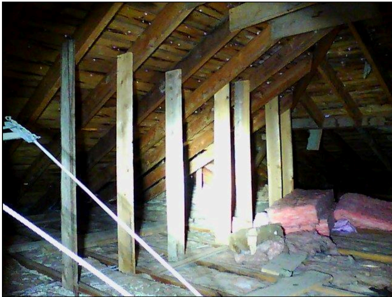
2.0 Item 6(Picture) Attic
