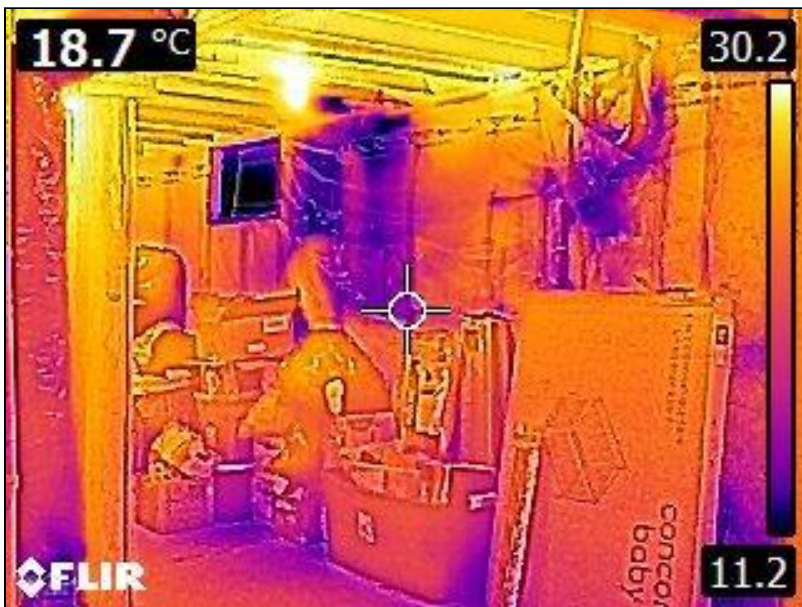
7.0 Item 11(Picture) Basement Foundation
