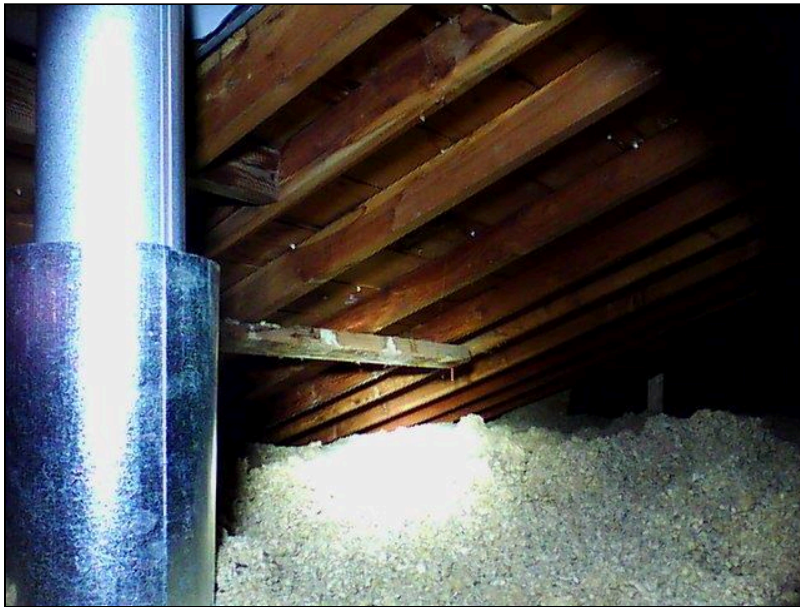
2.0 Item 8(Picture) Attic
