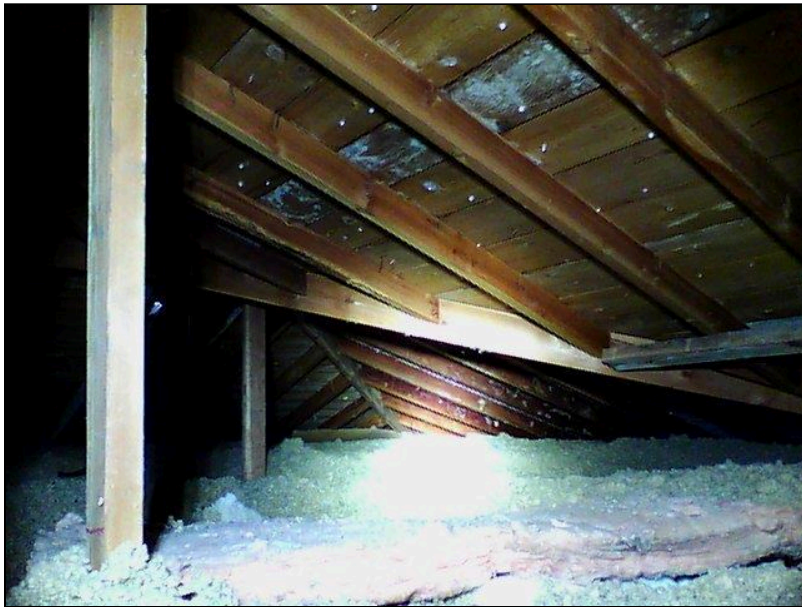
2.0 Item 2(Picture) Attic
