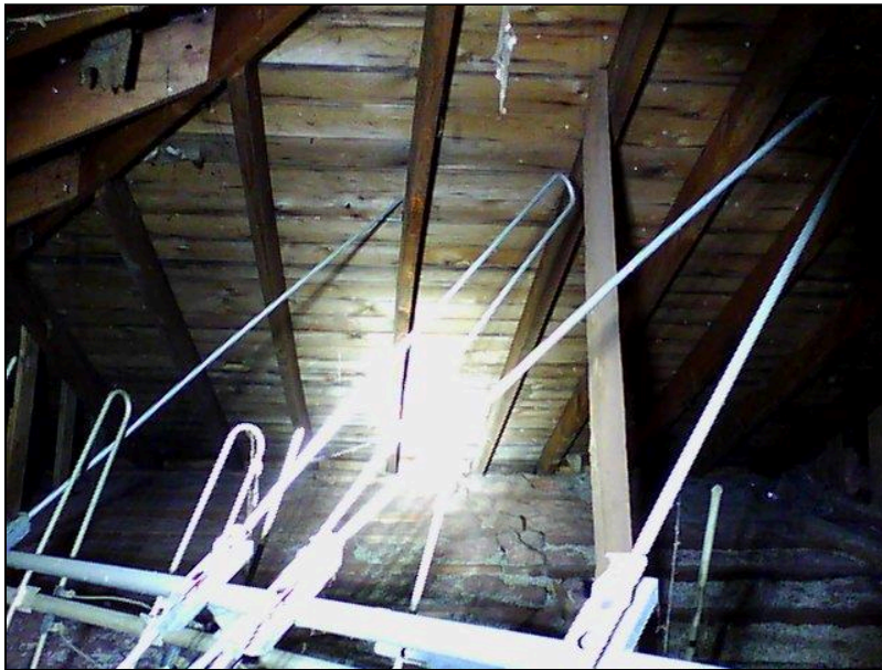
2.0 Item 16(Picture) Attic
