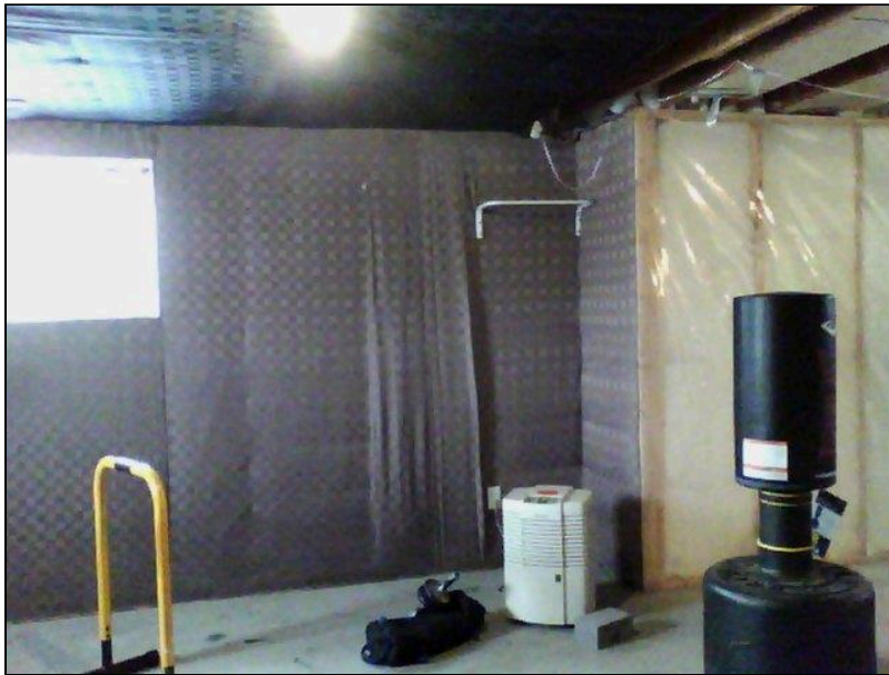
7.0 Item 12(Picture) Basement Foundation
