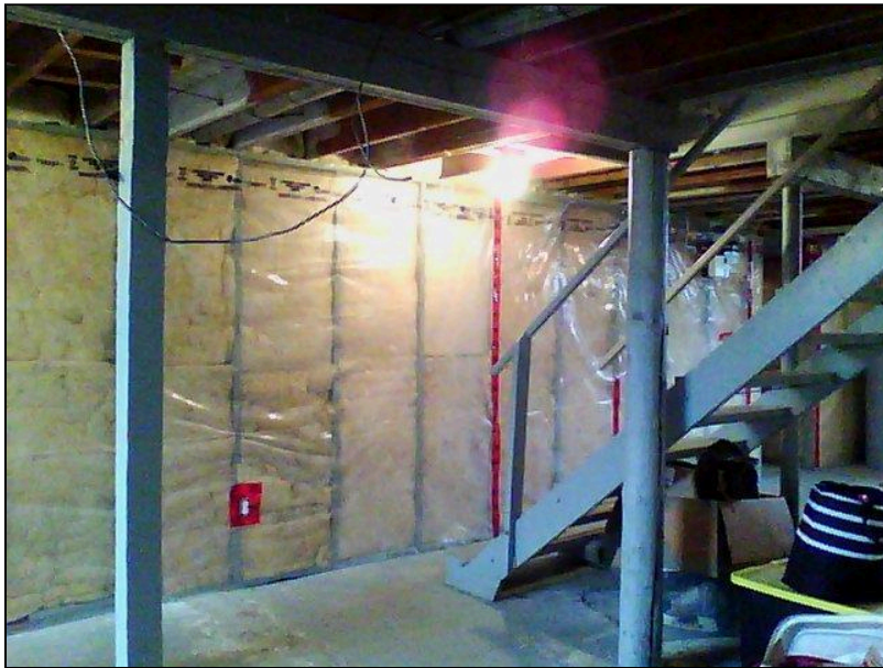
7.0 Item 10(Picture) Basement Foundation
