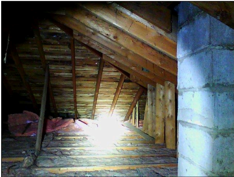
2.0 Item 2(Picture) Attic
