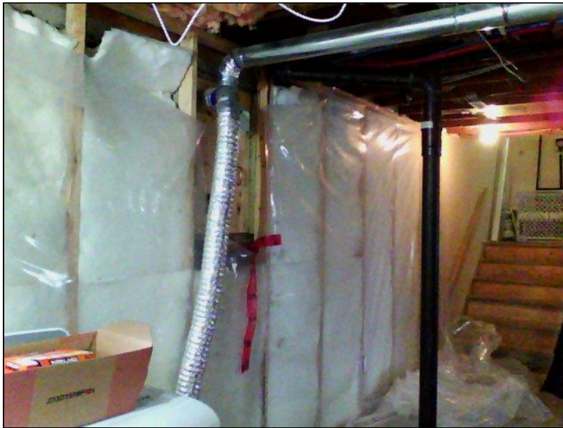
7.0 Item 8(Picture) Basement Foundation
