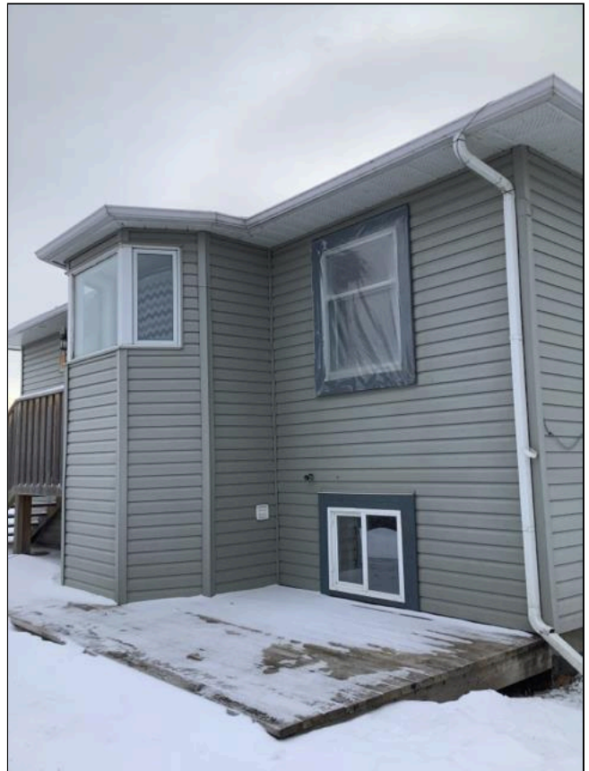
3.1 Item 4(Picture) Exterior
