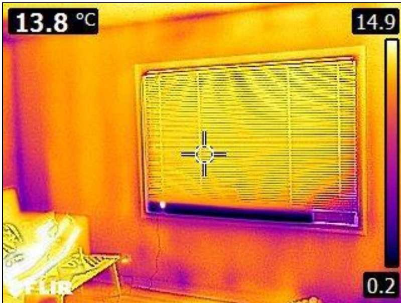
5.1 Item 26(Picture) Interior Walls
