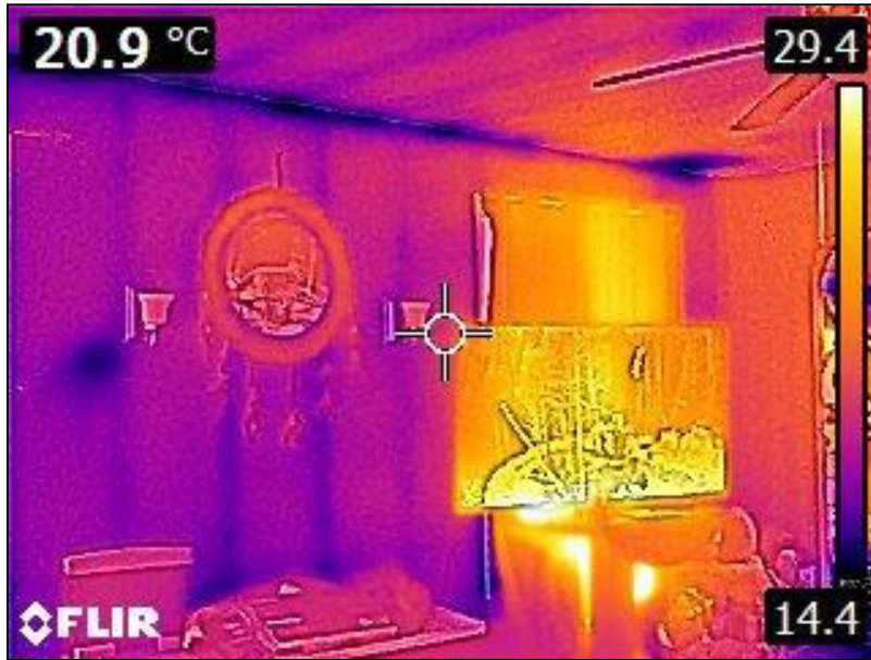
5.1 Item 29(Picture) Interior Walls
