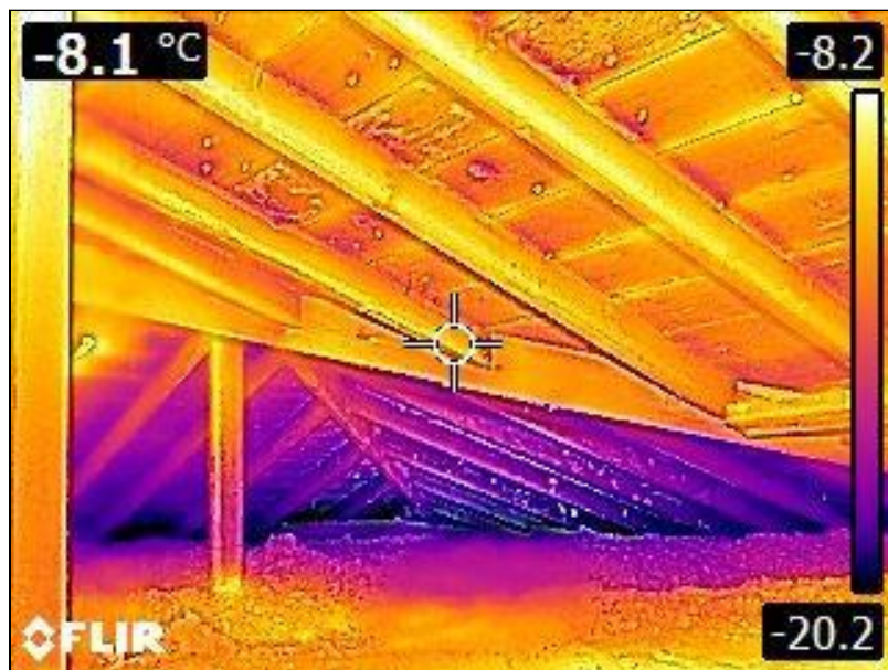
2.0 Item 1(Picture) Attic
