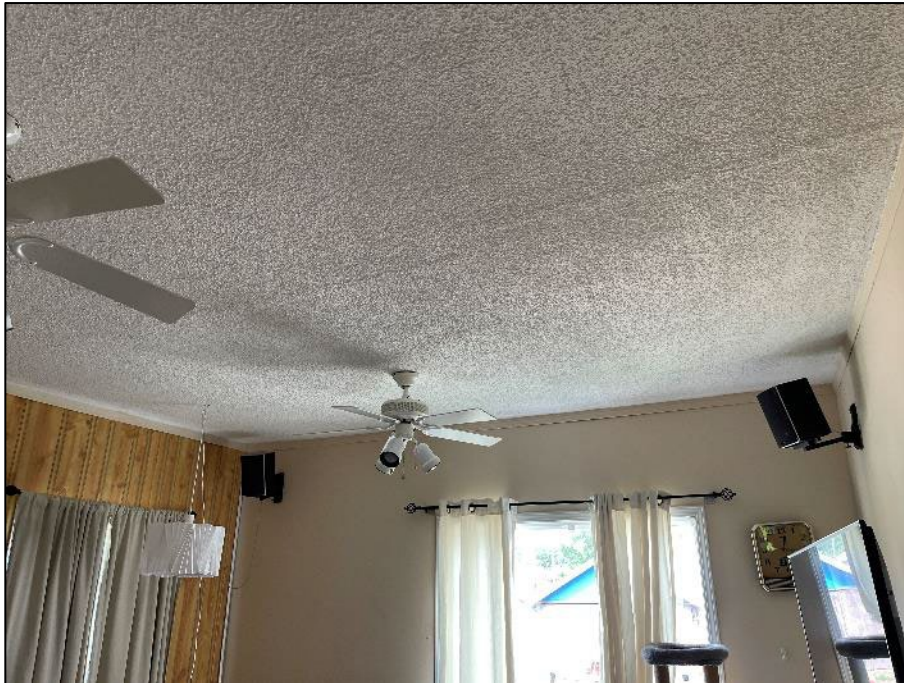
PHOTOGRAPH #7: Ceiling Texture - Level 1 Living Room (Non-Asbestos)
