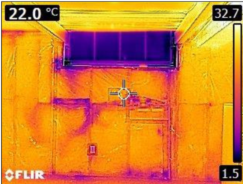
7.0 Item 15(Picture) Basement Foundation
