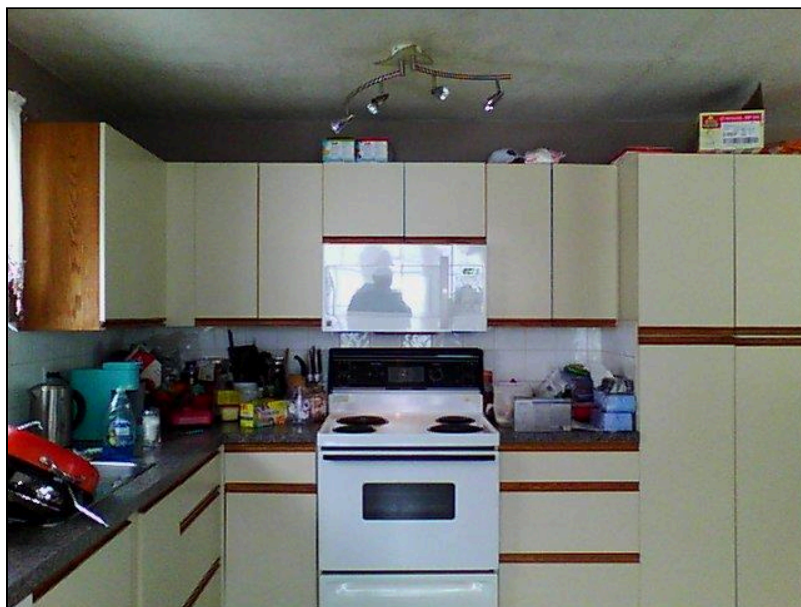
5.1 Item 46(Picture) Interior Walls
