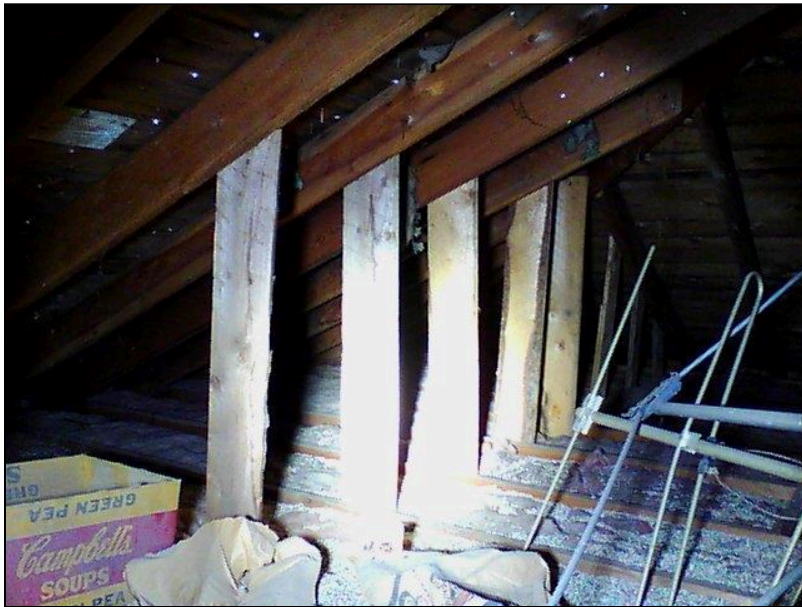
2.0 Item 14(Picture) Attic
