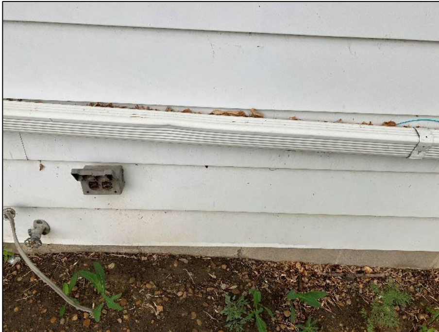
PHOTOGRAPH #17: Parging 1 – Exterior (Non-Asbestos)
