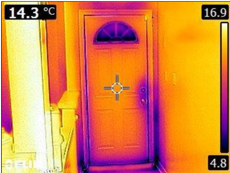
5.1 Item 22(Picture) Interior Walls
