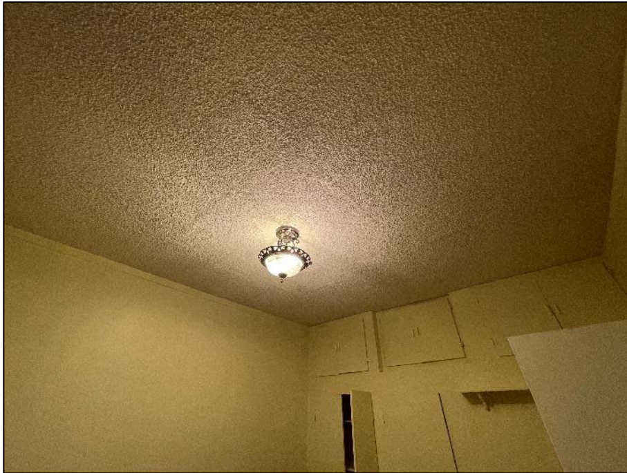
PHOTOGRAPH #9: Ceiling Texture - Level 1 SW Bedroom (Non-Asbestos)
