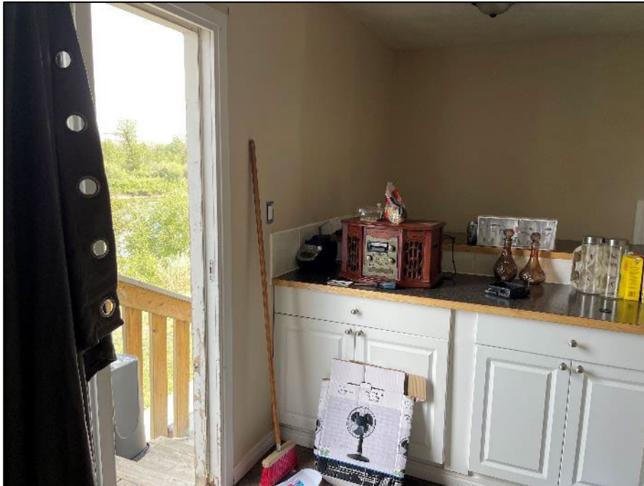
PHOTOGRAPH #1: Plaster - Level 1 Kitchen Exterior (<1% Actinolite)
