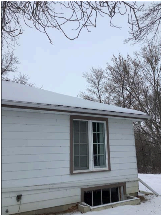
1.0 Item 7(Picture) Roof
