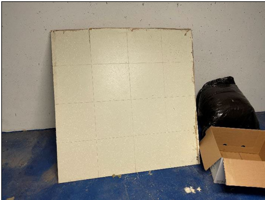
PHOTOGRAPH #10: Ceiling Tile - Basement (Non-Asbestos)
