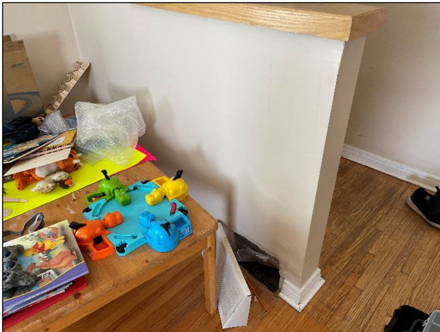
PHOTOGRAPH #4: Plaster - Level 1 Living Room Interior (<1% Actinolite)
