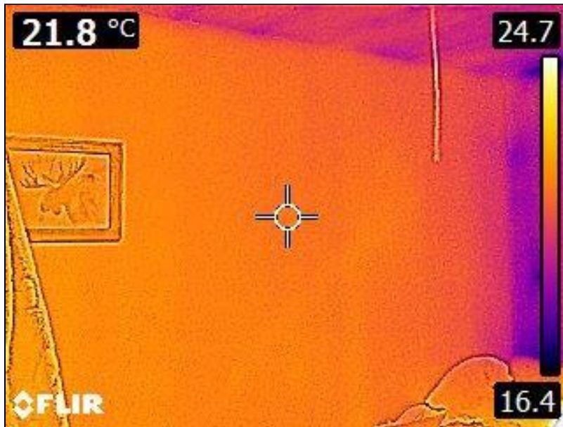
5.1 Item 13(Picture) Interior Walls
