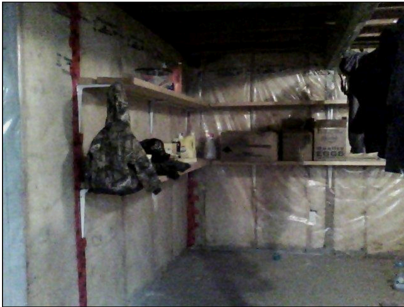
7.0 Item 26(Picture) Basement Foundation
