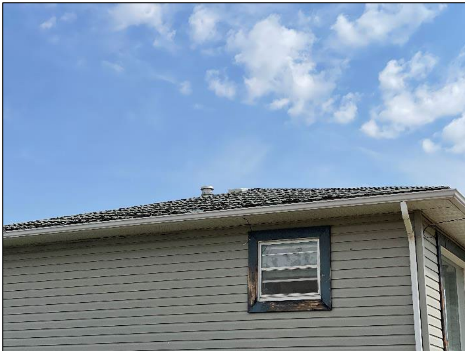
PHOTOGRAPH #10: Roofing (Non-Asbestos)
