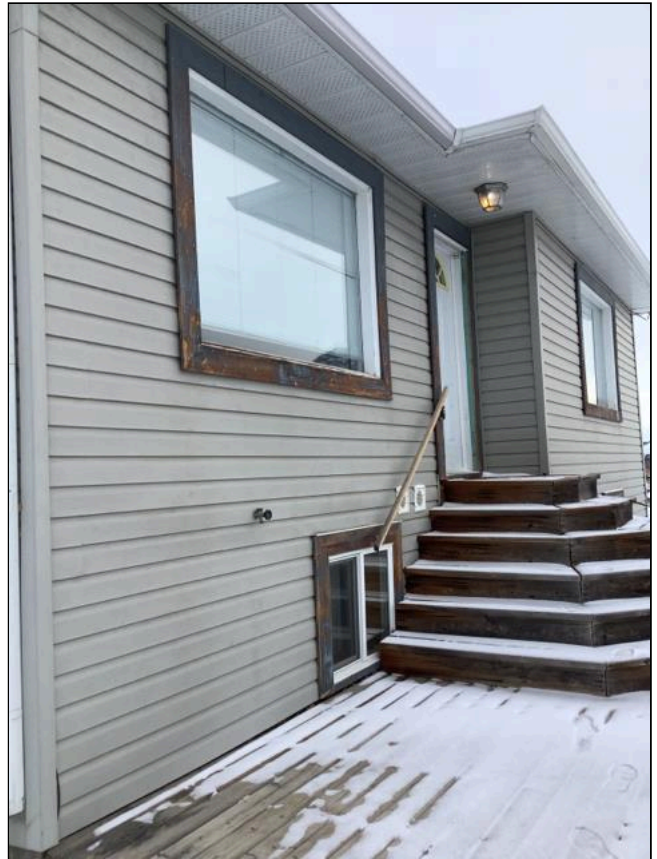
3.1 Item 2(Picture) Exterior
