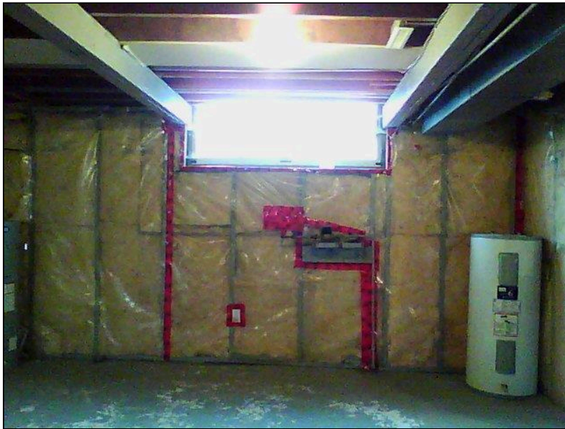
7.0 Item 16(Picture) Basement Foundation
