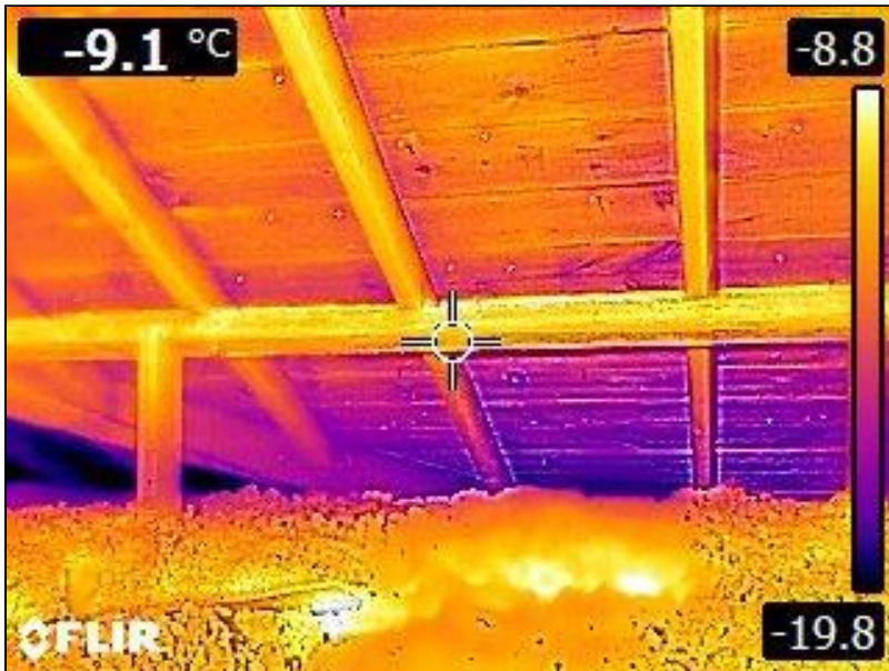
2.0 Item 13(Picture) Attic
