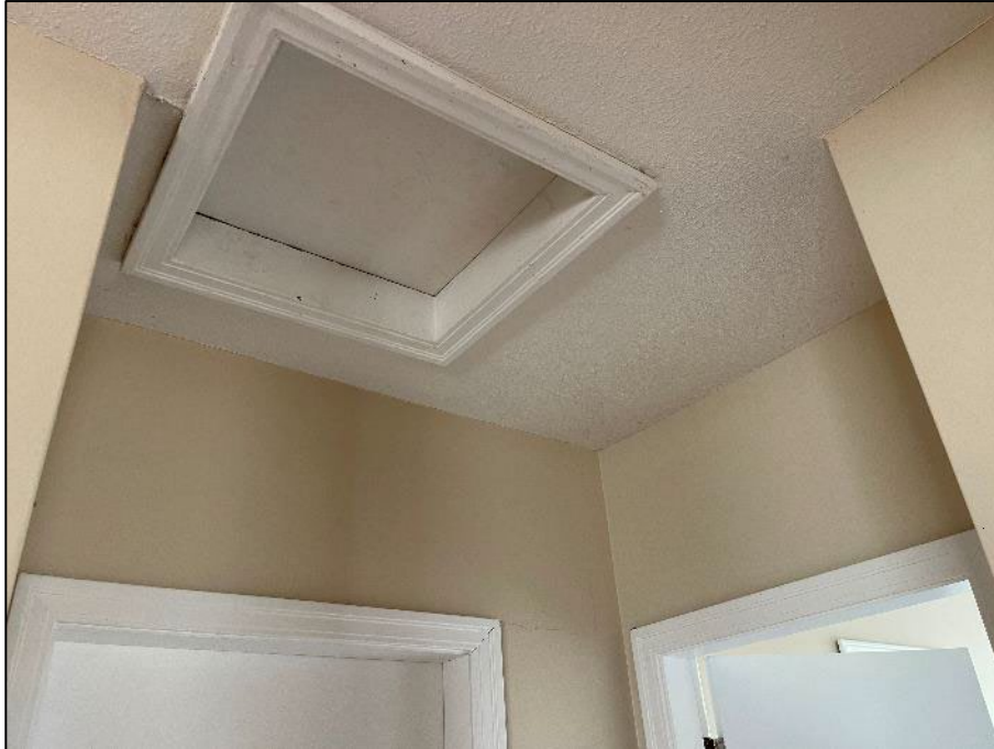
PHOTOGRAPH #17: Ceiling Texture - Level 1 Hallway (Non-Asbestos)
