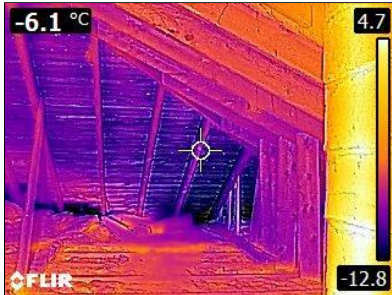
2.0 Item 1(Picture) Attic
