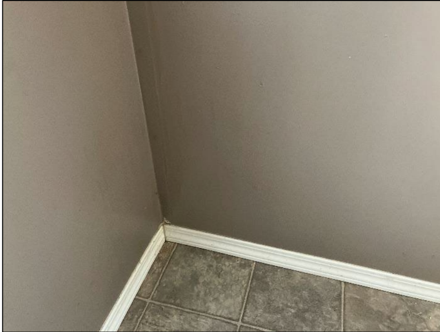
PHOTOGRAPH #1: Drywall Joint Compound - Floor 1 Ext Dining Room (2% Chrysotile)
