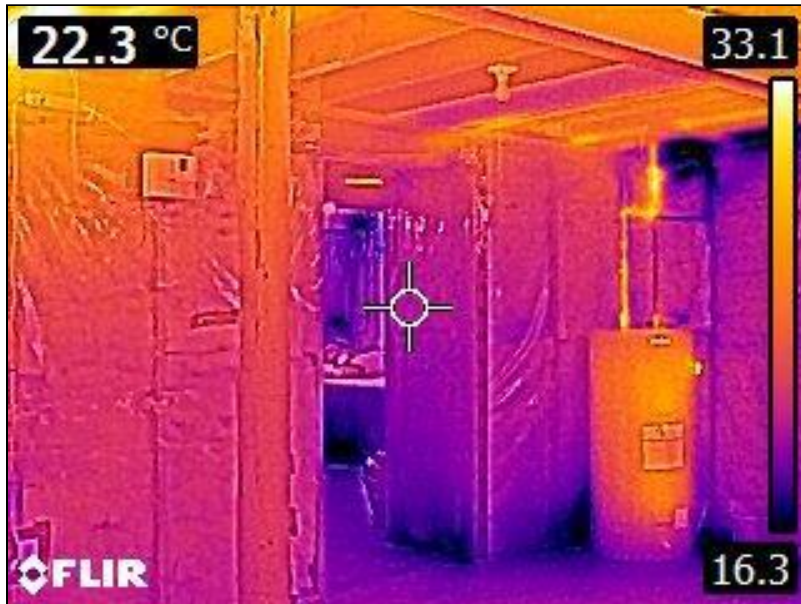
7.0 Item 13(Picture) Basement Foundation
