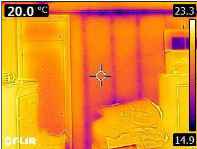
5.1 Item 11(Picture) Interior Walls
