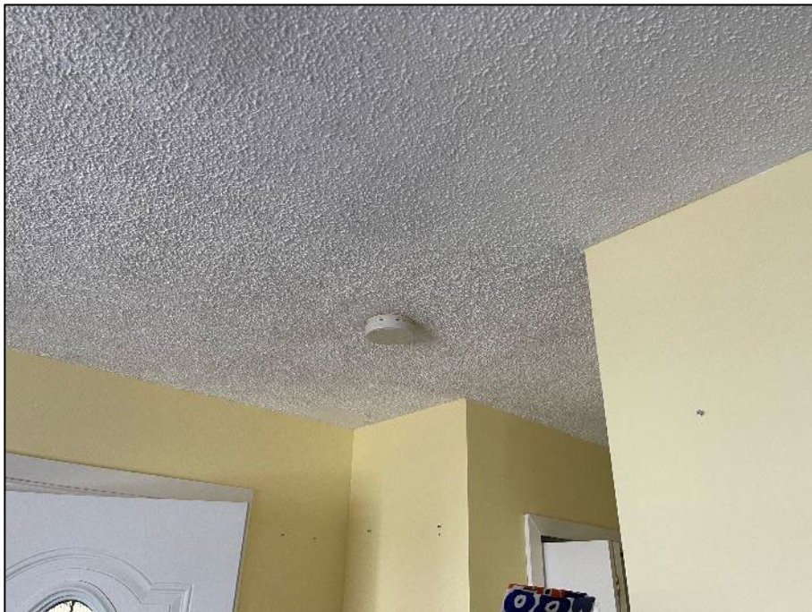
PHOTOGRAPH #20: Smoke Detectors Present (Radioactive Materials)
