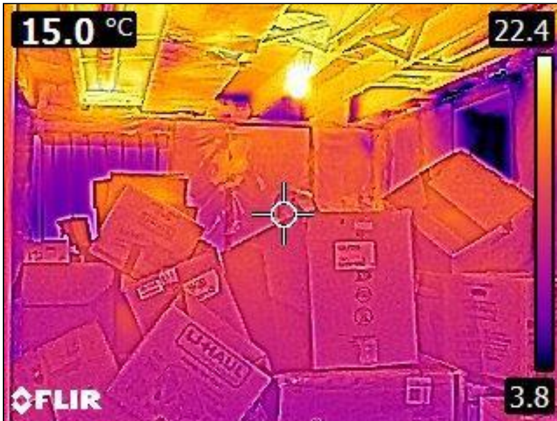
7.0 Item 5(Picture) Basement Foundation
