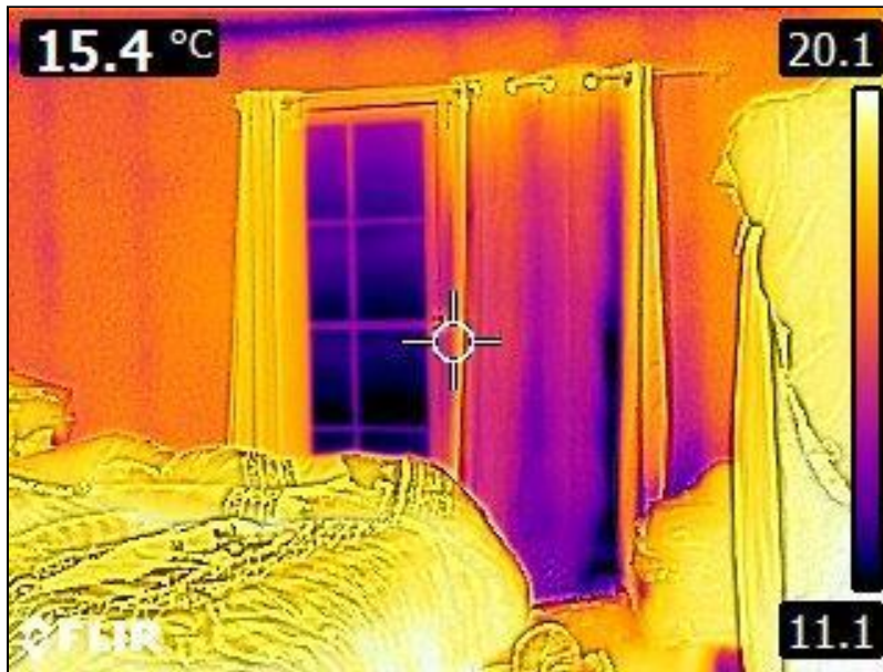
5.1 Item 3(Picture) Interior Walls
