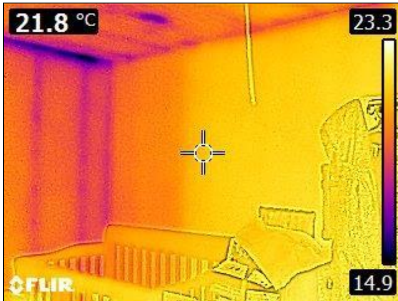
5.1 Item 17(Picture) Interior Walls
