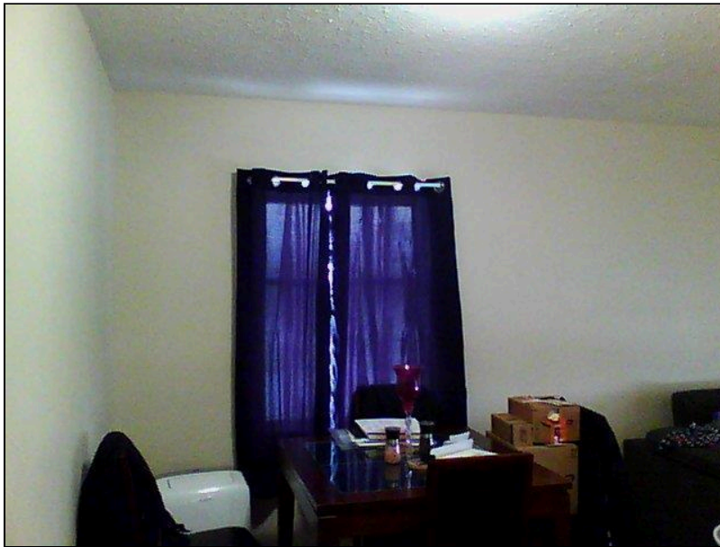
5.1 Item 31(Picture) Interior Walls
