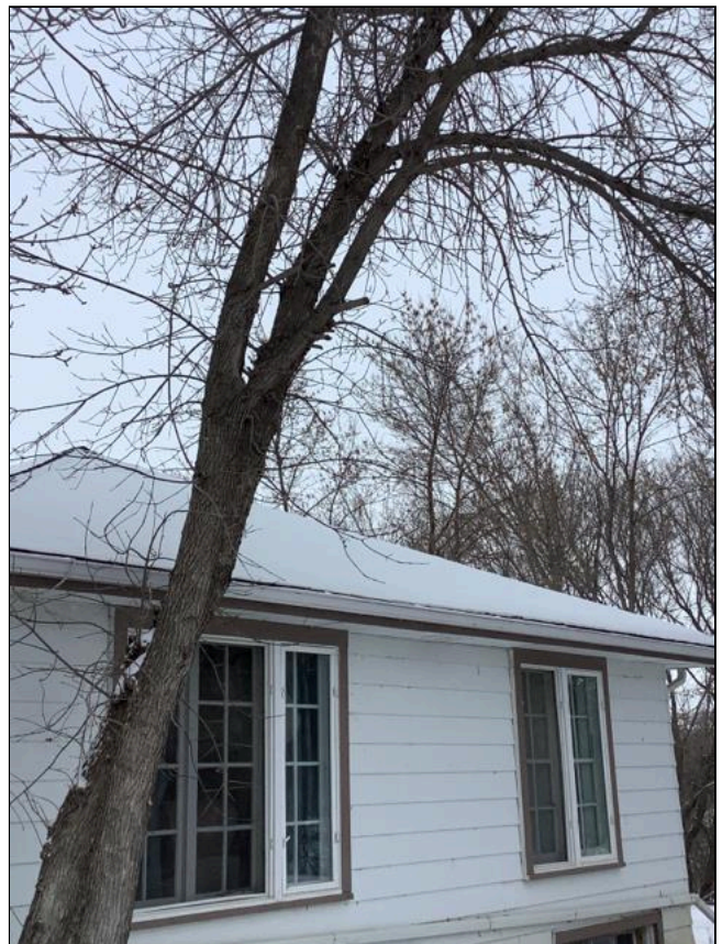
1.0 Item 6(Picture) Roof
