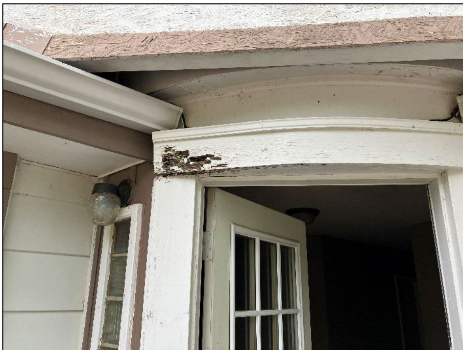
PHOTOGRAPH #26: Paint- White Exterior (Non-Lead Based)
