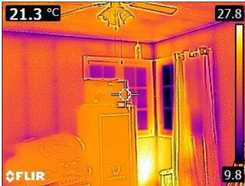
5.1 Item 9(Picture) Interior Walls
