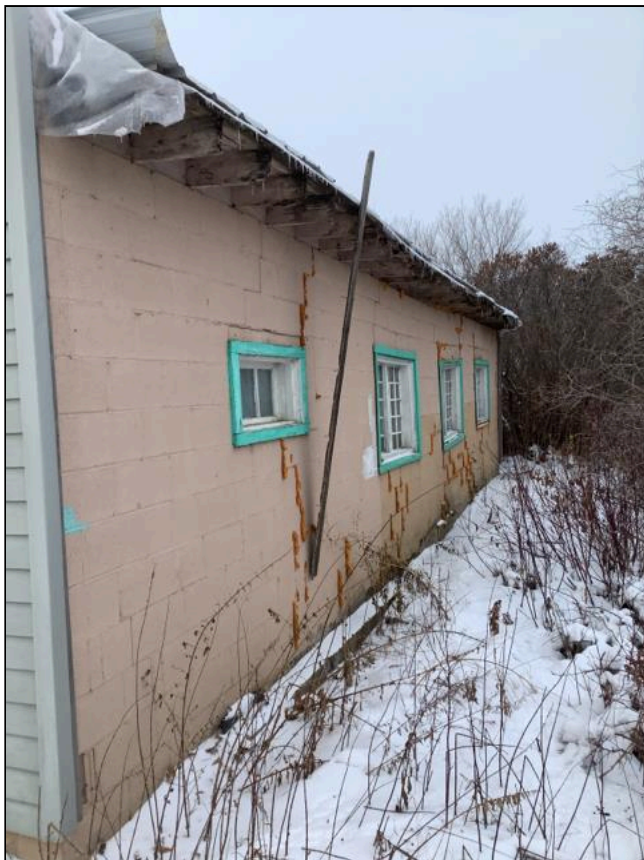
4.4 Item 3(Picture) Garage Exterior
