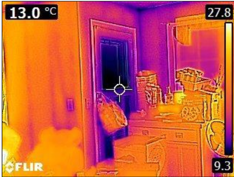
5.1 Item 37(Picture) Interior Walls
