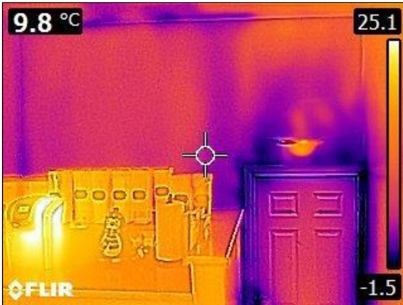
5.1 Item 36(Picture) Interior Walls
