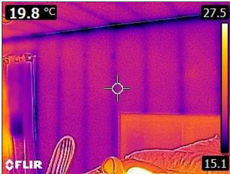
5.1 Item 7(Picture) Interior Walls
