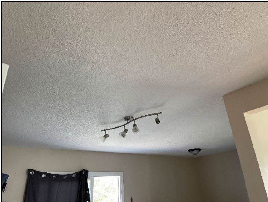
PHOTOGRAPH #18: Ceiling Texture - Level 1 Kitchen (Non-Asbestos)
