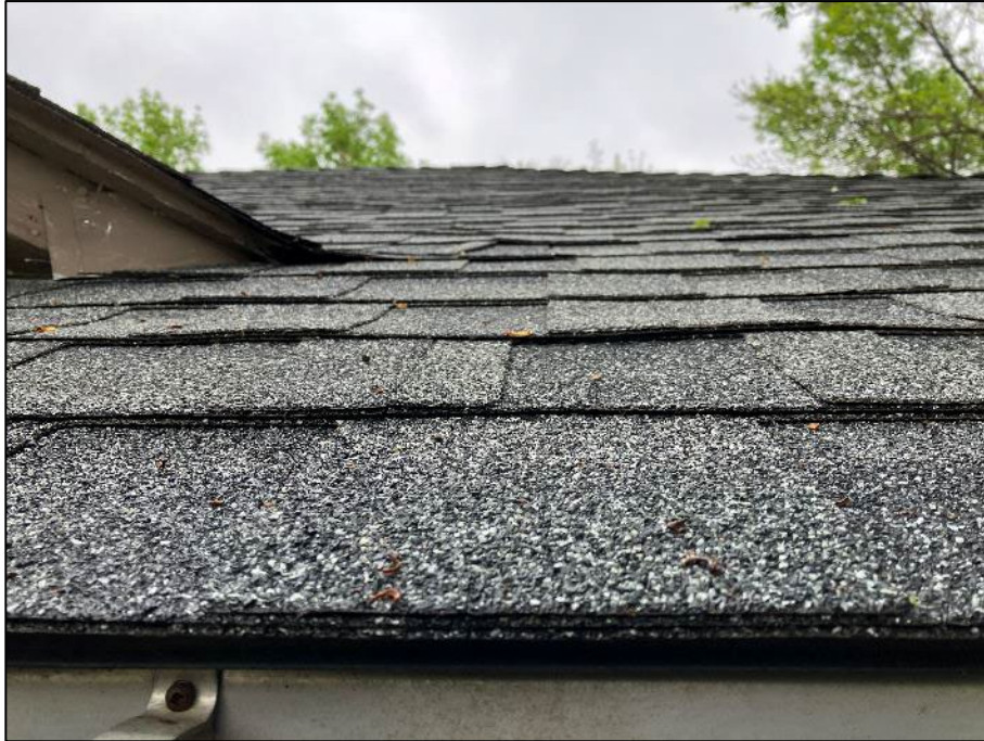
PHOTOGRAPH #19: Roof Shingle – Exterior (Non-Asbestos)
