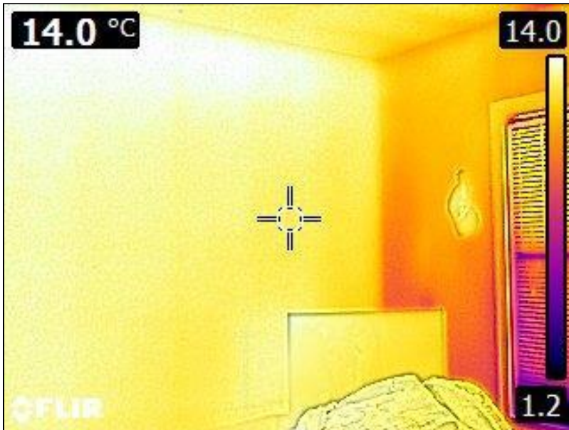
5.1 Item 20(Picture) Interior Walls
