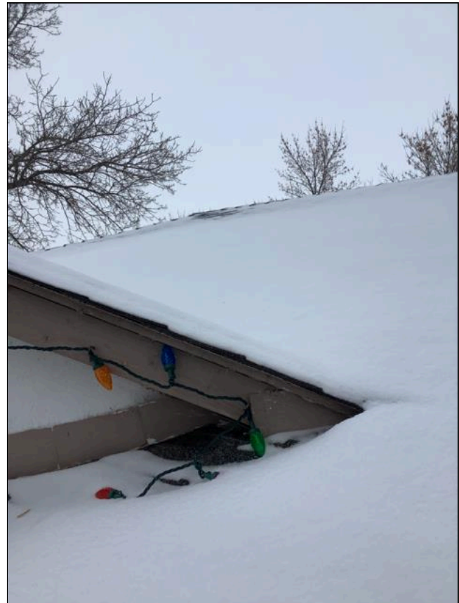
1.0 Item 2(Picture) Roof
