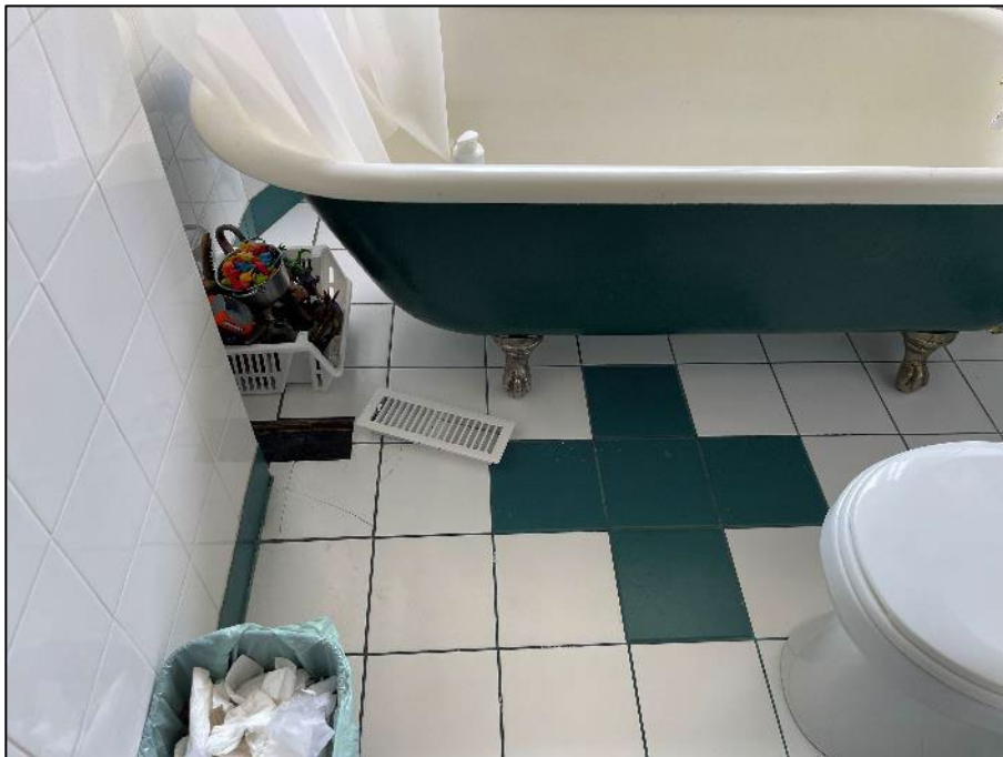
PHOTOGRAPH #8: Thinset – Bathroom (Non-Asbestos)
