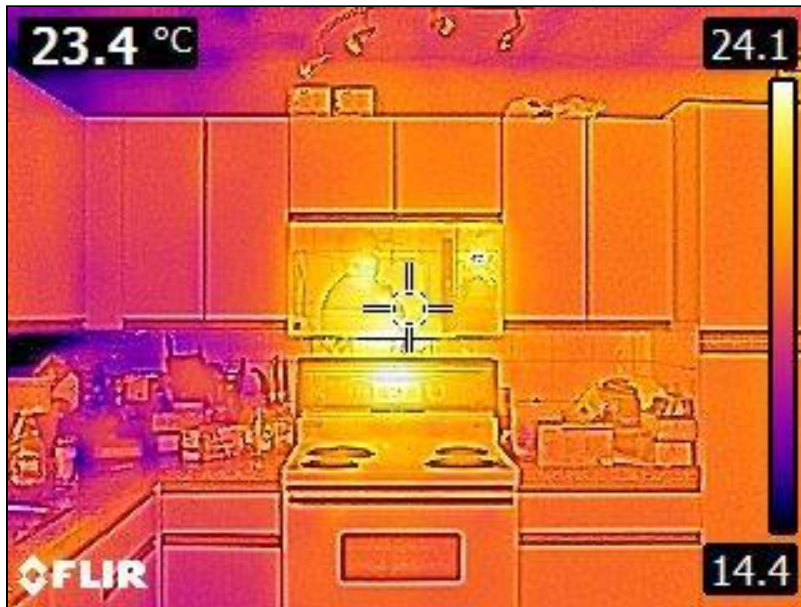
5.1 Item 45(Picture) Interior Walls
