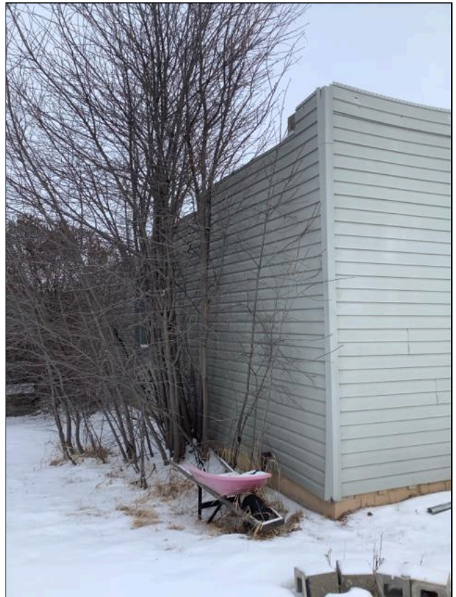
4.4 Item 4(Picture) Garage Exterior
