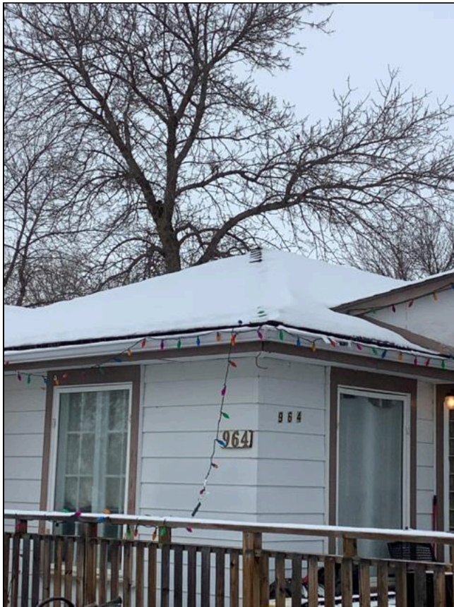
1.0 Item 3(Picture) Roof
