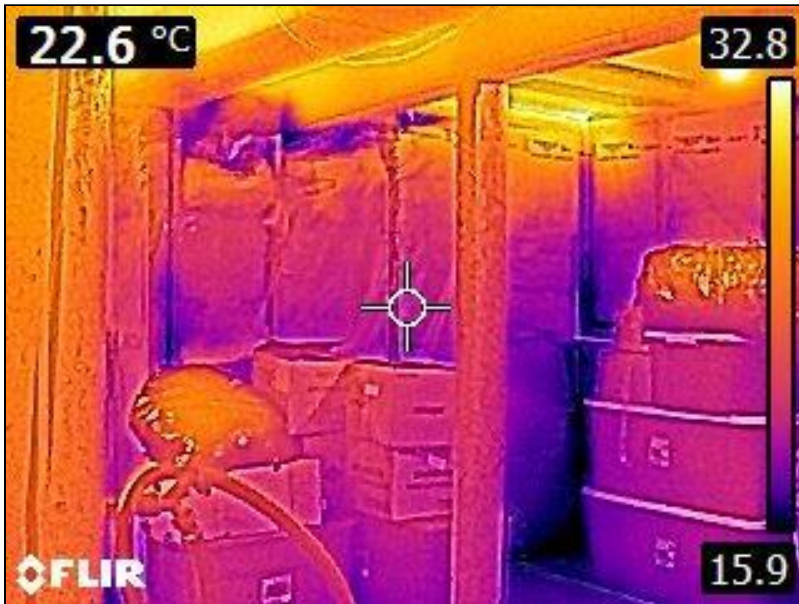
7.0 Item 17(Picture) Basement Foundation
