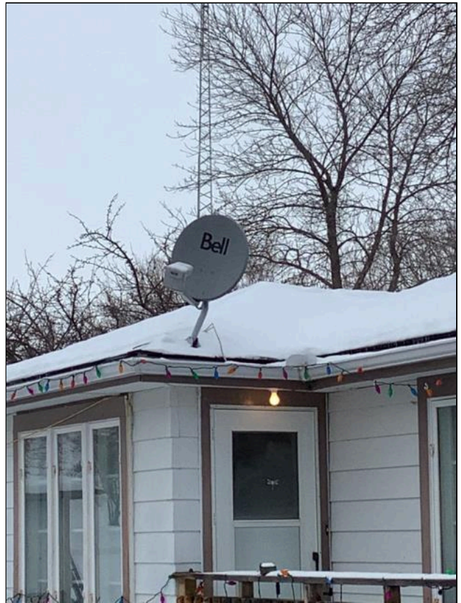
1.0 Item 4(Picture) Roof
