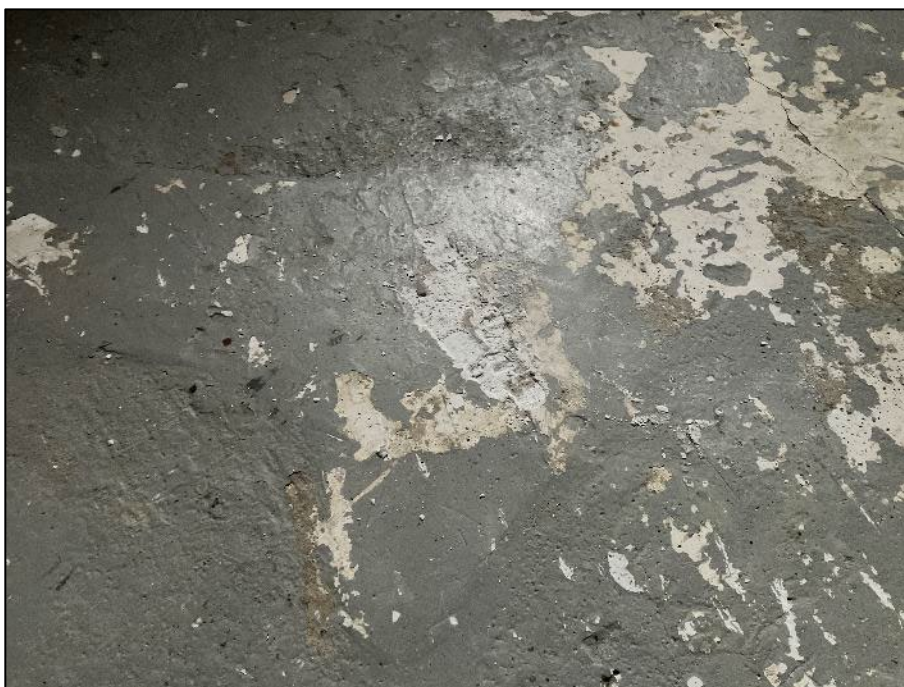
PHOTOGRAPH #24: Paint – Grey Basement (Non-Lead Based)
