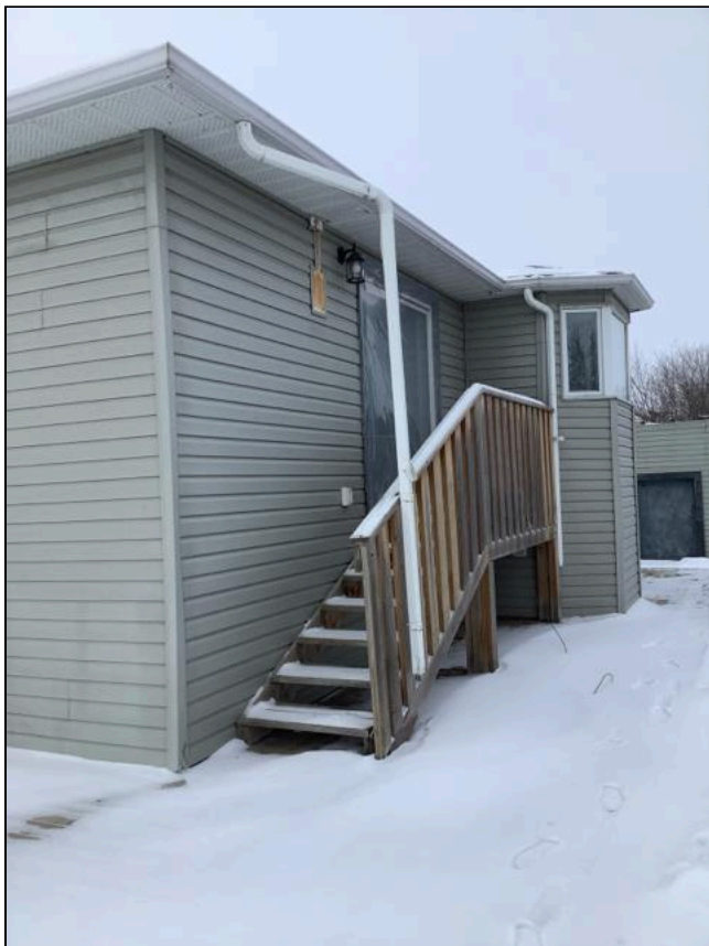
3.1 Item 5(Picture) Exterior
