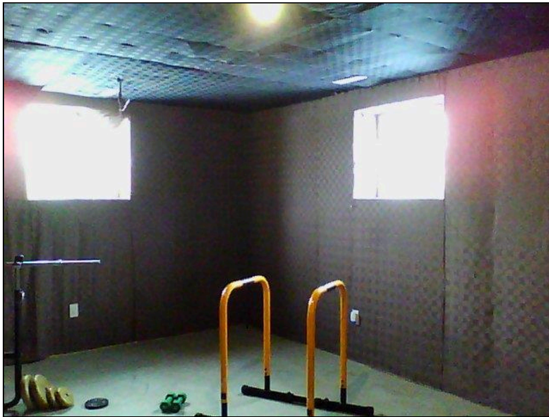
7.0 Item 14(Picture) Basement Foundation
