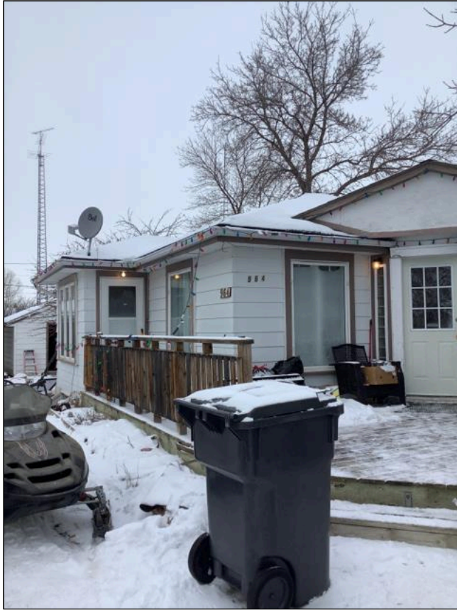
3.1 Item 9(Picture) Exterior
