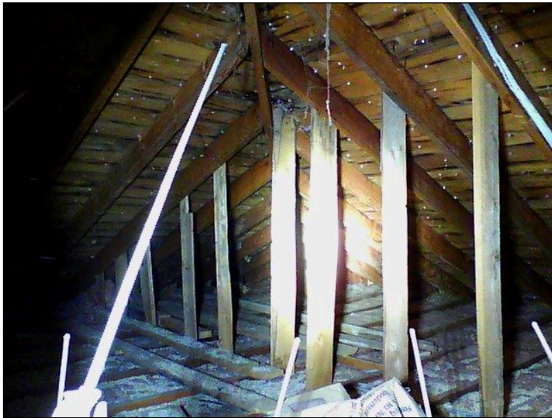
2.0 Item 10(Picture) Attic
