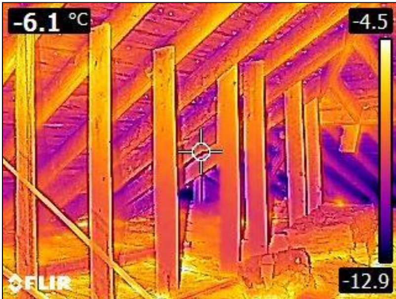
2.0 Item 5(Picture) Attic
