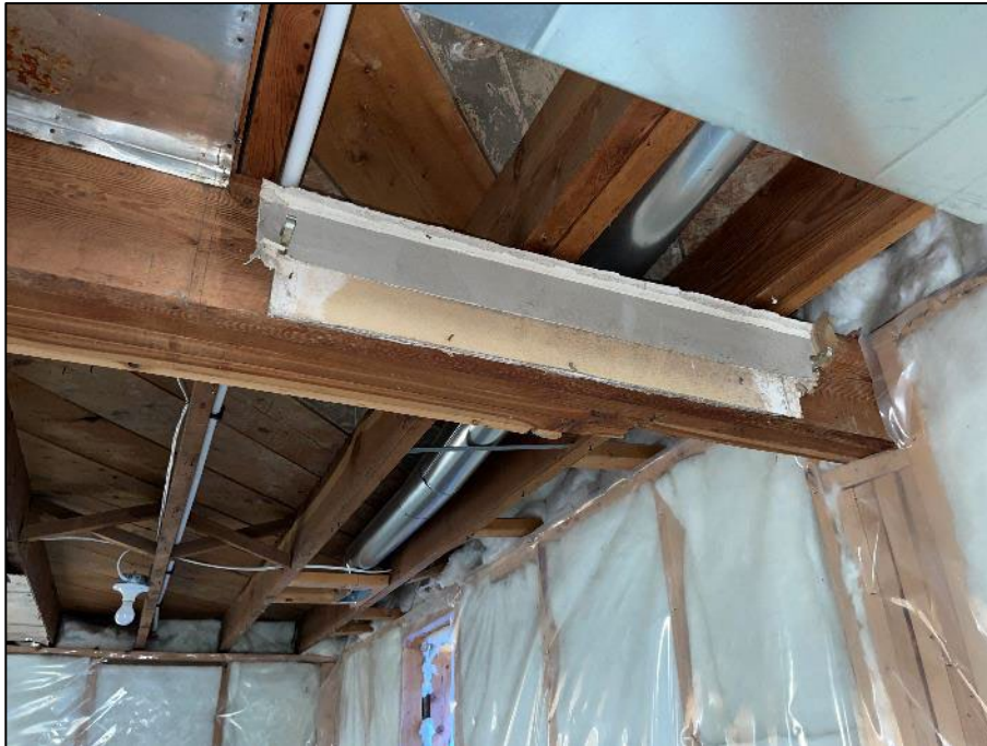
PHOTOGRAPH #15: Drywall Joint Compound - Basement Laundry Room (Non-Asbestos)
