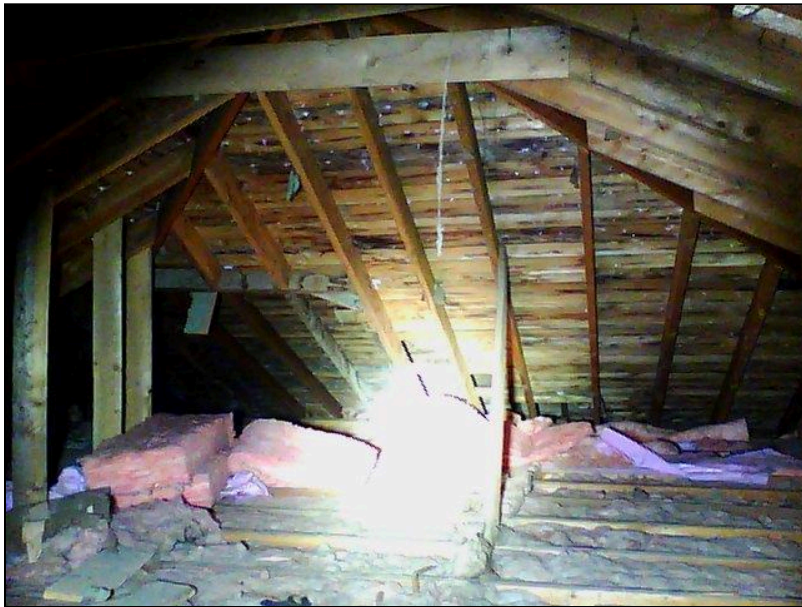
2.0 Item 4(Picture) Attic
