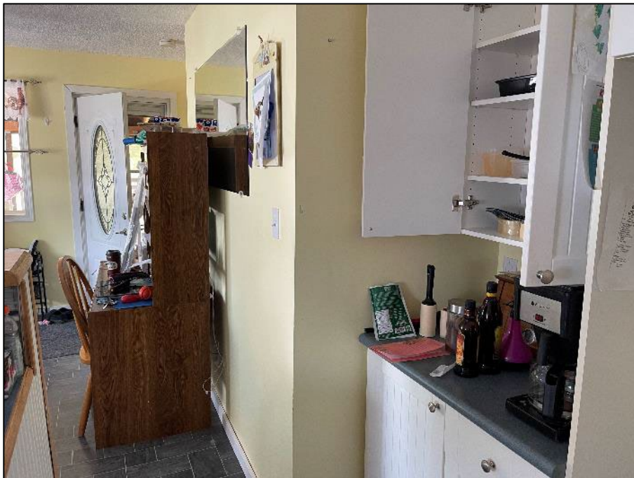
PHOTOGRAPH #6: Drywall Joint Compound - Level 1 Kitchen (Non-Asbestos)
