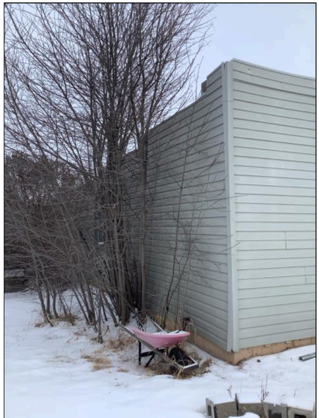
4.4 Item 4(Picture) Garage Exterior
