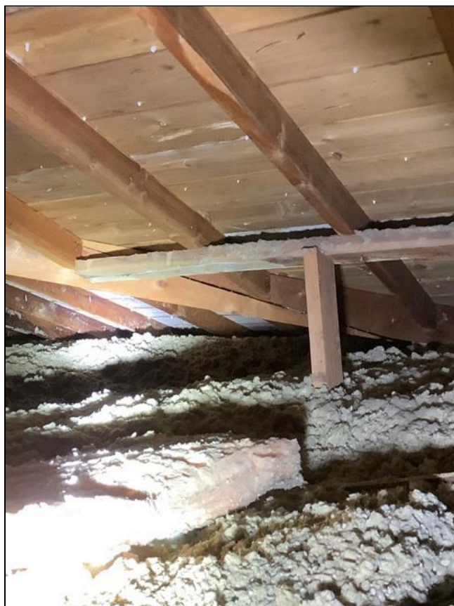
2.3 Item 1(Picture) Rafter - split, cross support bowed
