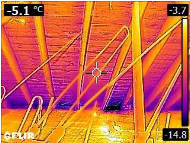
2.0 Item 15(Picture) Attic
