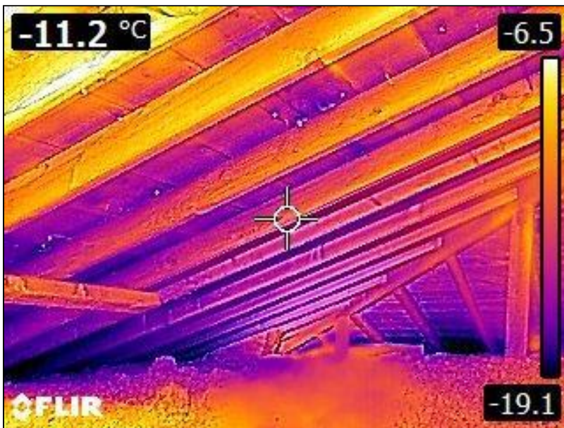
2.0 Item 5(Picture) Attic
