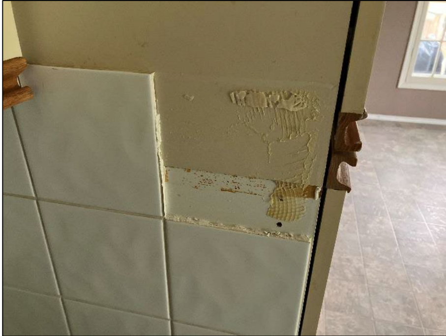
PHOTOGRAPH #13: Thinset – Kitchen (Non-Asbestos)
