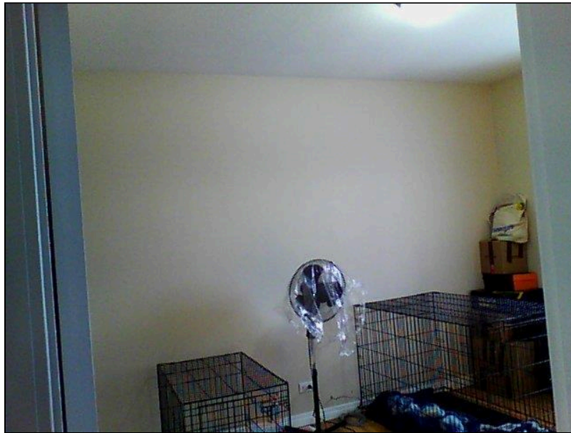
5.1 Item 11(Picture) Interior Walls
