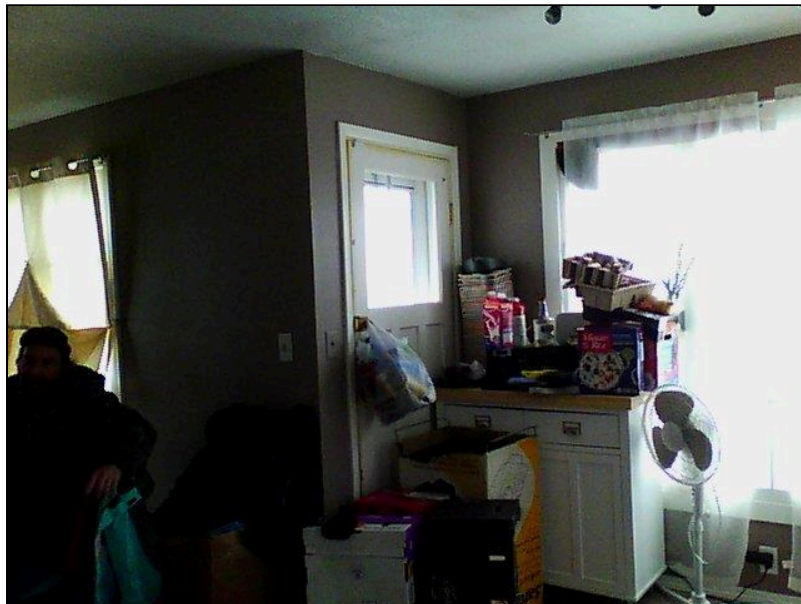
5.1 Item 38(Picture) Interior Walls
