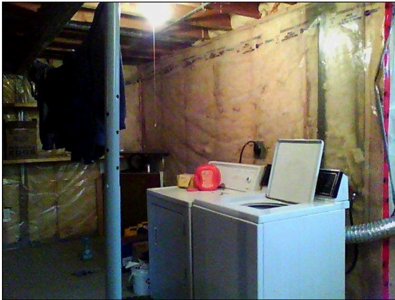
7.0 Item 24(Picture) Basement Foundation
