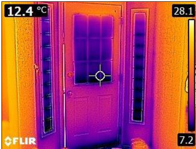
5.1 Item 31(Picture) Interior Walls
