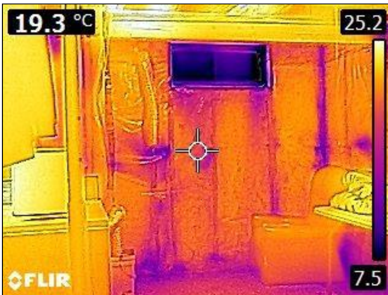
7.0 Item 21(Picture) Basement Foundation
