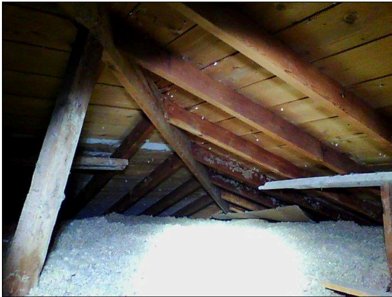
2.0 Item 12(Picture) Attic
