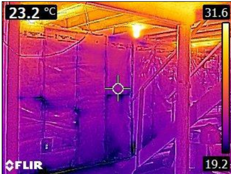
7.0 Item 9(Picture) Basement Foundation
