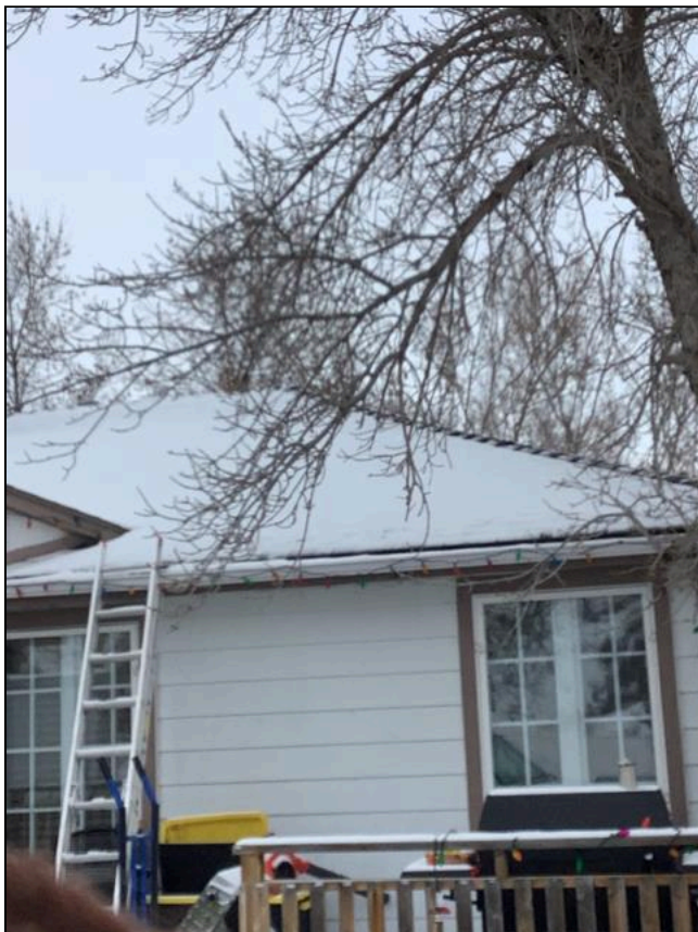
1.0 Item 5(Picture) Roof
