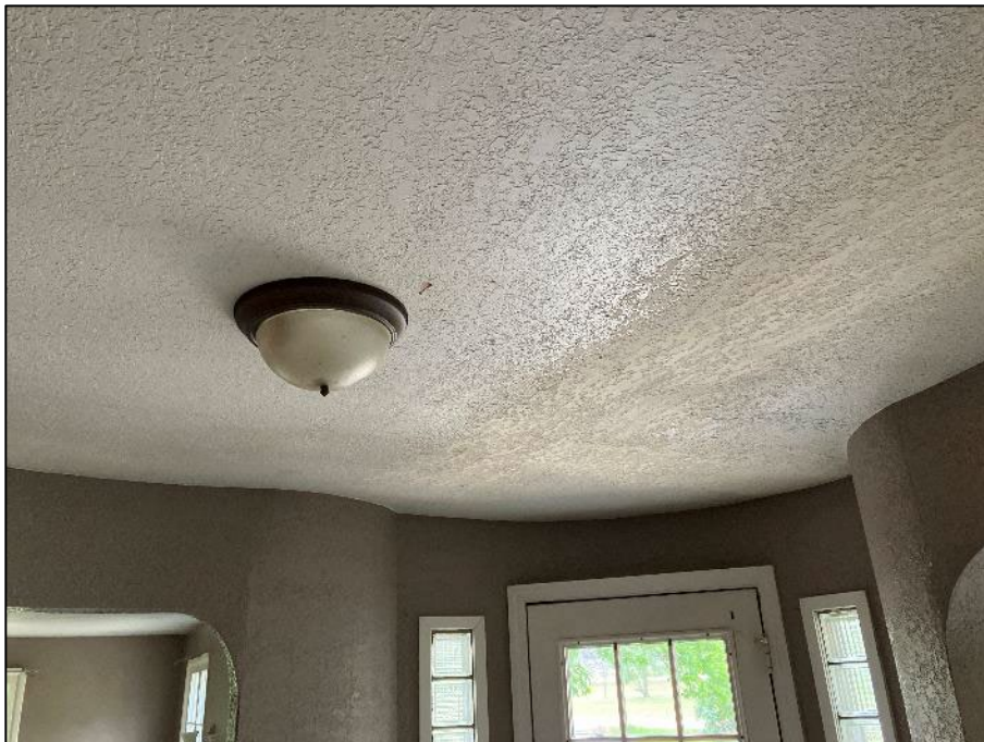
PHOTOGRAPH #10: Ceiling Texture - Floor 1 Foyer (Non-Asbestos)
