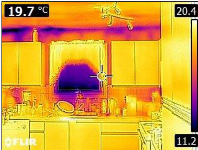
5.1 Item 33(Picture) Interior Walls
