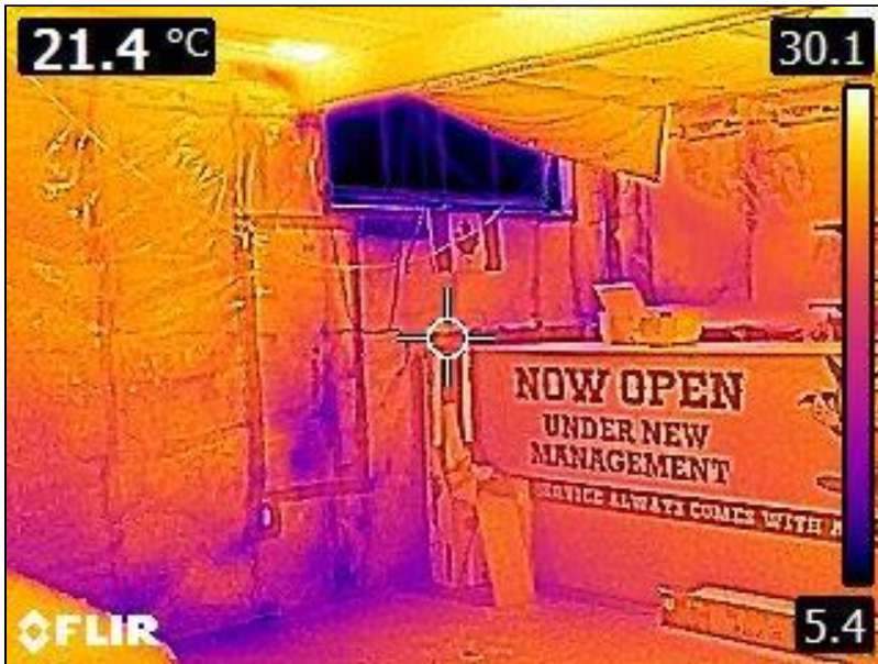
7.0 Item 5(Picture) Basement Foundation
