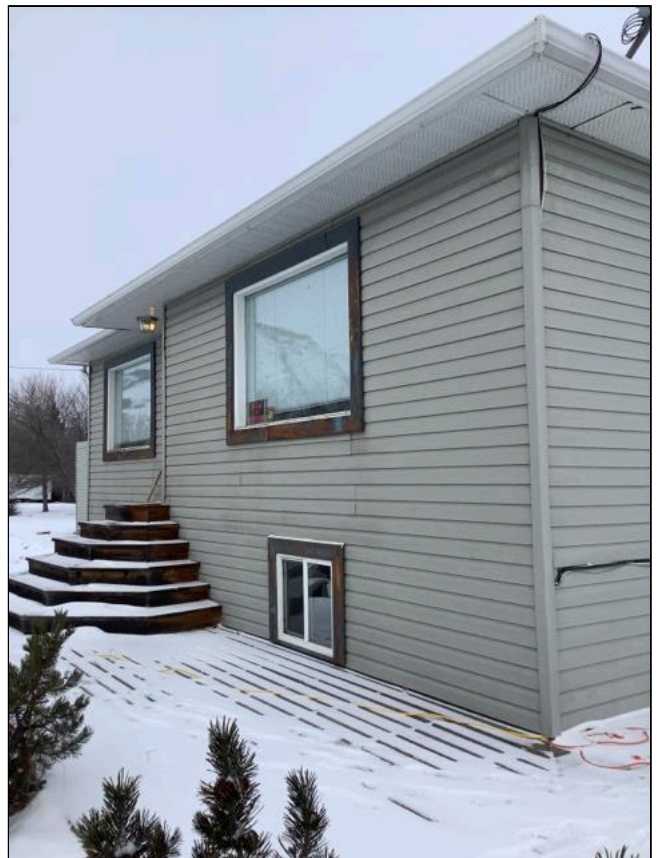
3.1 Item 8(Picture) Exterior
