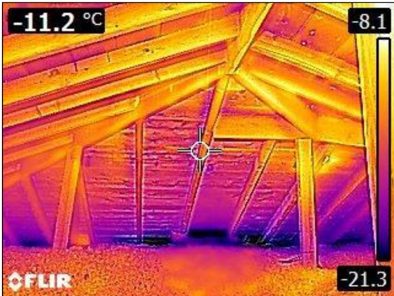
2.0 Item 3(Picture) Attic
