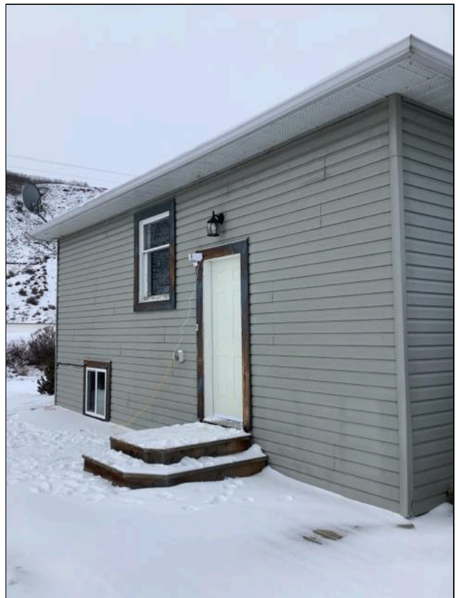
3.1 Item 6(Picture) Exterior
