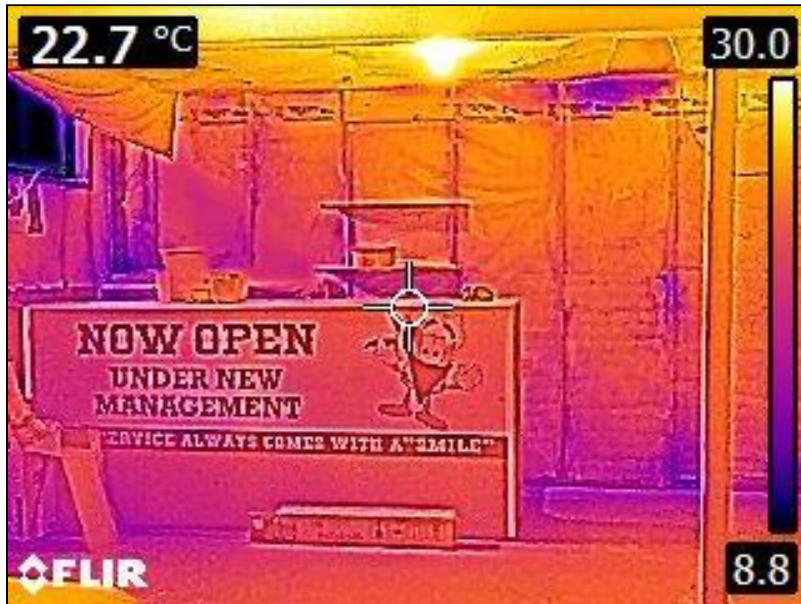
7.0 Item 7(Picture) Basement Foundation
