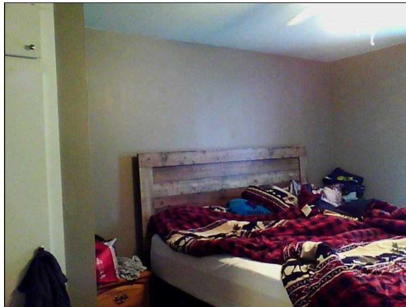
5.1 Item 2(Picture) Interior Walls
