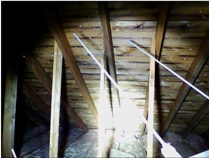
2.0 Item 8(Picture) Attic
