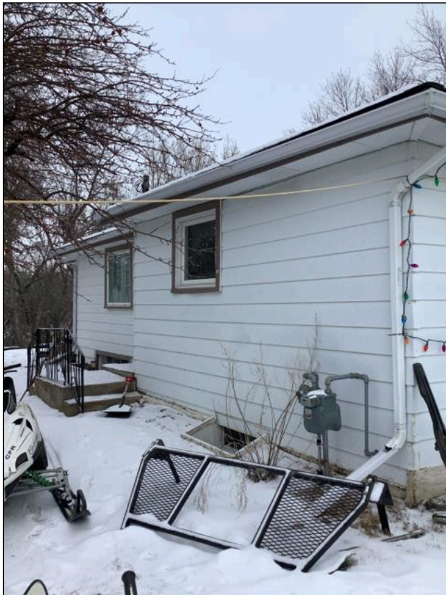
3.1 Item 3(Picture) Exterior
