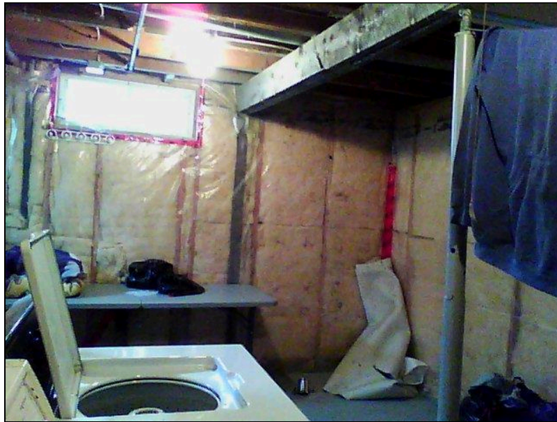
7.0 Item 28(Picture) Basement Foundation
