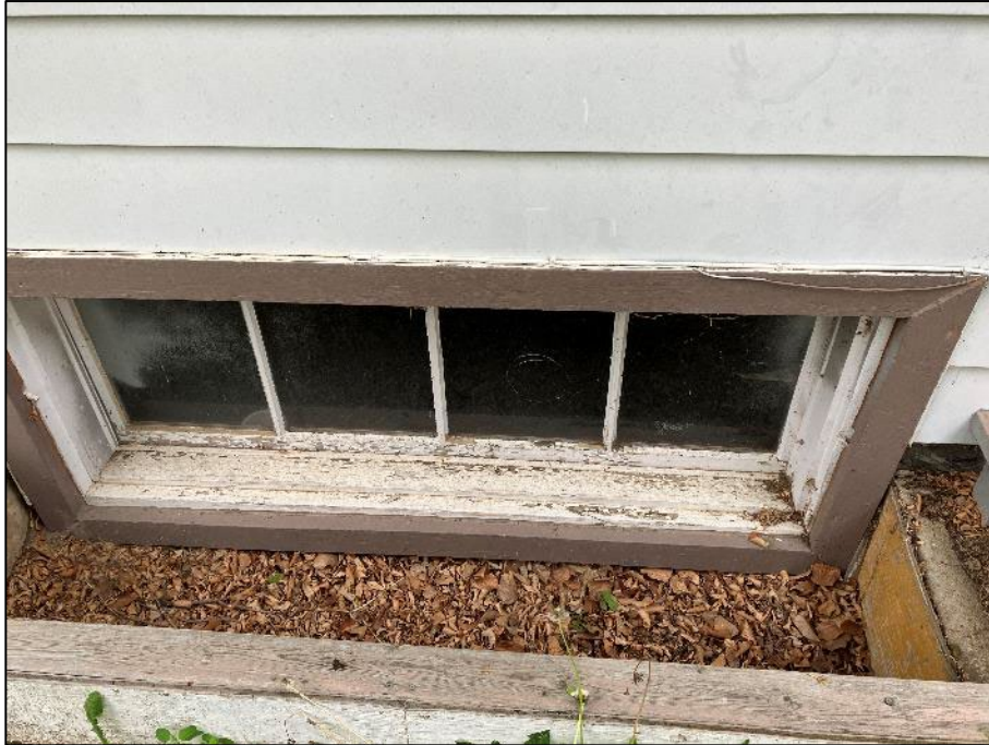
PHOTOGRAPH #15: Window Caulking – Exterior (Non-Asbestos)
