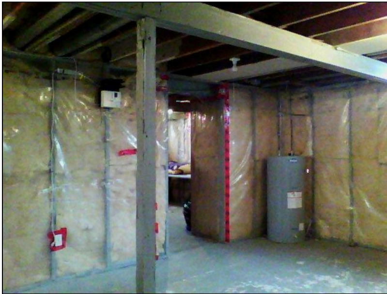
7.0 Item 14(Picture) Basement Foundation
