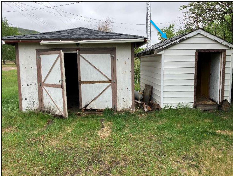
PHOTOGRAPH #20: Roof Shingle – Shed (Non-Asbestos)
