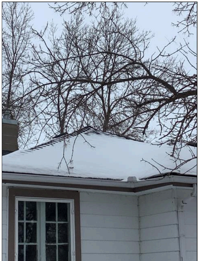
1.0 Item 10(Picture) Roof
