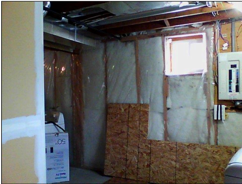
7.0 Item 4(Picture) Basement Foundation
