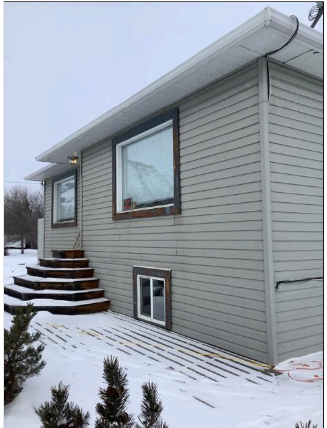
3.1 Item 8(Picture) Exterior
