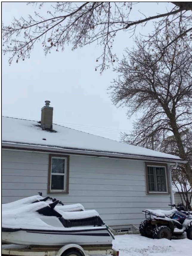
1.0 Item 9(Picture) Roof
