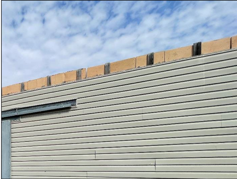
PHOTOGRAPH #27: Block Wall Used for Garage Construction – No Visible Vermiculite Identified
