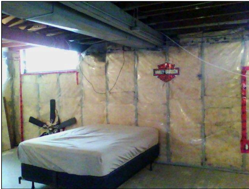
7.0 Item 4(Picture) Basement Foundation
