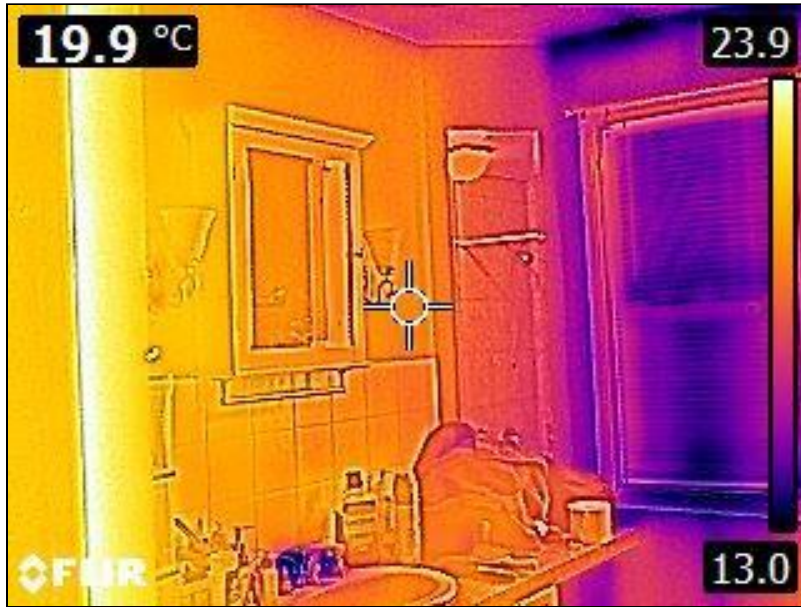
9.0 Item 2(Picture) Bathroom Walls
