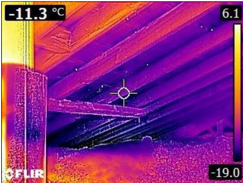
2.0 Item 7(Picture) Attic
