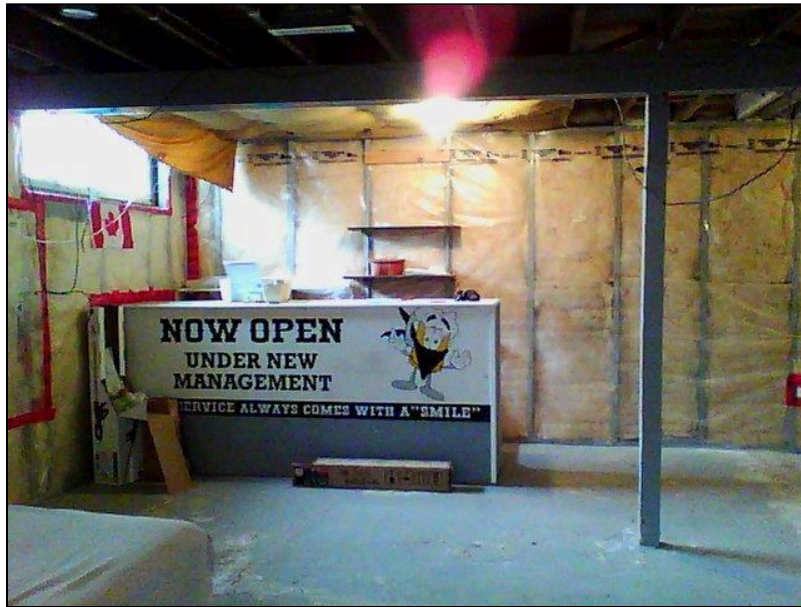
7.0 Item 8(Picture) Basement Foundation
