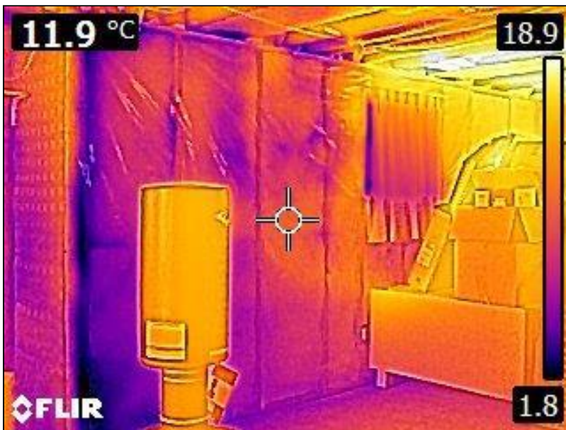
7.0 Item 9(Picture) Basement Foundation
