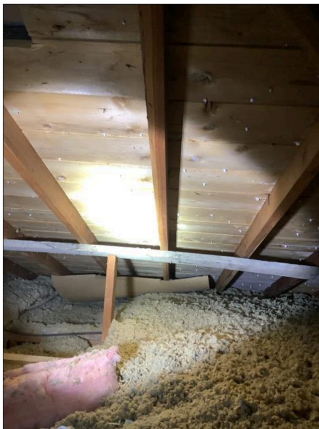
2.3 Item 2(Picture) Rafter - split, cross support bowed
