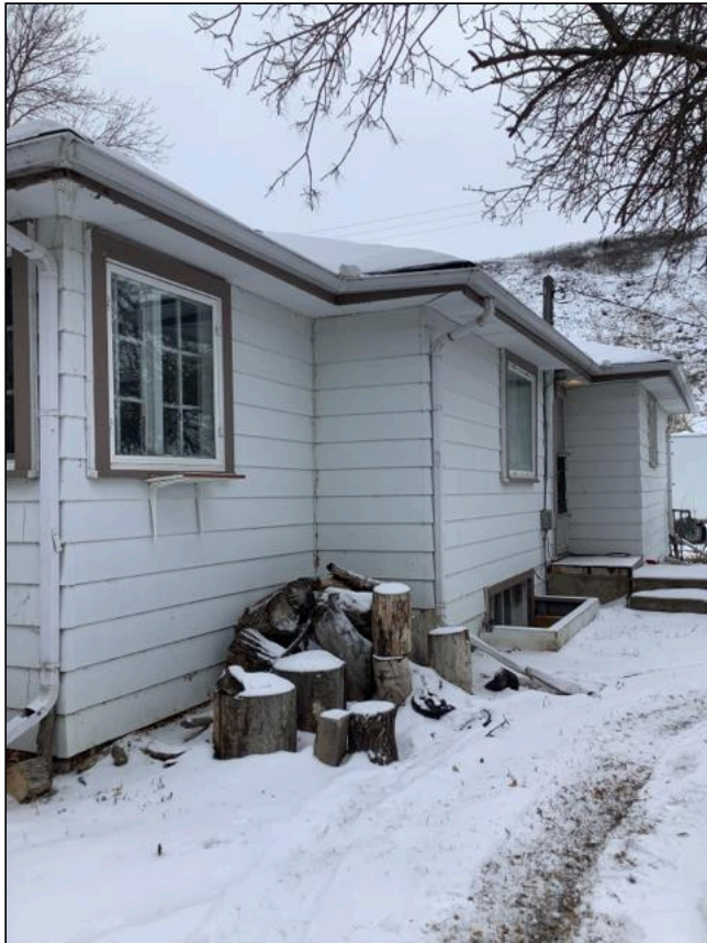
3.1 Item 5(Picture) Exterior
