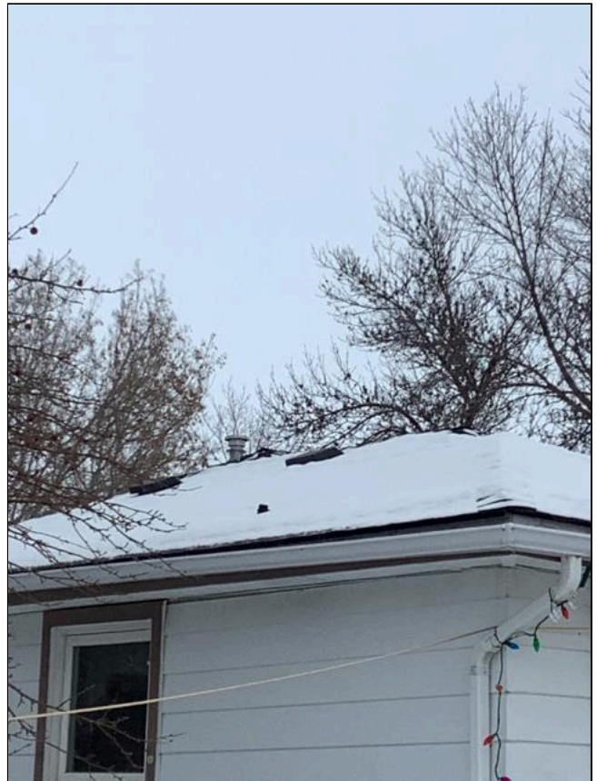
1.0 Item 12(Picture) Roof
