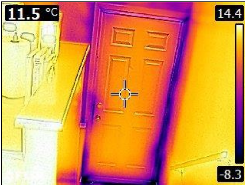
5.1 Item 40(Picture) Interior Walls
