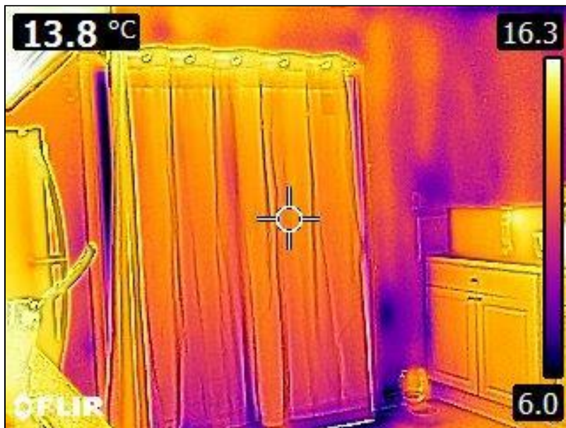
5.1 Item 34(Picture) Interior Walls
