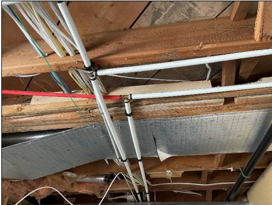
PHOTOGRAPH #9: Fibre Board - Basement Laundry (Non-Asbestos)
