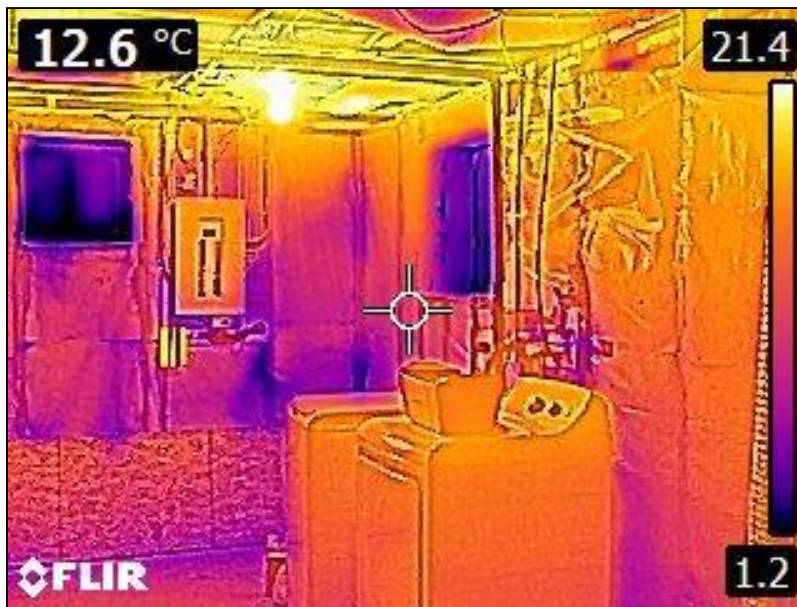
7.0 Item 1(Picture) Basement Foundation
