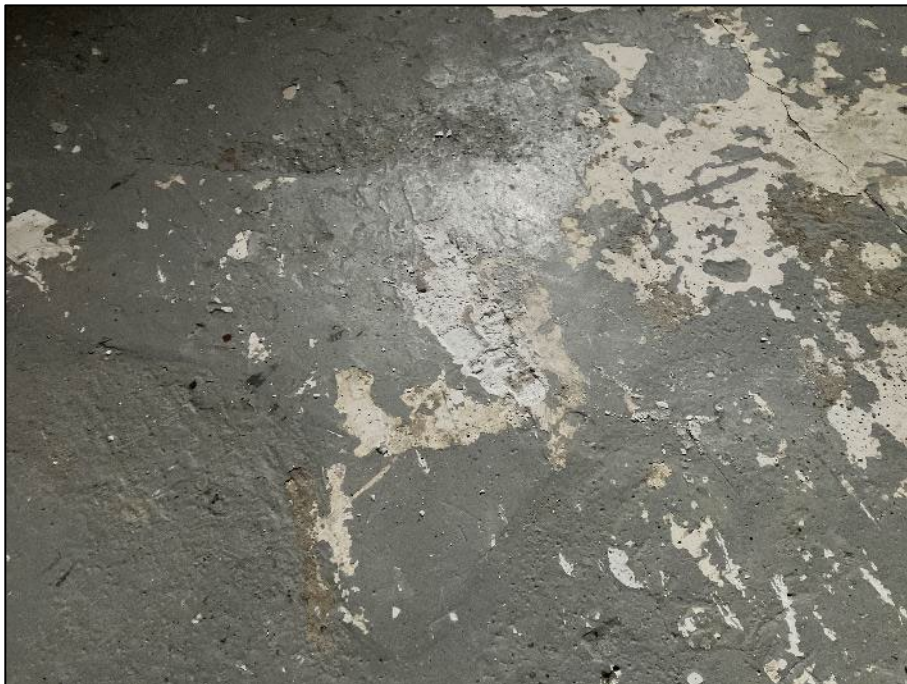
PHOTOGRAPH #14: Leveling Compound – Basement (Non-Asbestos)
