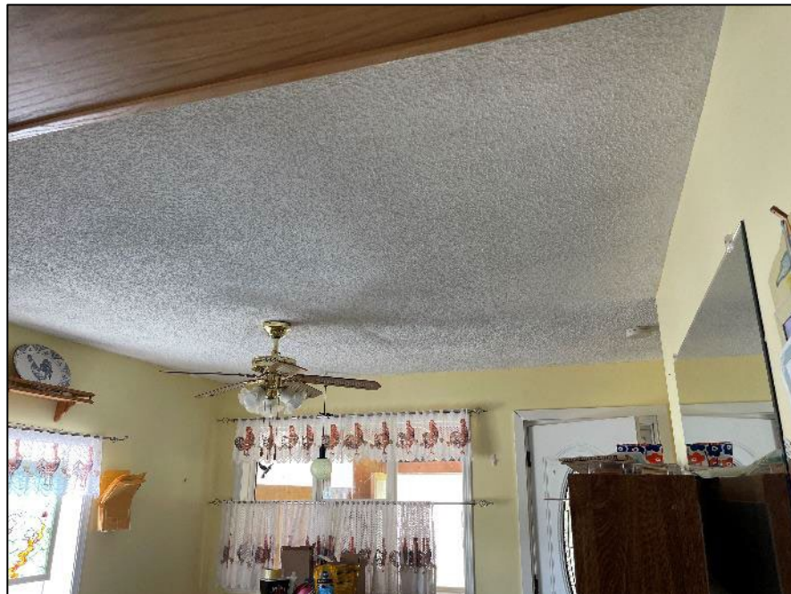
PHOTOGRAPH #8: Ceiling Texture - Level 1 Kitchen (Non-Asbestos)
