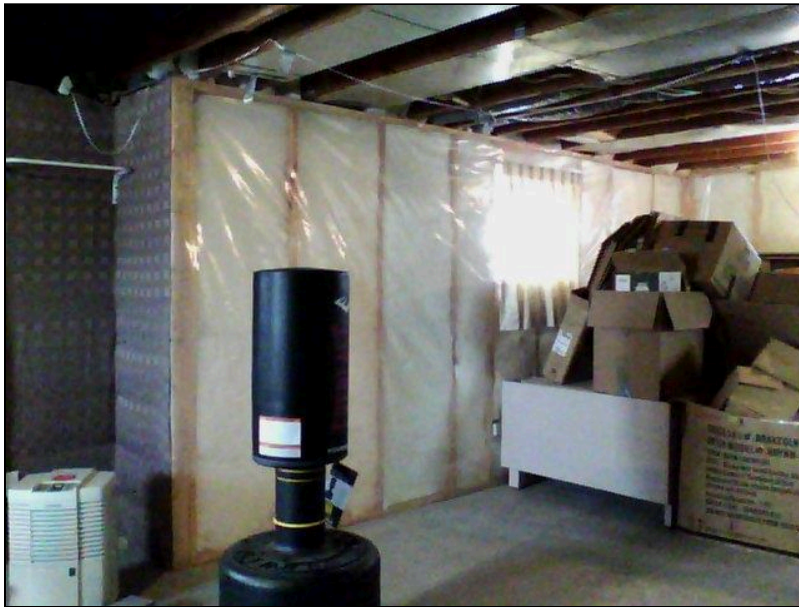
7.0 Item 10(Picture) Basement Foundation
