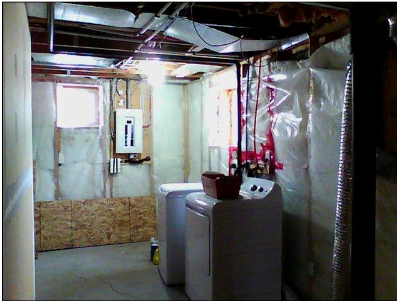
7.0 Item 2(Picture) Basement Foundation
