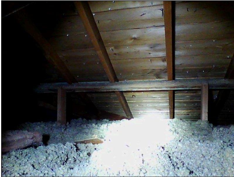
2.0 Item 14(Picture) Attic
