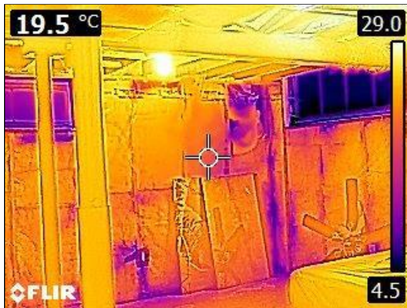
7.0 Item 1(Picture) Basement Foundation
