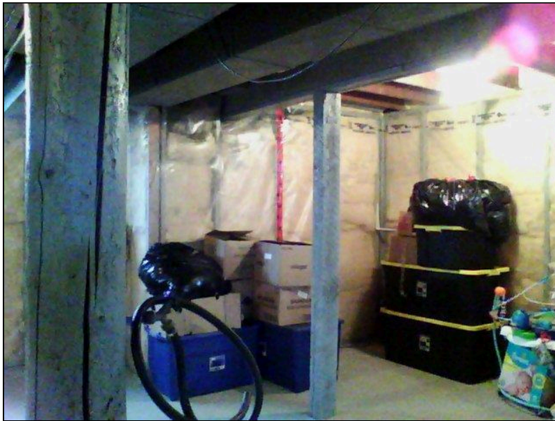
7.0 Item 18(Picture) Basement Foundation
