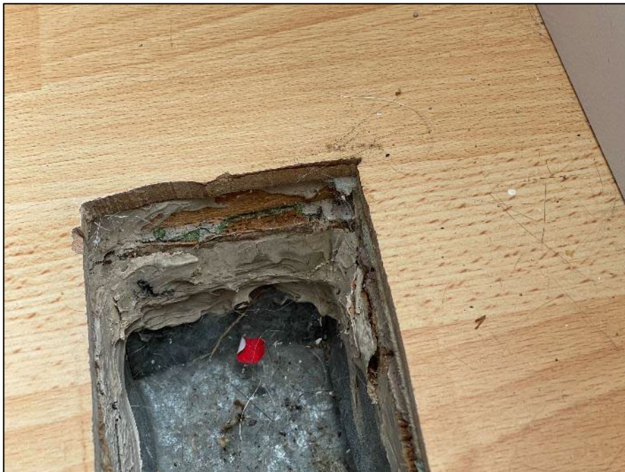
PHOTOGRAPH #12: Flooring - Level 1 Living Room (Non-Asbestos)
