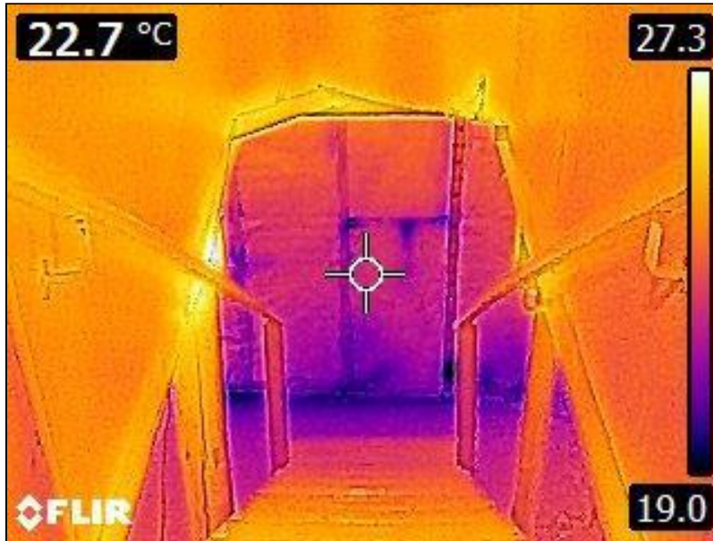
5.1 Item 47(Picture) Interior Walls
