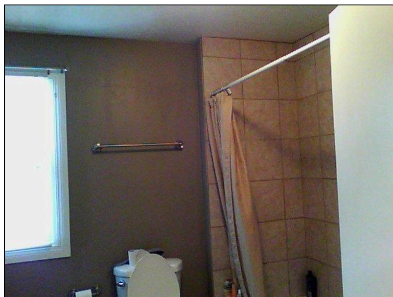
9.0 Item 5(Picture) Bathroom Walls
