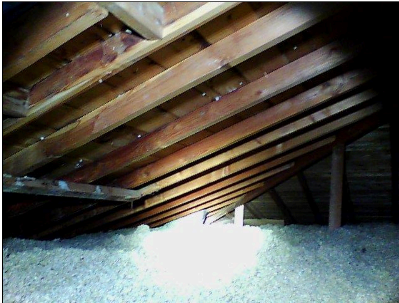
2.0 Item 6(Picture) Attic
