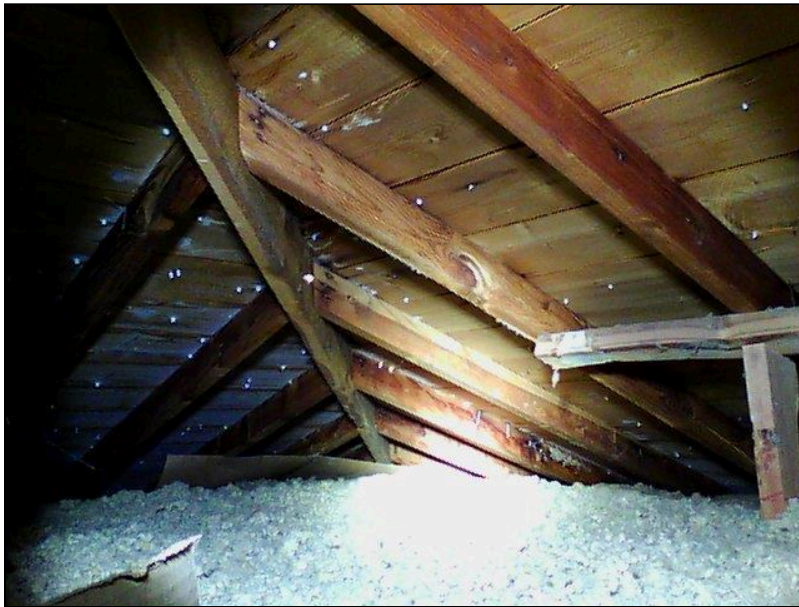
2.0 Item 10(Picture) Attic
