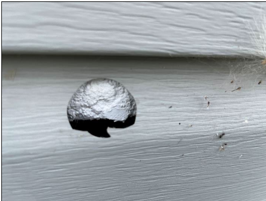
PHOTOGRAPH #12: Stucco 2 - West Face (<1% Chrysotile)
