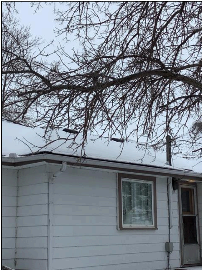
1.0 Item 11(Picture) Roof
