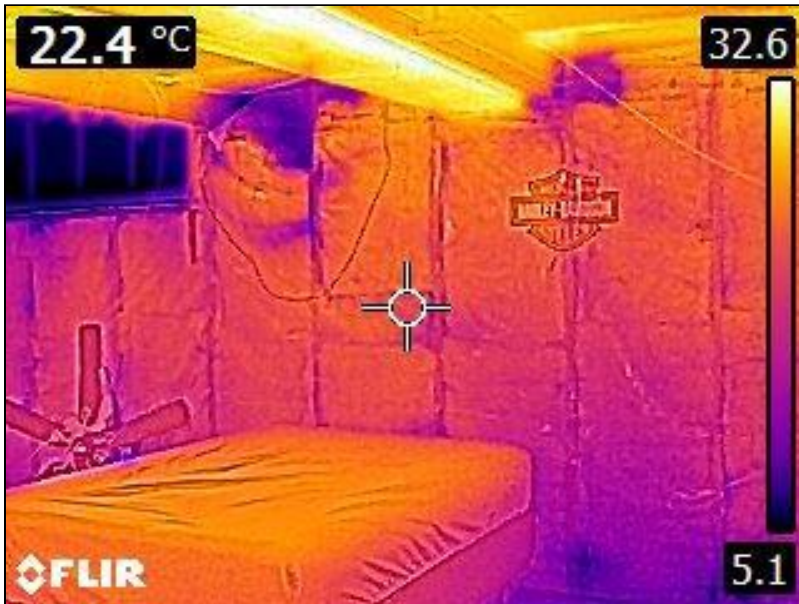
7.0 Item 3(Picture) Basement Foundation
