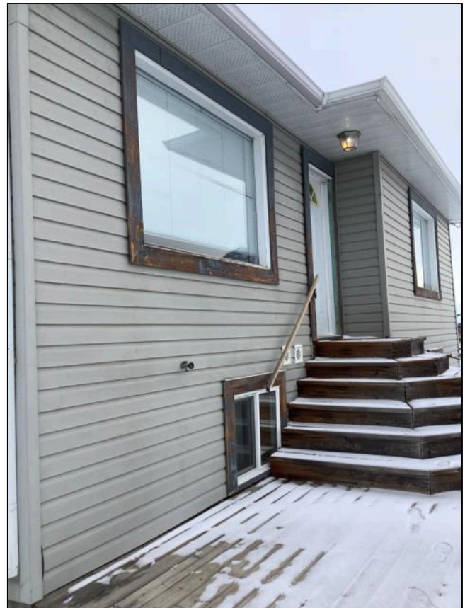
3.1 Item 2(Picture) Exterior
