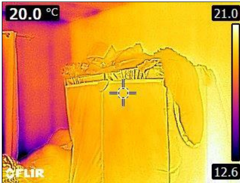
5.1 Item 5(Picture) Interior Walls
