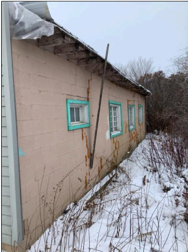
4.4 Item 3(Picture) Garage Exterior
