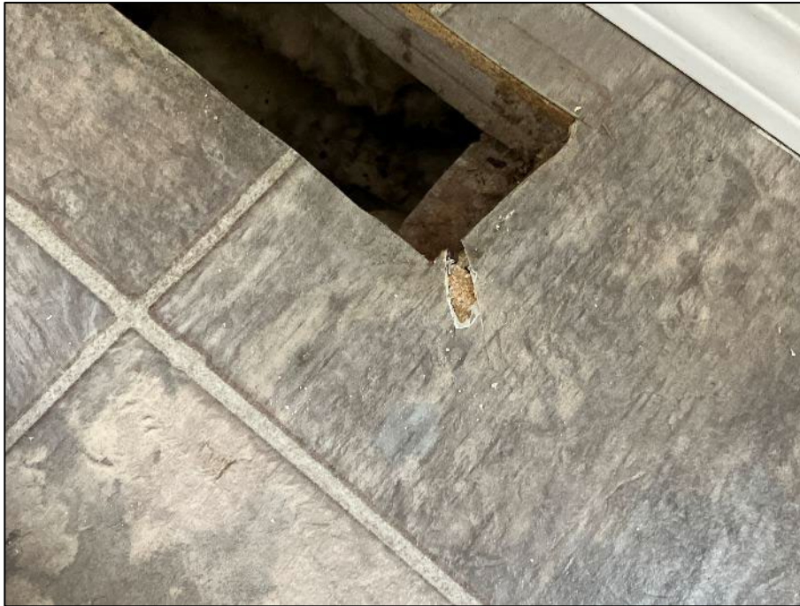
PHOTOGRAPH #11: Sheet Flooring – Floor 1 Kitchen (Non-Asbestos)
