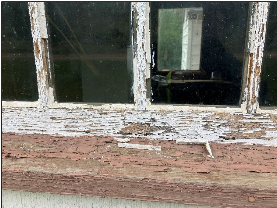
PHOTOGRAPH #16: Window Caulking – Shed (Non-Asbestos)
