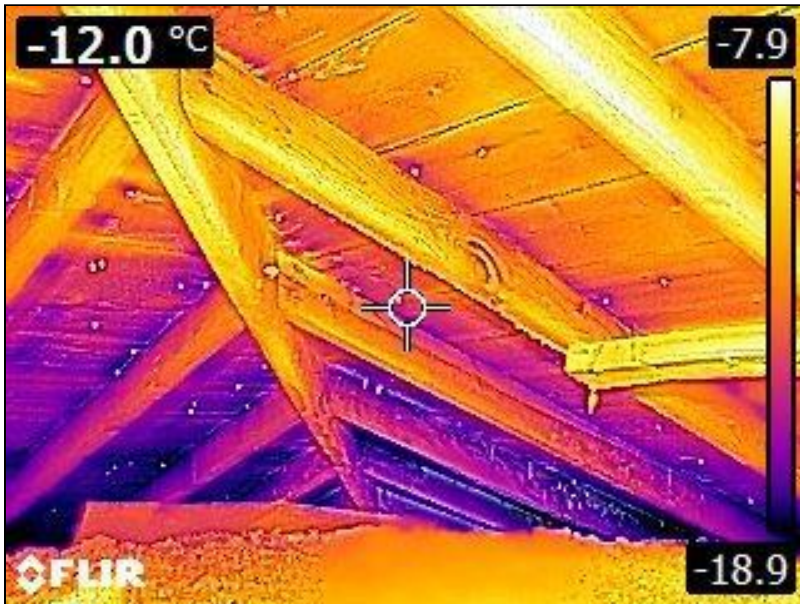
2.0 Item 9(Picture) Attic
