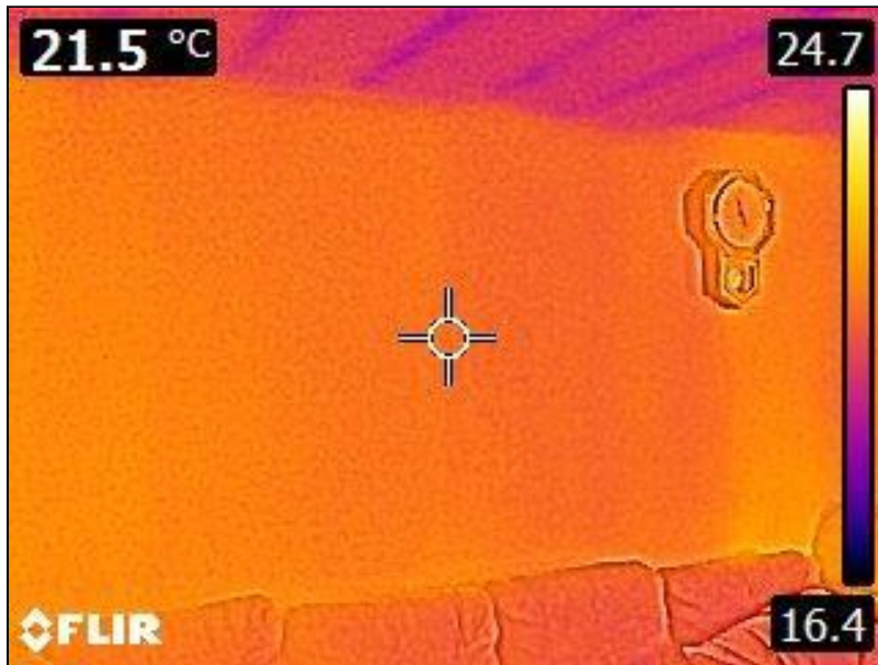
5.1 Item 21(Picture) Interior Walls
