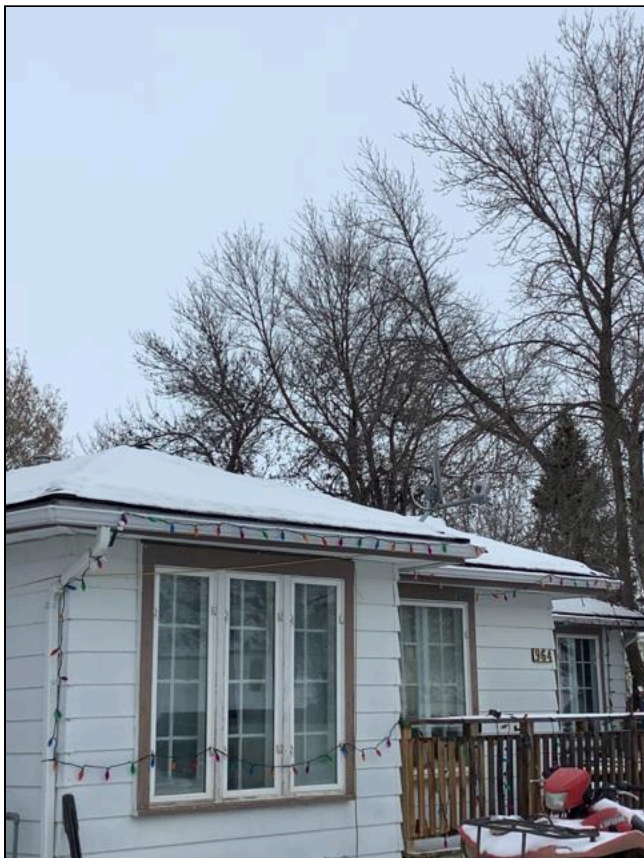
1.0 Item 13(Picture) Roof
