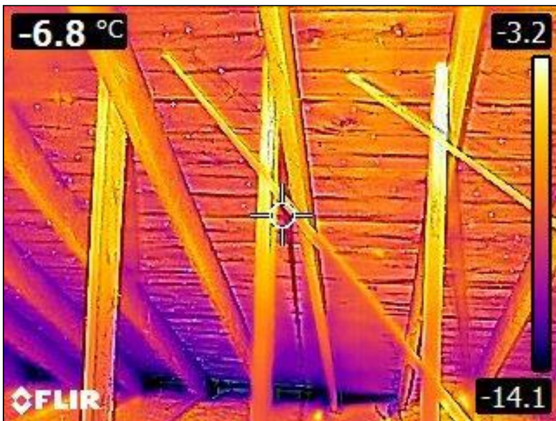
2.0 Item 7(Picture) Attic
