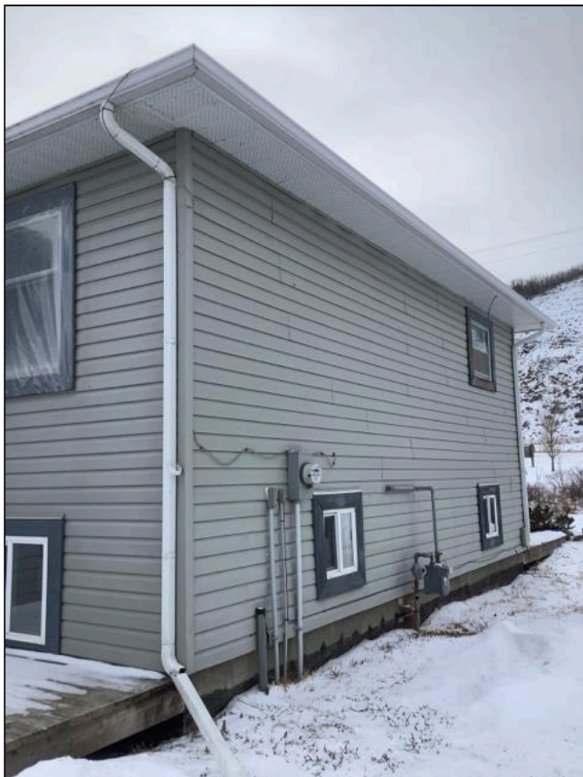
3.1 Item 3(Picture) Exterior
