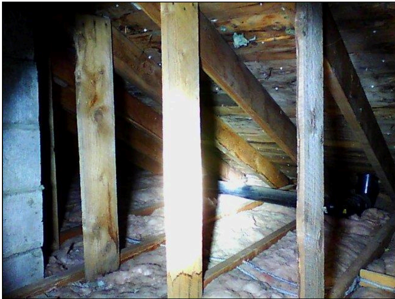
2.0 Item 12(Picture) Attic
