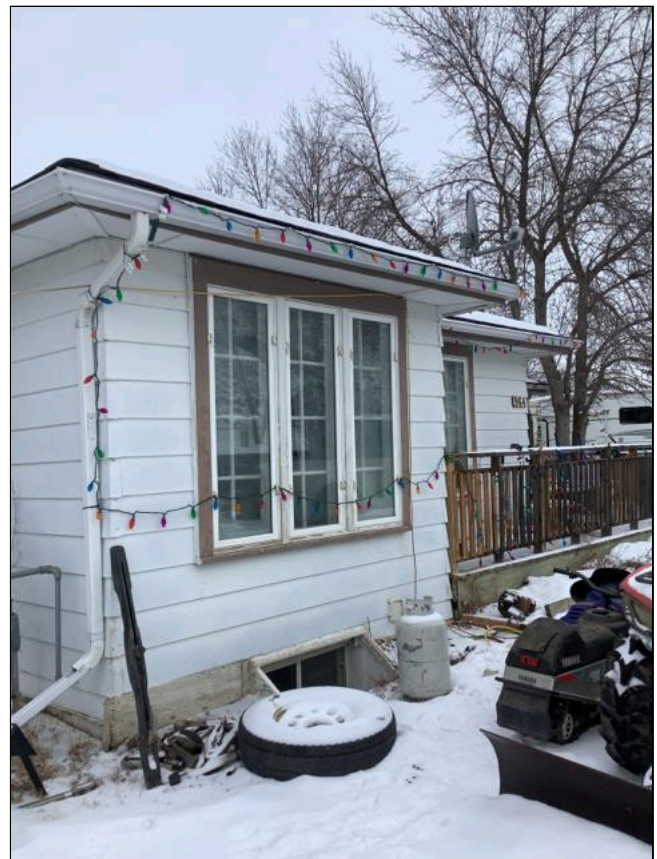
3.1 Item 2(Picture) Exterior
