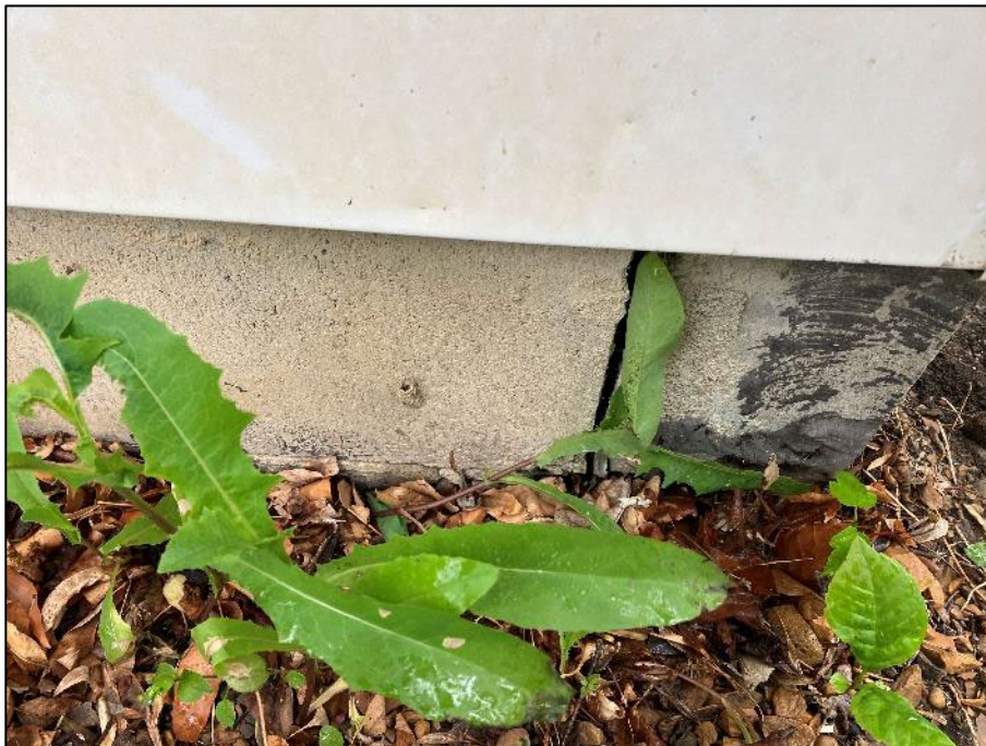
PHOTOGRAPH #18: Parging 2 – Exterior (Non-Asbestos)
