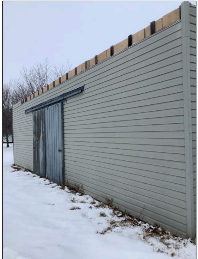
4.4 Item 2(Picture) Garage Exterior
