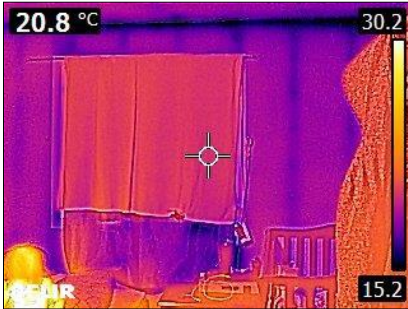
5.1 Item 15(Picture) Interior Walls
