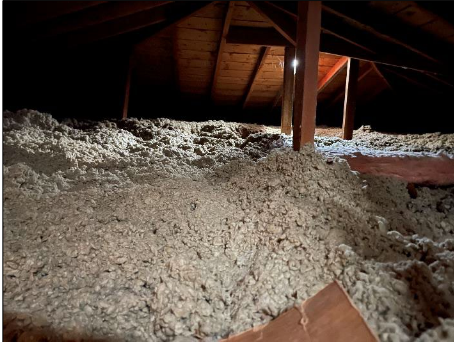
PHOTOGRAPH #13: Attic Insulation (Non-Asbestos)
