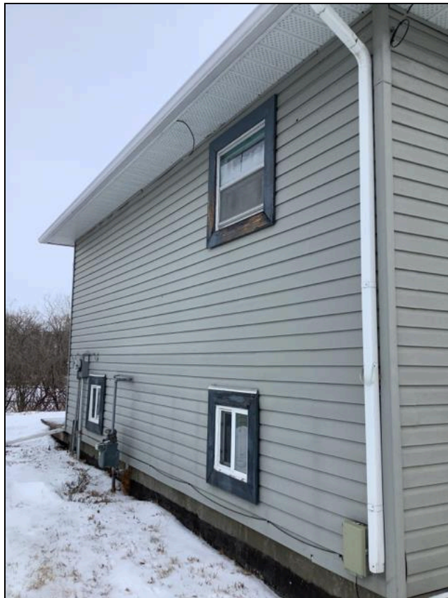
3.1 Item 1(Picture) Exterior
