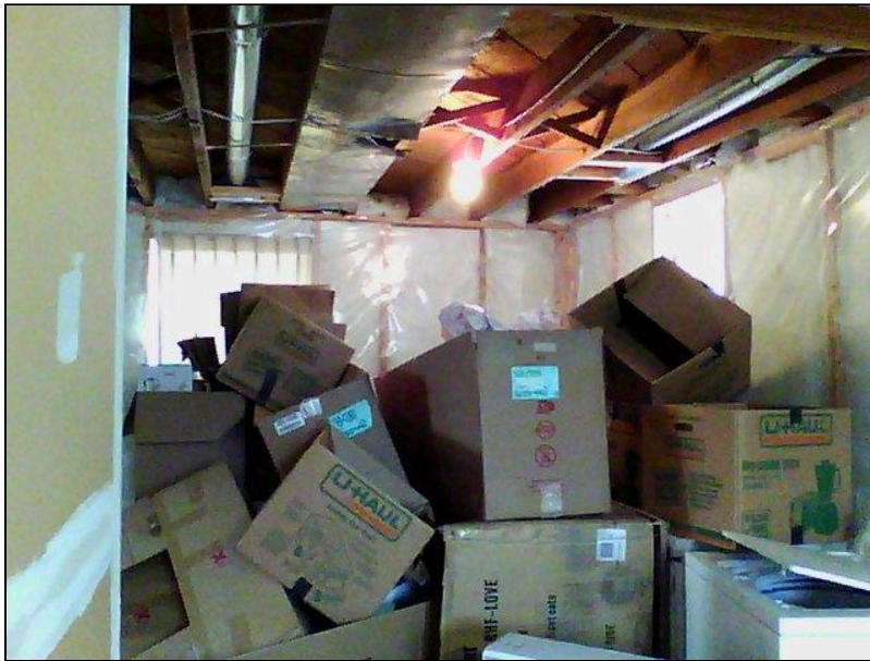
7.0 Item 6(Picture) Basement Foundation
