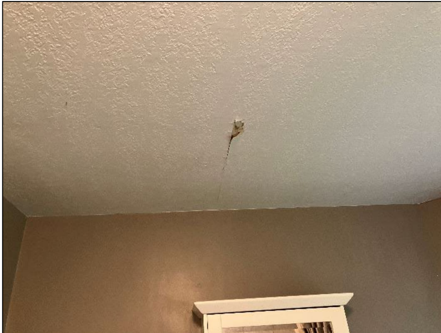
PHOTOGRAPH #9: Ceiling Texture - Floor 1 Bathroom (Non-Asbestos)
