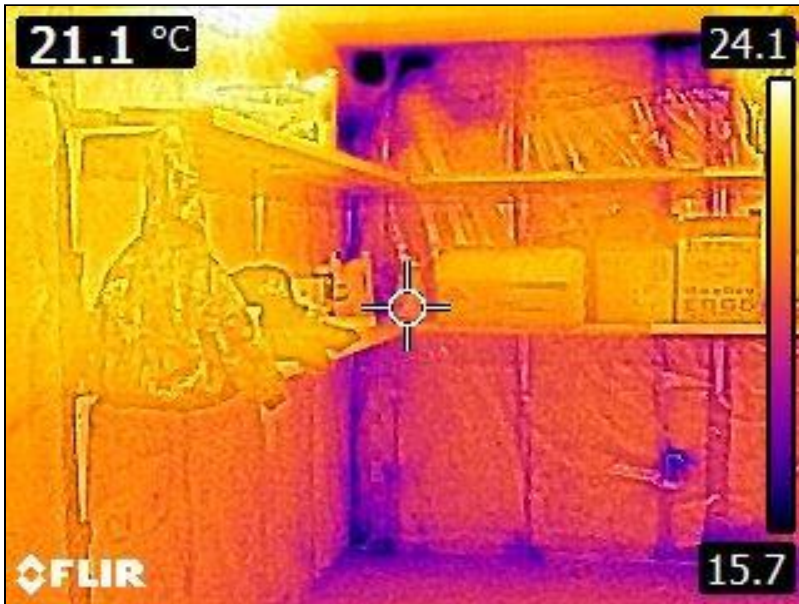
7.0 Item 25(Picture) Basement Foundation
