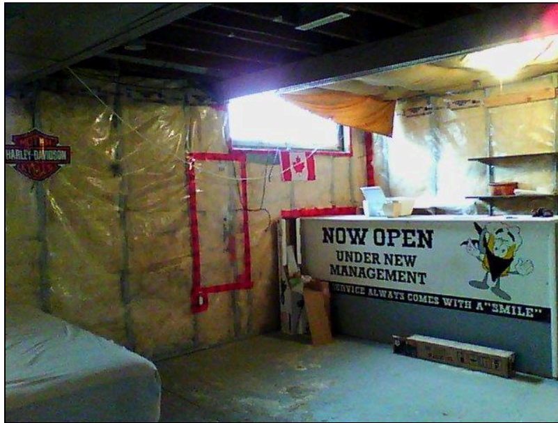
7.0 Item 6(Picture) Basement Foundation
