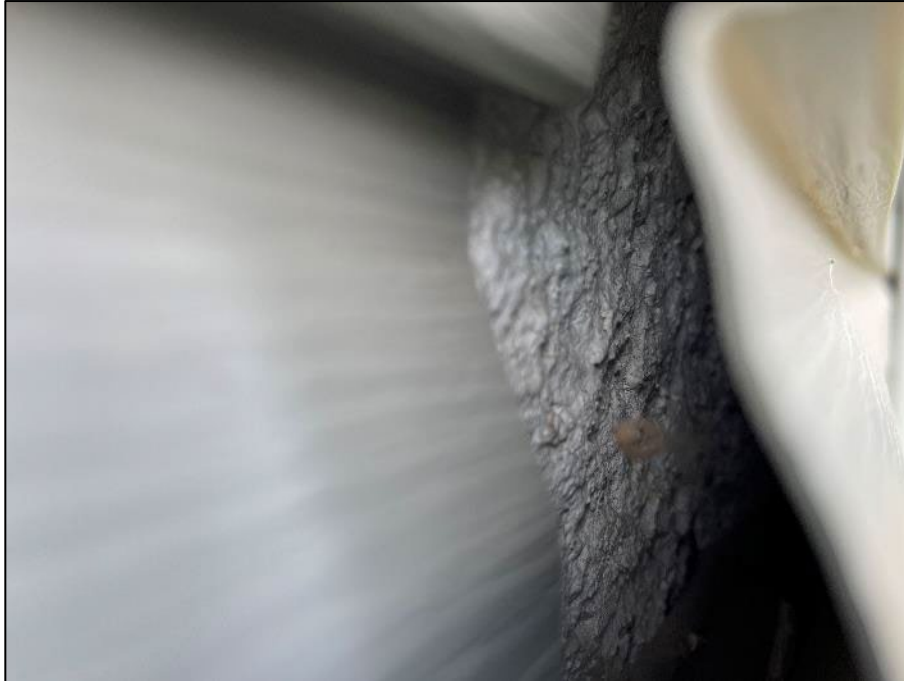
PHOTOGRAPH #11: Stucco 1 - West Face (<1% Chrysotile)
