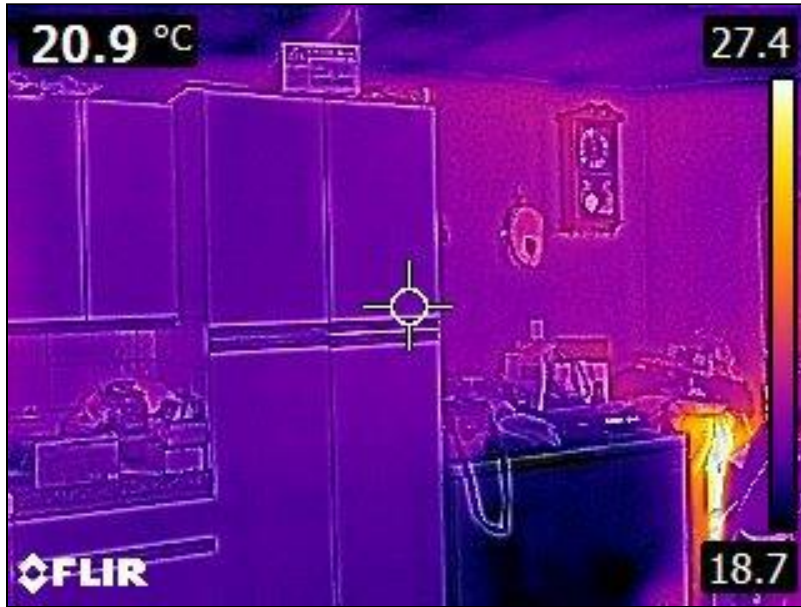
5.1 Item 43(Picture) Interior Walls
