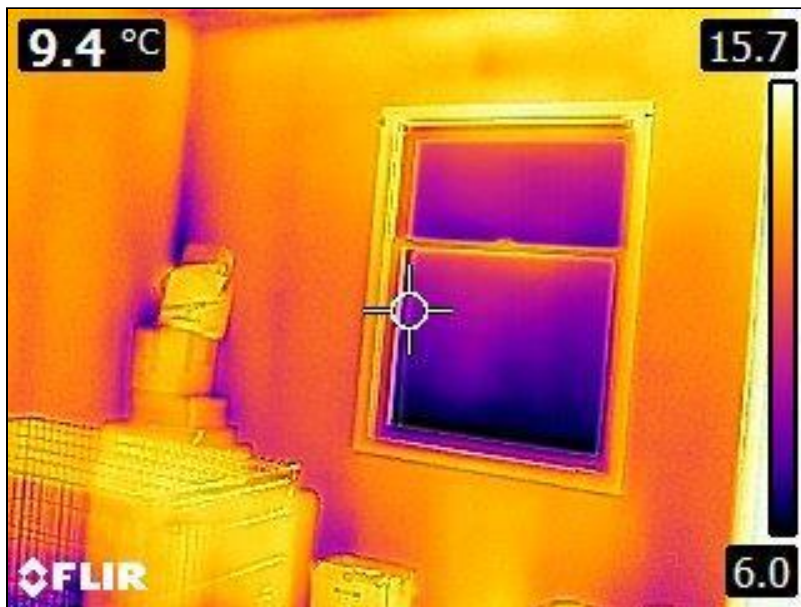
5.1 Item 12(Picture) Interior Walls
