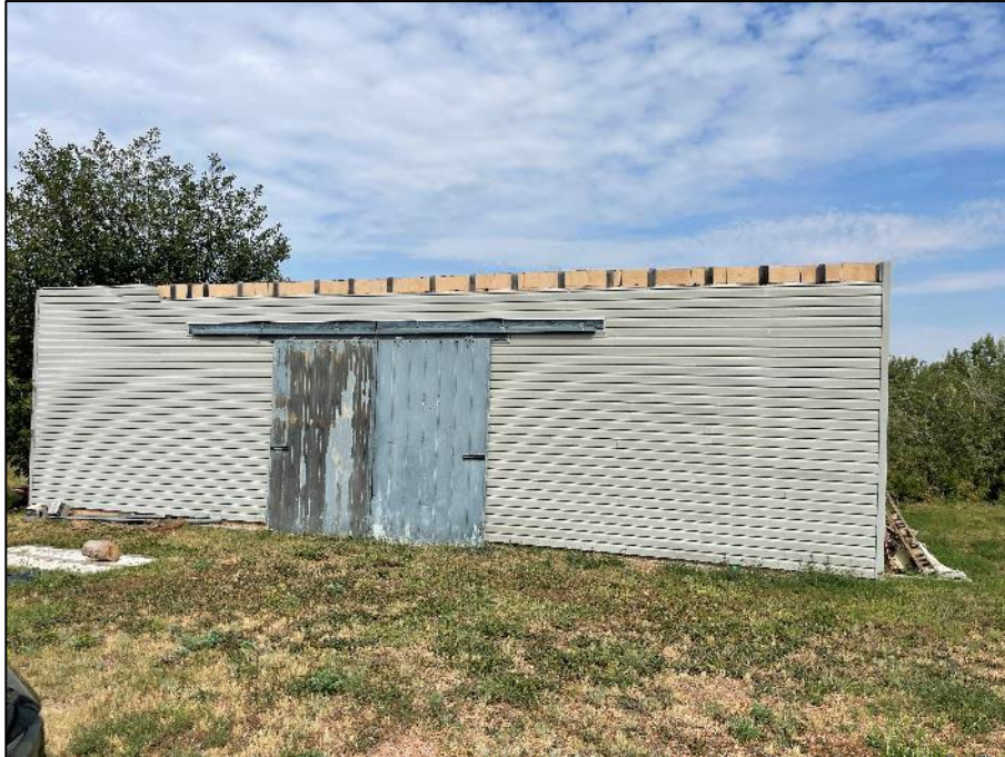
PHOTOGRAPH #23: Grey Paint – Garage Door (Lead Based)
