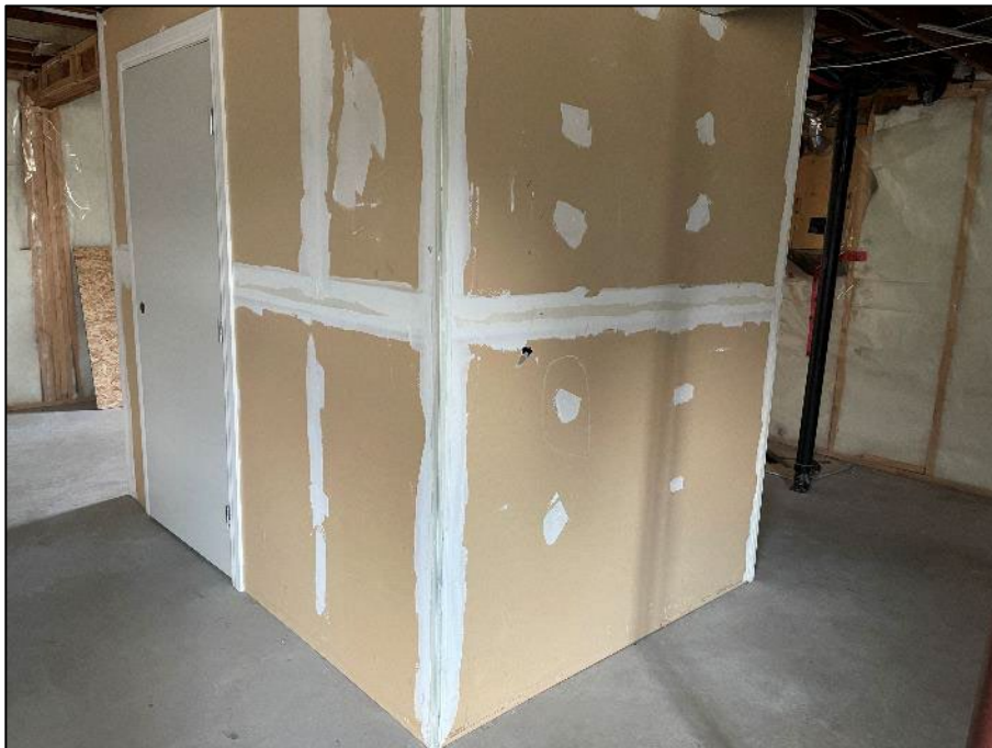
PHOTOGRAPH #14: Drywall Joint Compound - Basement Furnace Room (Non-Asbestos)
