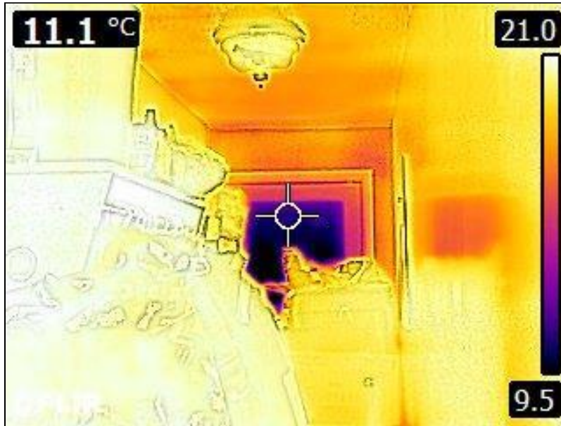
5.1 Item 19(Picture) Interior Walls
