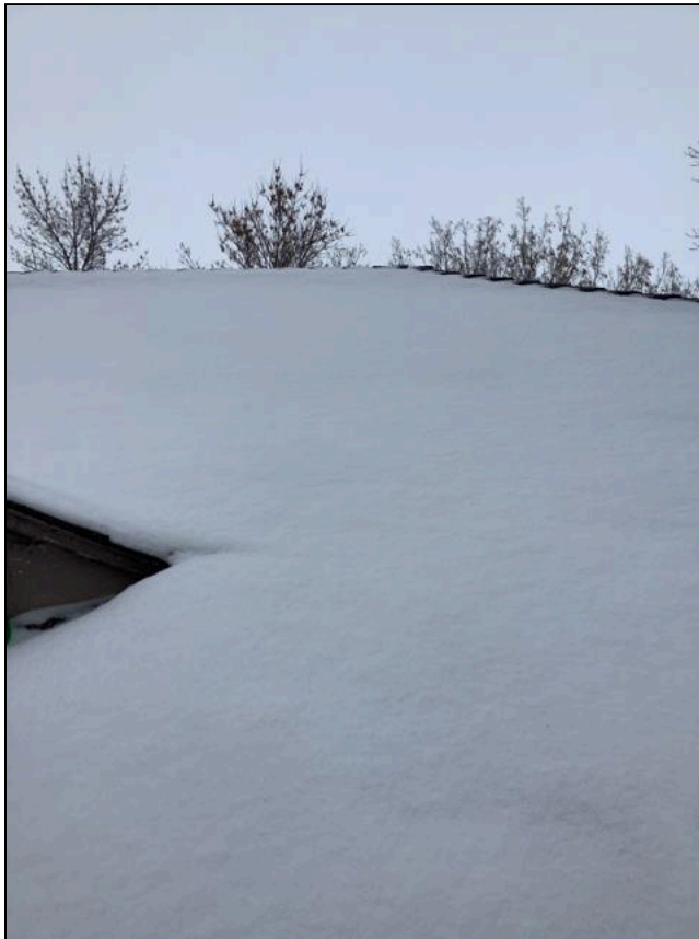
1.0 Item 1(Picture) Roof
