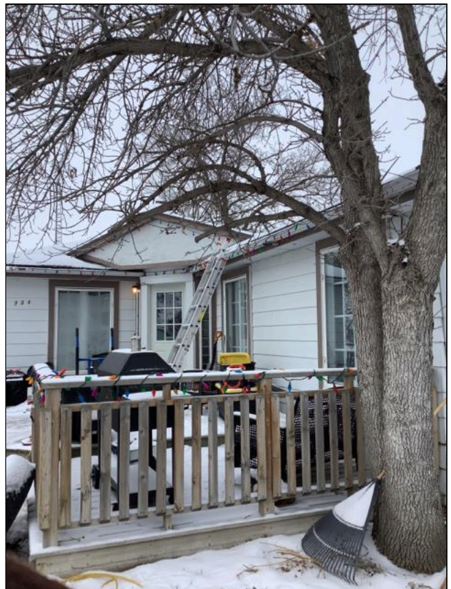
3.1 Item 8(Picture) Exterior
