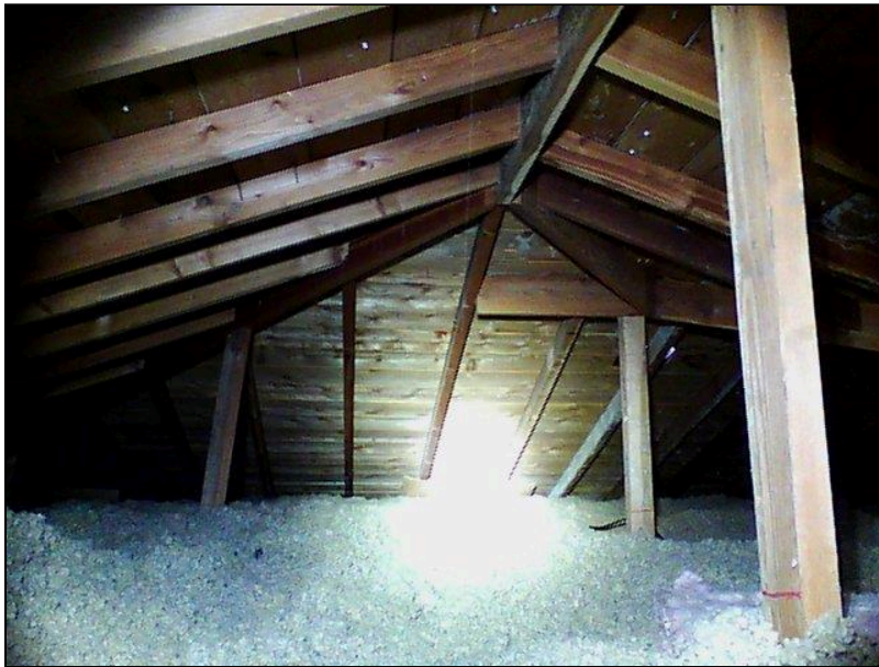
2.0 Item 4(Picture) Attic
