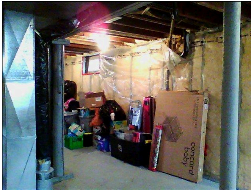
7.0 Item 12(Picture) Basement Foundation
