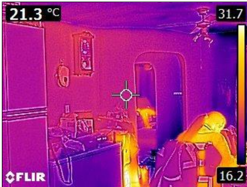
5.1 Item 41(Picture) Interior Walls
