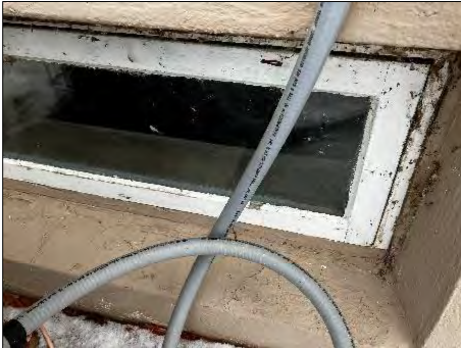
PHOTOGRAPH #22: Window Caulking Exterior (3% Chrysotile)
