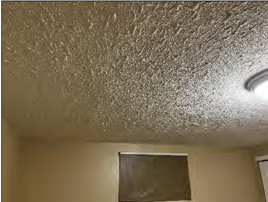
PHOTOGRAPH #7: Ceiling Texture - Basement Bedroom (None Detected)
