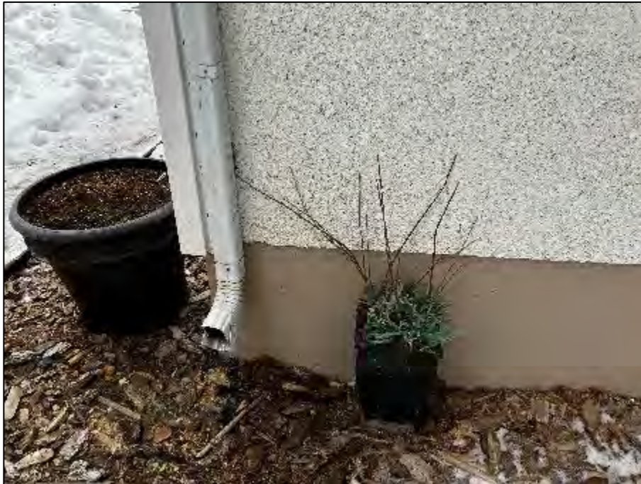
PHOTOGRAPH #20: Stucco - North Exterior (2% Chrysotile)
