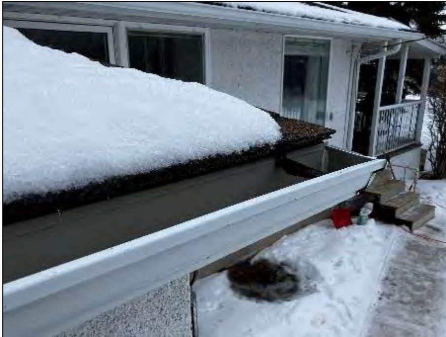
PHOTOGRAPH #24: Roof Shingle - House Exterior (None Detected)
