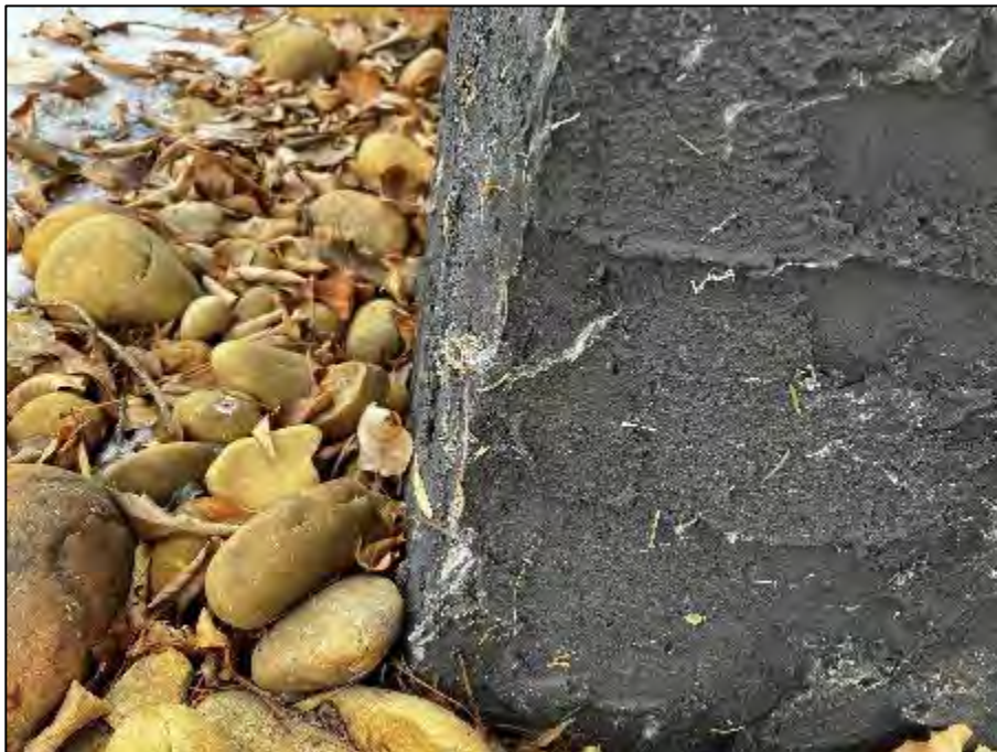
PHOTOGRAPH #20: Parging - Front Exterior (None Detected)
