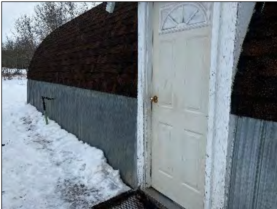
PHOTOGRAPH #23: Shed Roof Exterior (None Detected)
