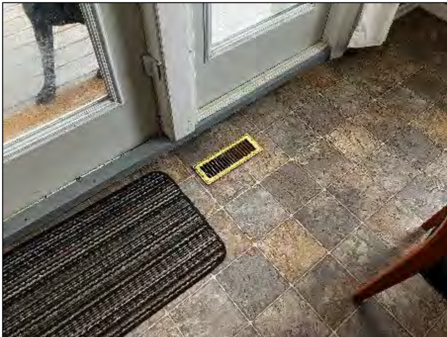
PHOTOGRAPH #10: Sheet Flooring - Level 1 Dining Room (None Detected)
