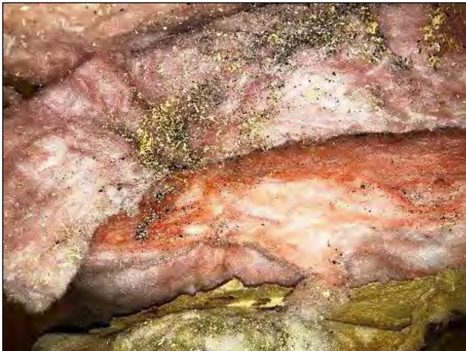
PHOTOGRAPH #16: Attic Insulation (None Detected)
