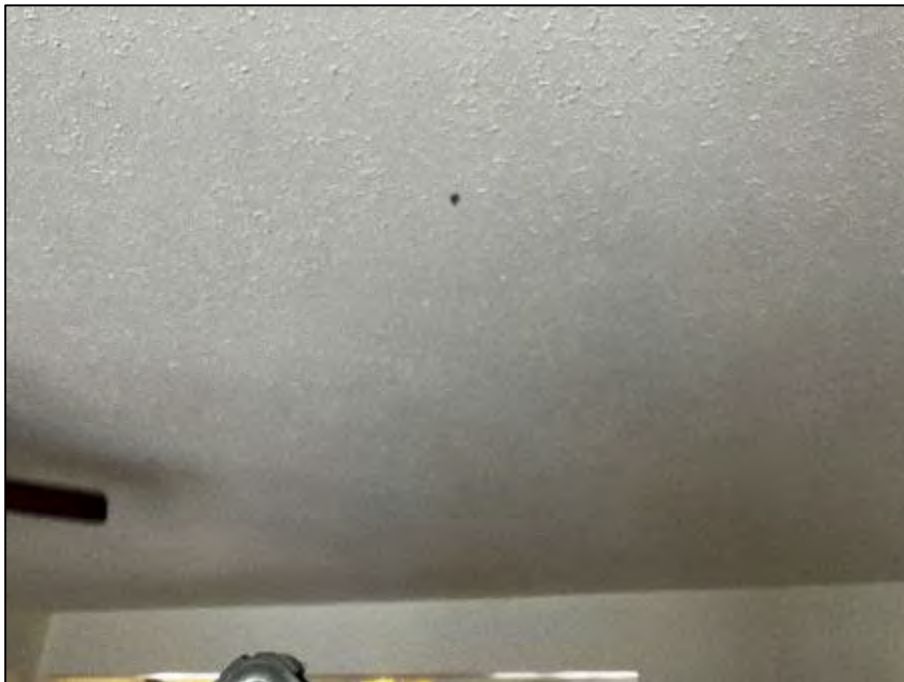
PHOTOGRAPH #12: Ceiling Texture - Level 1 Dining Room Popcorn (None Detected)
