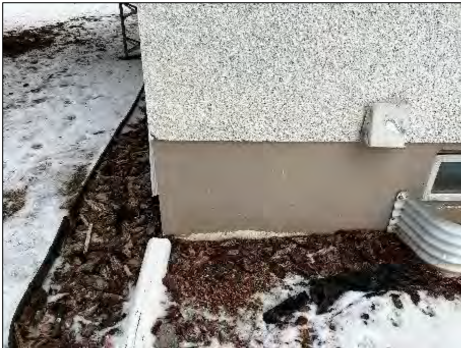
PHOTOGRAPH #29: Paint - Exterior House Brown (670 ppm Lead)
