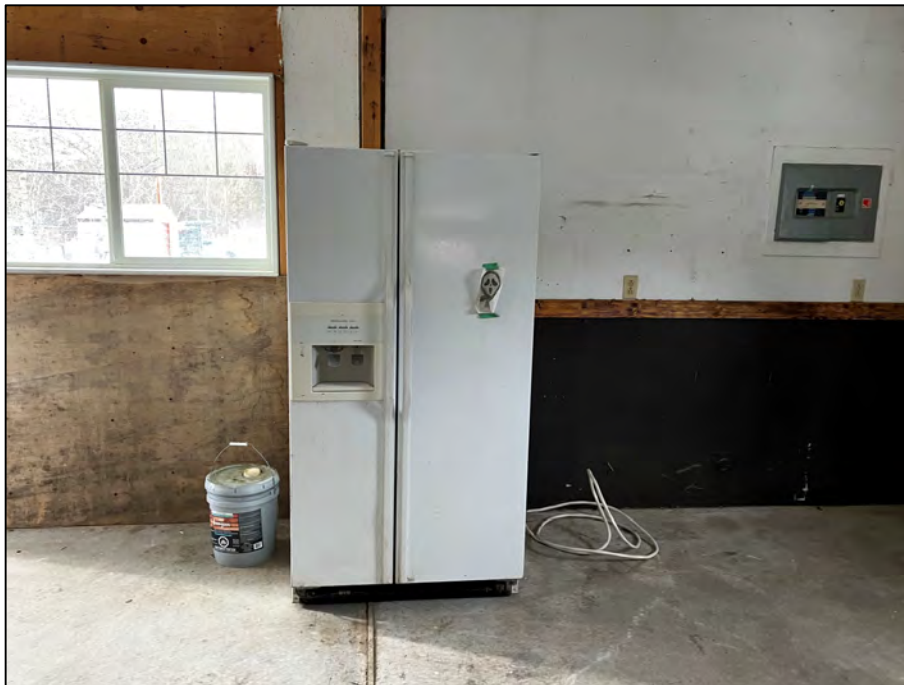
PHOTOGRAPH #11: Ozone Depleting Substances in Fridge
