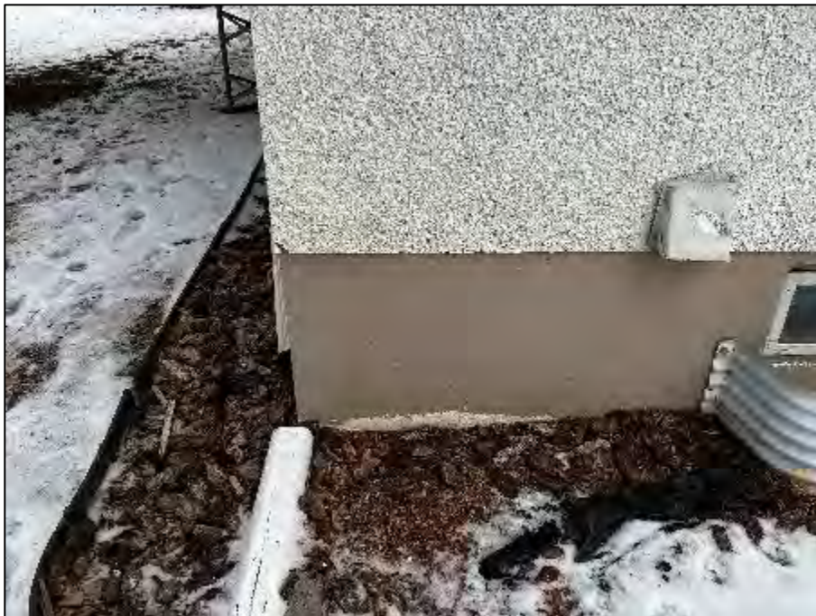
PHOTOGRAPH #19: Stucco - South Exterior (2% Chrysotile)
