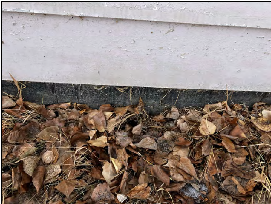
PHOTOGRAPH #16: Parging - Exterior (None Detected)
