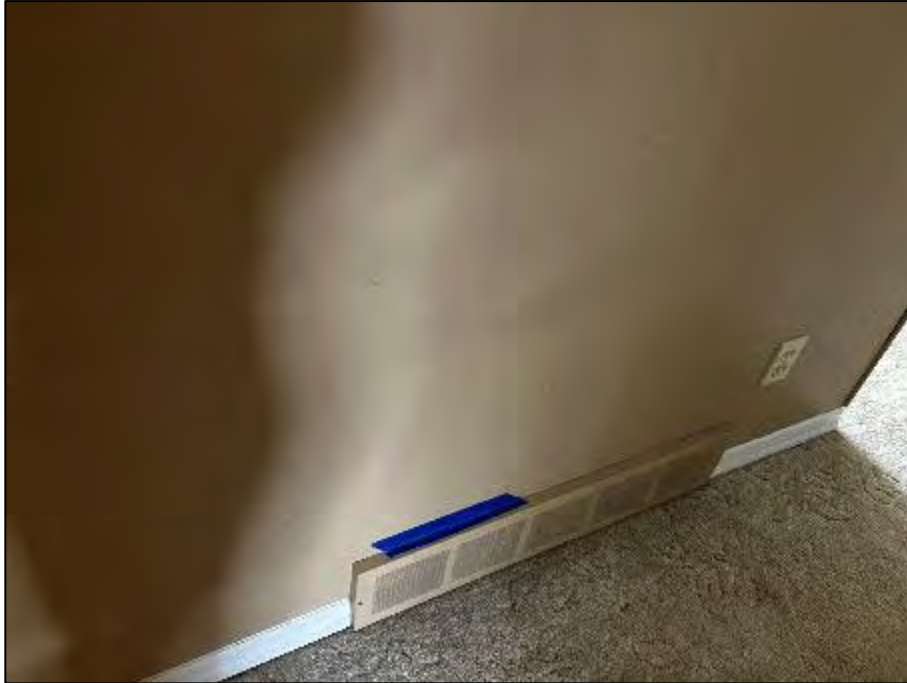
PHOTOGRAPH #14: Plaster - Level 1 Hallway Interior (None Detected)
