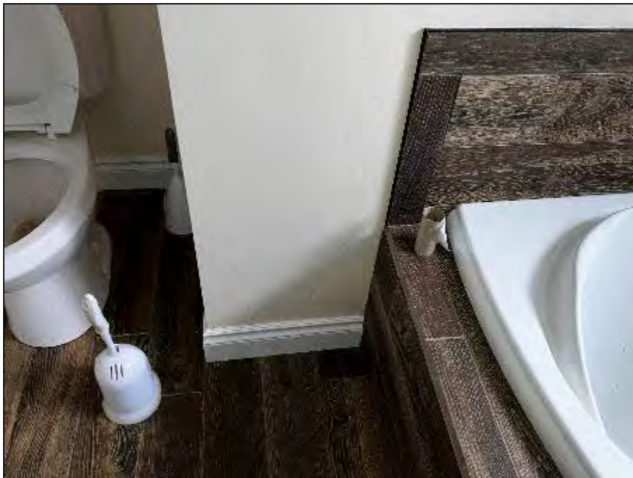
PHOTOGRAPH #10: Drywall Joint Compound - Level 1 Bathroom Interior (None Detected)
