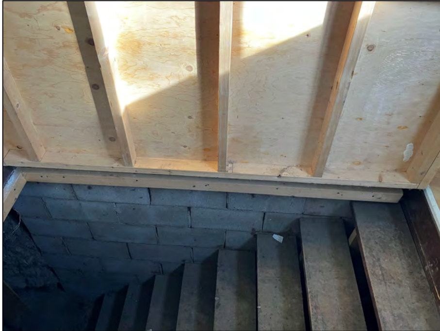
PHOTOGRAPH #15: Brick Mortar - Stairs (None Detected)
