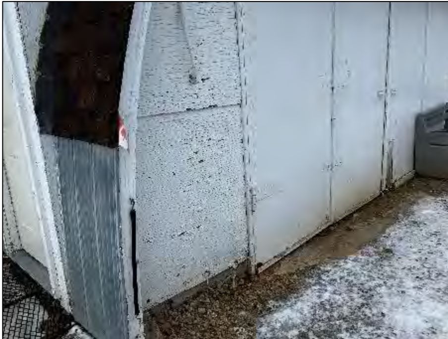
PHOTOGRAPH #30: Paint - Shed White (<80 ppm Lead)
