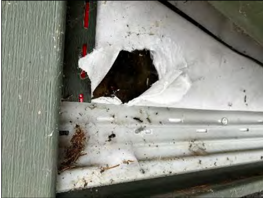
PHOTOGRAPH #17: Siding Paper (None Detected)
