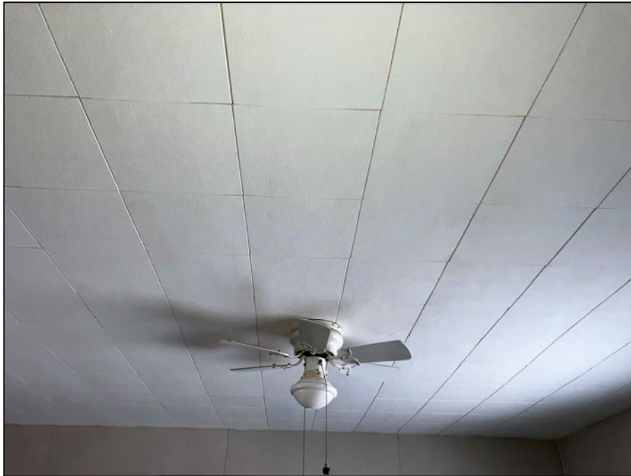
PHOTOGRAPH #9: Ceiling Tile - Level 1 Main Room (None Detected)
