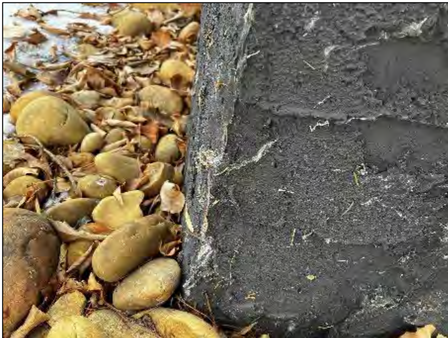
PHOTOGRAPH #24: Paint - Parging Exterior (<80 ppm Lead)
