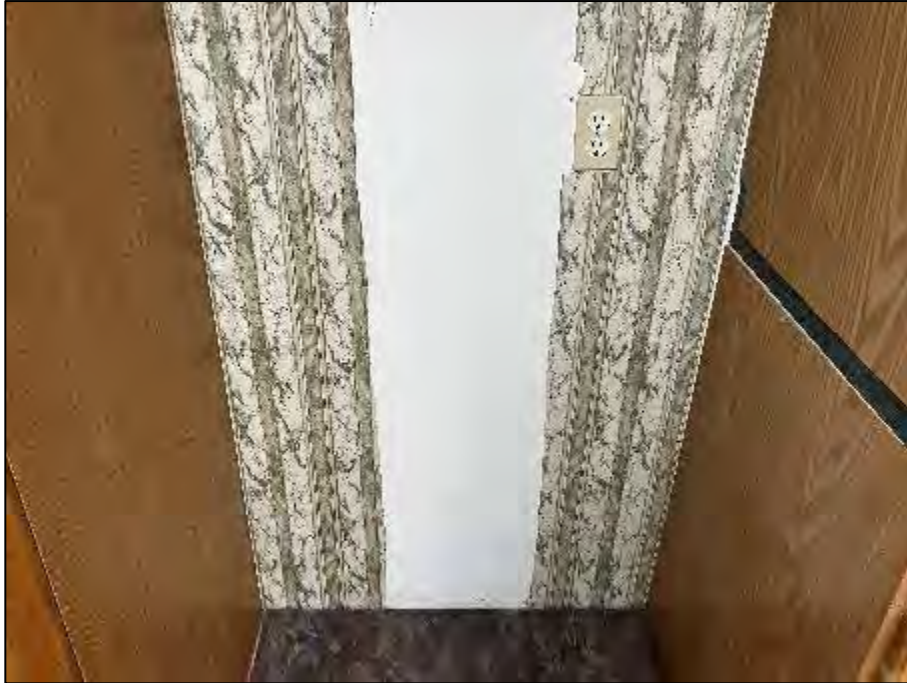
PHOTOGRAPH #15: Wall Paper - Level 1 Kitchen (None Detected)
