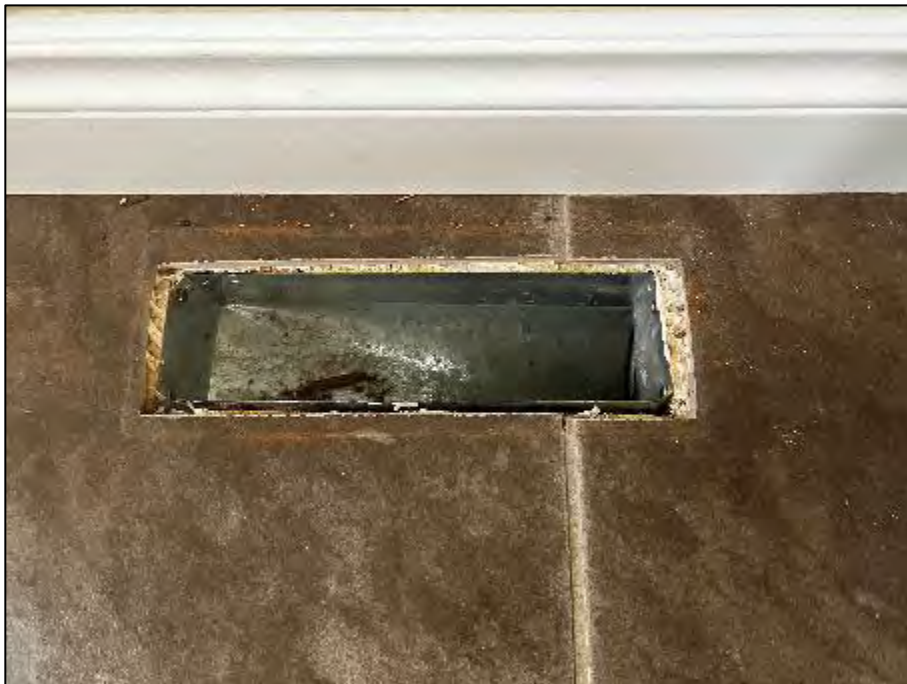
PHOTOGRAPH #18: Flooring - Level 1 Foyer (None Detected)
