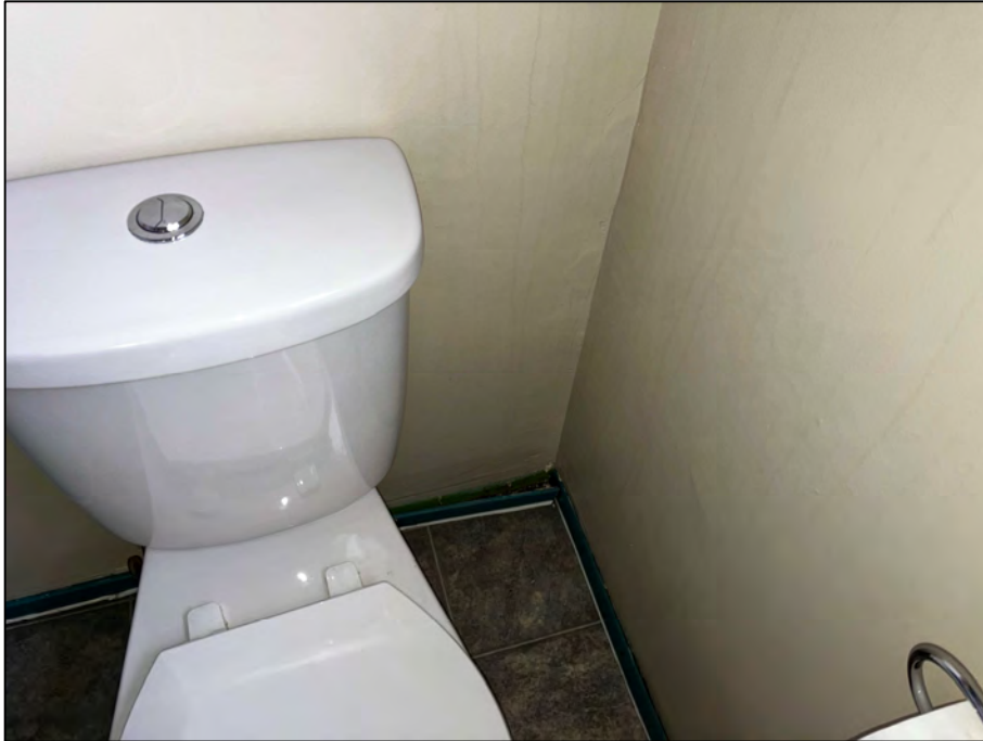
PHOTOGRAPH #3: Drywall Joint Compound - Level 1 Bathroom Exterior (2% Chrysotile)
