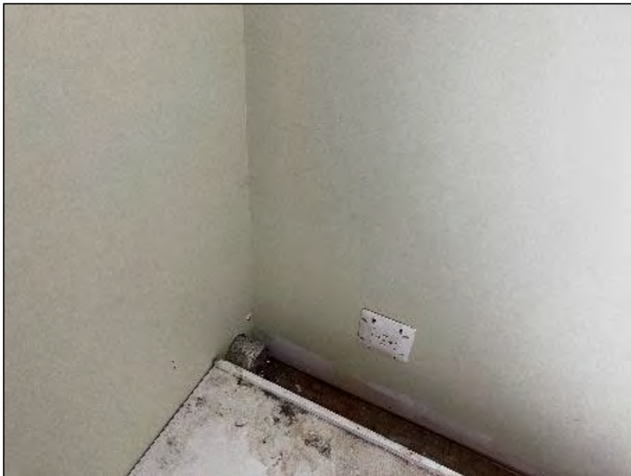
PHOTOGRAPH #4: Drywall Joint Compound - Level 1 Laundry Room Exterior (None Detected)
