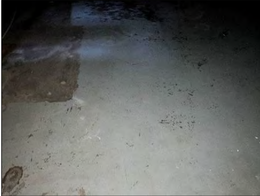
PHOTOGRAPH #23: Paint - Basement Floor Grey (<80 ppm Lead)
