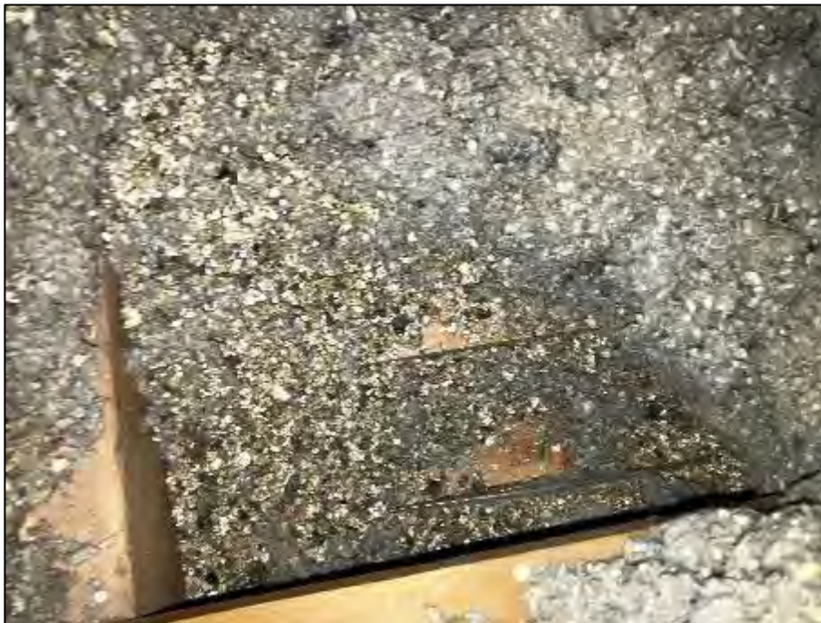
PHOTOGRAPH #27: Vermiculite - Attic (<1% Actinolite)
