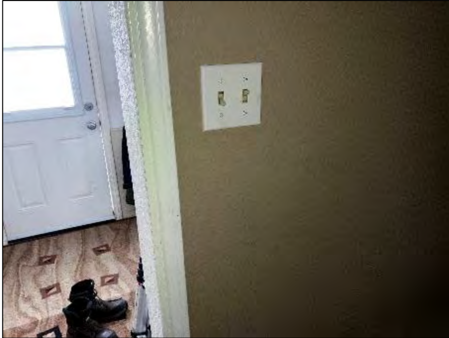
PHOTOGRAPH #16: Plaster - Level 1 Back Door Interior (None Detected)
