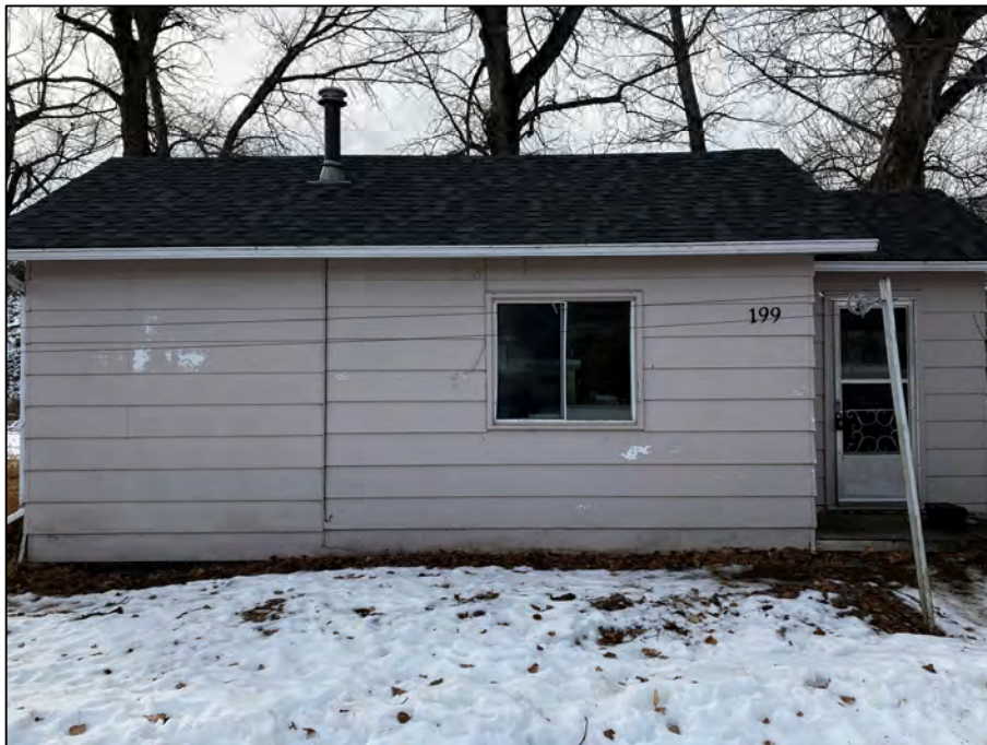
PHOTOGRAPH #20: Paint - Exterior Beige (<80 ppm Lead)
