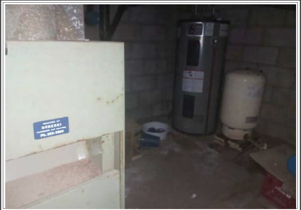
Utility Room Basement
