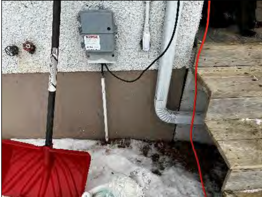
PHOTOGRAPH #18: Stucco - Back Exterior (2% Chrysotile)
