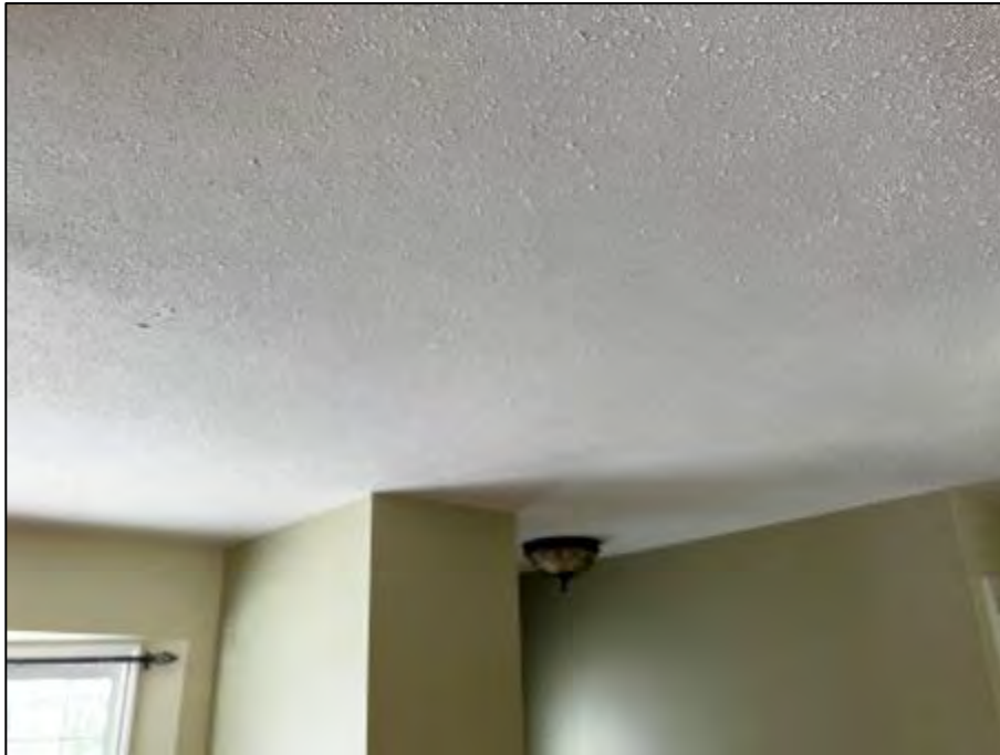
PHOTOGRAPH #11: Ceiling Texture - Level 1 Foyer Popcorn (None Detected)
