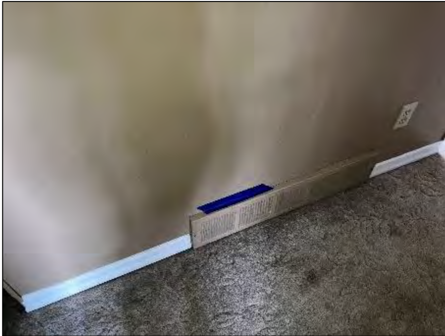
PHOTOGRAPH #28: Paint - Level 1 Hallway Brown (160 ppm Lead)
