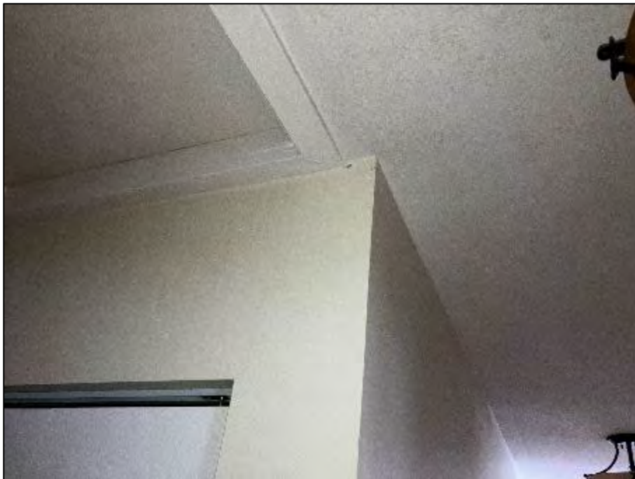
PHOTOGRAPH #6: Drywall Joint Compound - Level 1 Hallway Interior (None Detected)
