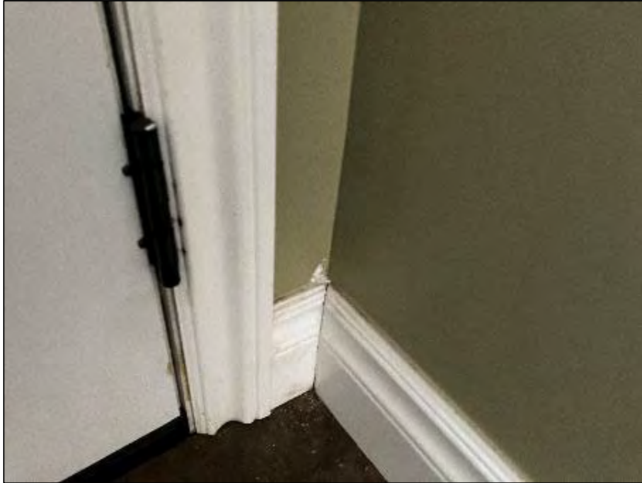
PHOTOGRAPH #5: Drywall Joint Compound - Level 1 Foyer Exterior (None Detected)
