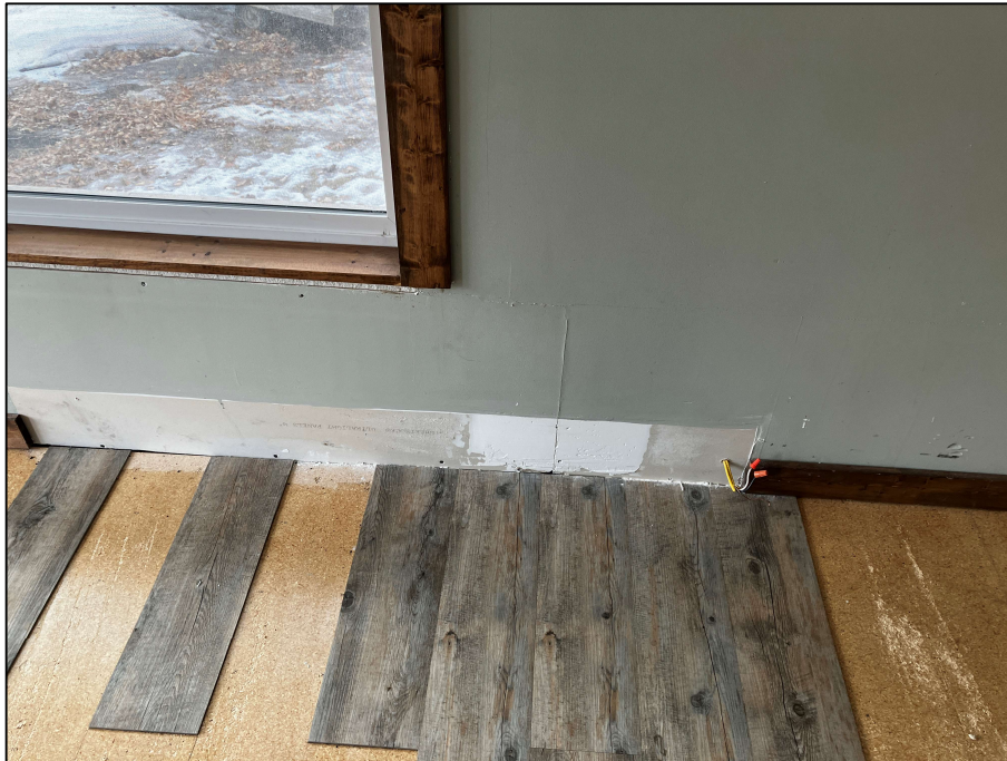
PHOTOGRAPH #3: Drywall Joint Compound - Level 1 Kitchen Exterior (None Detected)
