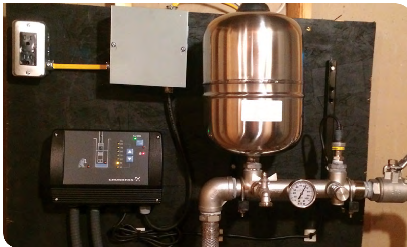
Figure 3-8, VFD System
