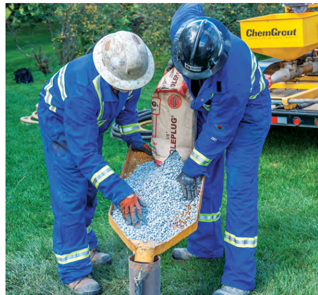
Figure 8-3, Pouring Bentonite Chips
