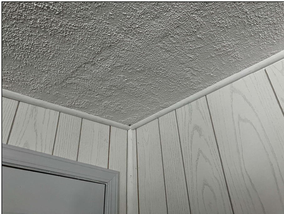
PHOTOGRAPH #6: Drywall Joint Compound - Level 1 Living Room Ceiling (None Detected)
