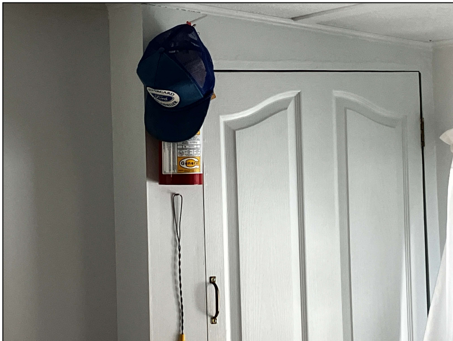
PHOTOGRAPH #33: Fire Extinguisher in Back Room
