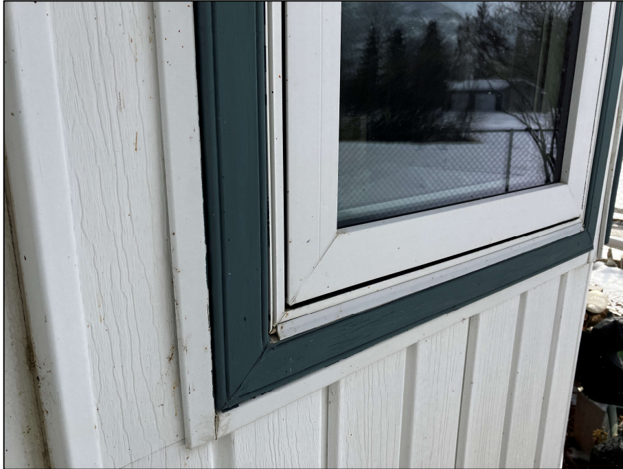
PHOTOGRAPH #21: Caulking - Exterior of Home (None Detected)
