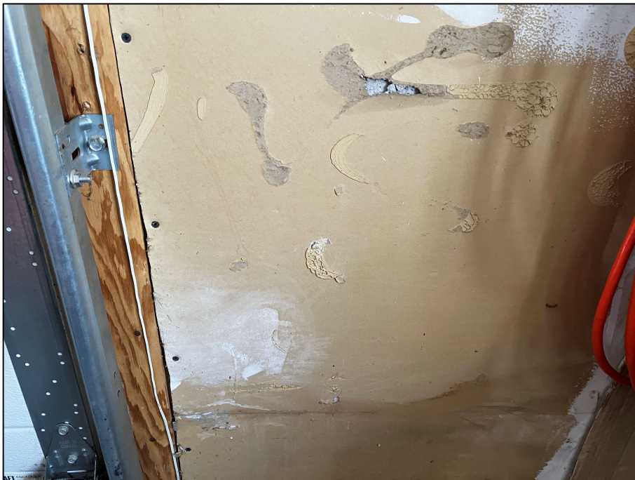
PHOTOGRAPH #20: Mastic - Level 1 Garage (None Detected)
