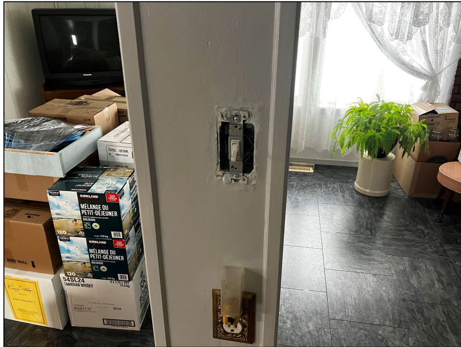
PHOTOGRAPH #3: Drywall Joint Compound - Level 1 Kitchen Pillar Interior (None Detected)
