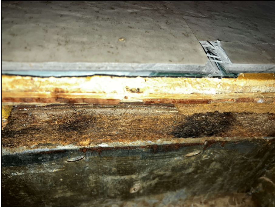
PHOTOGRAPH #19: Flooring - Level 1 Bathroom Layer 2 (None Detected)
