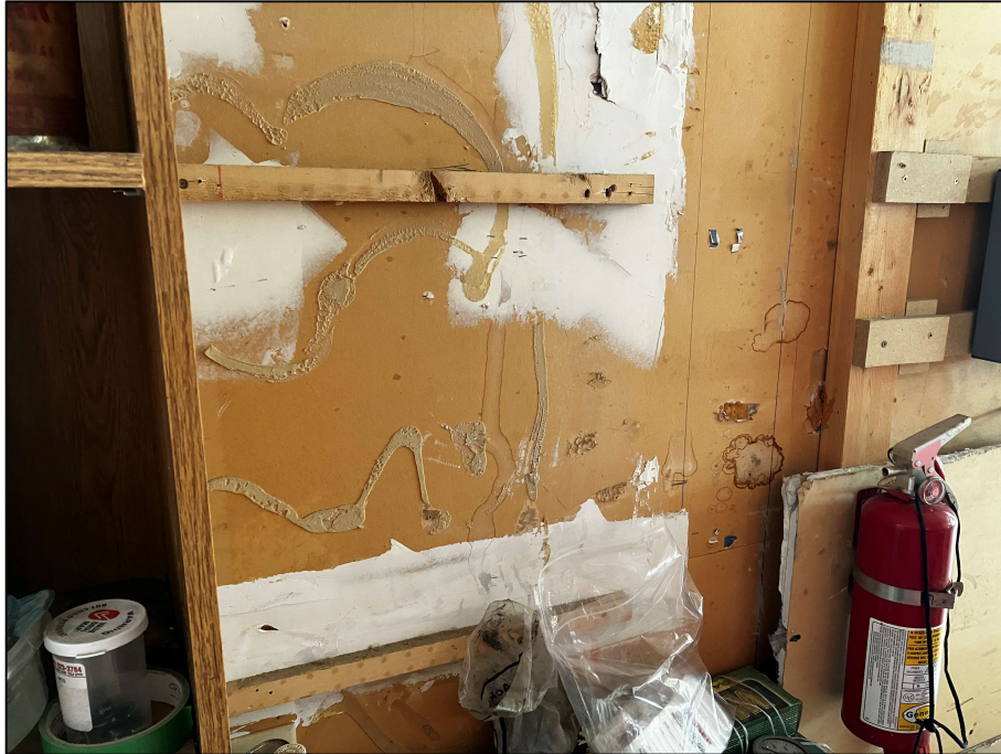
PHOTOGRAPH #9: Drywall Joint Compound - Level 1 Garage Interior (None Detected)
