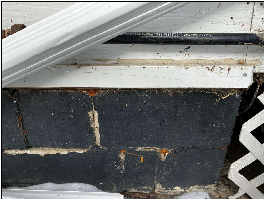
PHOTOGRAPH #22: Parging - Exterior of Home (None Detected)
