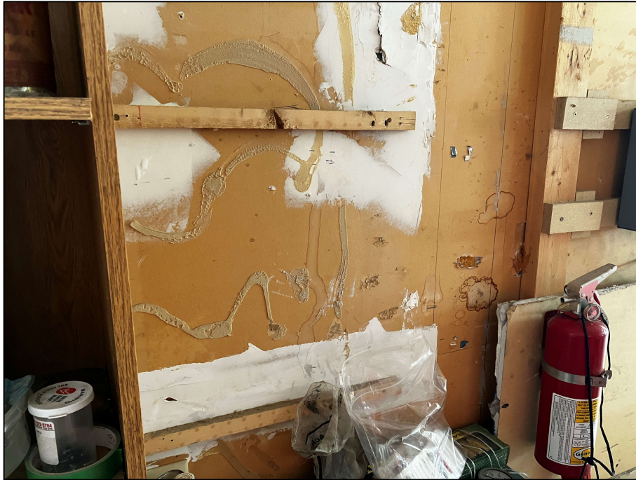
PHOTOGRAPH #34: Fire Extinguisher in Garage
