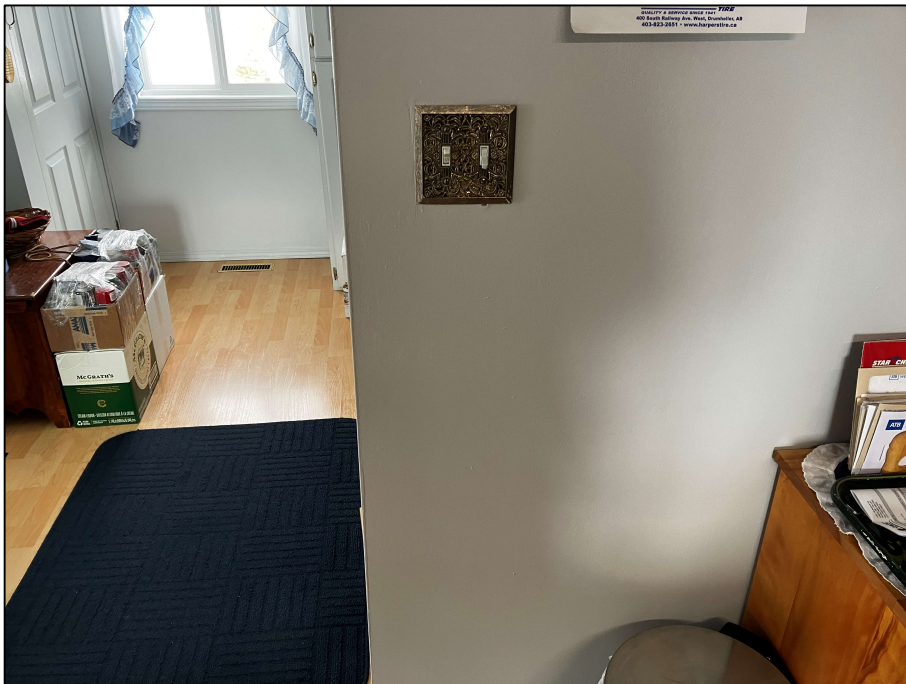
PHOTOGRAPH #2: Drywall Joint Compound - Level 1 Kitchen Interior (None Detected)
