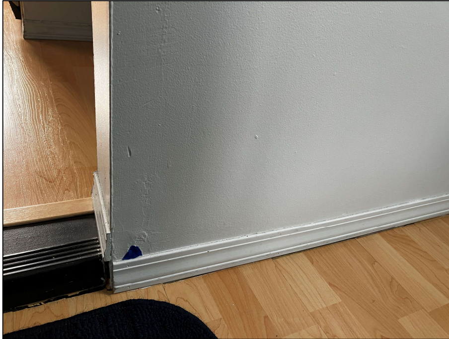
PHOTOGRAPH #7: Drywall Joint Compound - Level 1 Back Door Interior (None Detected)
