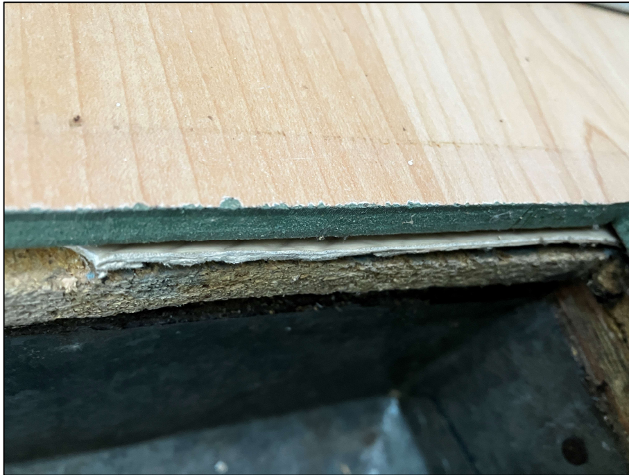
PHOTOGRAPH #15: Sheet Flooring - Level 1 Storage Room (None Detected)
