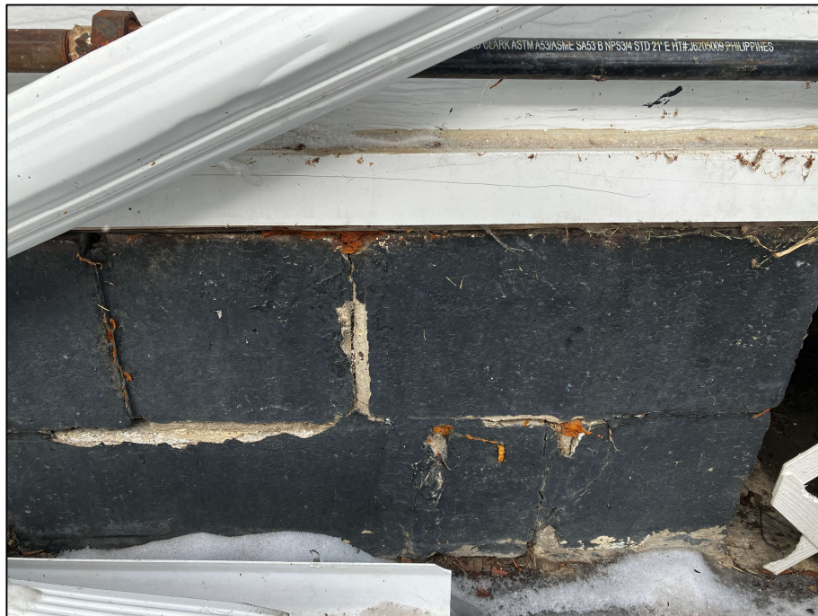
PHOTOGRAPH #26: Paint - Exterior of Home Black (510 ppm Lead)
