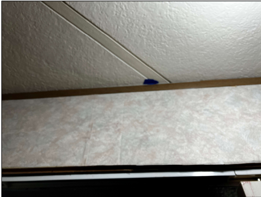
PHOTOGRAPH #11: Ceiling Tile - Level 1 Primary Bedroom Closet (None Detected)
