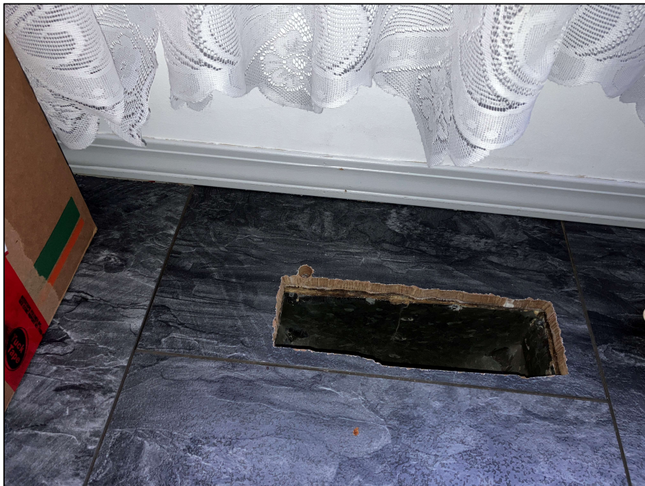
PHOTOGRAPH #16: Sheet Flooring - Level 1 Living Room (None Detected)
