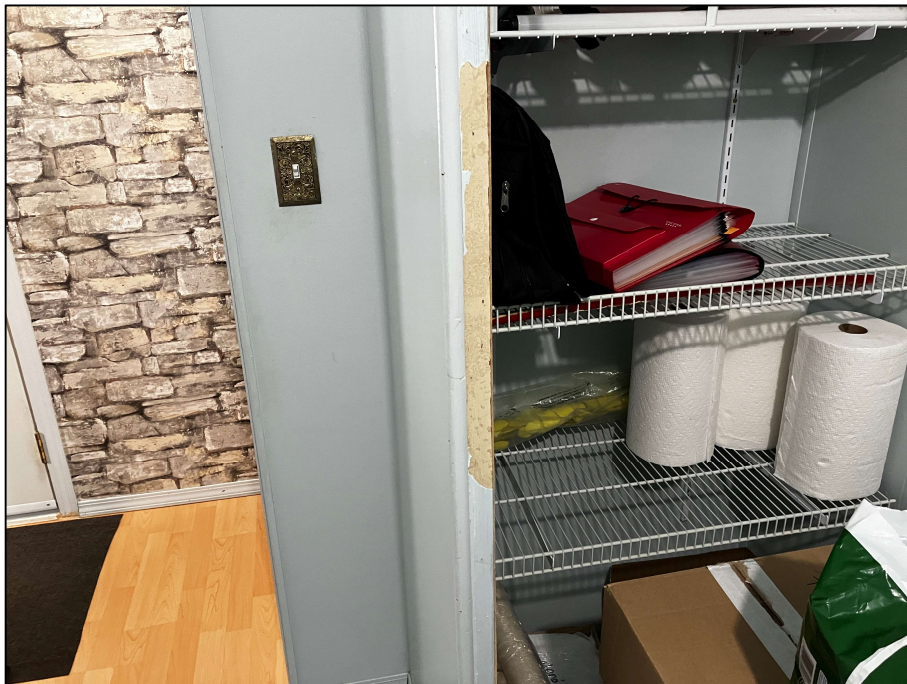
PHOTOGRAPH #24: Paint - Mud Room Light Blue (<80 ppm Lead)
