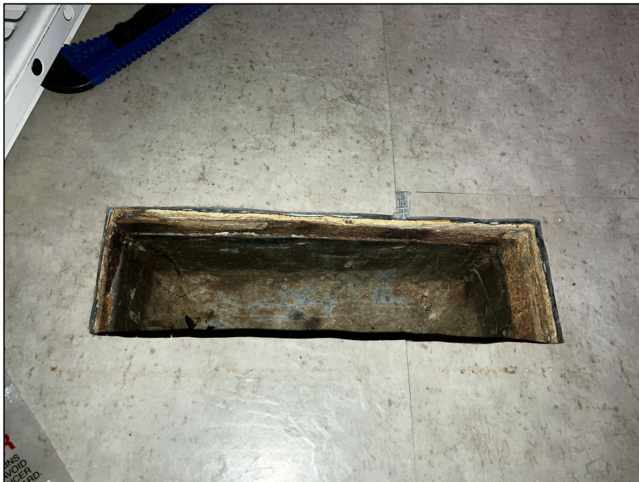
PHOTOGRAPH #18: Flooring - Level 1 Bathroom Layer 1 (None Detected)
