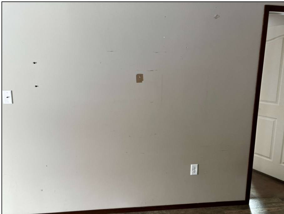
PHOTOGRAPH #6: Paint - Level 1 Dining Room Beige (<80 ppm Lead)
