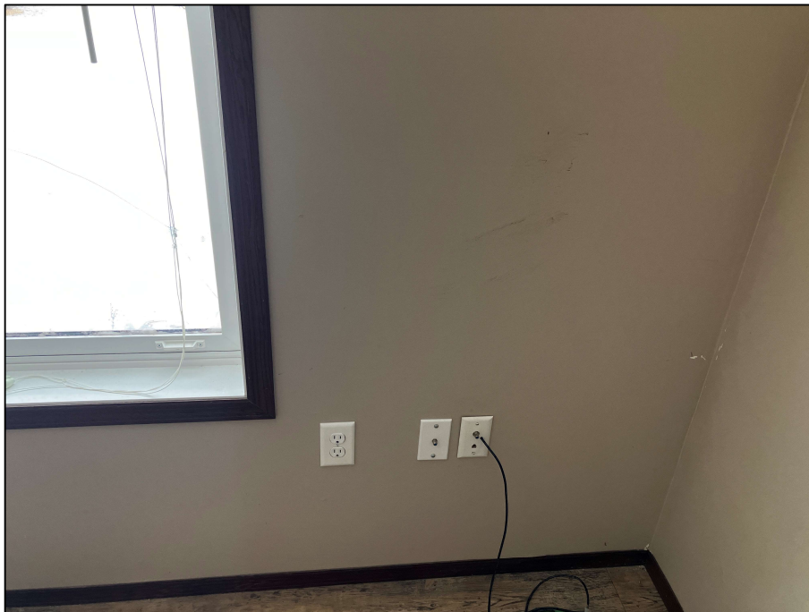
PHOTOGRAPH #4: Drywall Joint Compound - Level 1 NW Bedroom Interior (None Detected)
