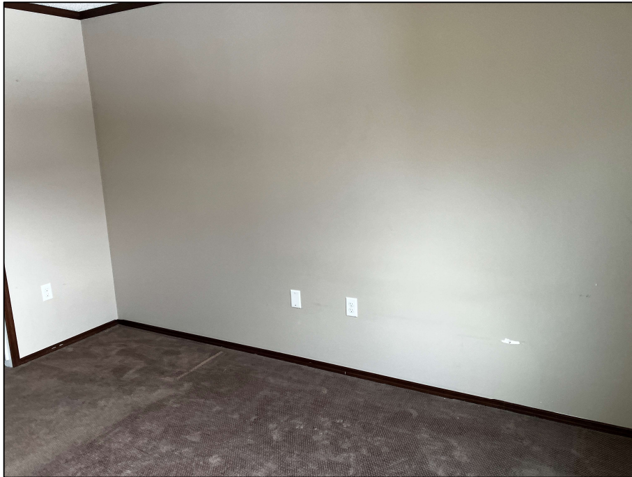
PHOTOGRAPH #1: Drywall Joint Compound - Level 1 Primary Bedroom Exterior (None Detected)
