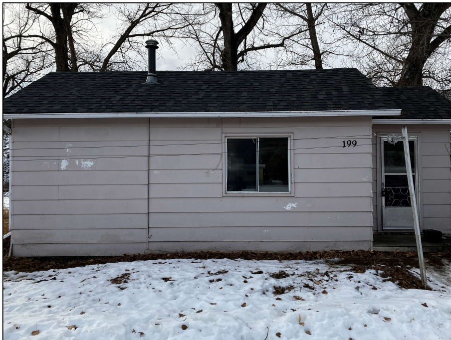
PHOTOGRAPH #20: Paint - Exterior Beige (<80 ppm Lead)
