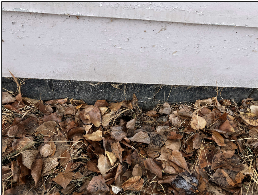
PHOTOGRAPH #16: Parging - Exterior (None Detected)
