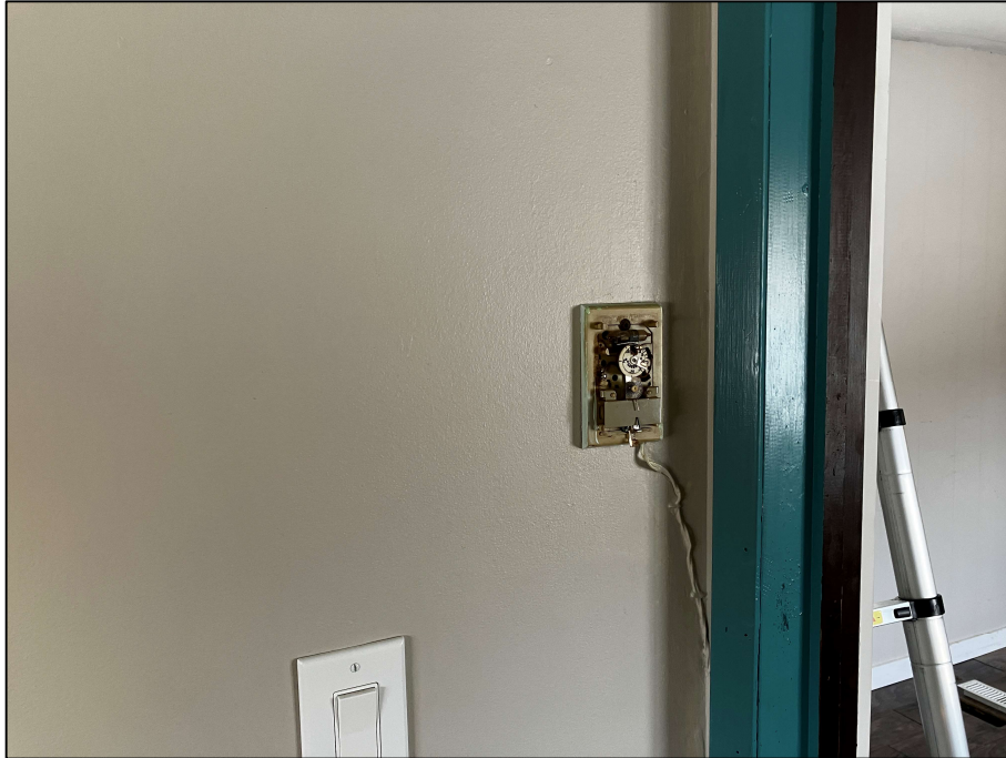
PHOTOGRAPH #30: Mercury Thermostat
