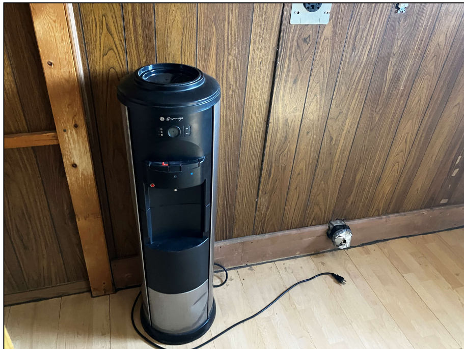
PHOTOGRAPH #27: Water Cooler with Ozone Deleting Substances
