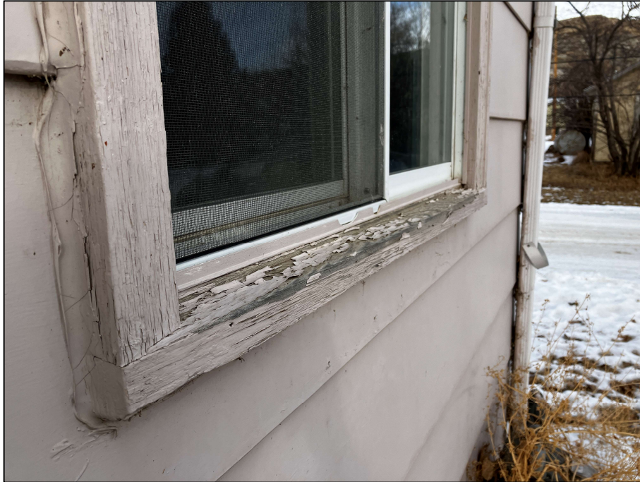
PHOTOGRAPH #17: Window Caulking - Exterior (None Detected)
