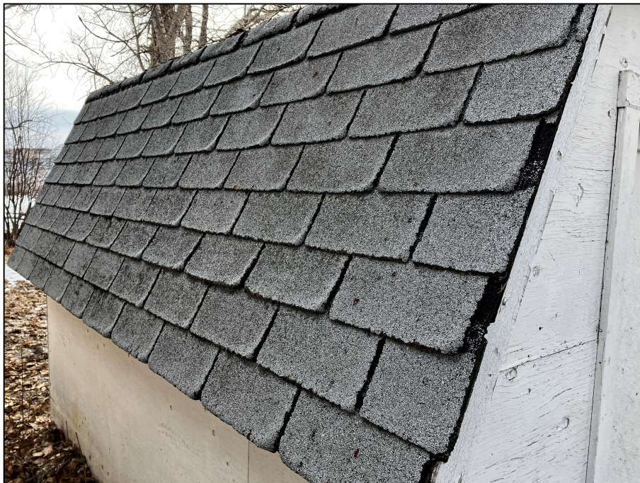
PHOTOGRAPH #14: Roof Shingle - Exterior Shed (None Detected)
