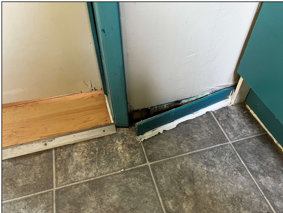
PHOTOGRAPH #12: Sheet Flooring - Level 1 Bathroom (None Detected)
