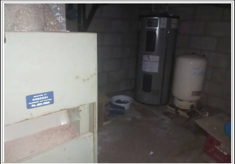
Utility Room Basement
