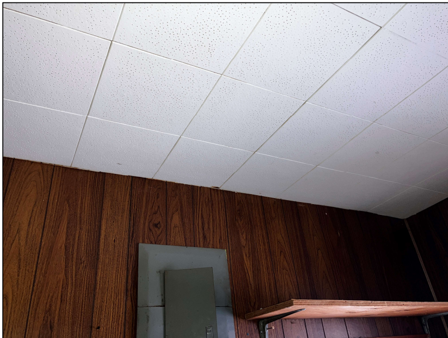
PHOTOGRAPH #10: Ceiling Tile - Level 1 Foyer (None Detected)
