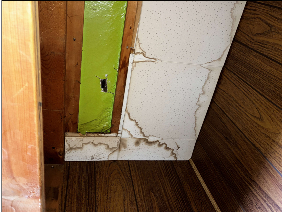
PHOTOGRAPH #11: Ceiling Tile - Level 1 Foyer (None Detected)
