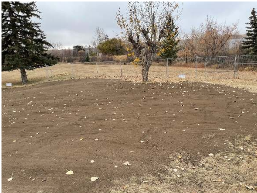
25 Roper Road – After Demolition and Cleanup
