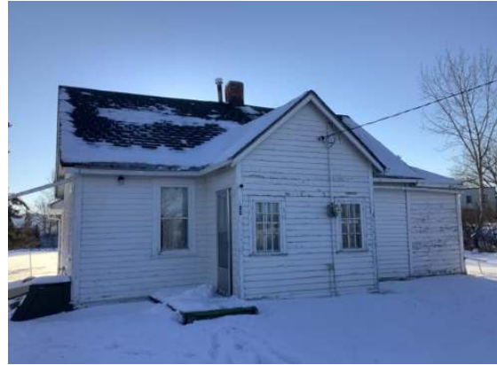
25 Roper Road – Prior to Demolition
