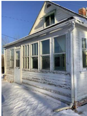
25 Roper Road – Prior to Demolition
