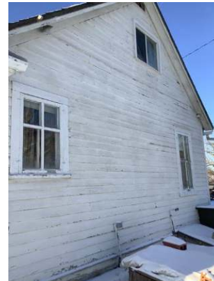
25 Roper Road– Prior to Demolition
