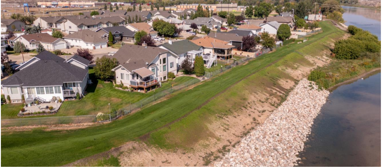
Willow Estates Berm – Construction Complete
